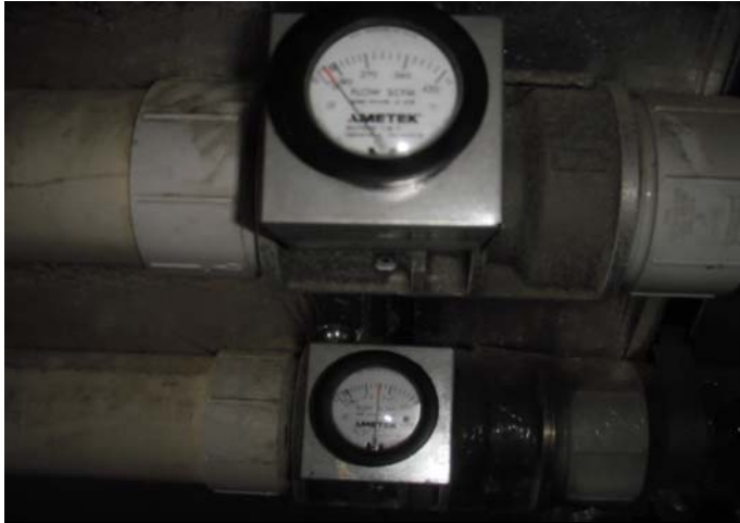
Picture 004 - View of the flow gauges within the System #1 trailer. Flow meter, FI-01, was gauged to read 90 SCFM.
