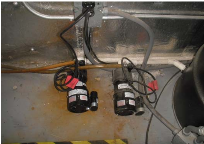
Picture 005 - The knock-out pumps within the System #1 trailer are functioning as indicated by the empty knock-out tanks.
