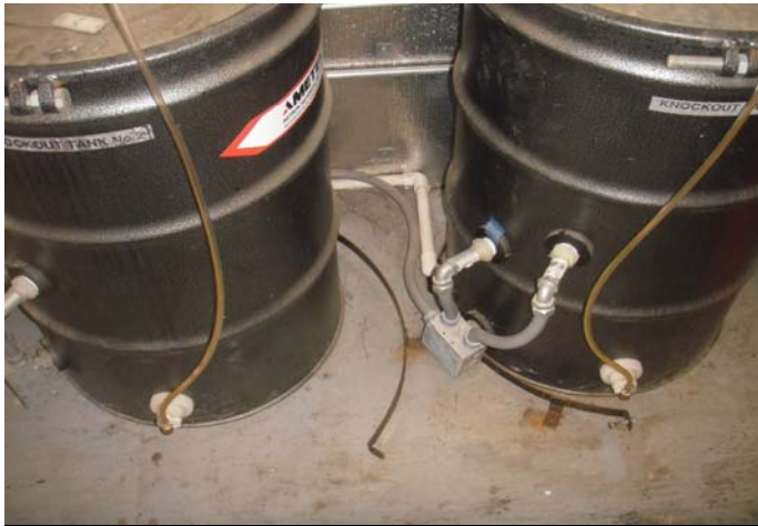
Picture 0019 - No water was observed in the site glasses of the knock-out tanks associated with System #1.
