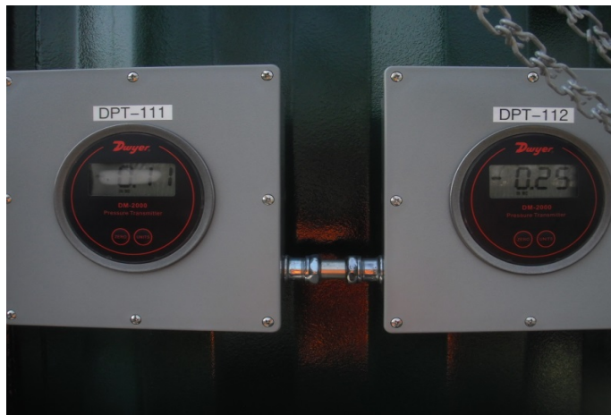
Picture 0035- Three (3) of the digital differential pressure gauges on the four (4)-inch injection lines were observed to be negative.
