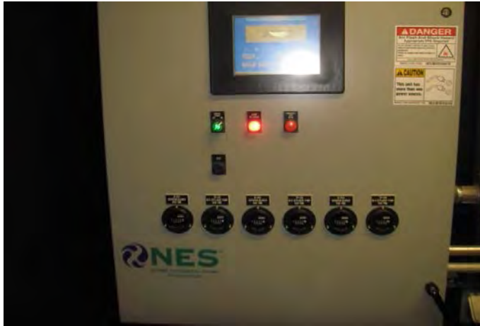
Picture 0074- Five (5) alarms were triggered on the control panel upon arrival.
