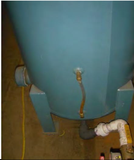
Picture P5090068 - No water was detected within the site glass of the knock-out tank.
