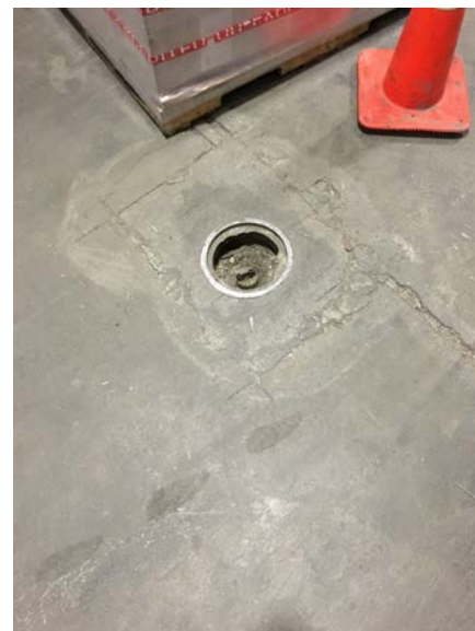
Missing well cap inside 1 Adams Blvd.
