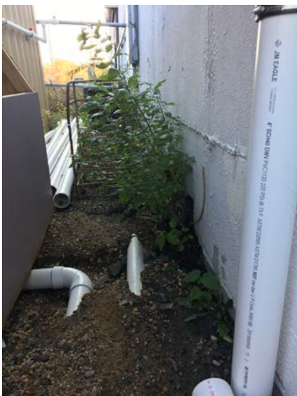
Erosion near SVE manifold
