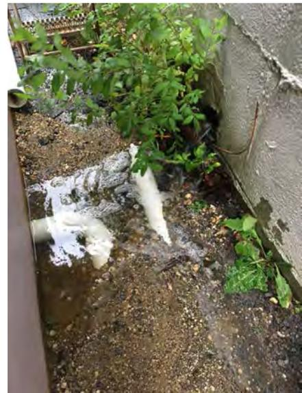
Water from roof drain ponding over horizontal well manifold
