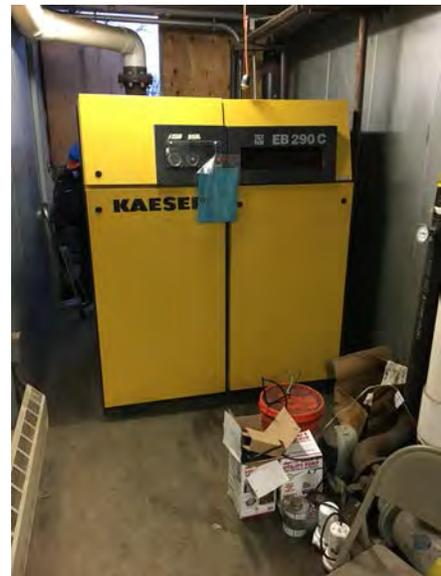
Blower in System #2 with faulty pressure gauge.
