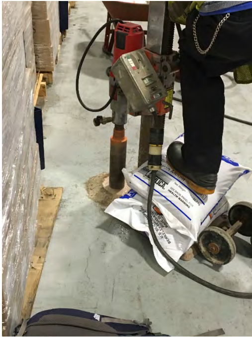
Concrete coring at ISB-01
