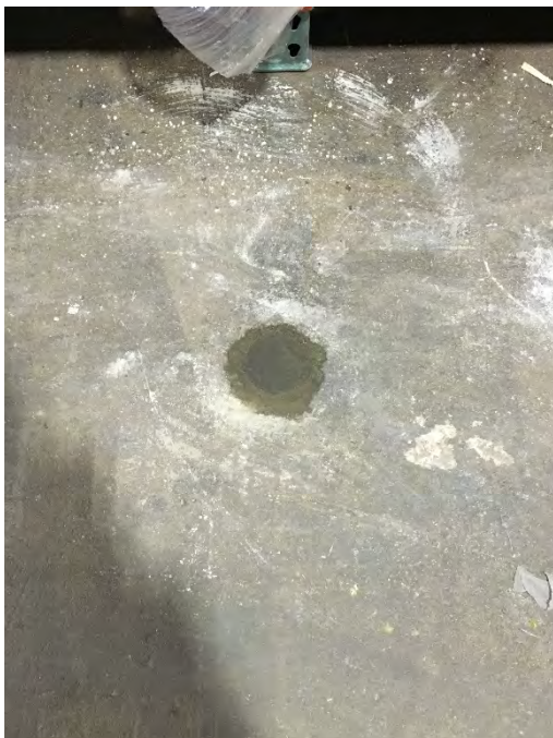
Example of abandoned soil boring
