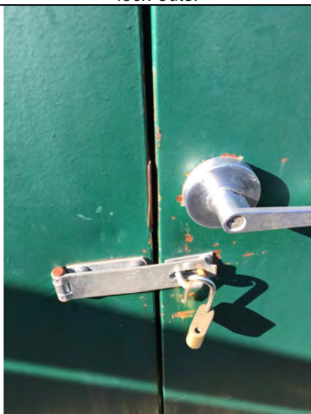
Door locked with exterior latch only – interior door latches removed.
