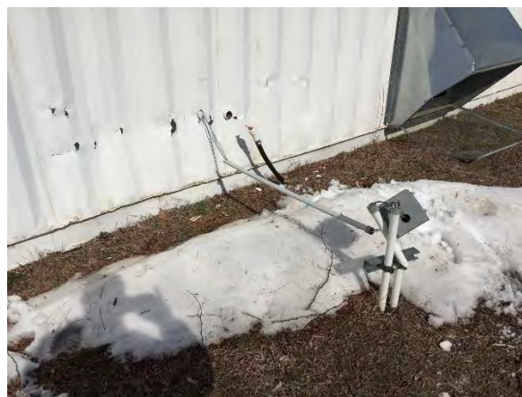
Damage to exterior of onsite DDC system #2 incurred in winter 2017. Snowplow collided with system trailer and damaged exterior electrical conduit.
