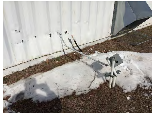
Damage to exterior of onsite DDC system #2 incurred in winter 2017. Snowplow collided with system trailer and damaged exterior electrical conduit.
