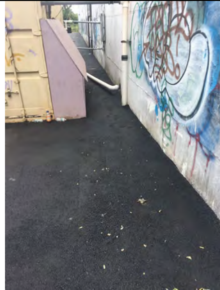
Paving completed behind 1 Adams boulevard building
