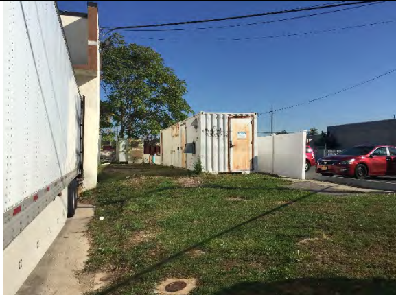
Onsite DDC System #1 trailer & general vicinity
