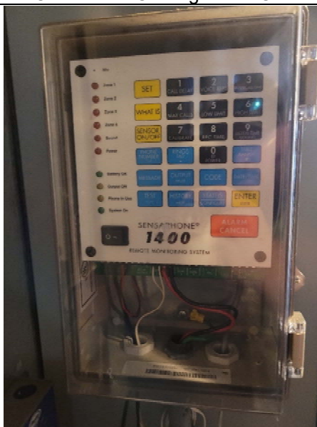
Sensaphone for DDC System #1 remains off
