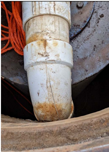
Cracked PVC fitting on DDC-2
