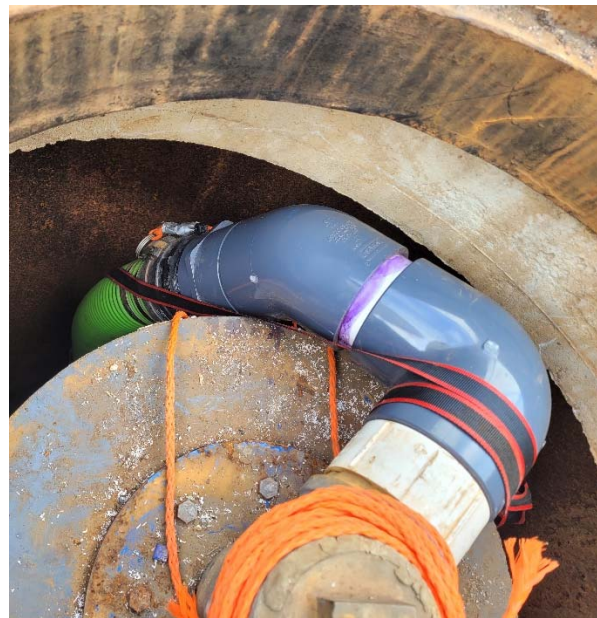
DDC-2 after replacing cracked PVC
