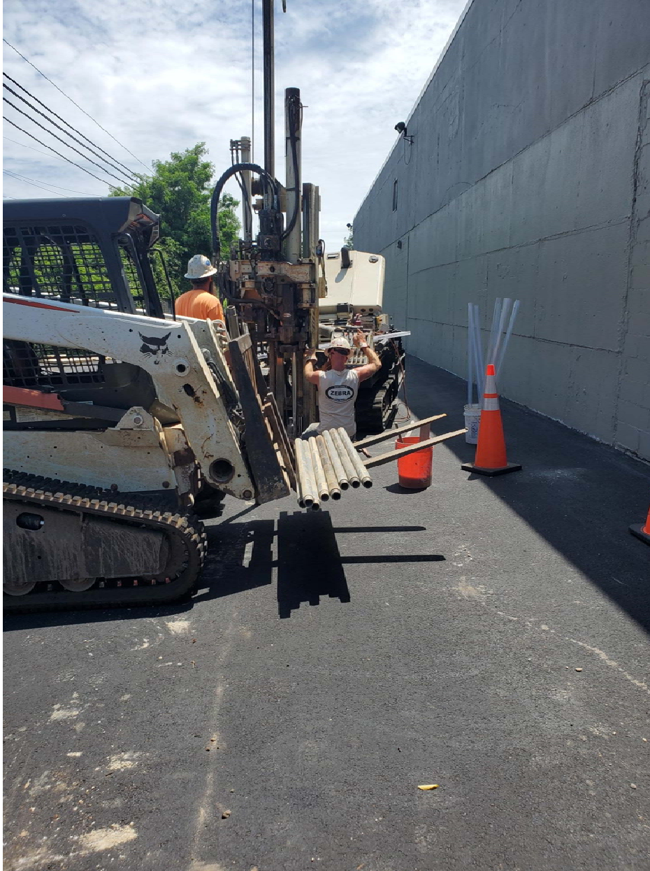
SB-01D: Soil boring SB-01D in progress
