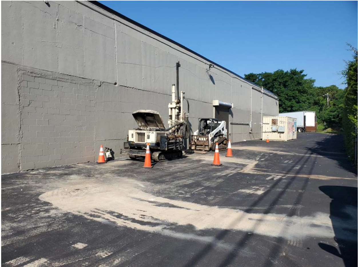
View of where soil borings SB-01B, SB-01C, SB-01D were conducted.
