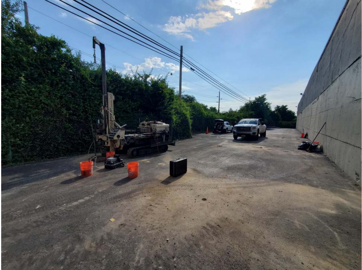
Purging at SPC-01BN-84.
