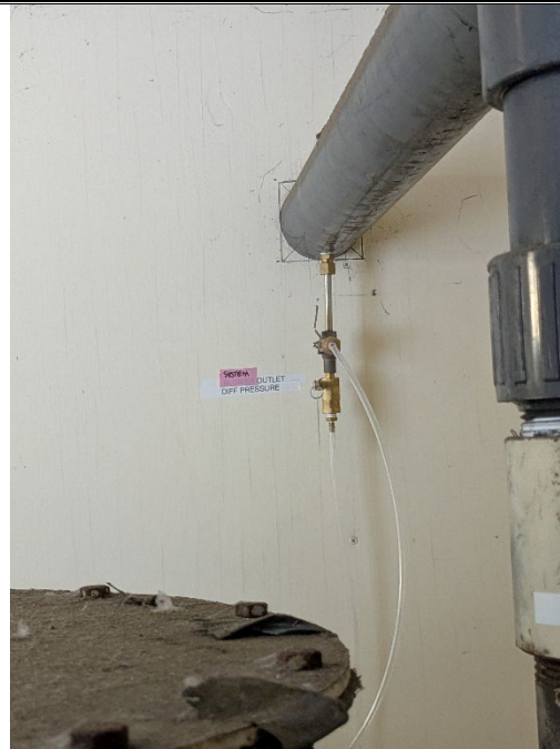
Pitot Tube on outlet piping from second carbon vessel (discharge line / system effluent) renamed as System Outlet Differential Pressure for clarity.
