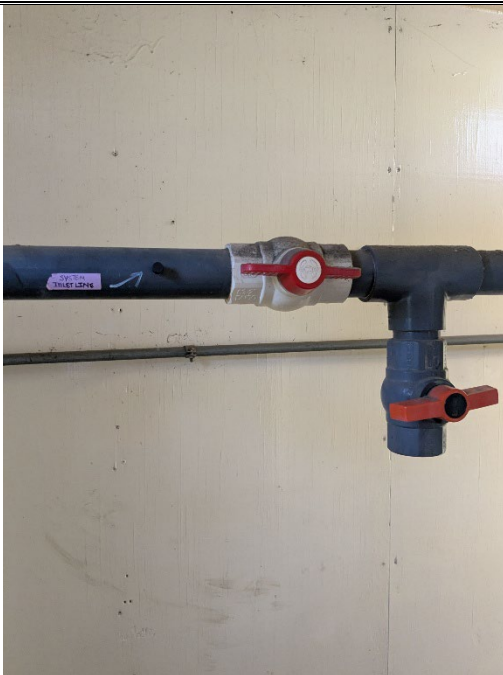
System Inlet Port before blower and dilution Valve to collect flow, PID, and temp readings as needed.
