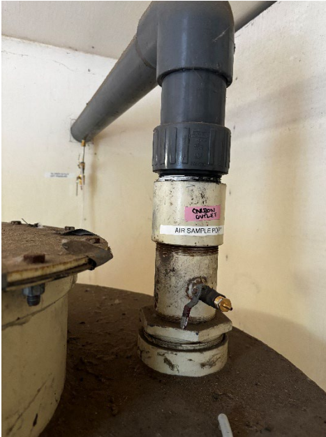
Carbon treatment effluent sample port
