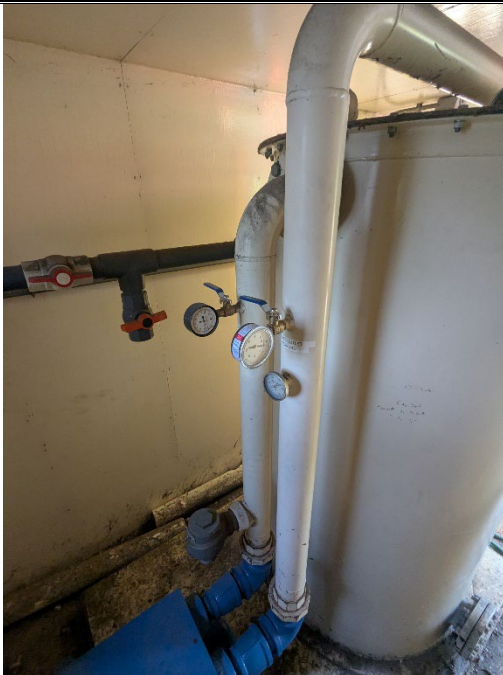
Vacuum and Pressure Gauges added to ball valve ports on Blower Inlet and Outlet lines
