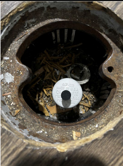
New vapor point caps installed inside 1 Adams Blvd for better reading collection
