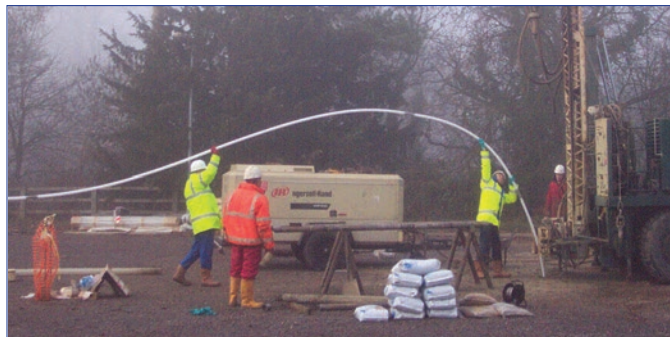
CMT Installation at UK Chlorinated Solvents Site (Source: Waterra. UK)
