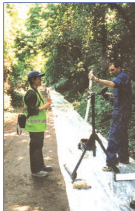
CMT System installed to a 60 m (200 ft) depth with seven monitoring zones. Installation was completed by placing layers of sand and bentonite to monitor a BTEX/MTBE plume in a Chalk aquifer, United Kingdom.
