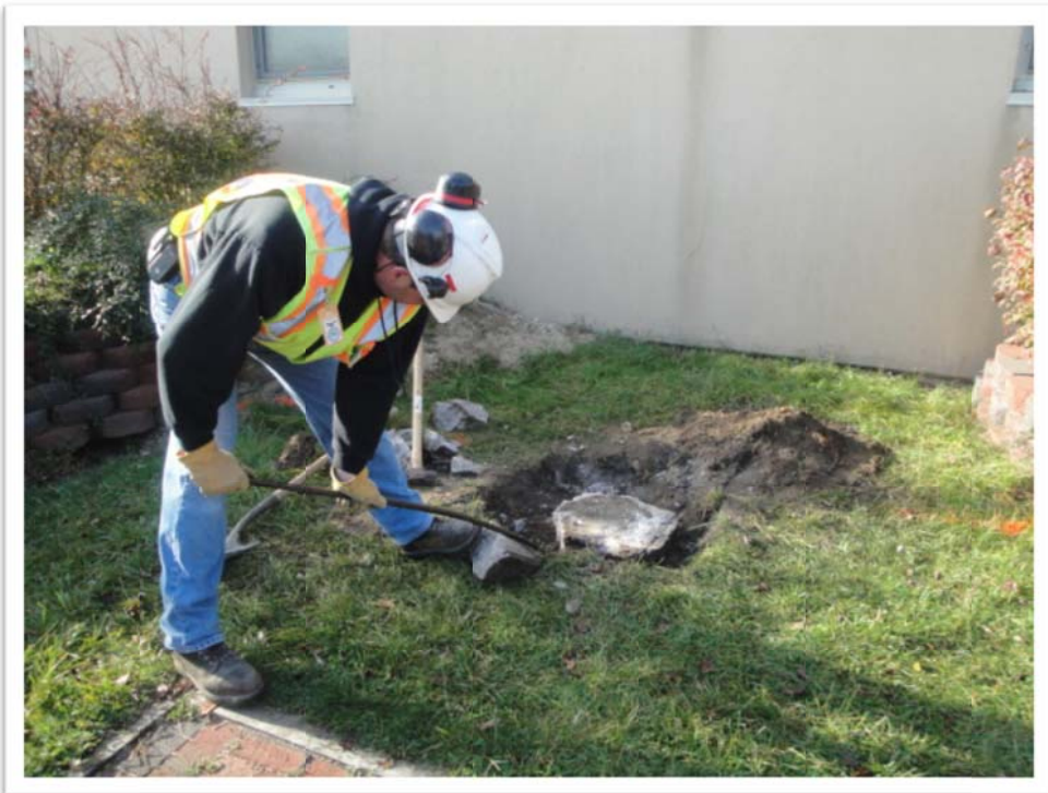
Digging up the Concrete Pad for Well S2-MW02
