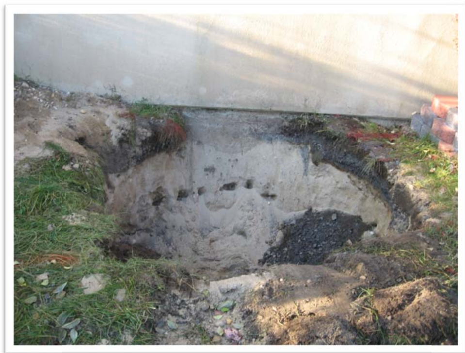
Open Excavation After Confirmation Sampling
