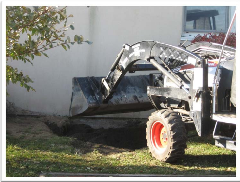
Backfilling the Excavation
