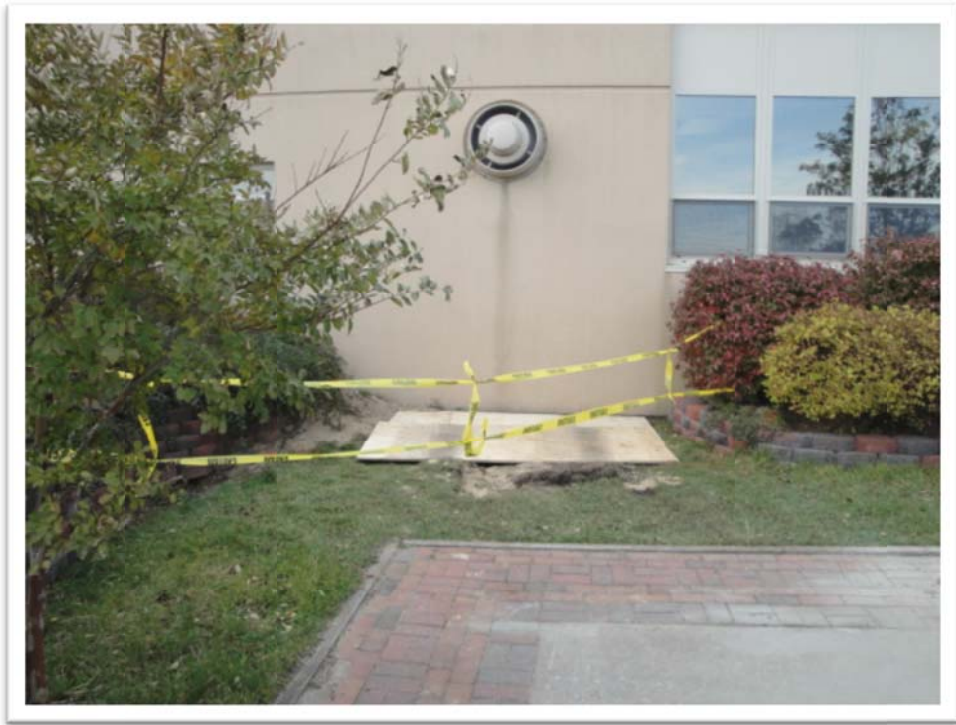
Securing the Excavation
