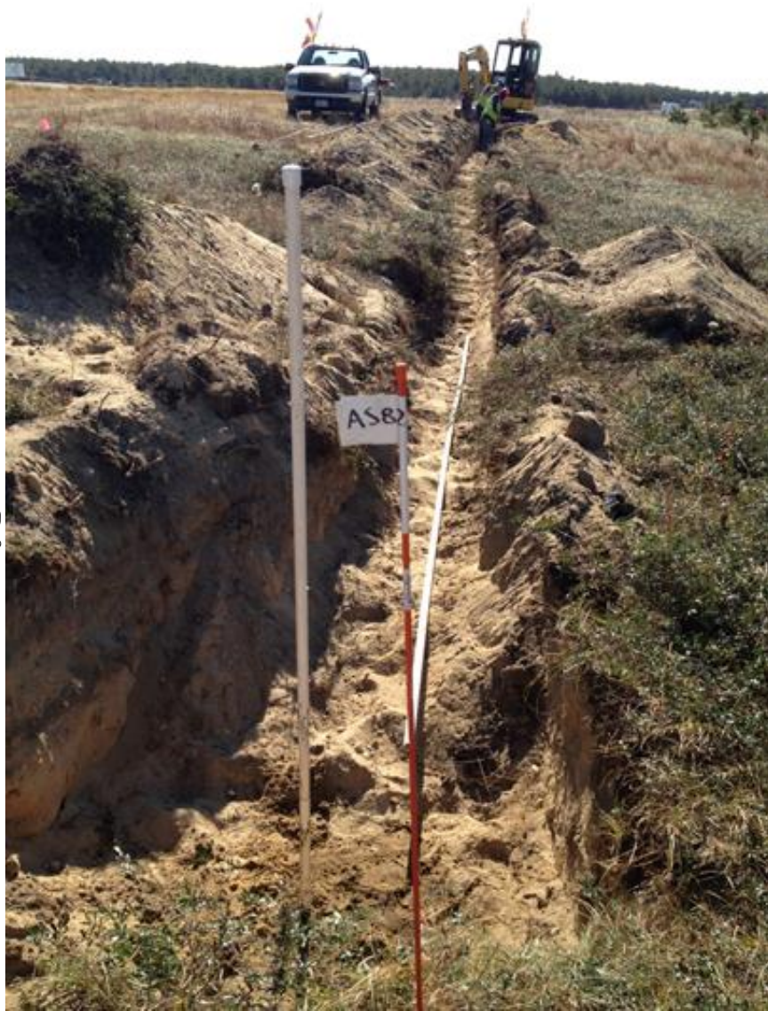
13. Trench to New AS-P2 Sparge Well
