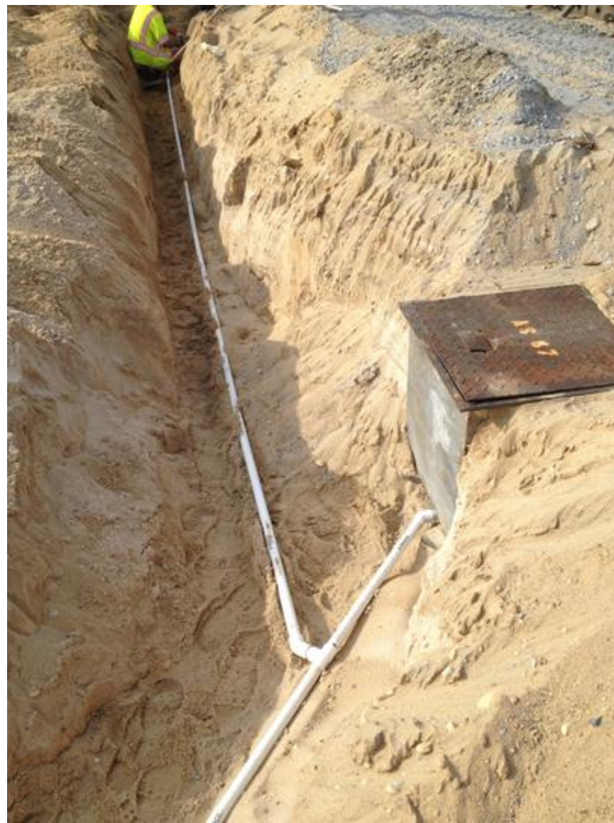
26. PVC Piping Installation to AS-66 and AS-67 Sparge Well
