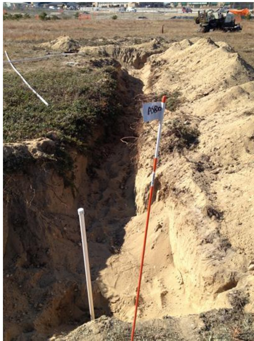
12. Trench to New AS-P2 Sparge Well
