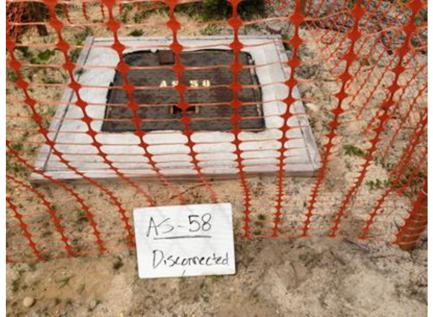
4. Valve Vault Protective Measure Example
