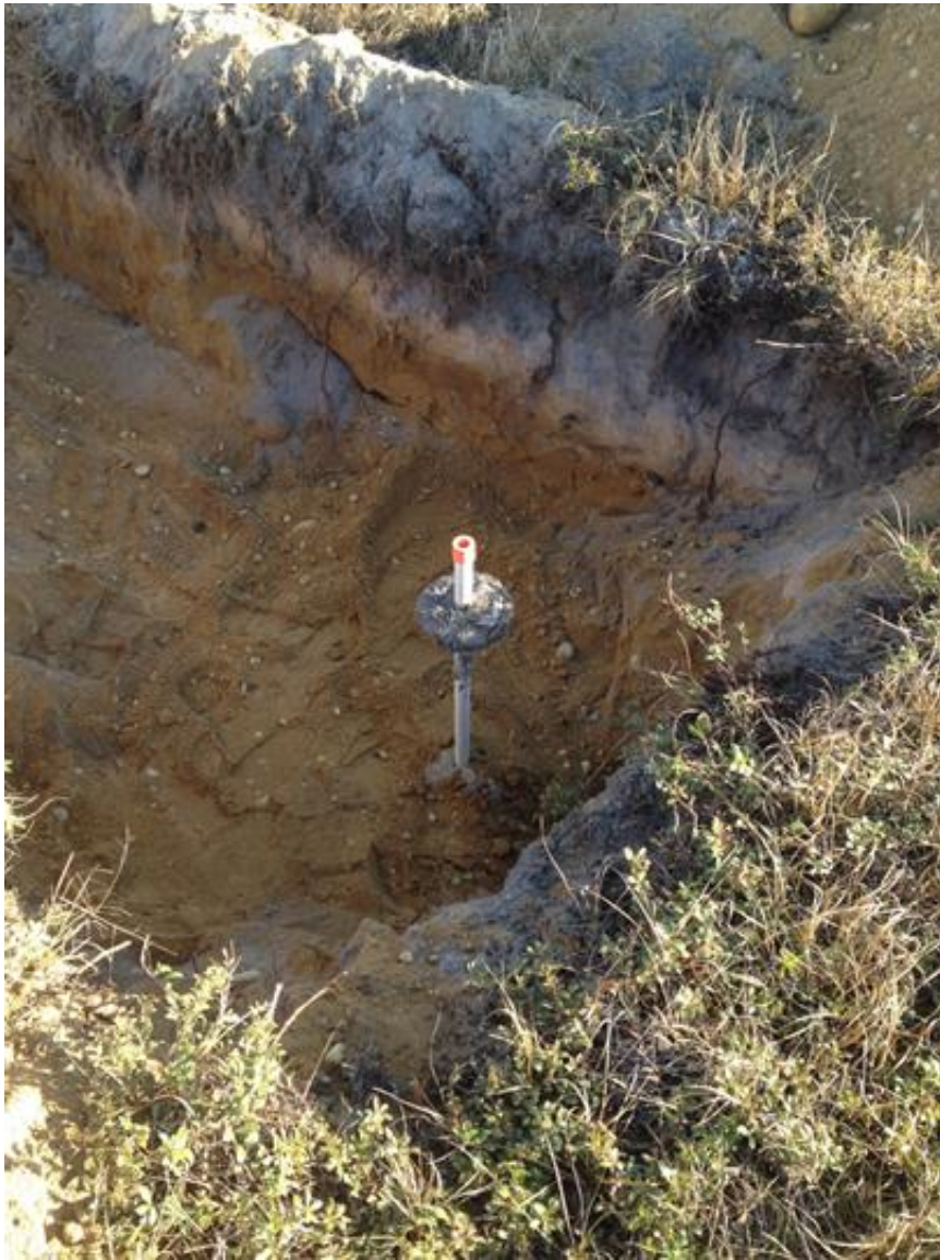
9. Trench to New AS-78 Sparge Well
