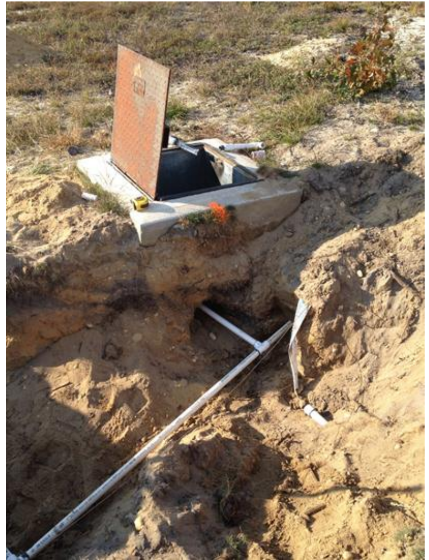
18. PVC Piping Installation at AS-P2 Sparge Well
