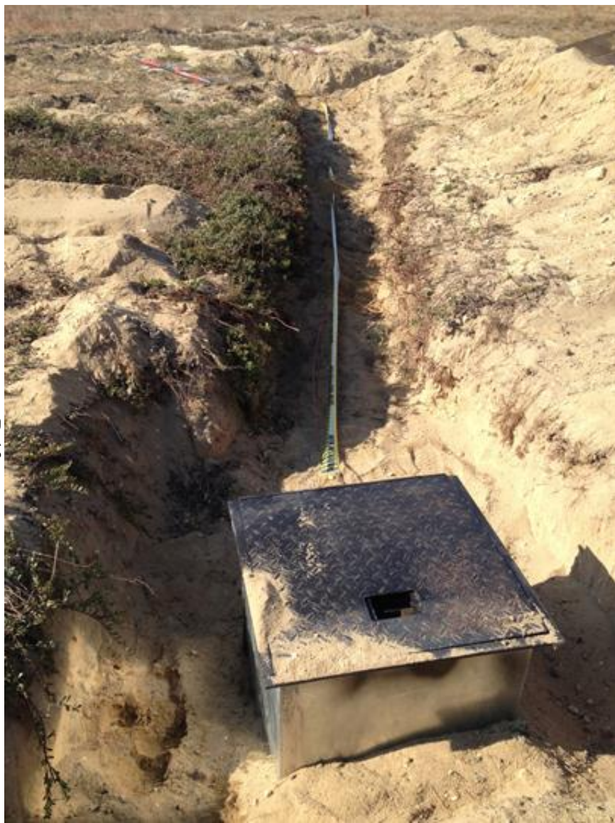
21. Vault Placement at AS-78 Sparge Well
