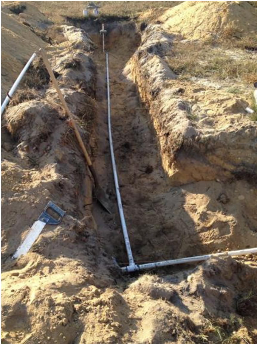
17. PVC Piping Installation to AS-78 Sparge Well
