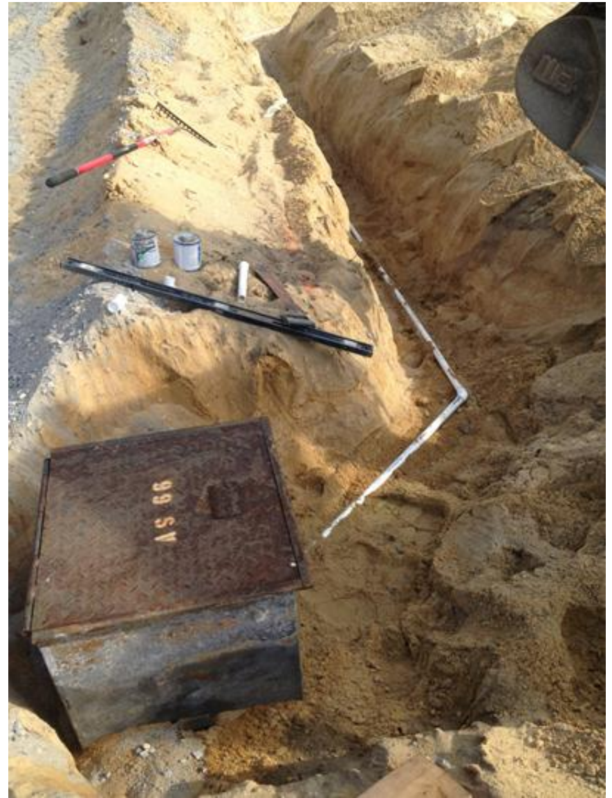
28. Vault Placement at AS-66 Sparge Well
