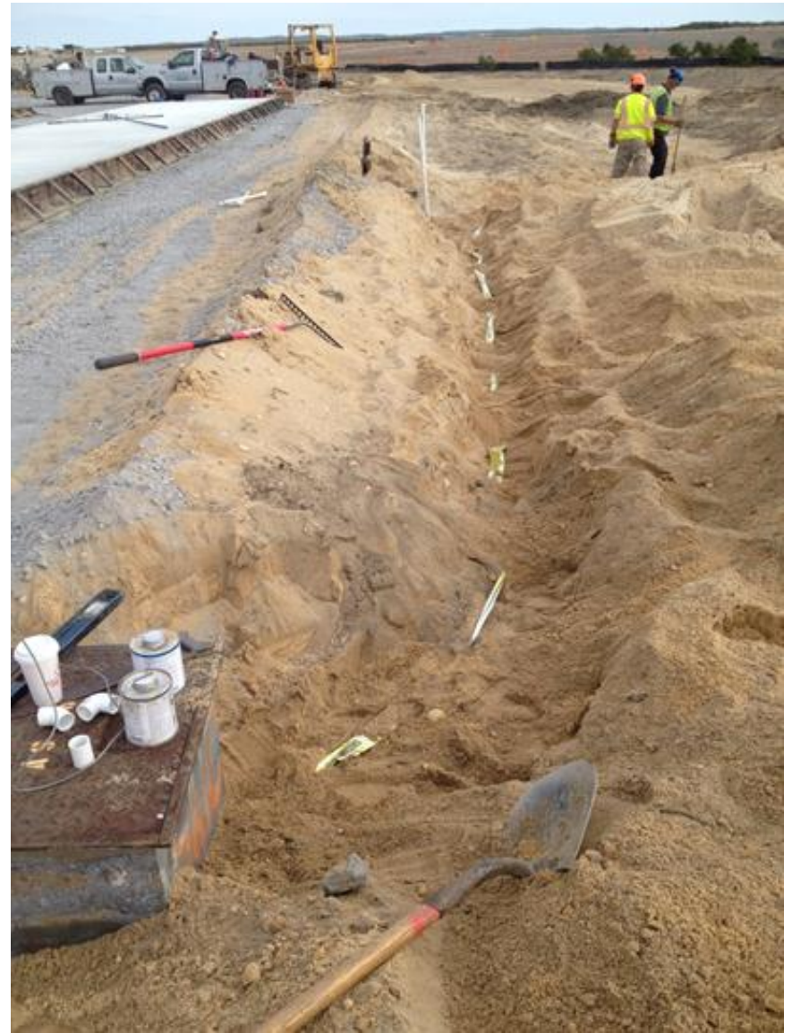
30. Utility Locate Wire Installation at AS-66
