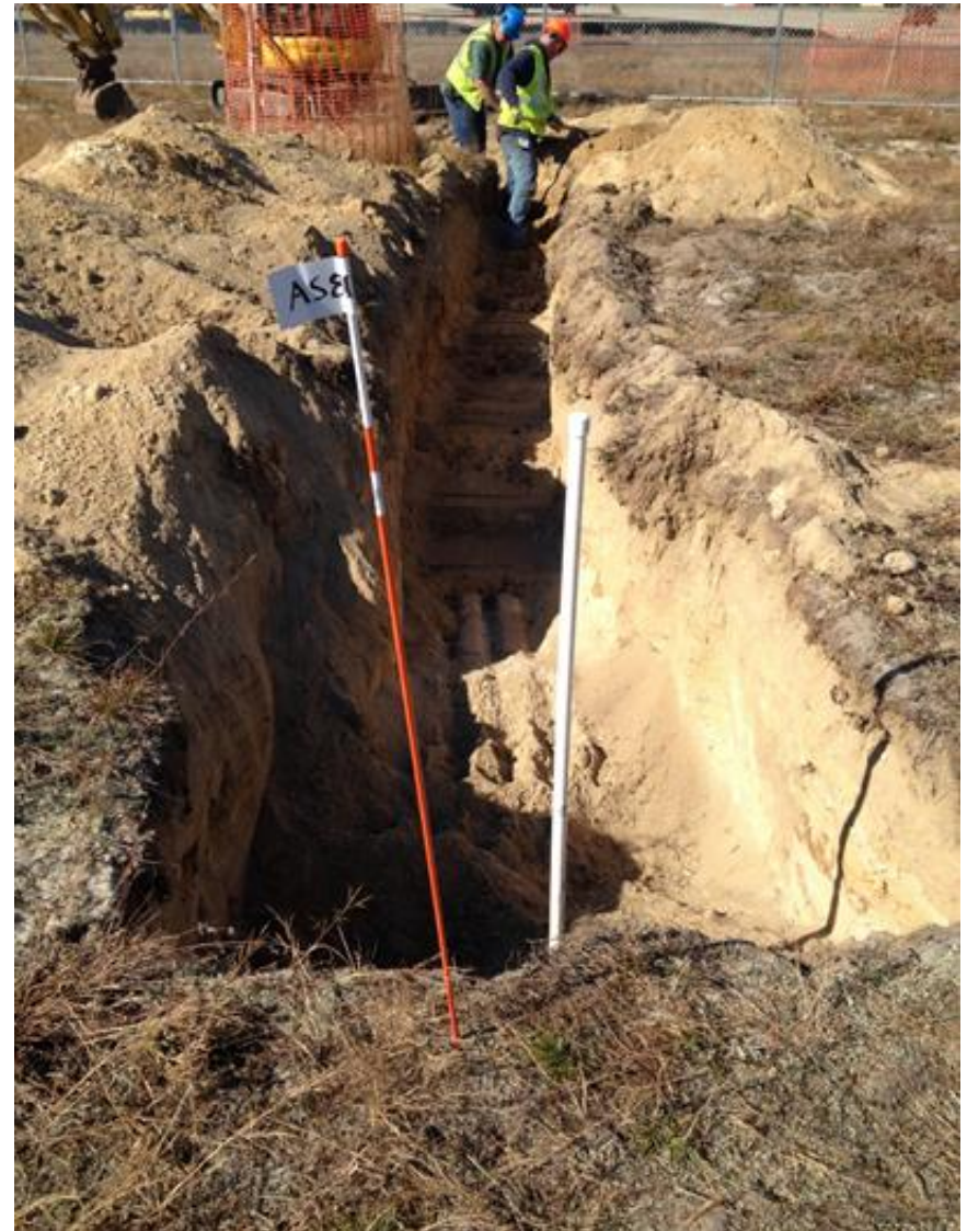
10. Trench to New AS-81 Sparge Well
