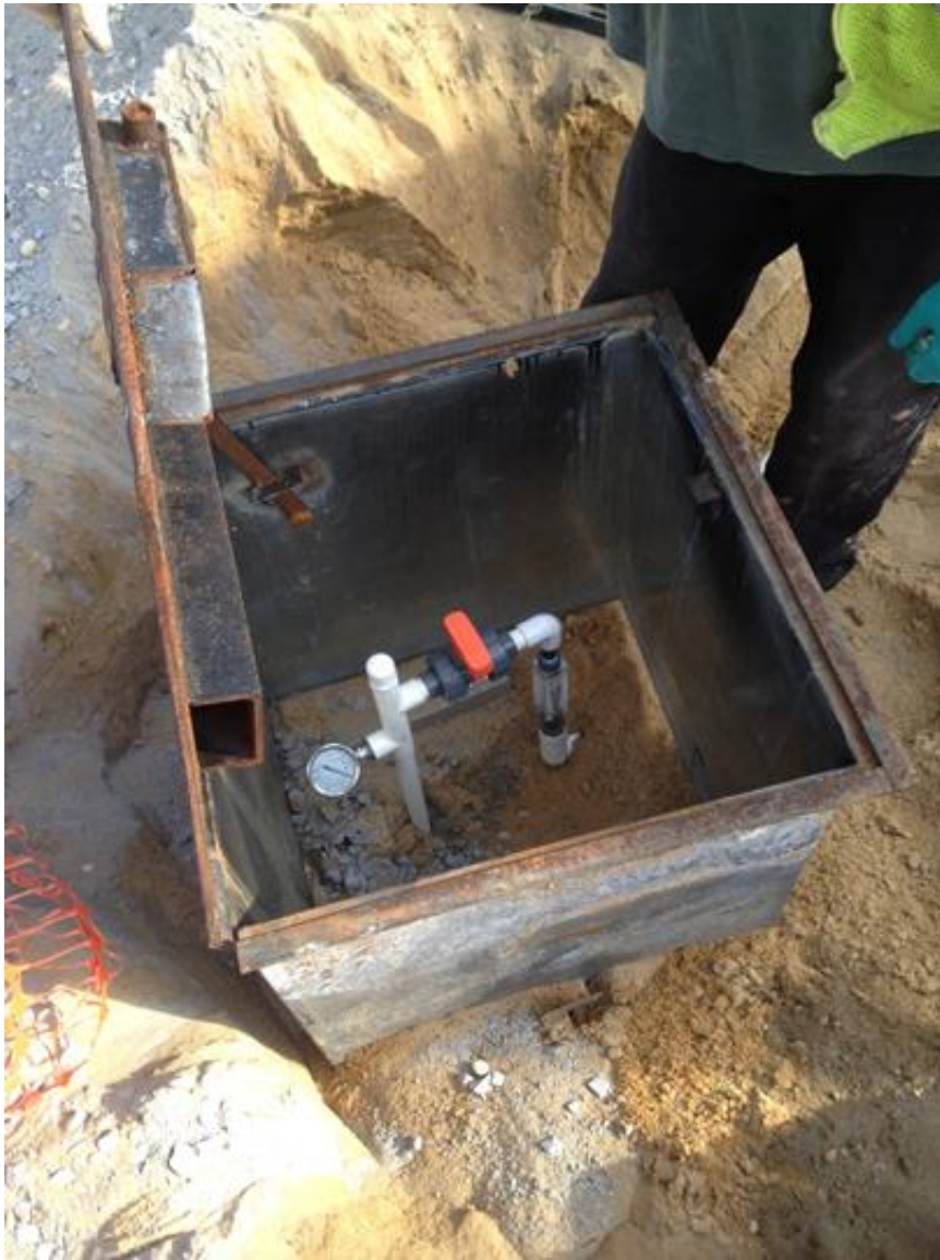
27. Vault Placement at AS-66 Sparge Well
