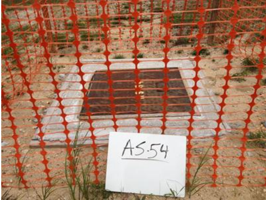
3. Valve Vault Protective Measure Example
