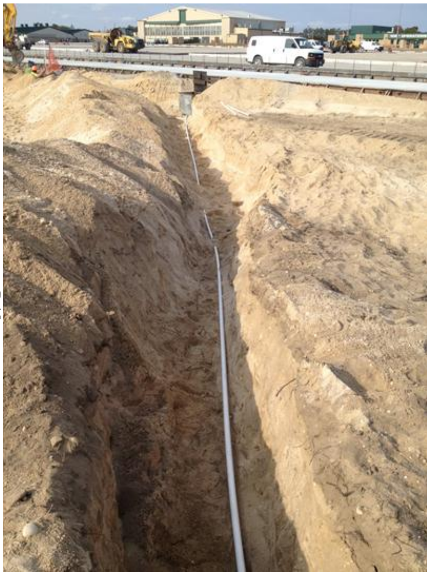
25. PVC Piping Installation to AS-67 Sparge Well
