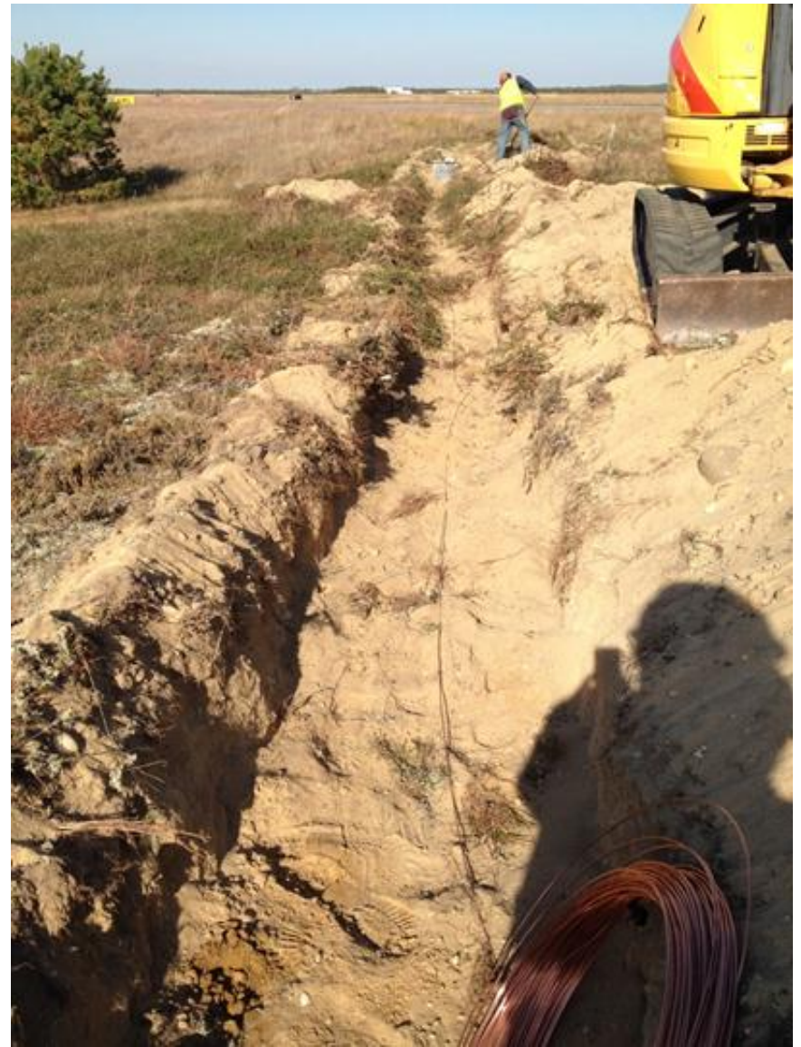
14. Utility Locate Wire Installation
