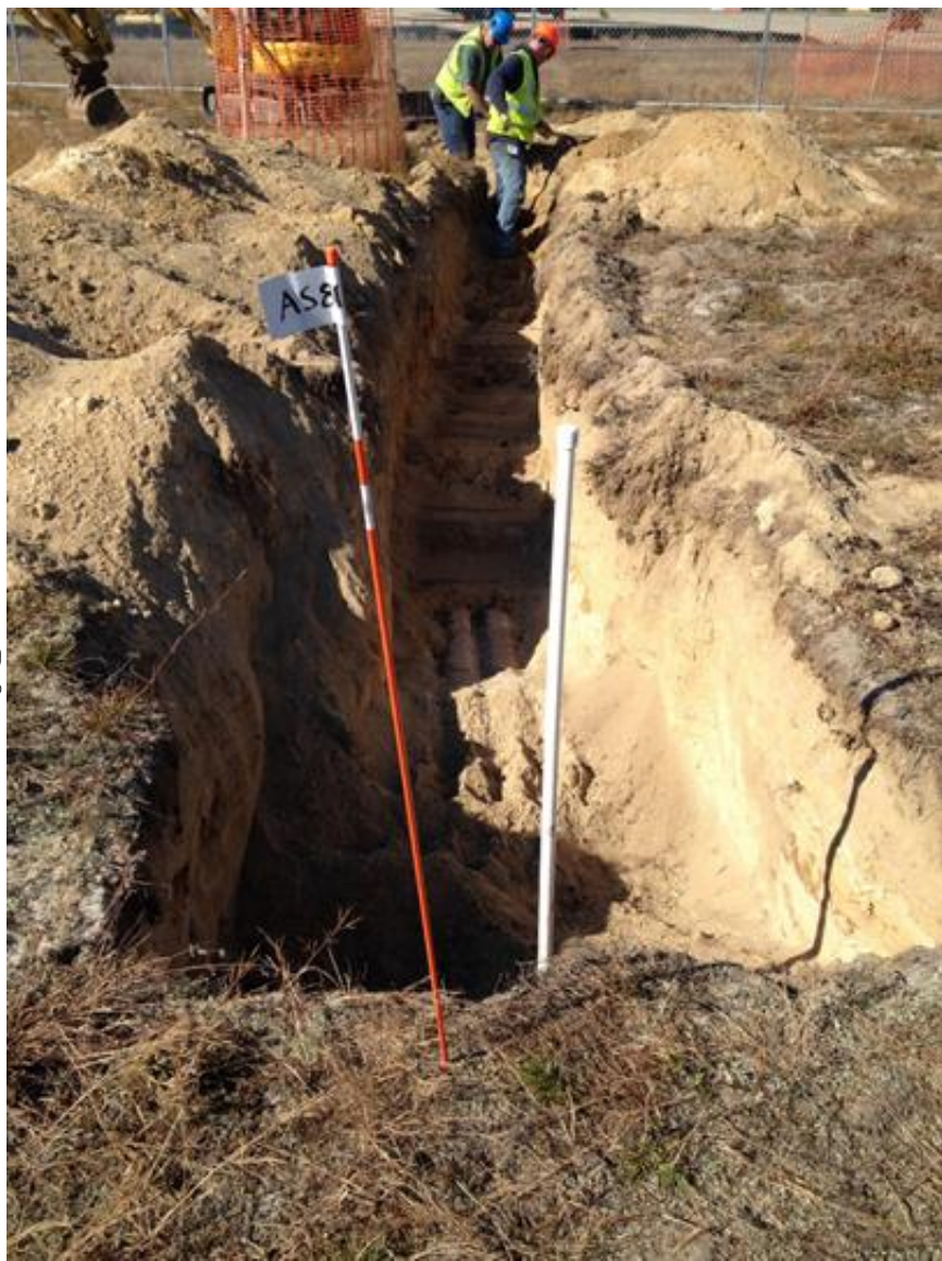
11. Trench to New AS-81 Sparge Well
