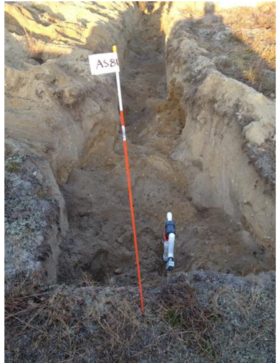
16. PVC Piping Installation at AS-81 Sparge Well
