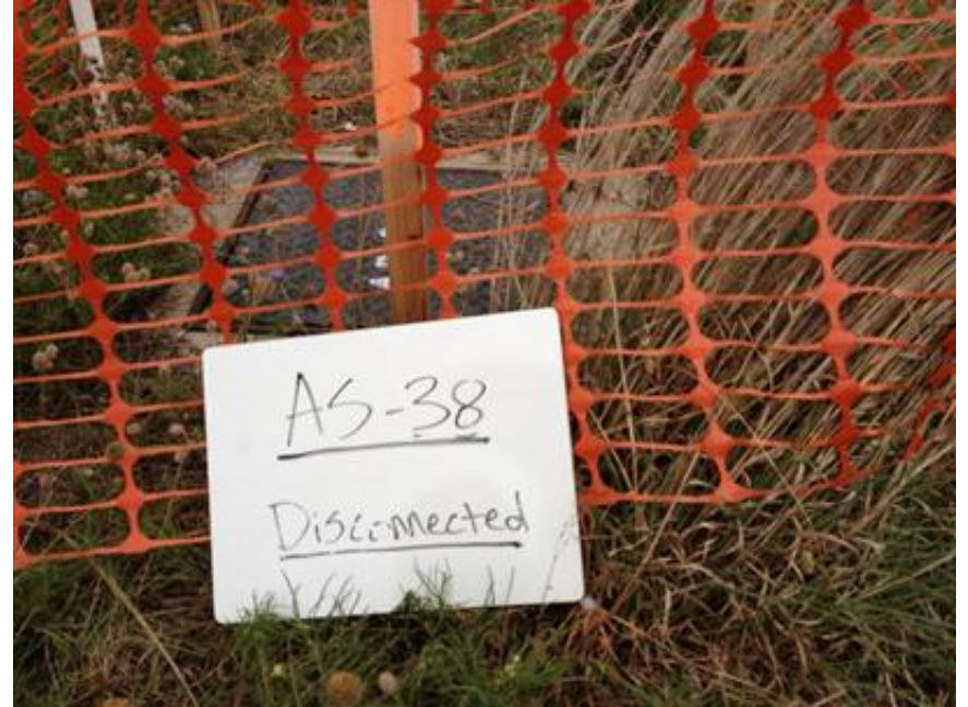
2. Valve Vault Protective Measure Example
