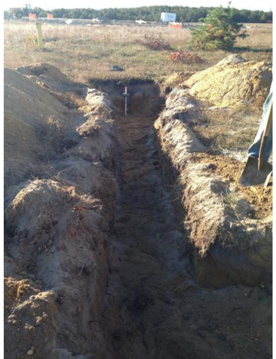
8. Trench to New AS-78 Sparge Well
