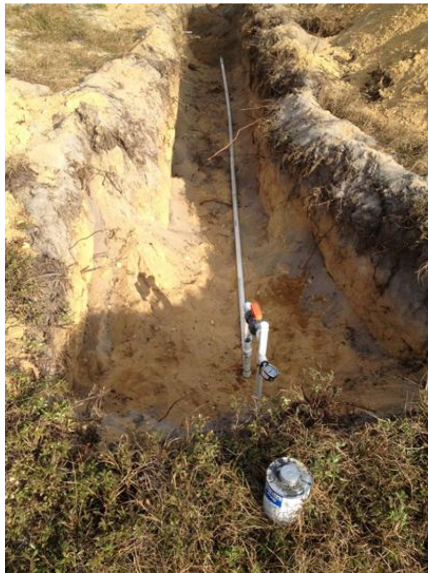
20. PVC Piping Installation at AS-78 Sparge Well
