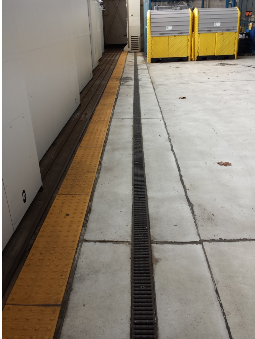
Photo 6: Trench drains were present in Hangar 370.
