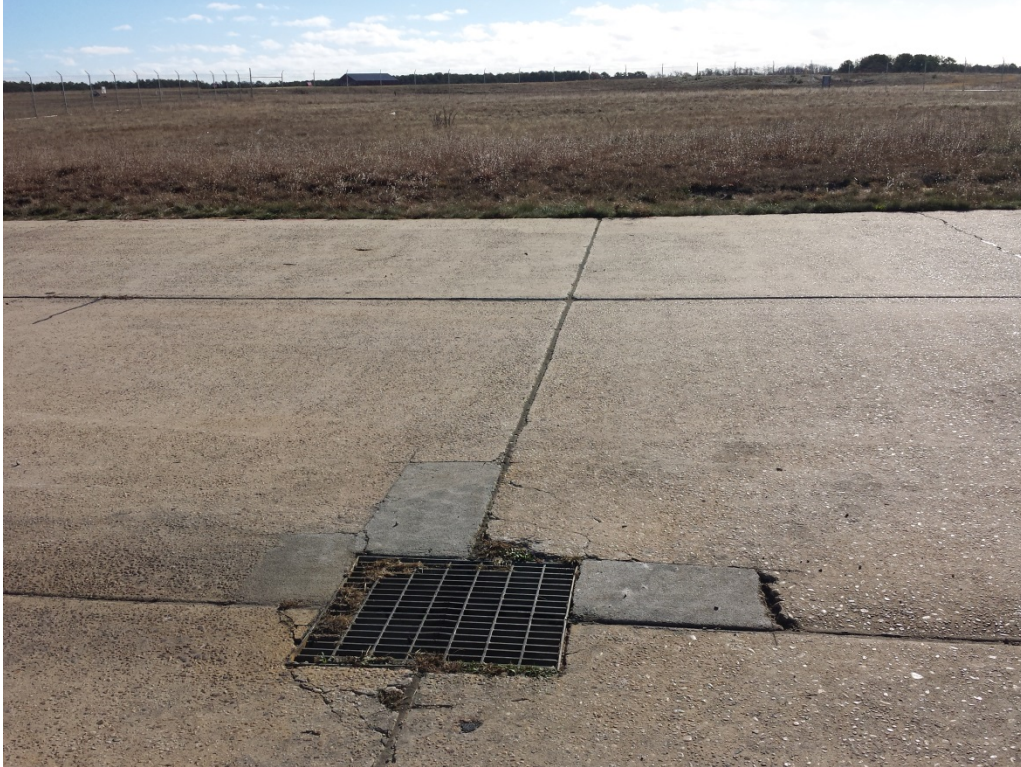
Photo 3: Drains were present on the apron.
