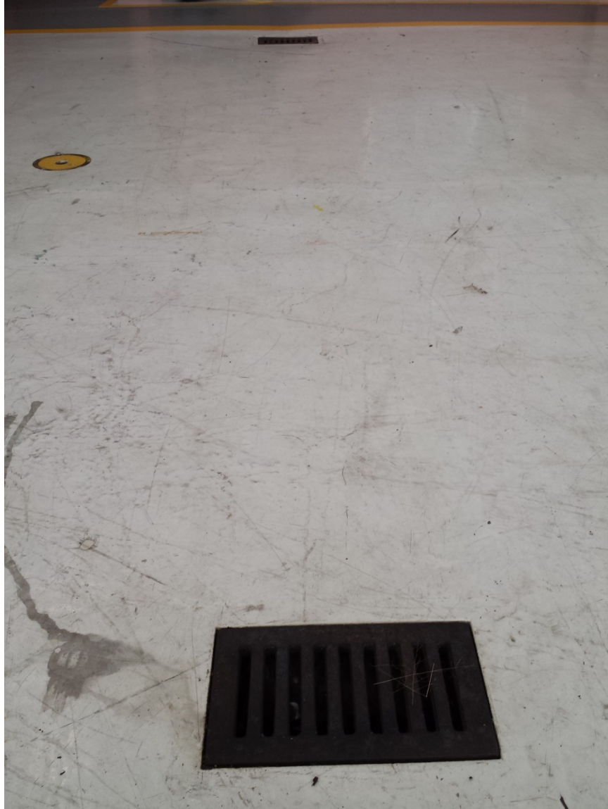
Photo 5: Floor drains were present in Hangar 358.
