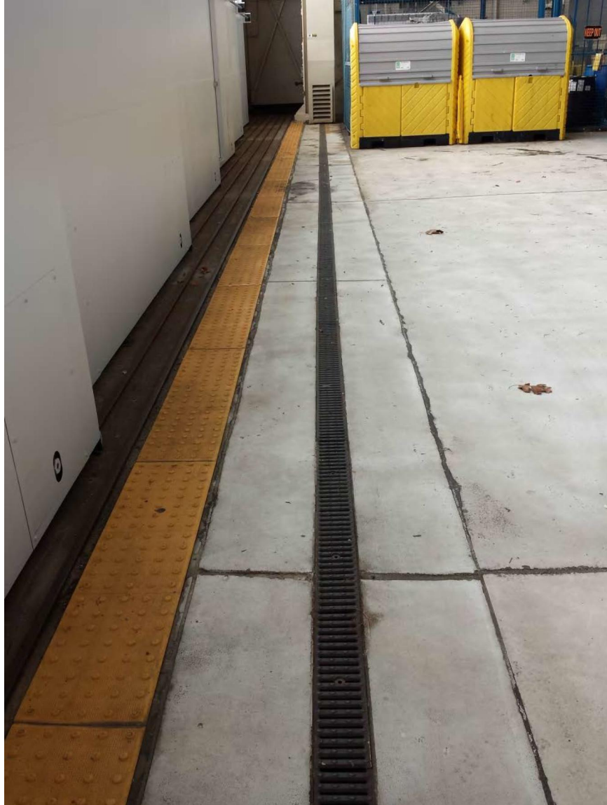
Photo 6: Trench drains were present in Hangar 370.
