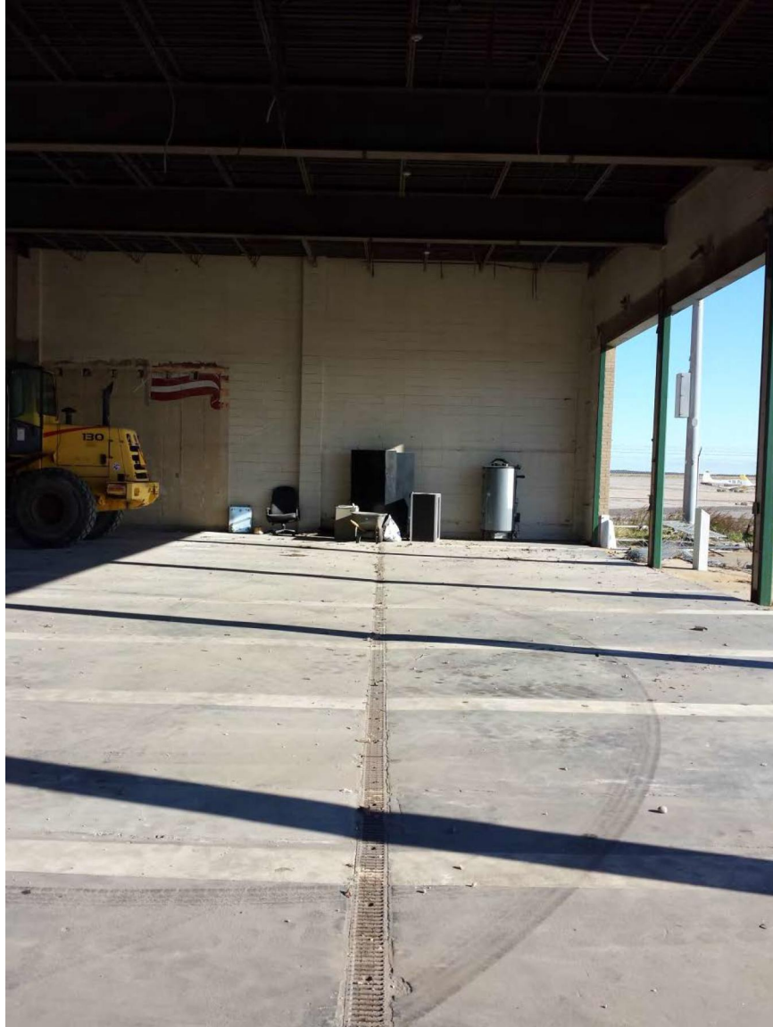
Photo 1: Trench drains were present in Building 300 (Fire Station), which was undergoing construction during the PA site visit. Fire Department vehicles were stored in this area. AFFF pallets were historically stored on the far (northeasterly) wall.
