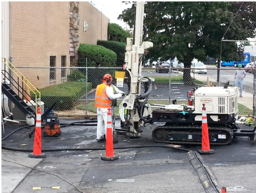
Photo 5 – Driving rods to inject in Area B. 10/01/14
