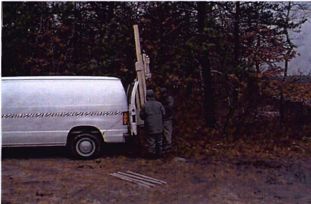
Photograph 2 Installation of DP-01 (Looking West)
