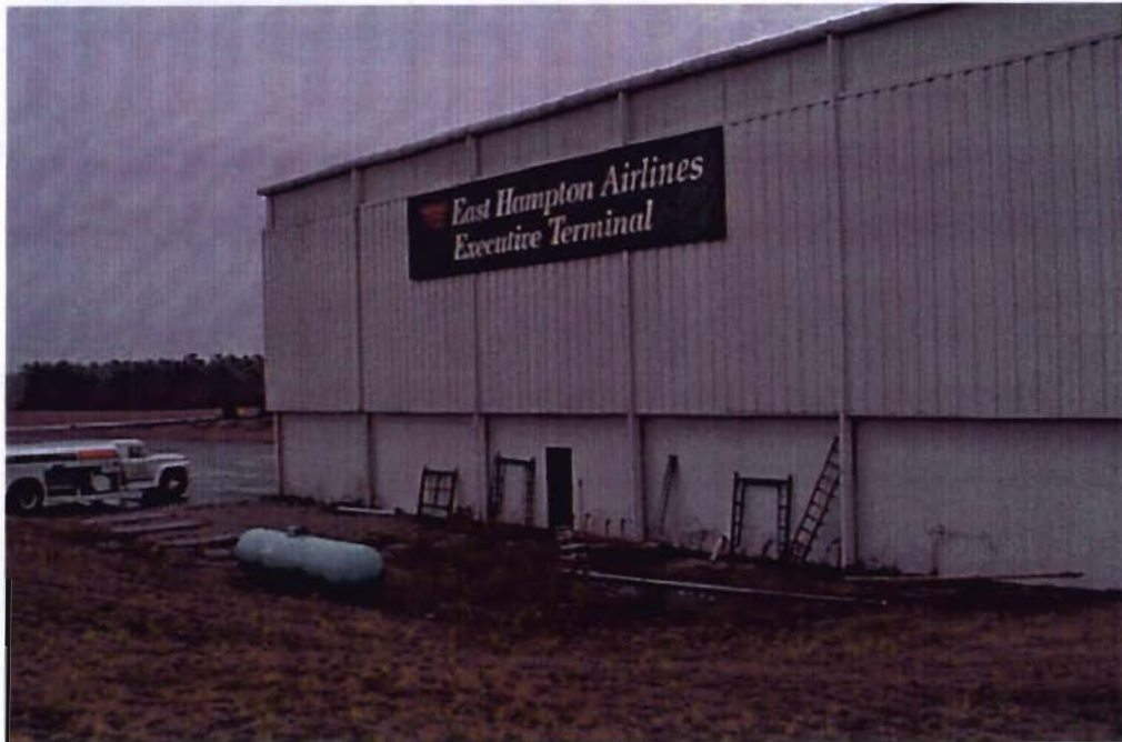
Photograph 3 North side of hanger – dry well cover at center and concrete tank pads at left (Looking Southeast)
