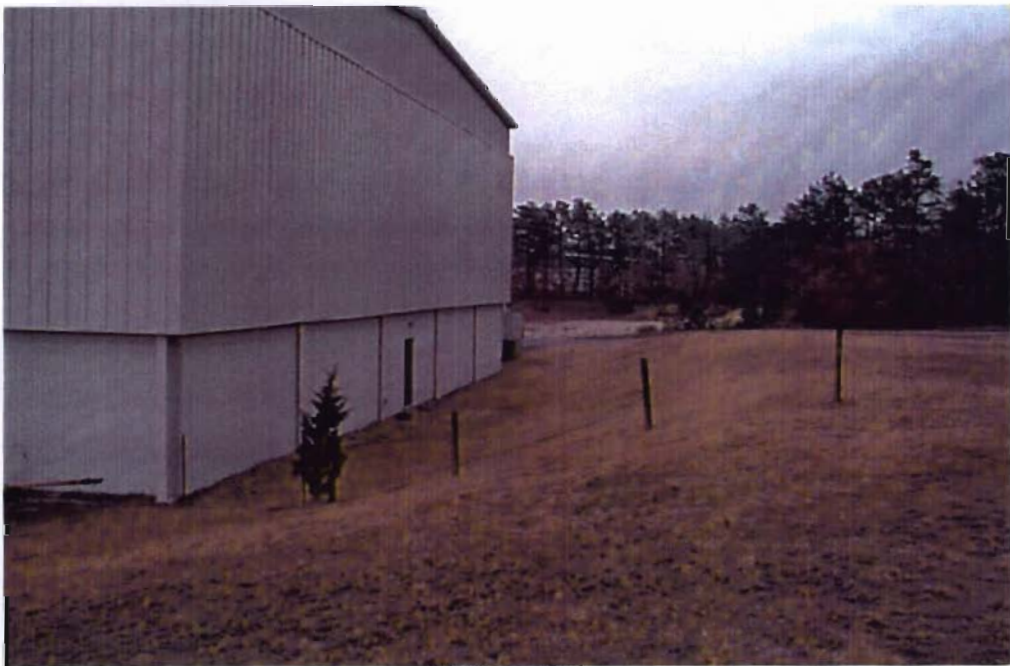
Photograph 4 West side of hanger (Looking South)
