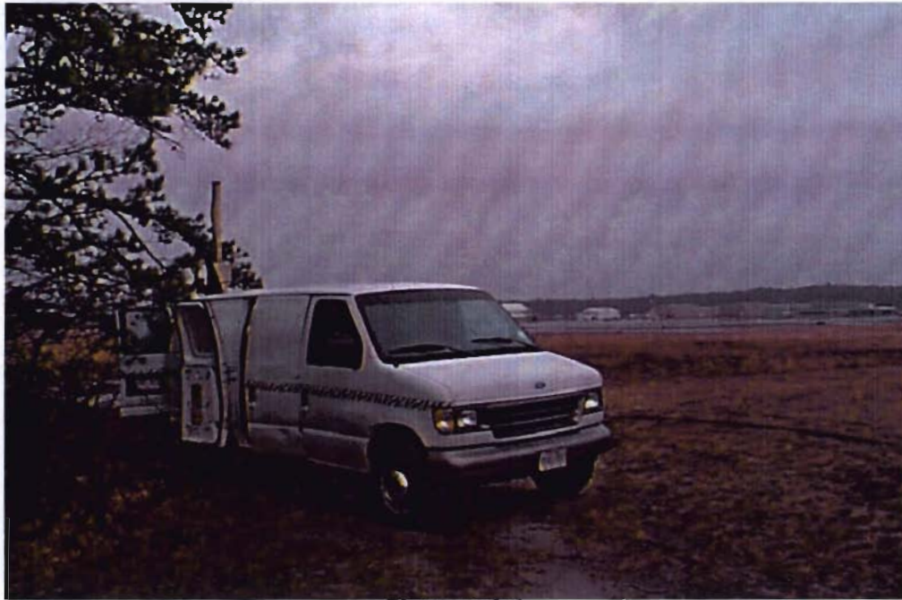
Photograph 1 Installation of DP-01 – East Hampton Airport in background (Looking North)
