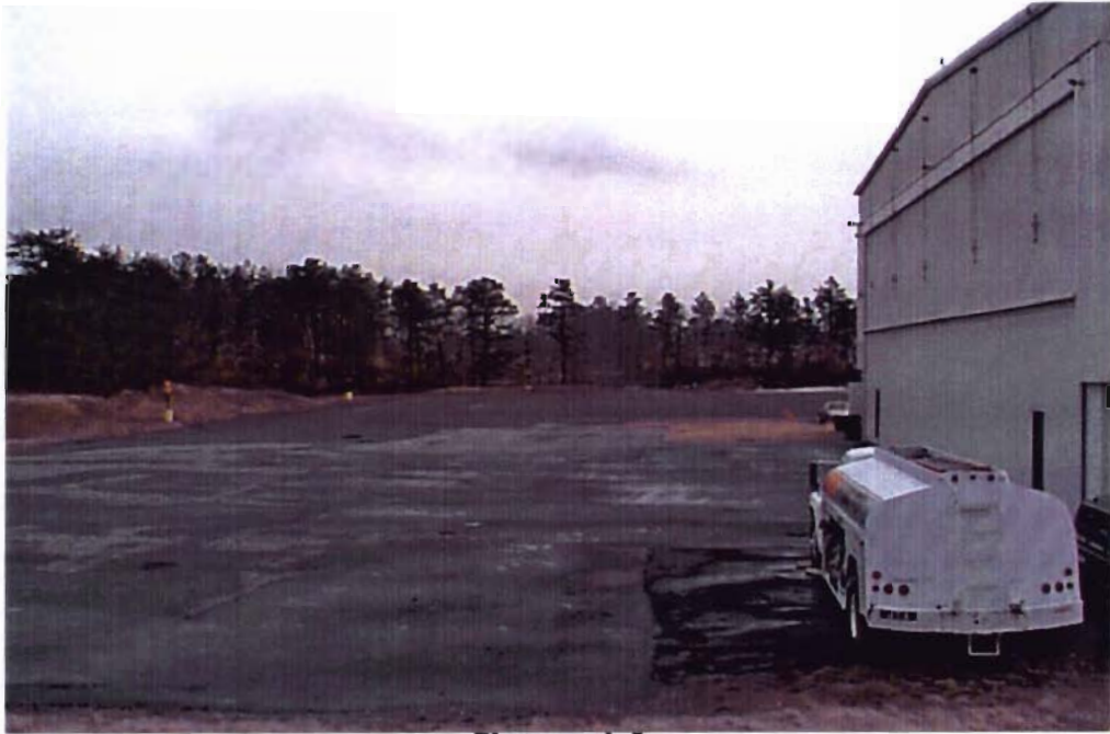
Photograph 5 East side of hanger – taxi area at left and fuel truck in foreground (Looking South)
