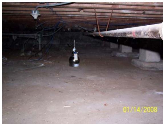
EC Structure 05 Basement Air.
