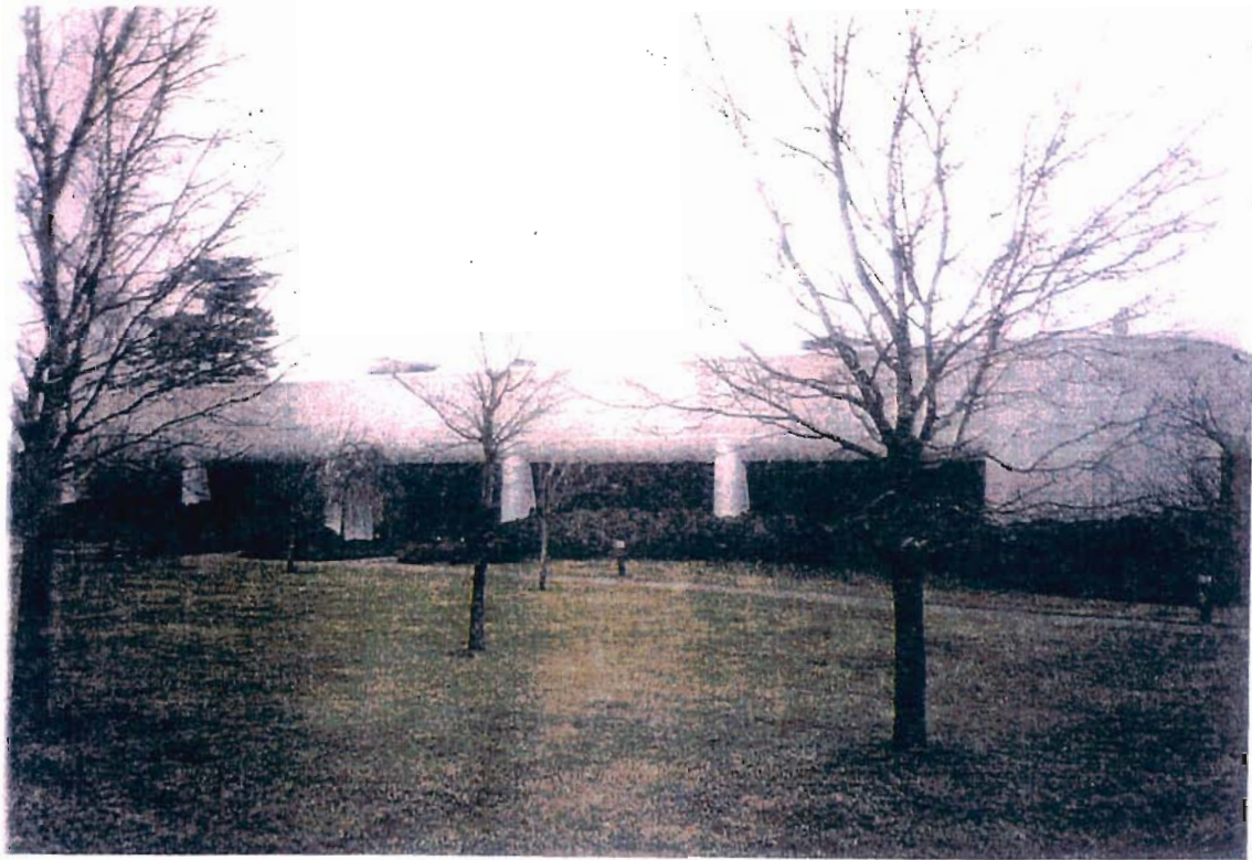
5. View of the front (north) side of the subject building.
