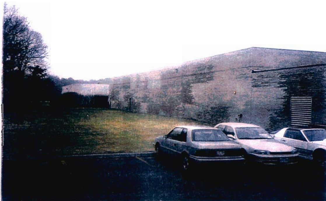
8. View of the west side of the subject building.
