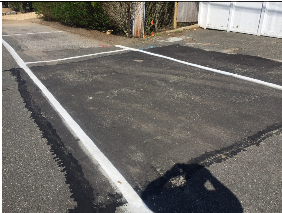
Photo 3 – Other new asphalt patch within composite cover located next to the building.
