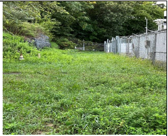
2. Adjacent to east side of substation.
