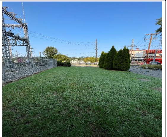
4. Northern Portion of Lowland Area.
