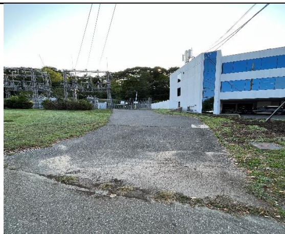
5. Southern side of Site and substation driveway.
