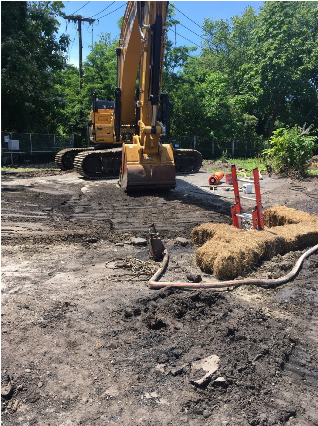
Photo 2: Backfilled trench used for plugging clay pipe
