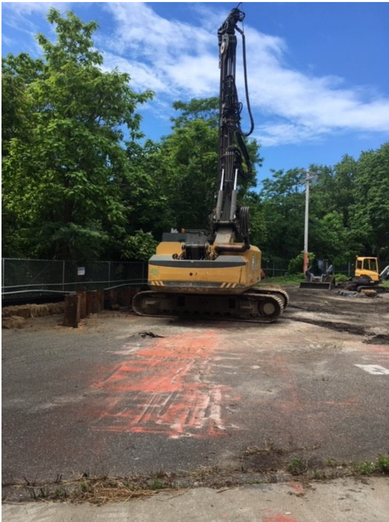
Photo 1: Sheet pile wall installation.
