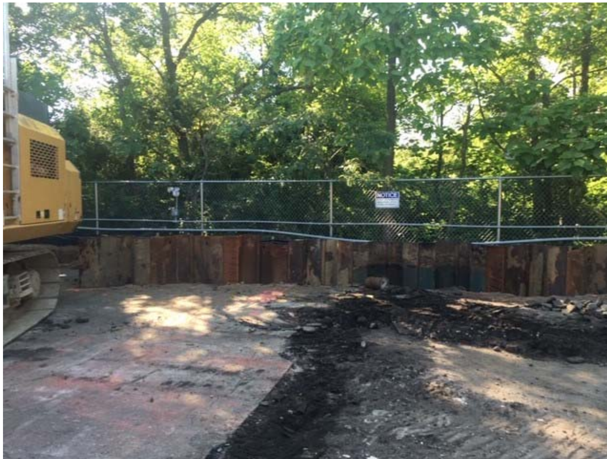
Photo 1: Installed sheet pile wall.
