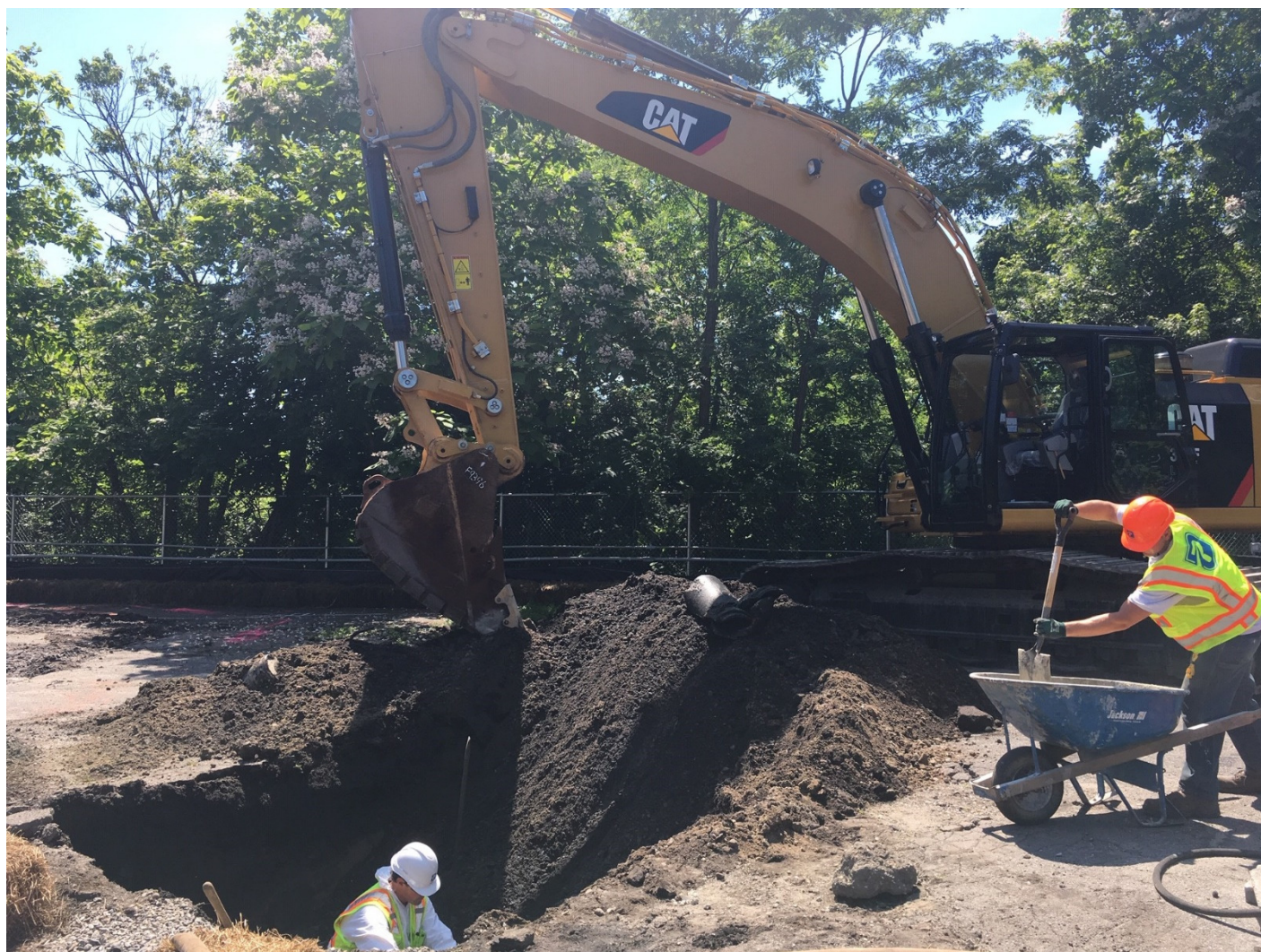
Photo 1: Plugging clay pipe outflowing from southern catch basin (located at the bottom left corner of the picture).
