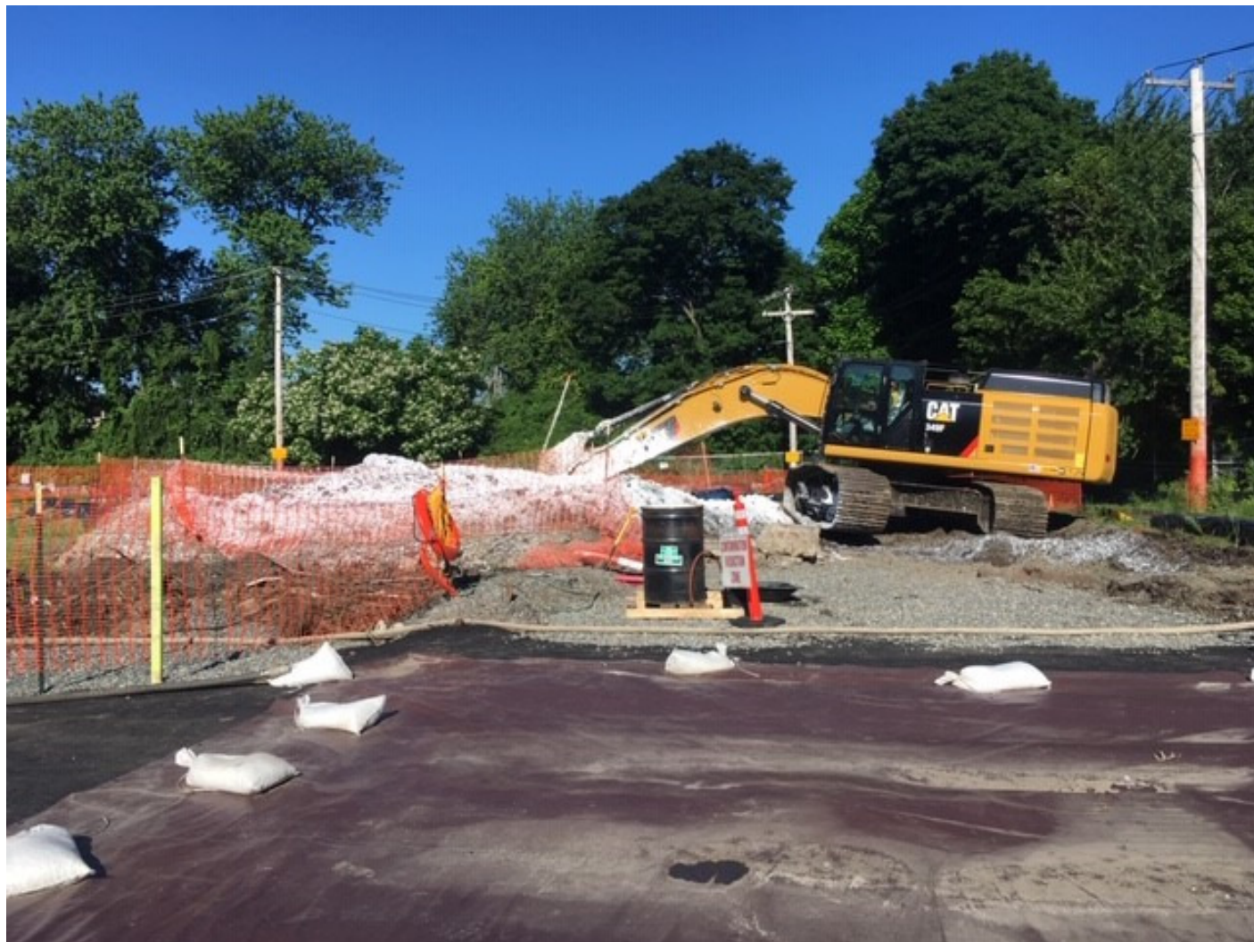
Photo 2: Mixing in Cell A13 after application of foam to reduce odors.
