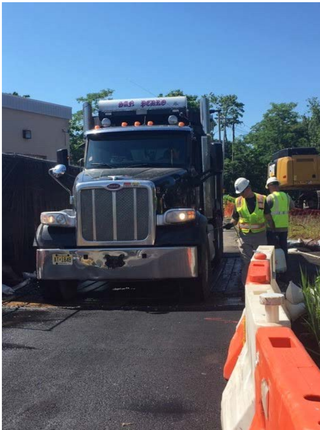
Photo 1: Truck being decontaminated after being filled with excavated soil.
