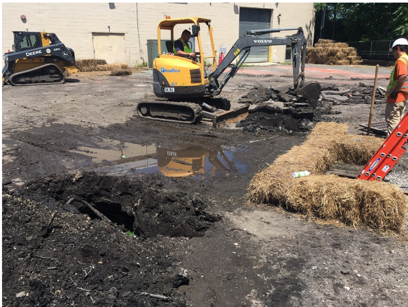
Photo 3: Trenching to locate east-west running clay pipe.
