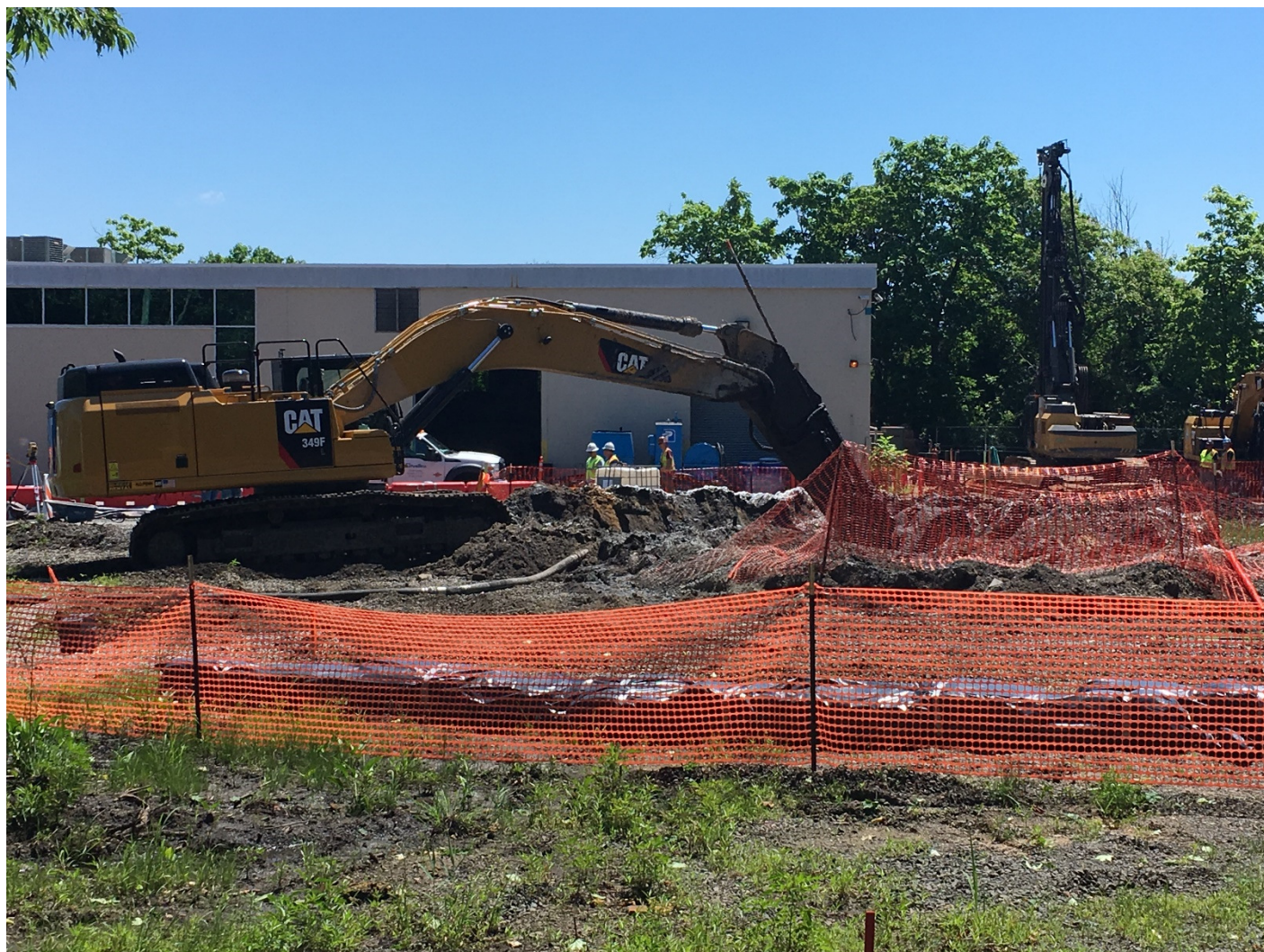
Photo 1: Bucket mixing in Pilot Test Cell A14.
