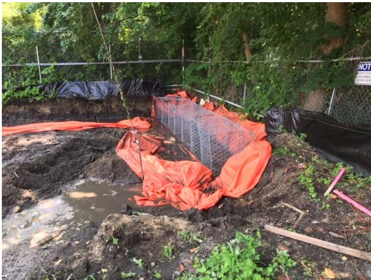
Photo 1: Gabion baskets at southwest corner of two-foot excavation area.
