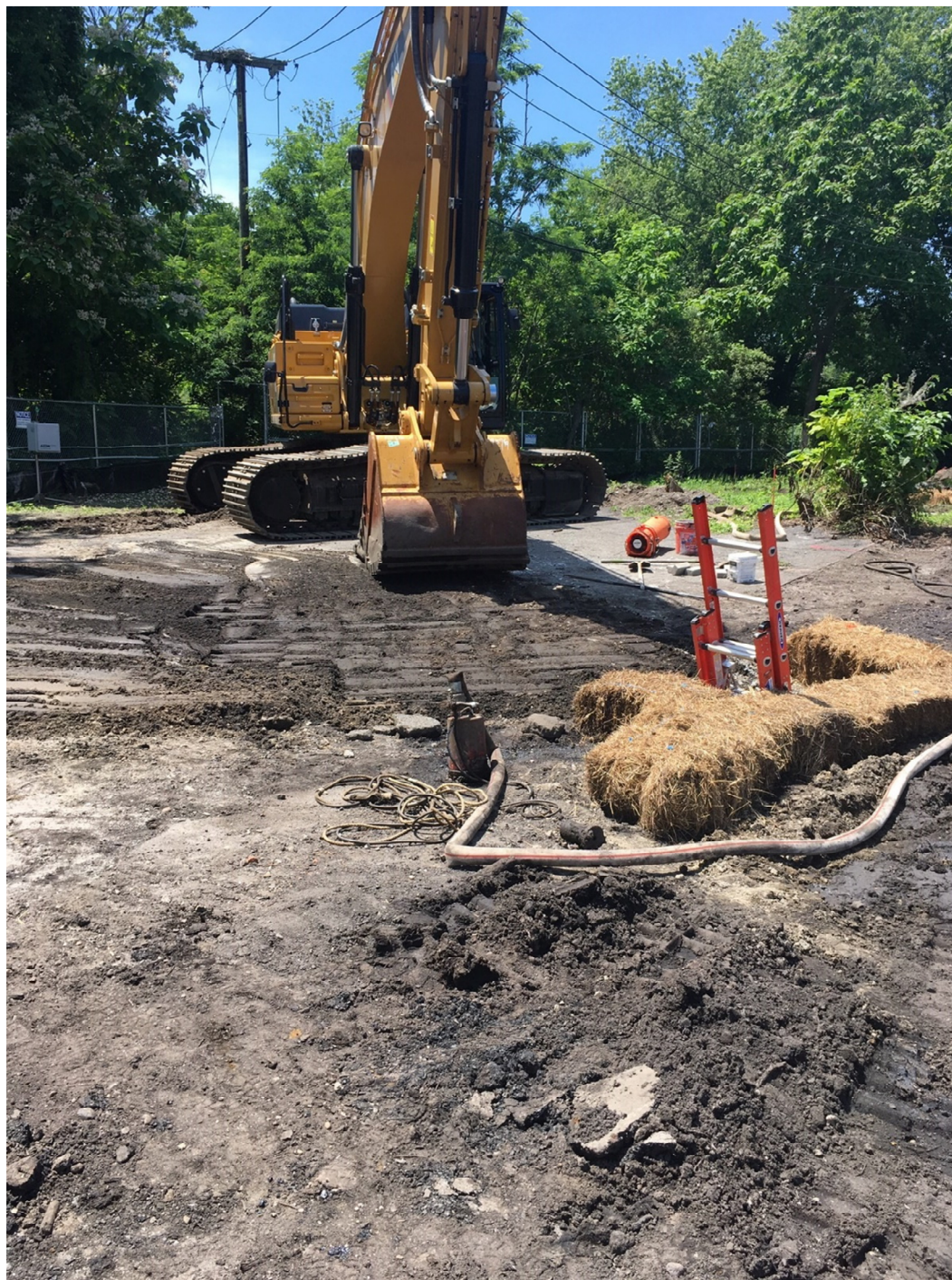
Photo 2: Backfilled trench used for plugging clay pipe
