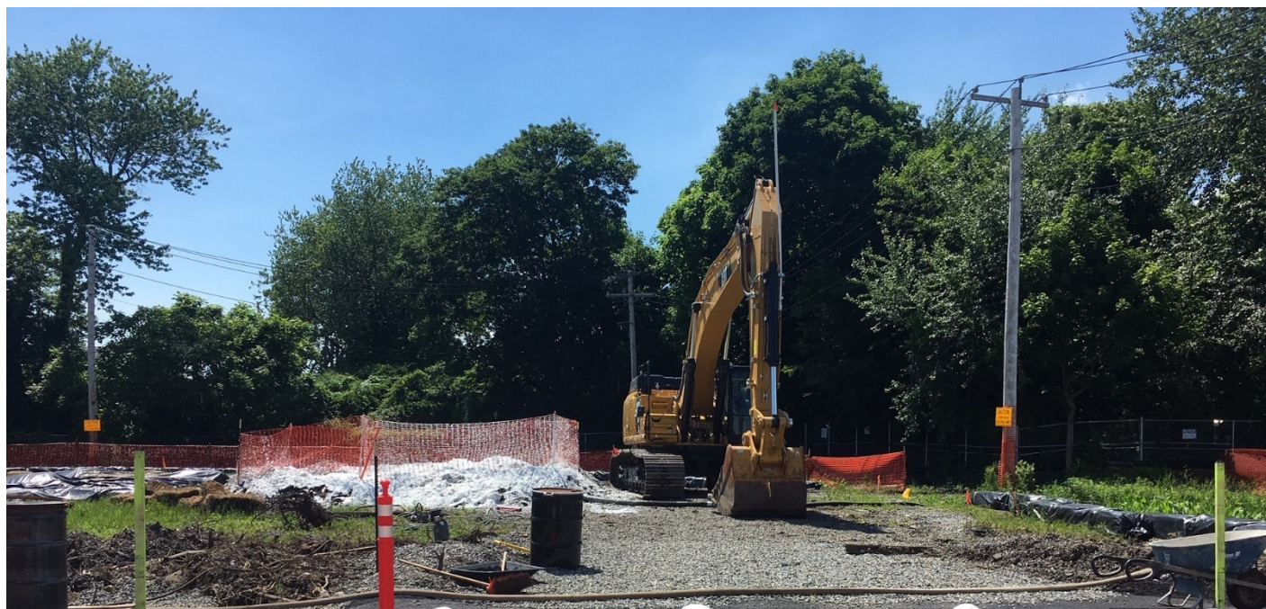
Photo 3: Pilot test area at end of work day. Excavation area is fenced and covered with foam to prevent odors.
