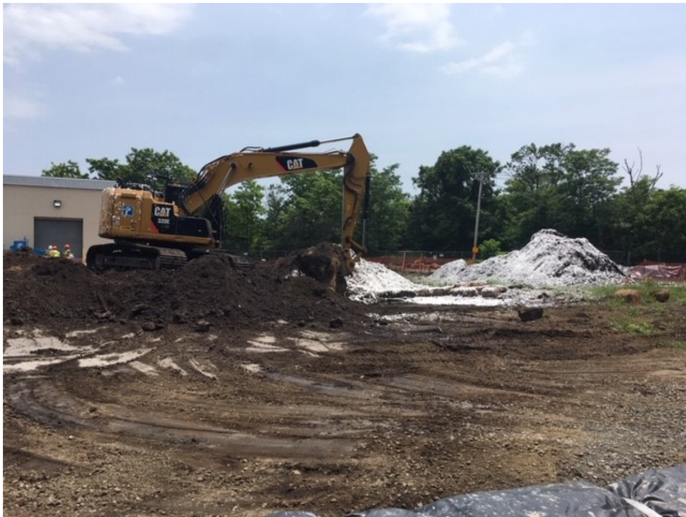
Photo 3: Excavating and stockpiling ISS pilot study swell.
