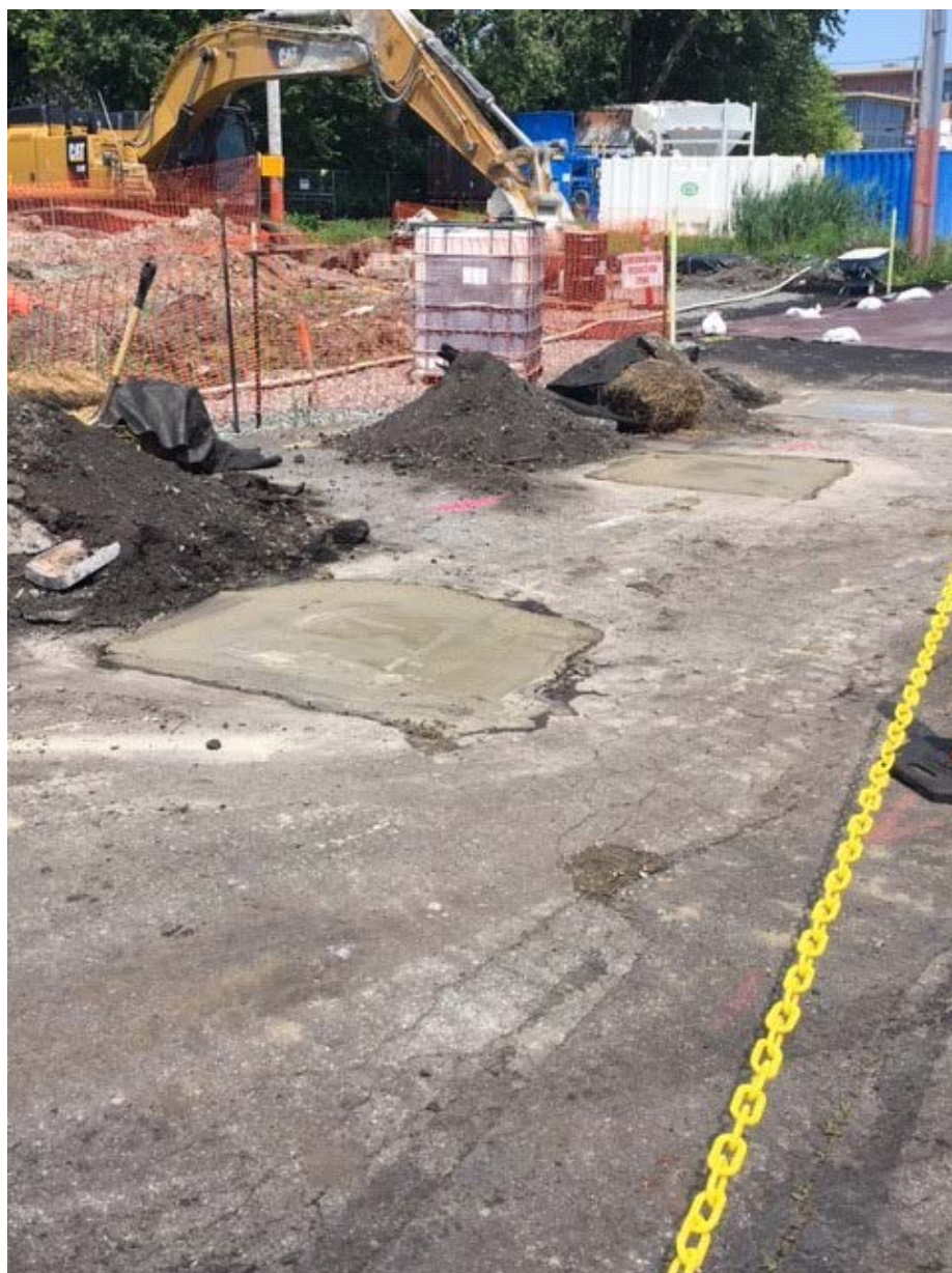
Photo 1: Three of the areas excavated to plug pipe between northern and southern catch basins, filled in with cement.
