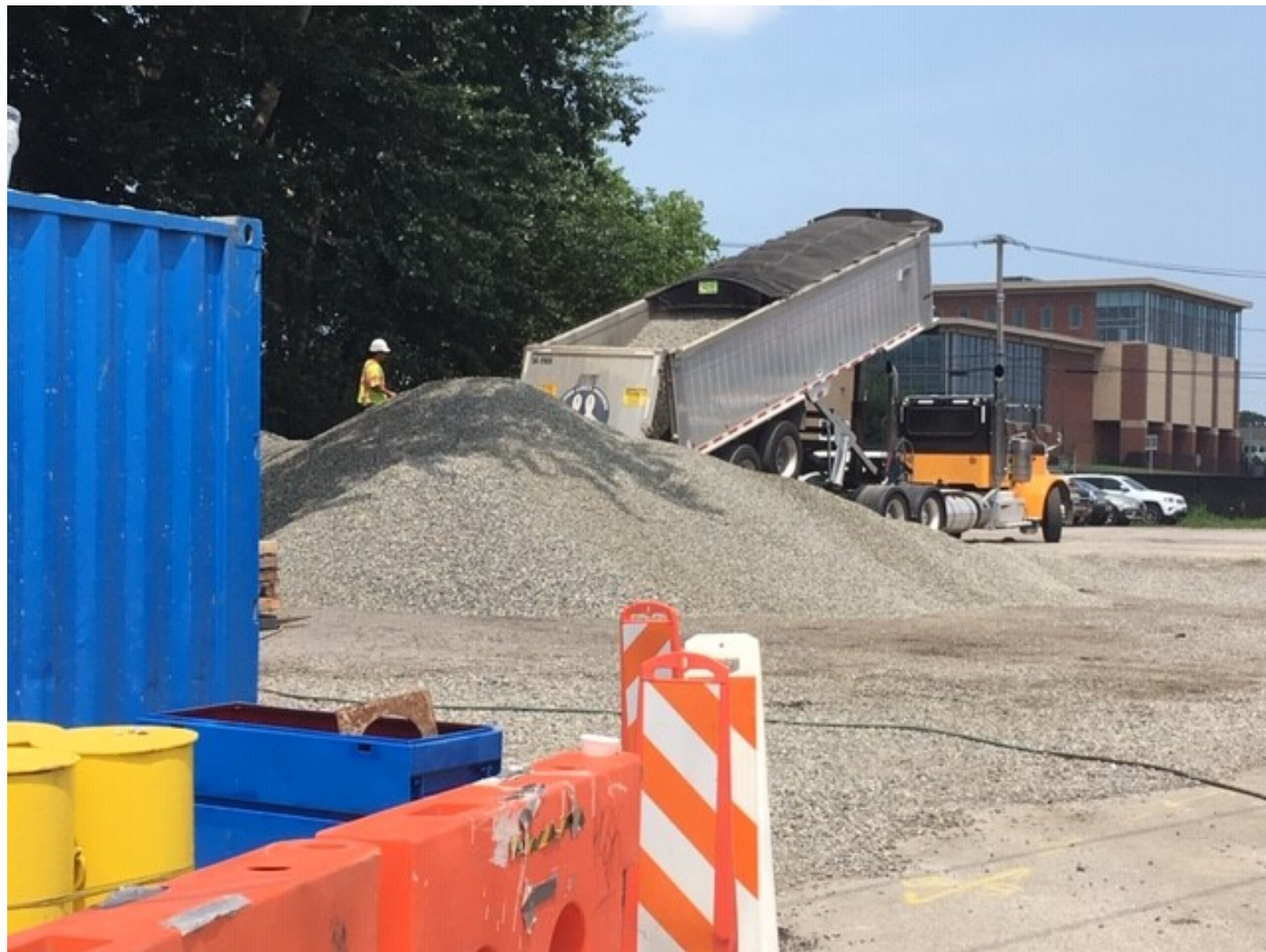
Photo 2: Crushed stone delivery. Posillico sprayed stone with water during delivery to mitigate dust.
