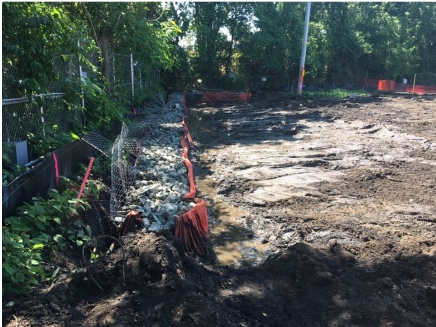
Photo 2: Installed gabion baskets.
