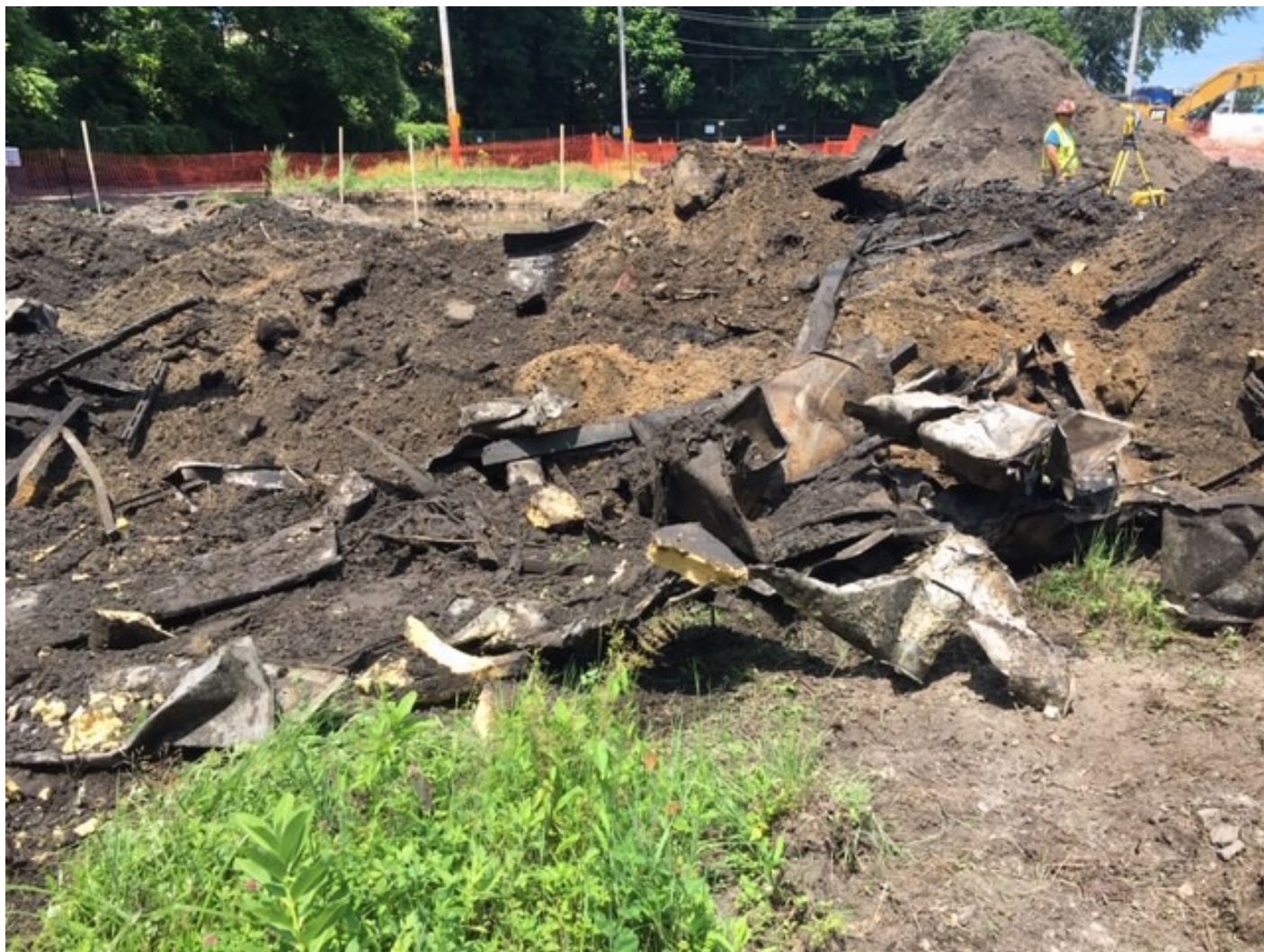
Photo 3: Excavated debris consisting primarily of scrap metal, foam, and wood.
