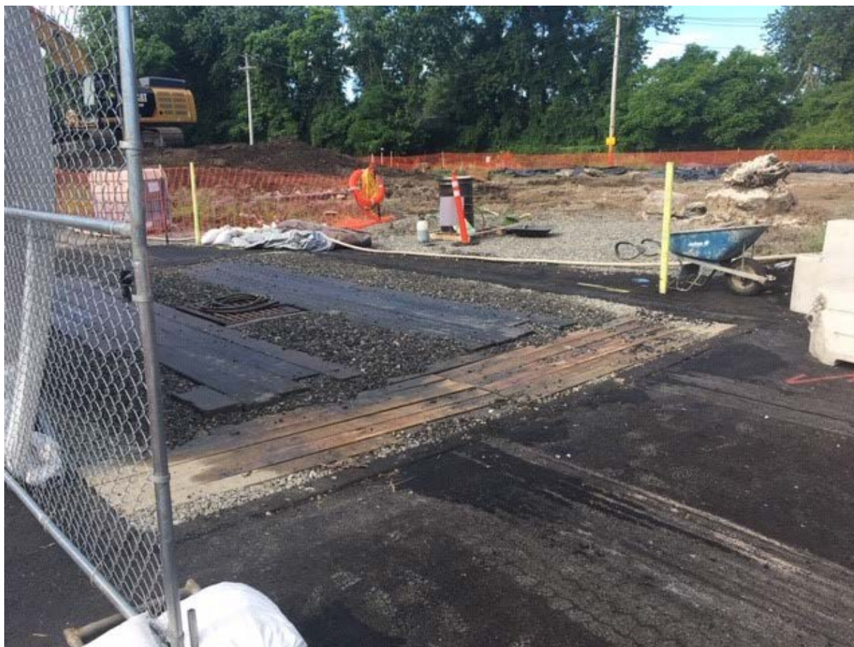
Photo 1: Decontamination pad.
