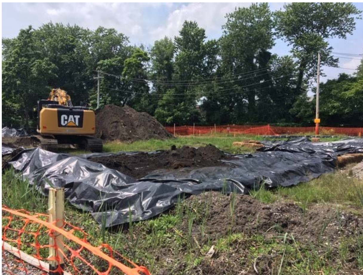
Photo 1: Area where excavated soil and ISS swell was placed.
