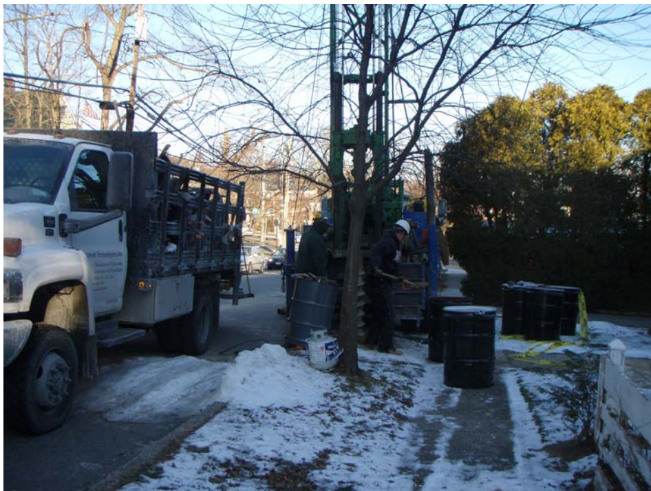
Aztech Technologies HSA Rig and Support Vehicle at MW-1S
