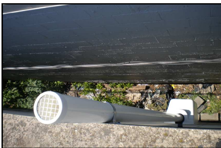
System 1 - discharge piping
