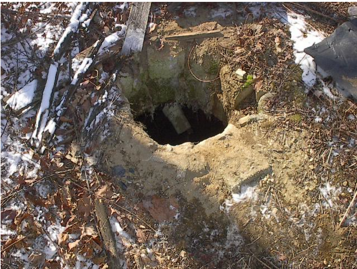
Photo 2: Close up of cesspool manway, observed in excavation pit.
