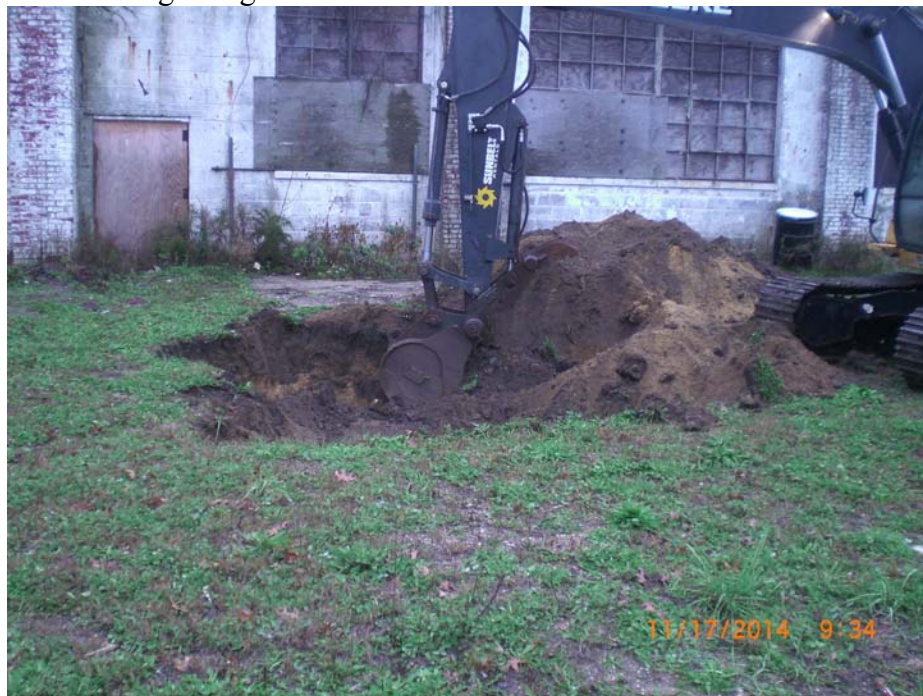
Photo 1: Beginning CP-5 Excavation
