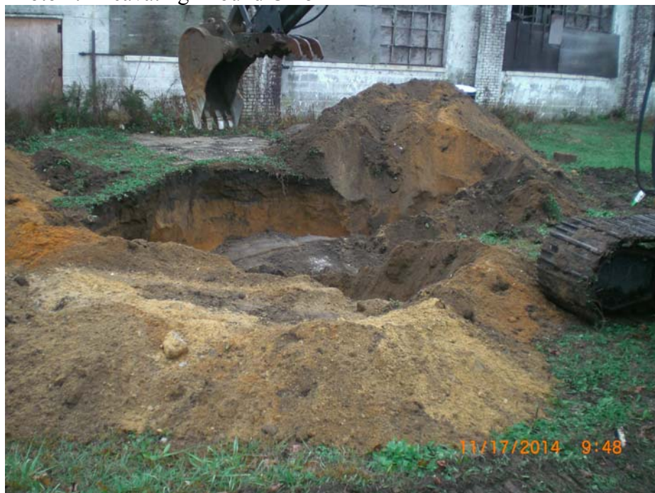
Photo 2: Excavating Around CP-5
