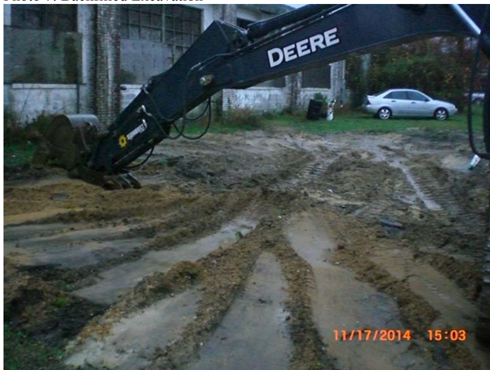
Photo 7: Backfilled Excavation
