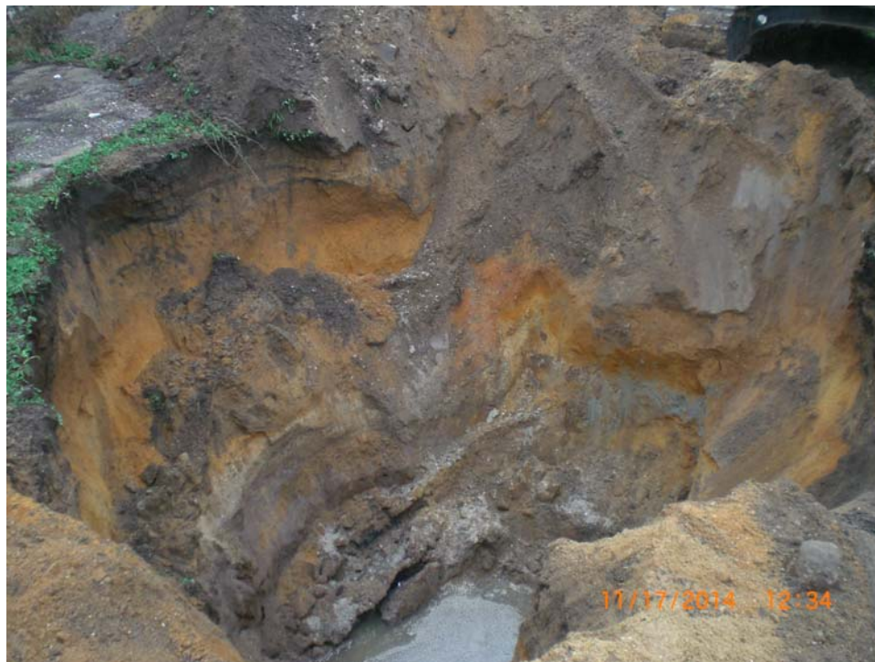
Photo 5: Excavation w/ CP-5 Removed
