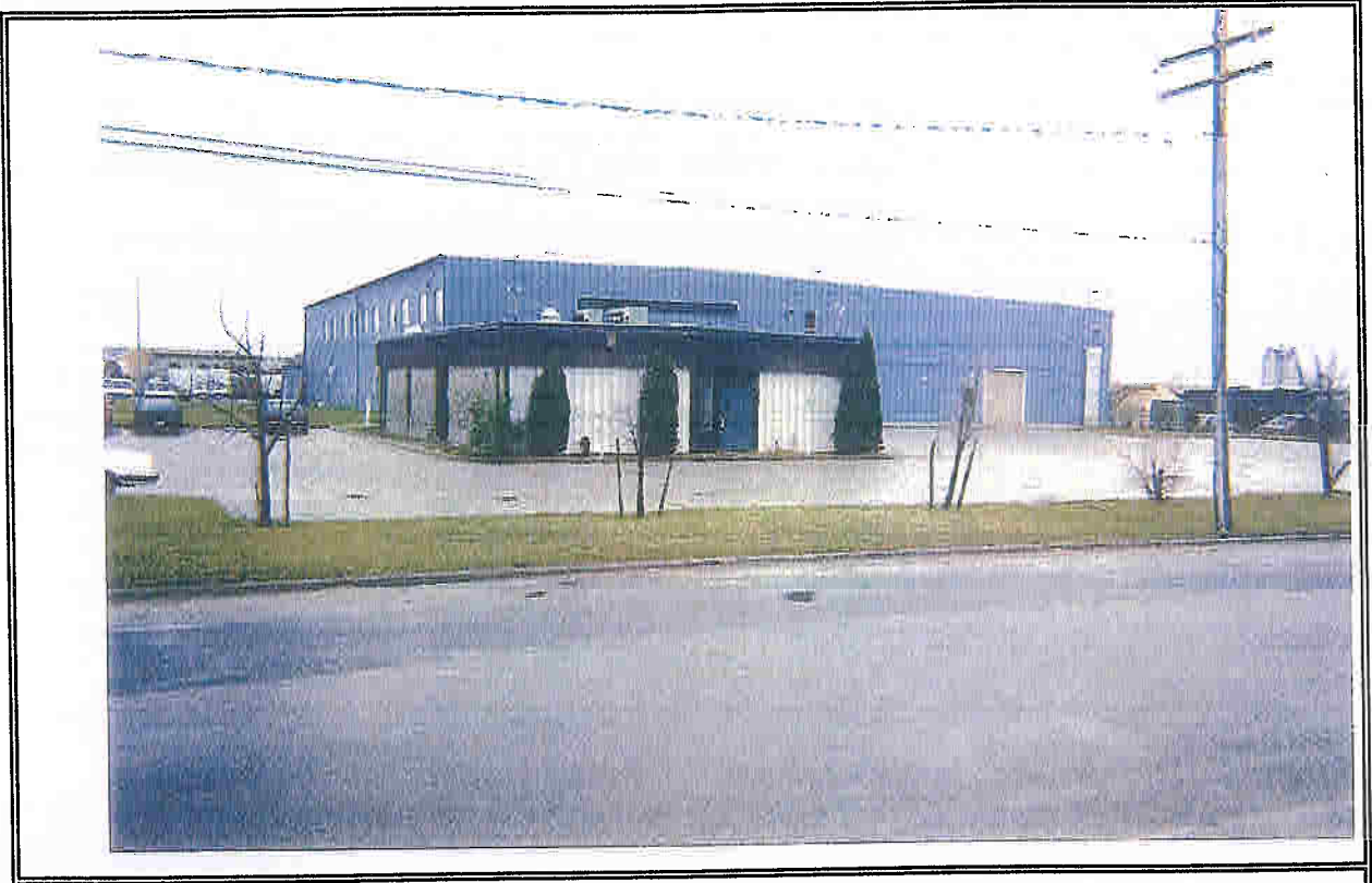
PHOTO 01: View of site looking south.
