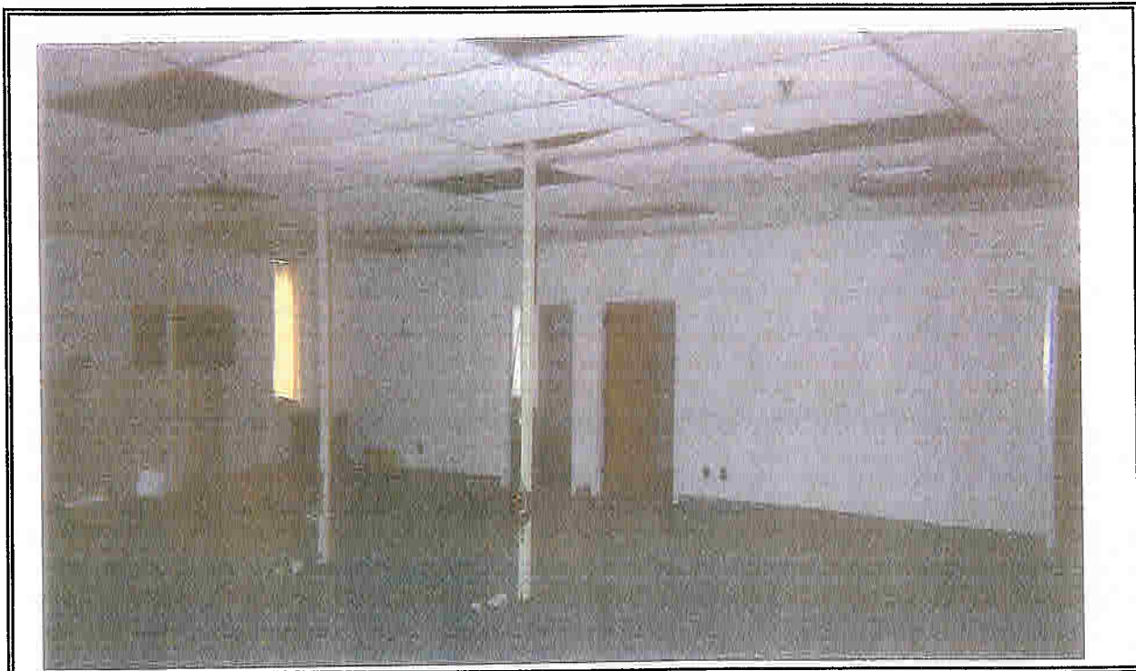
PHOTO 10: View of vacated office area.
