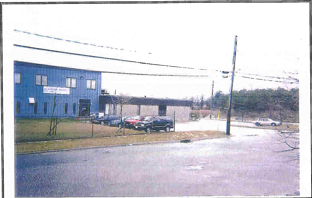
PHOTO 03: View of office and adjacent vacant lot, looking northwest from Cleveland Avenue.
