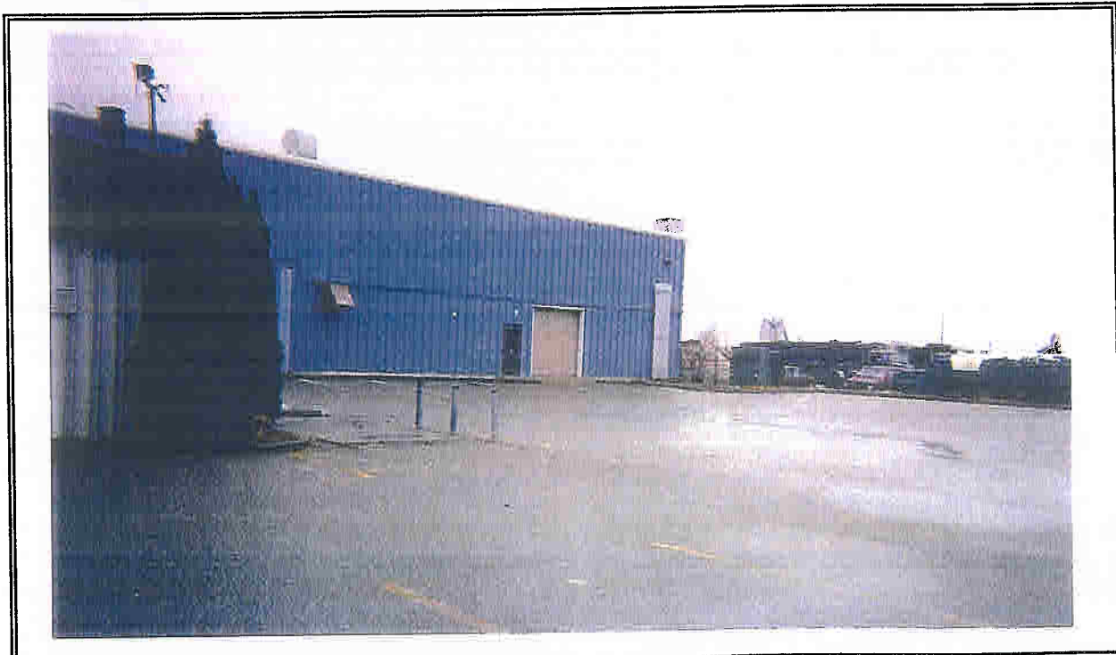
PHOTO 02: View of north side of Production area , pad mounted transformer and adjacent truck parking lot.
