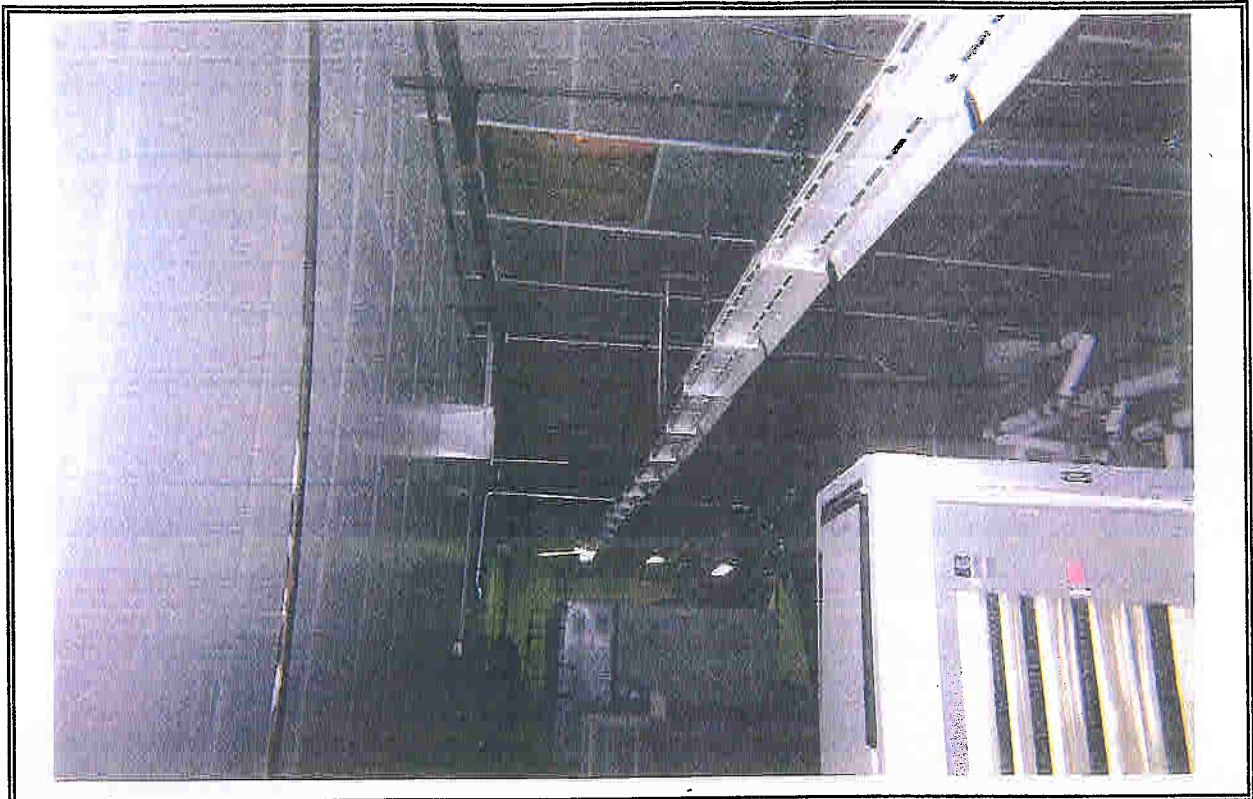
PHOTO 09: View of Fuel Test Cell with exposed ceiling insulation.
