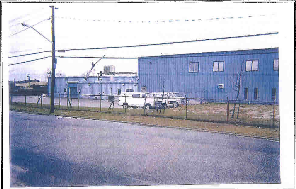
PHOTO 05: View of production area and shipping area from Cleveland Avenue.
