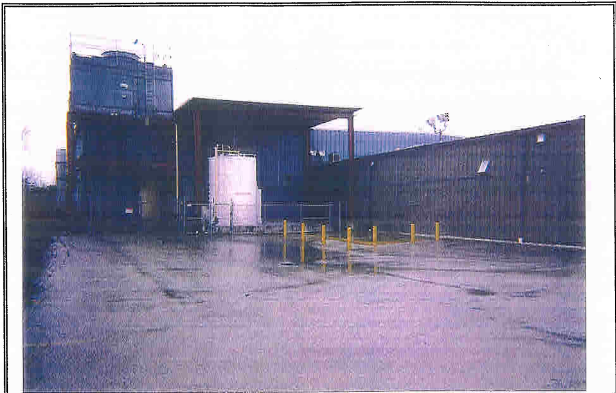
PHOTO 07: View of AST's, cooling tower and production and shipping areas looking northeast. Note: Yellow posts outline former hazardous materials storage shed location.
