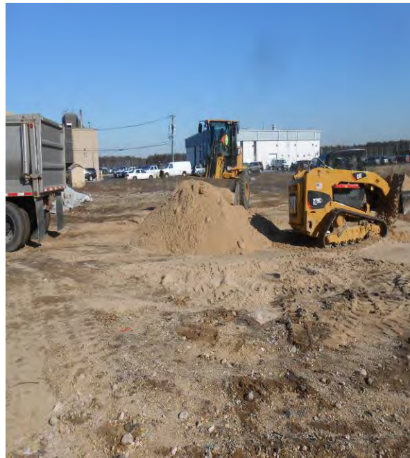
3. Backfilling the Excavation
