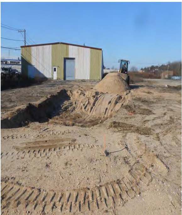
2. Backfilling the Excavation
