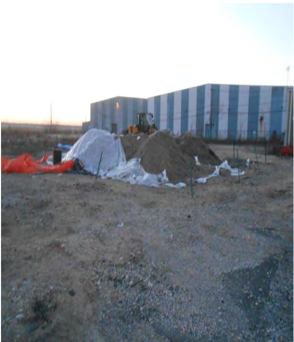
1. Stockpile With Top Tarp Removed
