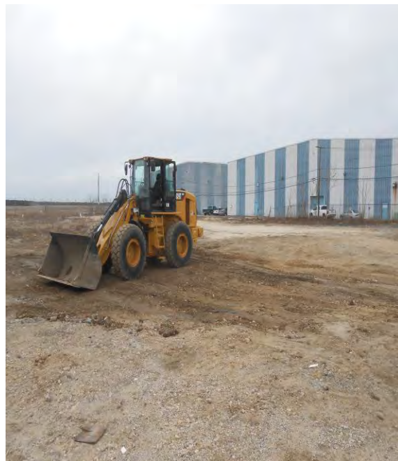
4. Soil Loadout Complete
