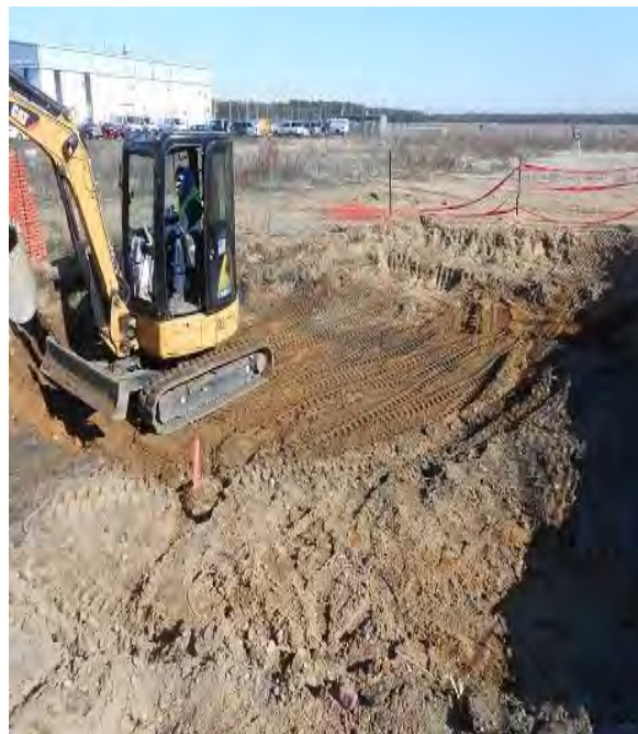
11. Excavation nearing completion of dark material removal
