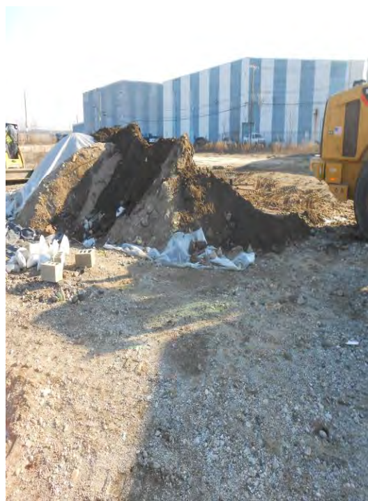
4. Remaining Stockpile at Completion of Soil Loadout Day 1
