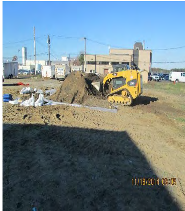
7. Stockpile construction in progress
