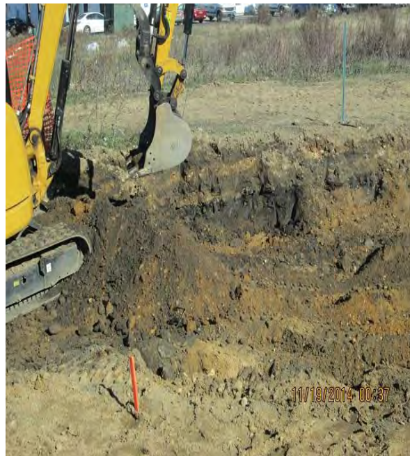
8. Southeast corner excavation showing dark stained layer
