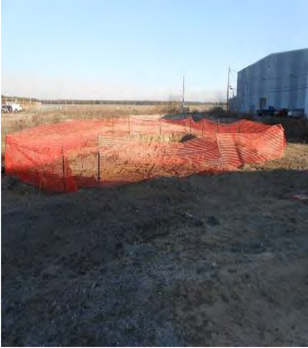
13. Secured excavation area
