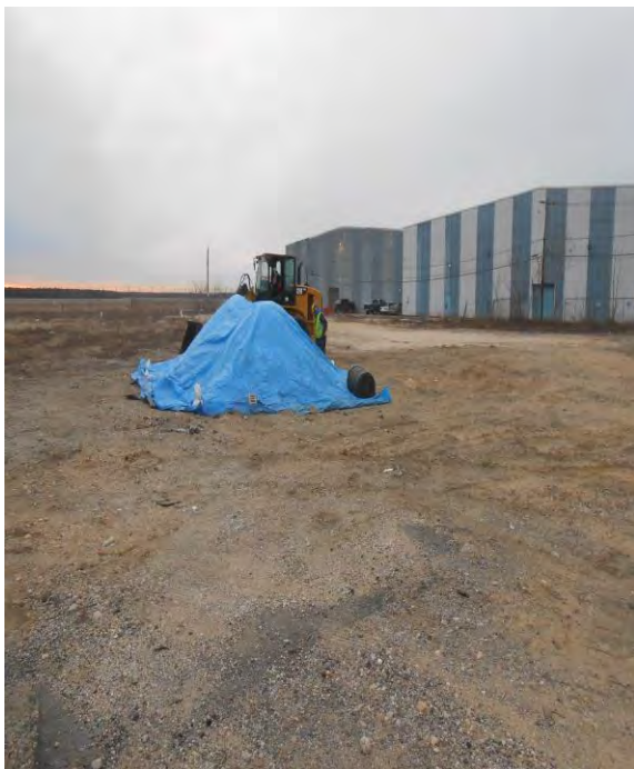
1. Stockpile Start of Soil Loadout Day 2
