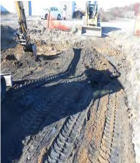
5. Excavation with dark material
