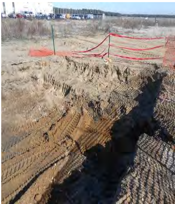
10. SE corner after removal of dark material
