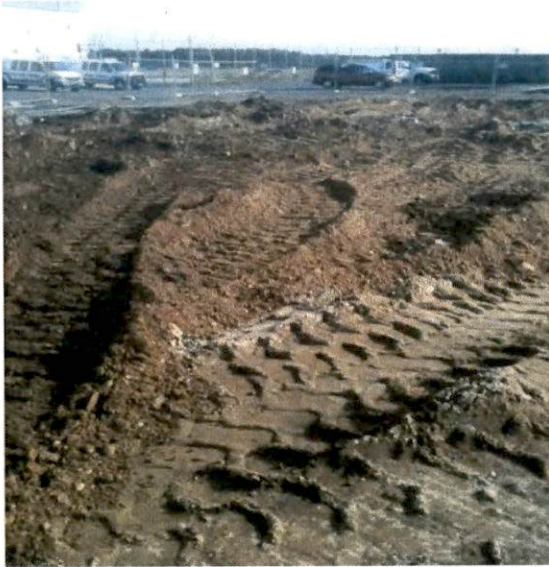
9.) View of the soil on the northern portion of the Site after excavation activities.
