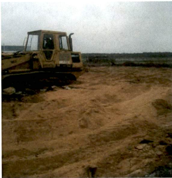
10.) View of the sand across the central portion of the site post concrete removal.
