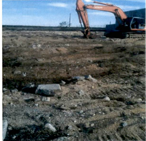
15.) View looking East across the Site post concrete foundation removal.
