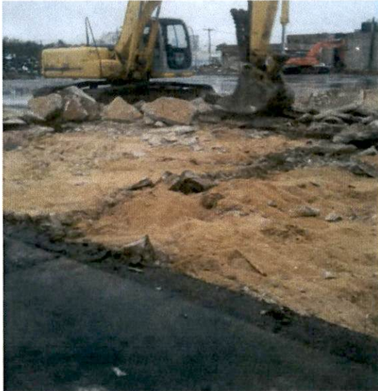
13.) View looking northwest during concrete removal activities in the southeastern portion of the Site.
