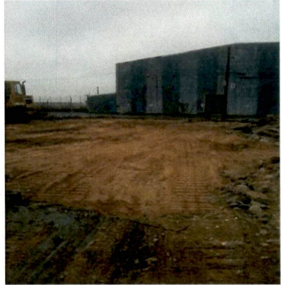
18.) View from the northwest section of the Site looking Southeast post foundation removal.
