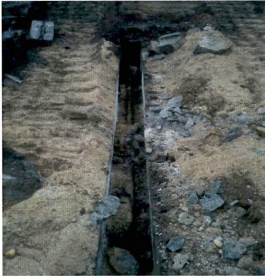
17.) Old abandoned gas line trench on the southern portion of the Site.
