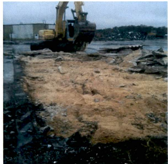
16.) View looking west from the southeastern portion of the Site.
