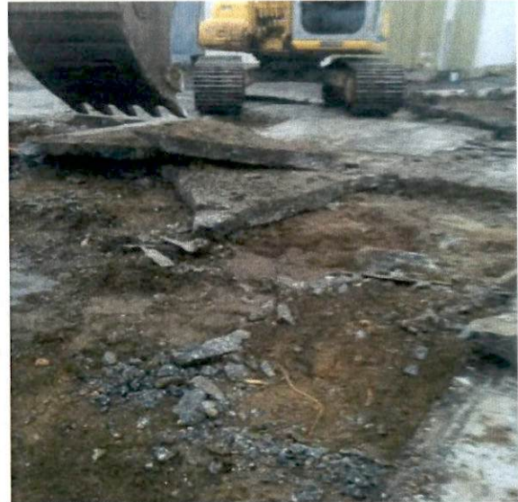
11. Concrete removal activities at the former drum storage area. (SG-7)
