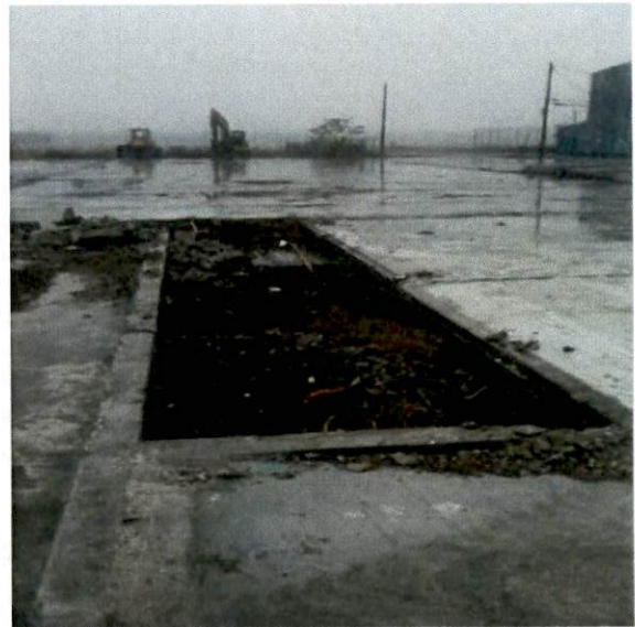
12.) View of the former drum storage area prior to concrete removal activities. (SG-7)
