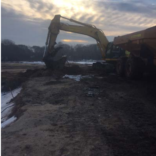
Excavation conducted in Area 8 cell J5 to 4' BGS (left picture) and JD-744K loader maintaining stockpile (right picture).
