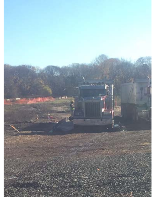
Kobelco SK350 Excavator and End Dump excavating 5 feet of material from cell K9 (left picture) and truck utilizing decontamination pad prior to being weighed. (right picture).
