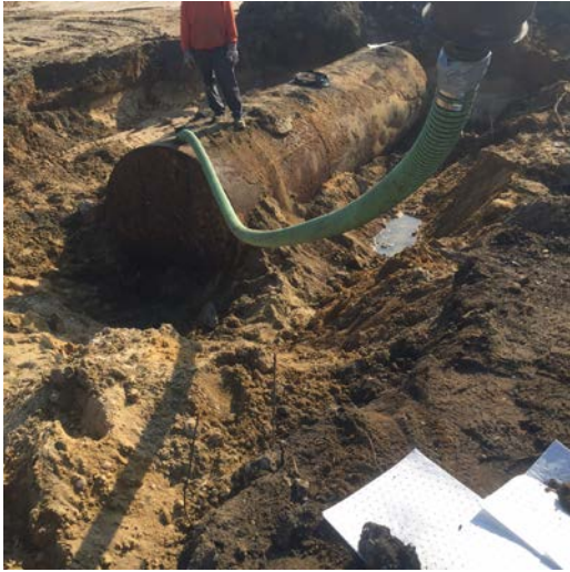
UST being vacuumed out prior to removing from the excavation (left picture) and excavation conducted in Area 4 cell I10 to 4-5' BGS
