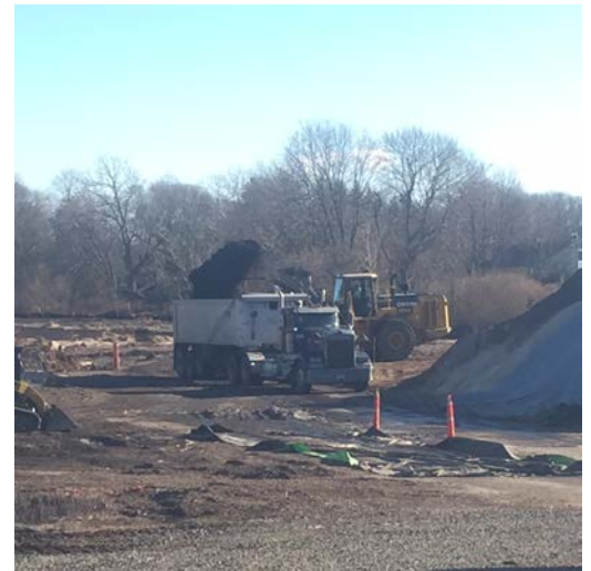
Excavation observed in Area 19 cell EOI (left picture) and JD 744K loading trucks from the Excavated Soil Stockpile (right picture).
