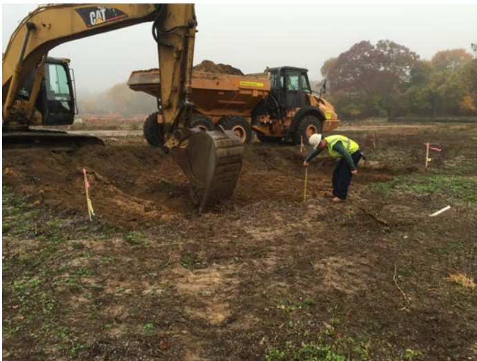
CAT 320 Excavator and End Dump excavating 2 feet of material from cell X7.
