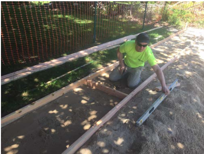
Concrete form work construction observed (left picture). Compaction observed on common fill material in form area (right picture).
