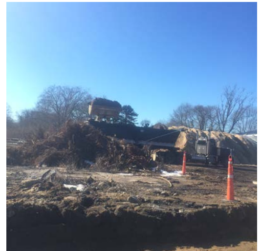
Excavation conducted in Area 14 cell F5 to 1-2' BGS (left picture) and JD-744K loader used to load trucks from the stockpile (right picture).
