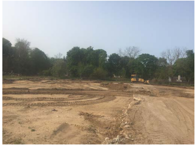
End dump loaded with regrading material in Area 9 (left picture). JD-750J dozer observed regrading in Area 2 (right picture).
