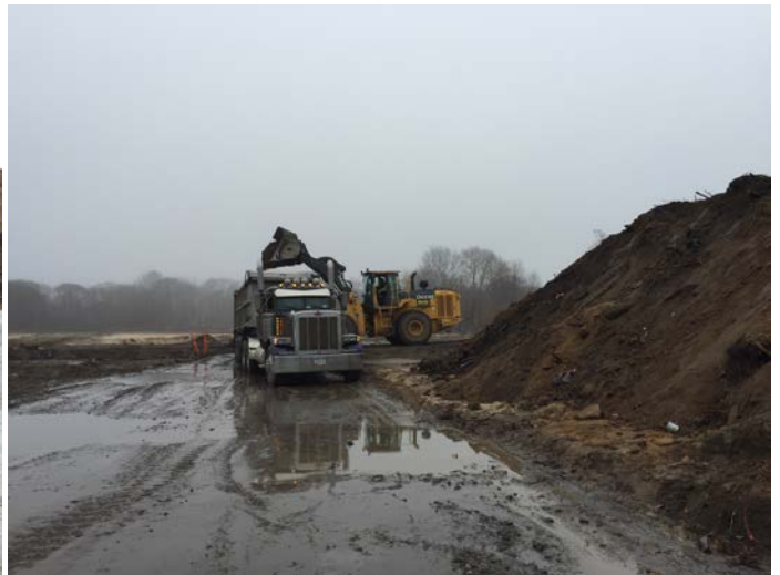
JD 744K loading trucks from the Excavated Soil Stockpile.
