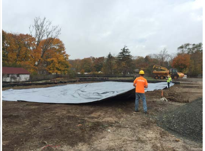
EnviroTrac installing Supreme UV Tarp in stockpile area.
