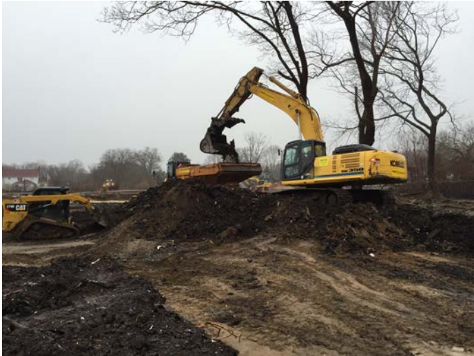
Excavation conducted with Kobelco SK350 in Area 18 cell GOC to 1' BGS (left picture) and completed excavation in Area 18 cells GOB and GOC to 1' BGS (right picture).
