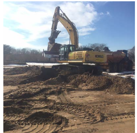
Excavation conducted in Area 8 cell N5 to 1-2' BGS (left picture) and excavation conducted in Area 8 cell M5 (right picture).
