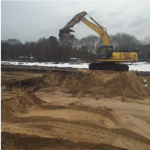
Excavation conducted in Area 8 cell O1 to 5' BGS (left picture) and excavation conducted in Area 8 cell O4 (right picture).
