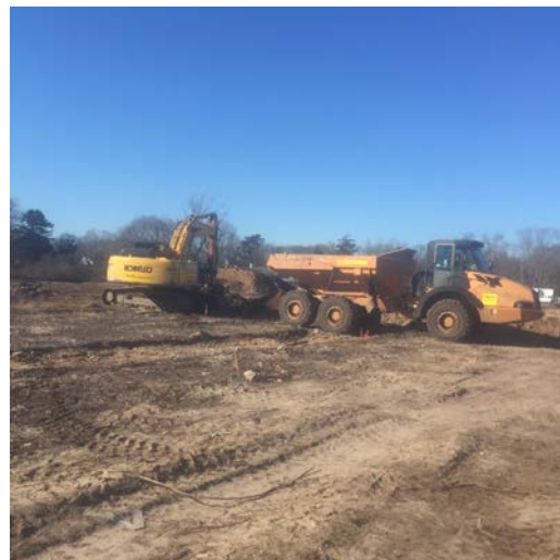
Concrete/Debris removal conducted in Area 8 (left picture) and excavation conducted in Area 8 cell K2 to 1' BGS (right picture).
