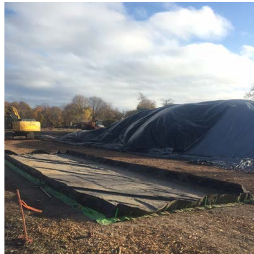
EnviroTrac covered the stockpile with the Supreme UV tarp and secured it to the ground
