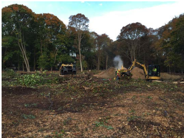
Tree/wood debris and smaller tree trunk gathering for wood chipping with the CAT 279C and the CAT 304E.
