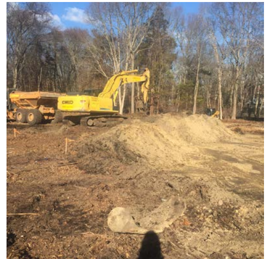
Excavation conducted with Kobelco SK350 in Area 19 cell FOJ to 1' BGS (left picture) and excavation conducted in Area 19 cell DOK to 1' BGS (right picture).
