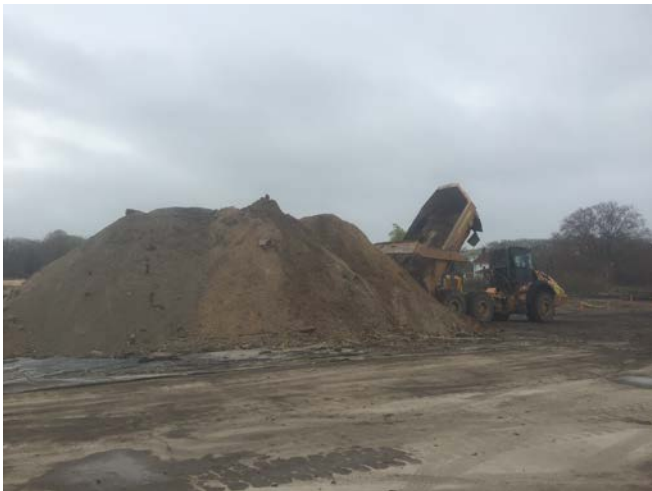
End dump placing excavated material into the stockpile (left picture). Excavation observed in Area 11 in half of cell AA11 to 3' BGS (right picture).
