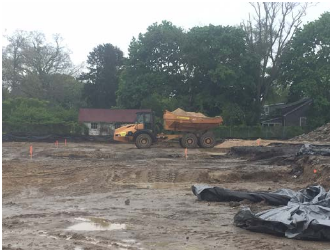
End dump placing regrading material in Area 11 (left picture). JD-750J dozer grading in Area 9 (right picture).
