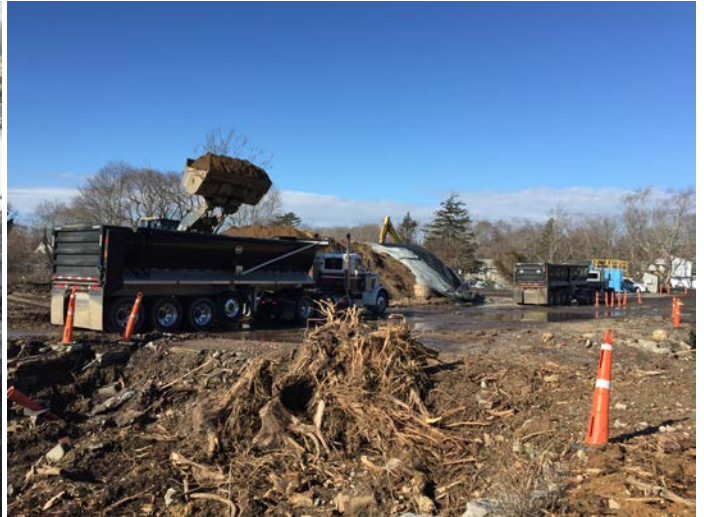
Dewatering conducted in the truck loading and Decontamination Pad areas (left picture). JD 744K loading trucks from the Excavated Soil Stockpile (right picture).
