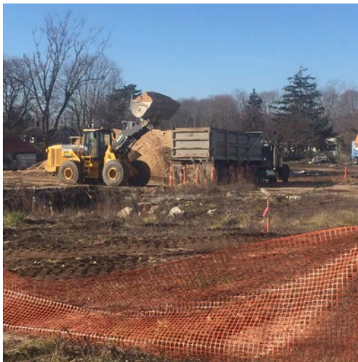
Truck loaded using JD744K loader
