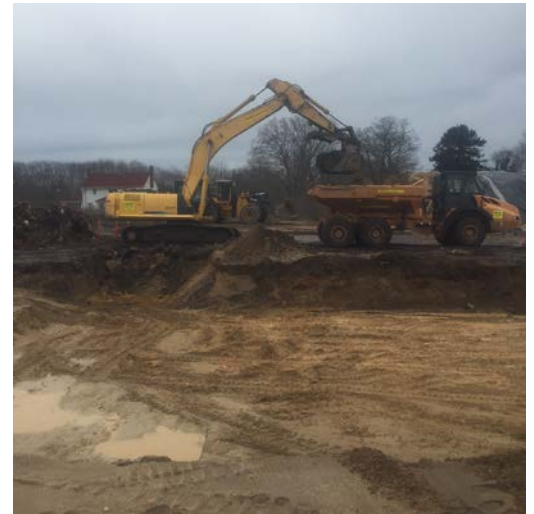
Truck loaded using the JD-744K loader from the stockpile (left picture) and excavation observed in Area 16 half of cell E6 to 4' BGS (right picture).
