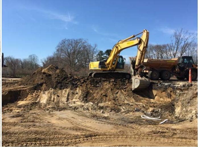
Excavation conducted in Area 9 in cell H8 with Kobelco SK350 to 1' BGS (left picture) and in Area 9 half of cell G9 (right picture).
