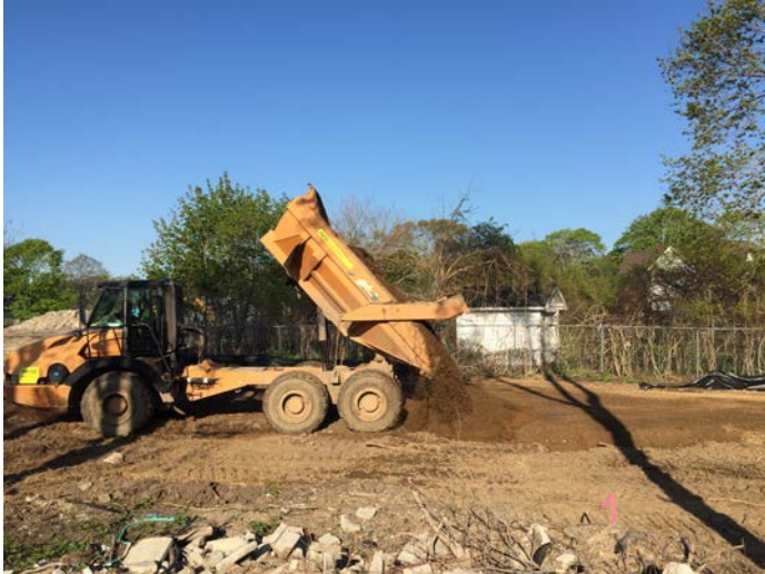
The end dump placing reg grading material in Area 19 (left picture). Backfilling/regrading observed in Area 19 (right picture).
