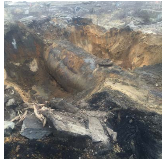
UST first exposed and depth measurement being taken (left picture). Sides of the UST exposed at the end of the day (right picture).
