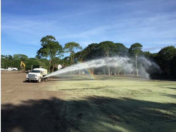
Watering already hydroseeded areas (left picture). Hydroseed mix being prepared (right picture).
