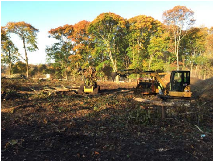
Tree/wood debris and smaller tree trunk gathering for wood chipping with the CAT 304E Excavator and CAT 279C Compact Track Loader.
