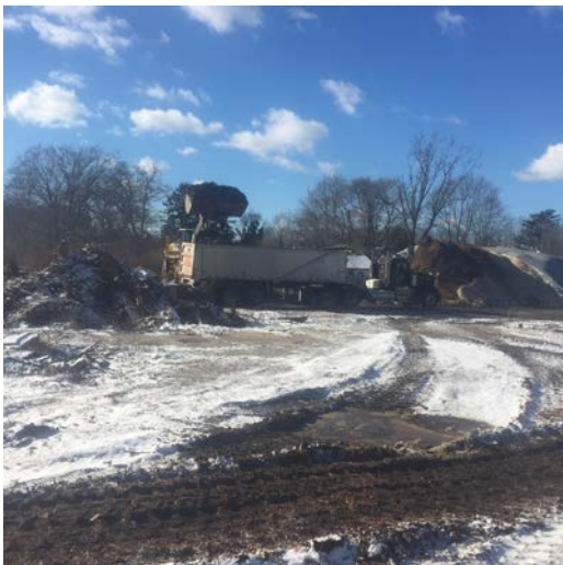
JD-744K loader loading truck with stockpiled soil (left picture) and excavation observed in Area 17 cell LOC to 1' BGS (right picture).
