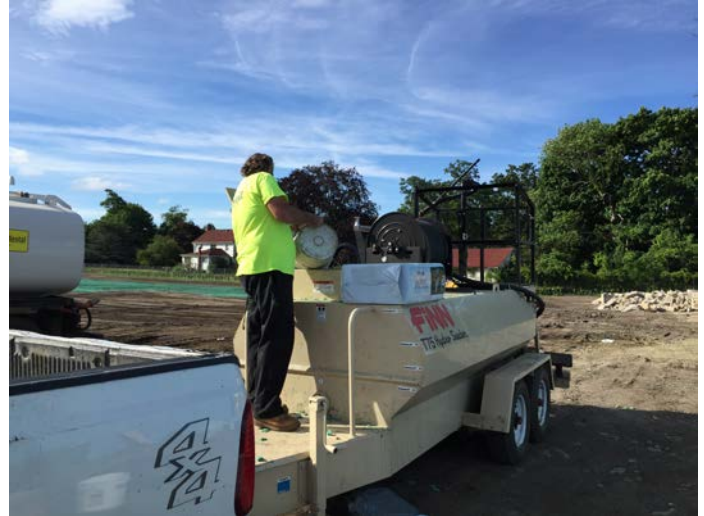
Watering already hydroseeded areas (left picture). Hydroseed mix being prepared (right picture).
