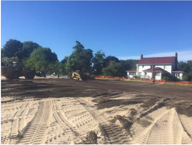
Onsite topsoil being placed spread in Area 5 (left picture). Onsite topsoil being delivered to the site while also being loaded into end dump (right picture).
