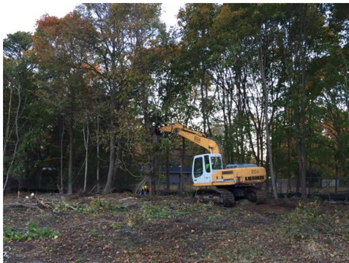
Tree cutting with chainsaw and the Liebherr 904.
