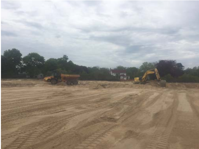
Excess regrading material loaded into end dump in Area 8 (left picture). Regrading observed in Area 2 (right picture).
