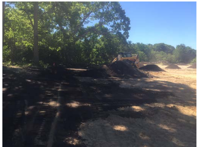
Onsite topsoil being placed in mini-piles in Areas 6 and 7 (left picture). Onsite topsoil being spread in Area 17 (right picture).
