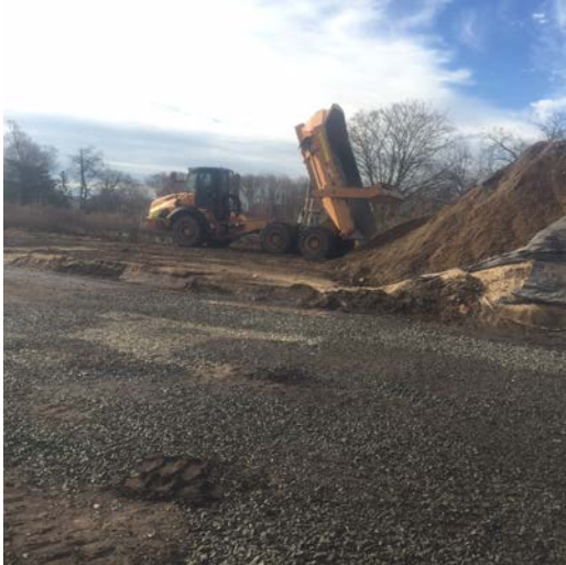
End dump placing excavated material into the stockpile (left picture) and redig excavation conducted in Area 2 cell T8 per Field Order #7(right picture).
