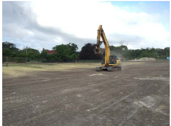
Hydroseed mix being prepared (left picture). Excavator tracking over topsoil in preparation of hydroseeding (right picture).
