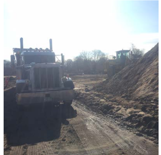
Excavation conducted in Area 14 cell F6 with Kobelco SK350 to 3' BGS (left picture) and truck being loaded using the JD-744K loader
