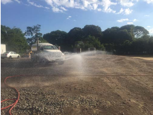
Water truck controlling dust and watering the already hydroseeded areas (left picture). Hydroseed mix being prepared (right picture).
