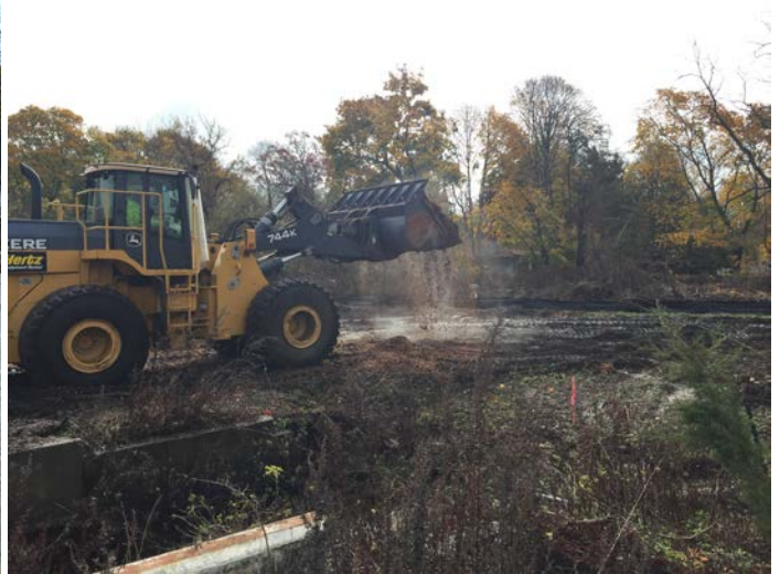
JD744K Front End Loader spreading woodchips along temporary access road.
