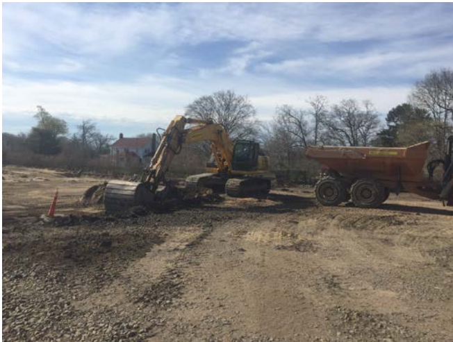
Excavation conducted in Area 11 in half of cell B9 to 1' BGS (left picture). Excavation conducted in Area 11 in half of cell B10 to 1' BGS (right picture).
