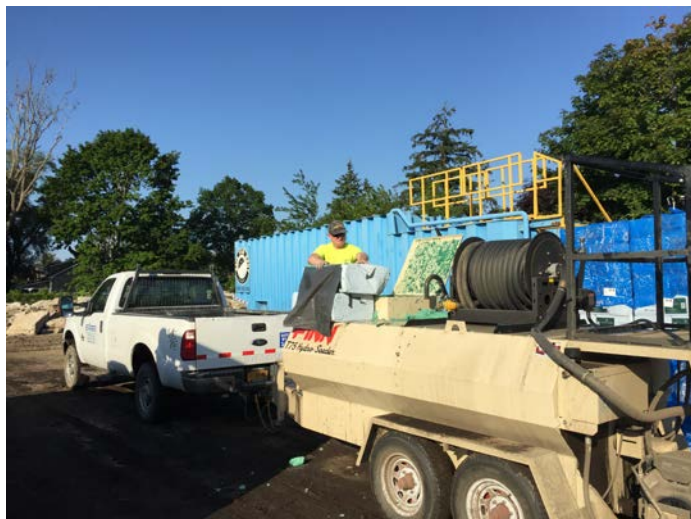
Hydroseed mix being prepared (left picture). Watering hydroseeded areas (right picture).
