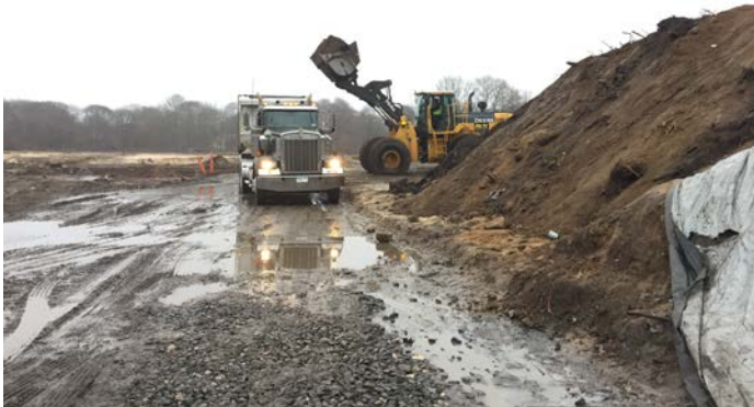
JD 744K loading trucks from the Excavated Soil Stockpile.
