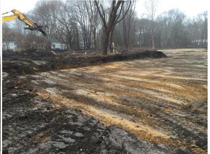
Excavation conducted with Kobelco SK350 in Area 18 cell GOC to 1' BGS (left picture) and completed excavation in Area 18 cells GOB and GOC to 1' BGS (right picture).
