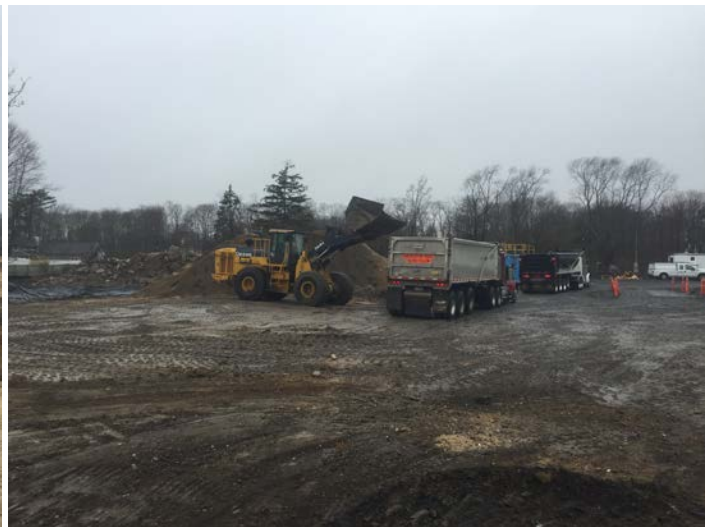
Excavation conducted in Area 10 cell F9 to 3' BGS (left picture). Truck being loaded using the JD-744K loader (right picture).
