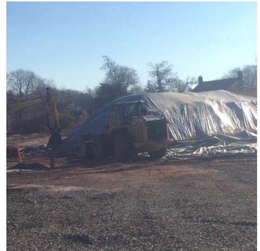
Stockpile covered with poly liner
