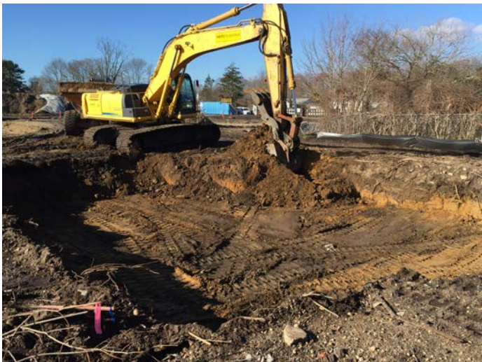
Excavation conducted with Kobelco SK350 in Area 19 cell EOB to 3' BGS (left picture) and completed excavation in Area 19 cells EOA and EOB to 3' BGS (right picture).
