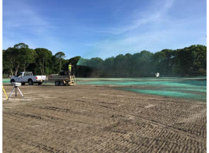
Hydroseed mix being prepared (left picture). Hydroseeding observed (right picture).
