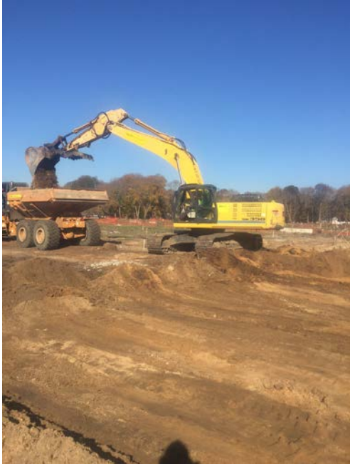
Kobelco SK350 Excavator and End Dump excavating 1 feet of material from cell Q9 (left picture) and soil stockpile being shaped by the JD744K (right picture).
