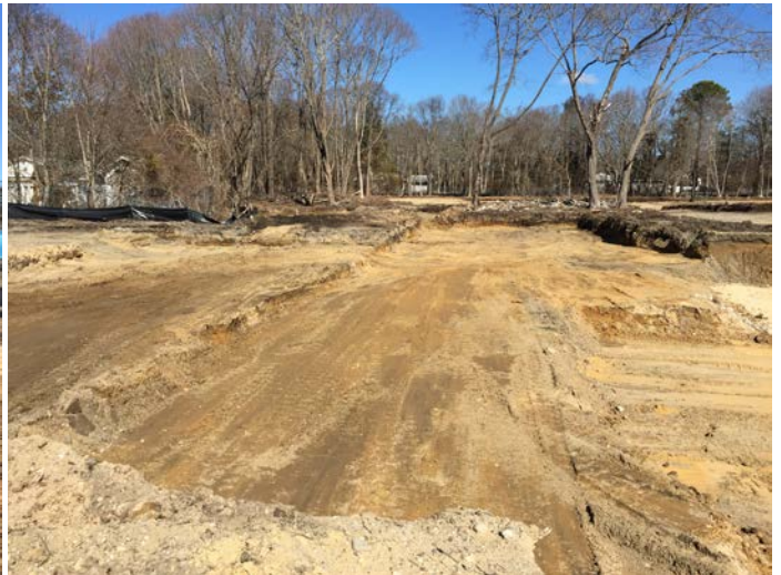
Excavation conducted with Kobelco SK350 in Area 15 cell D2 to 2' BGS (left picture). Completed excavation in Area 15 cells D1 and D2 to 2' BGS and cells E1 and half of E2 to 3' BGS (right picture).
