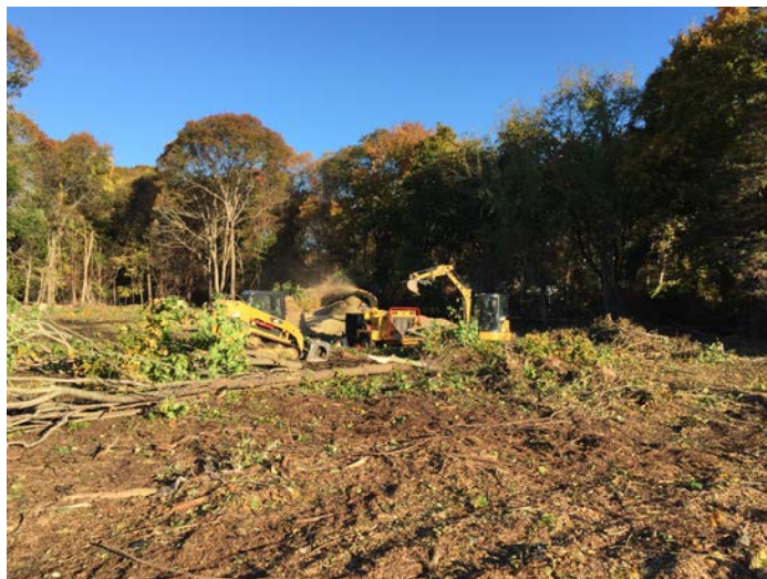
Wood chipping conducted with the CAT 279C and the CAT 304E.
