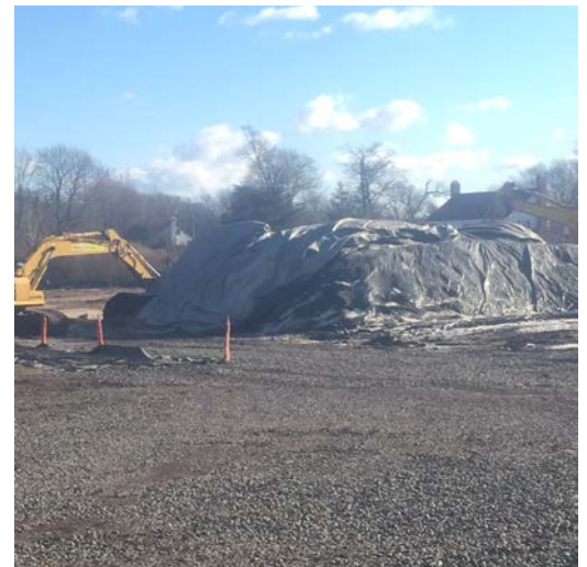
JD-744K loader loading truck with stockpiled soil (left picture) and stockpile covered with poly liner before leaving the site (right picture).
