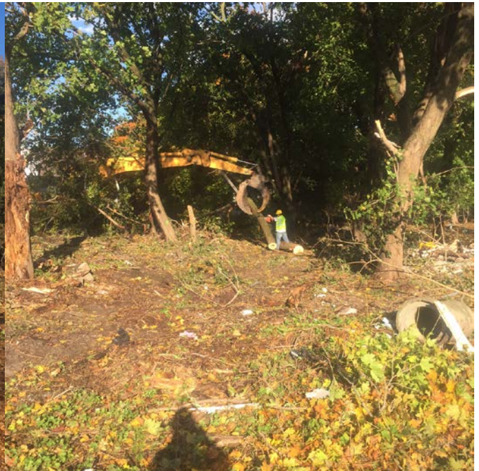
Tree cutting with chainsaw and the Liebherr 904
