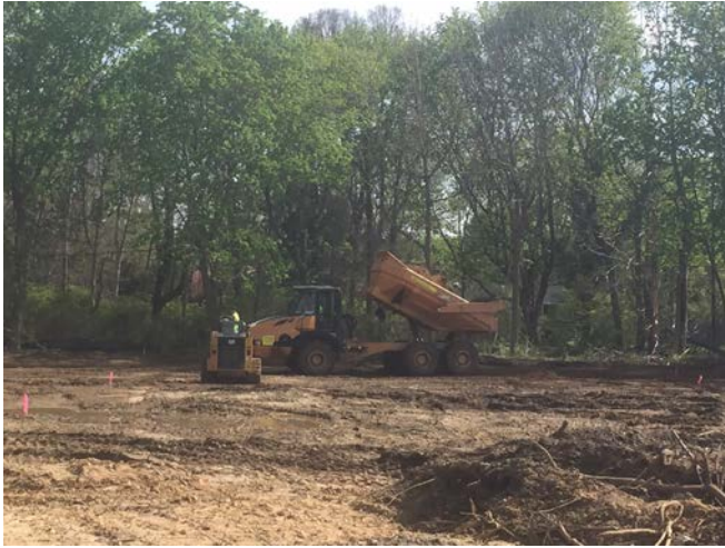
Backfilling/regrading observed in Area 19 (left picture) and the JD-750J bulldozer regrading in Area 19 (right picture).
