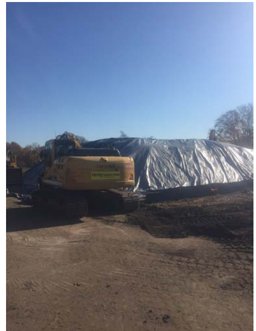
Excavated Soil Stockpile covered with the Supreme UV tarp and secured at end of day.
