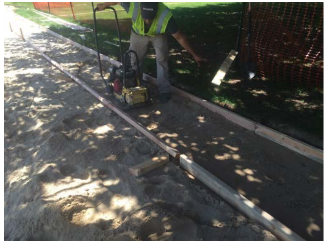
Concrete form work construction observed (left picture). Compaction observed on common fill material in form area (right picture).
