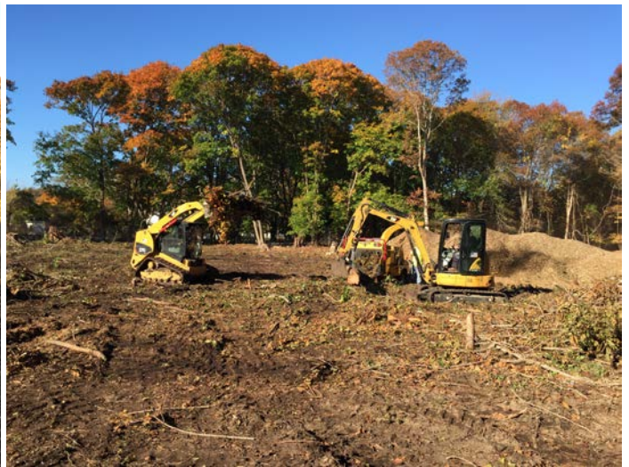
Tree/wood debris and smaller tree trunk gathering for wood chipping with the CAT 304E Excavator and CAT 279C Compact Track Loader.
