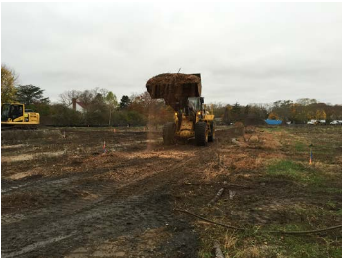
JD744K Front End Loader spreading woodchips along temporary haul road.
