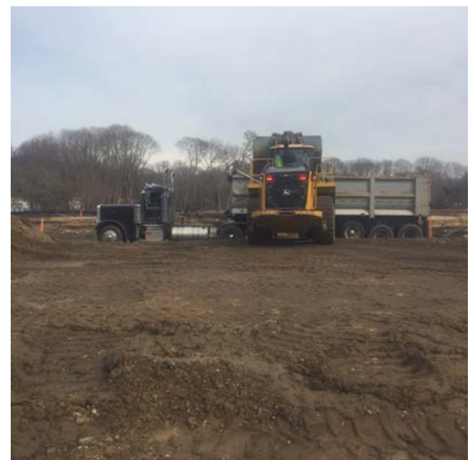
End dump placing excavated material into the stockpile (left picture). JD-744K loader loading a truck from the stockpile (right picture).
