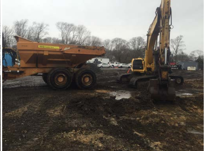
End dump placing excavated material into the stockpile (left picture) and excavation conducted in Area 16 in cell B6 to 1' BGS (right picture).
