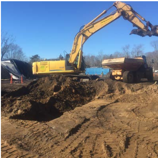
Excavation conducted in Area 14 cell F5 to 1-2' BGS (left picture) and JD-744K loader used to load trucks from the stockpile (right picture).
