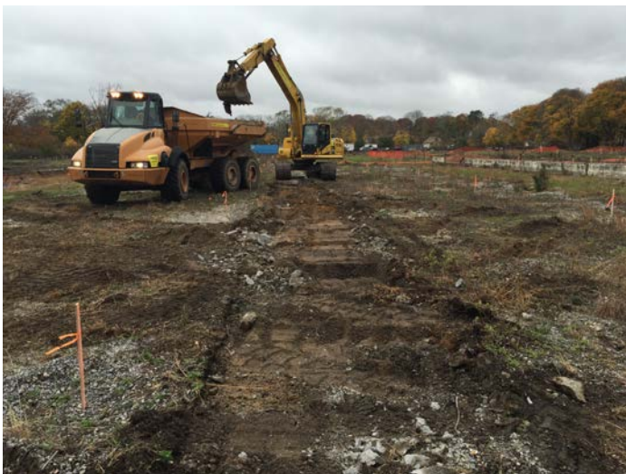
PC210 Excavator and End Dump removing concrete from cells Q7 – T7.
