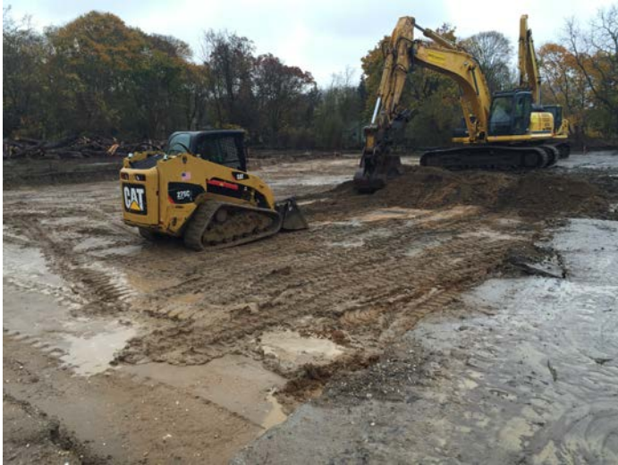
Kobelco SK250 Excavator and CAT 279C Compact Track Loader excavating 2 feet of material from cells V7 and V8.
