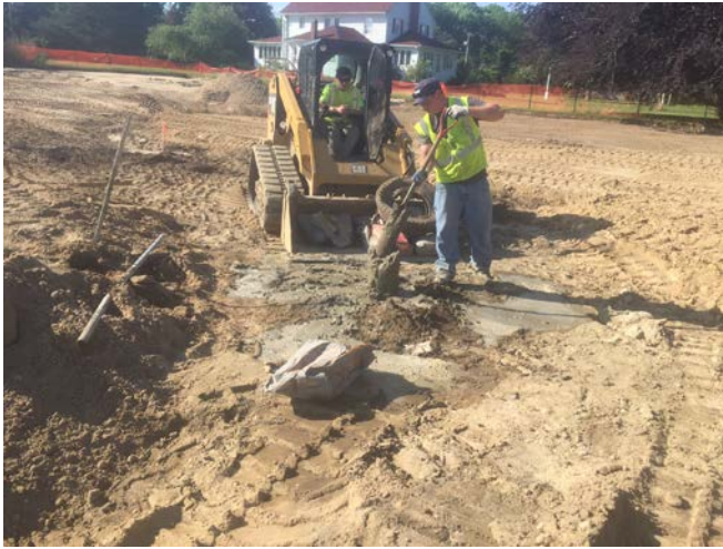
Irrigation well being filled with concrete (left picture). Regrading continued in Area 11 (right picture).
