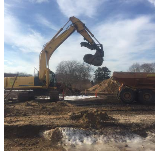
Excavation conducted in Area 14 cell H5 to 5' BGS (left and right pictures).
