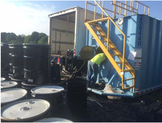
Metro Environmental conducting frac tank cleanout (left picture). End dump loaded with regrading material in Area 8 (right picture).
