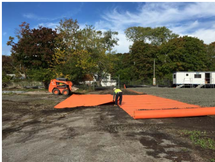
EnviroTrac installing construction entrance tracking pad.
