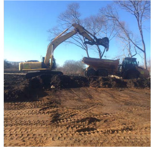
End dump placing excavated material into the stockpile (left picture) and excavation being conducted in Area 19 cell FOF to 1' BGS(right picture).
