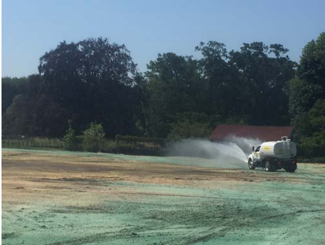
Water truck watering the already hydroseeded areas (left picture). Hydroseed mix being prepared (right picture).
