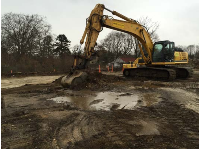
Excavation conducted in Area 9 cell G10 with Kobelco SK350 to 2' BGS (left picture) and excavation conducted in Area 10 cell F10 to 6' BGS (right picture).
