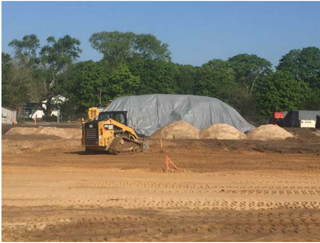
CAT-279D grading regrading material in Area 16 (left picture). Kobelco SK-350 loading regrading material into the end dump in Area 9 (right picture).
