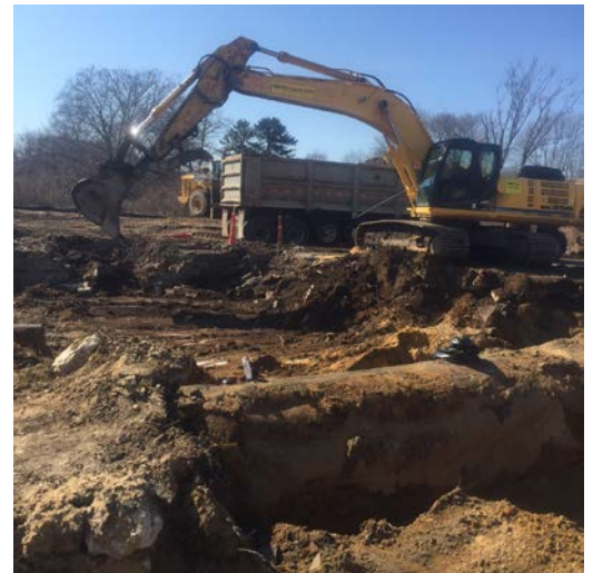
Small container of suspected fuel oil liquid that was removed from the UST (left picture). Excavation conducted in Area 9 cell G7 to 1'BGS and to expose UST (right picture).
