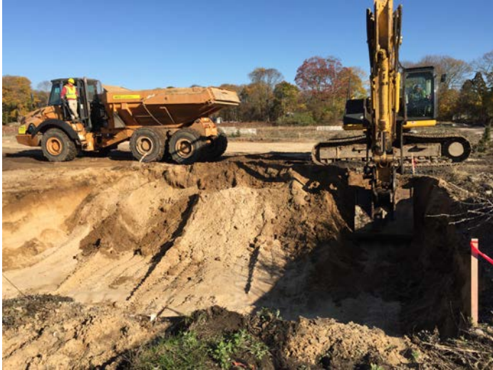
Kobelco SK250 Excavator and End Dump excavating 5 feet of material from cell T10 (left picture) and excavating 3 feet of material from cell T9 (right picture).
