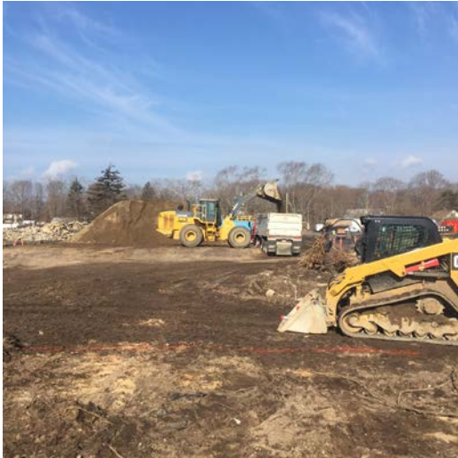
Truck being loaded using the JD-744K loader from the stockpile (left picture) and excavation conducted in Area 4 cell J10 to 5' BGS
