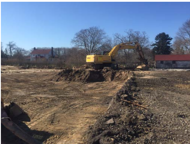
Excavation conducted in Area 11 the remaining half of cell D10 to 1' BGS (left picture). Loaded truck utilizing the onsite scale (right picture).
