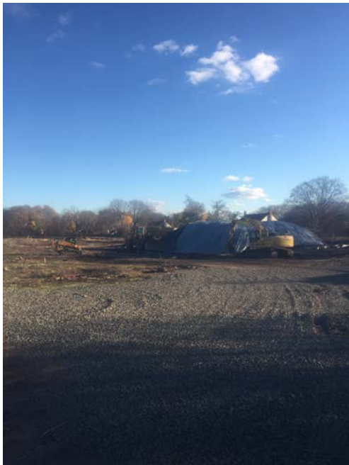
EnviroTrac covered the stockpile with the Supreme UV tarp and secured it to the ground
