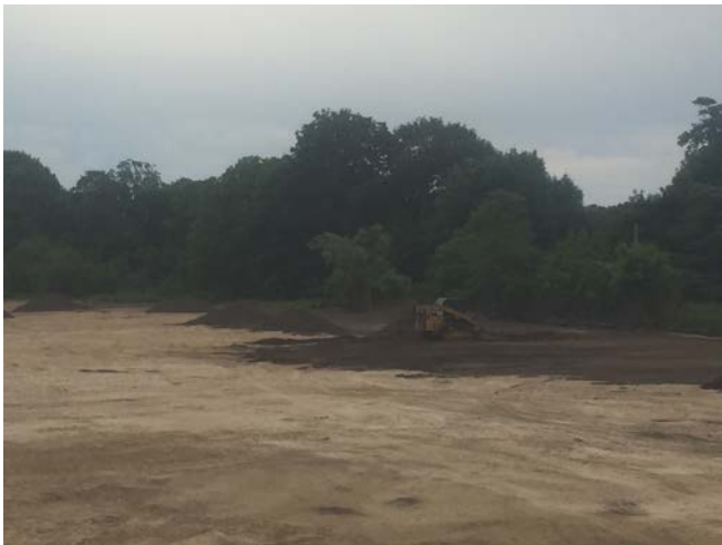
Topsoil being spread in Area 5 (left picture). Topsoil spread in Area 15. Topsoil being delivered to stockpile. End dump loaded from the stockpile (right picture).
