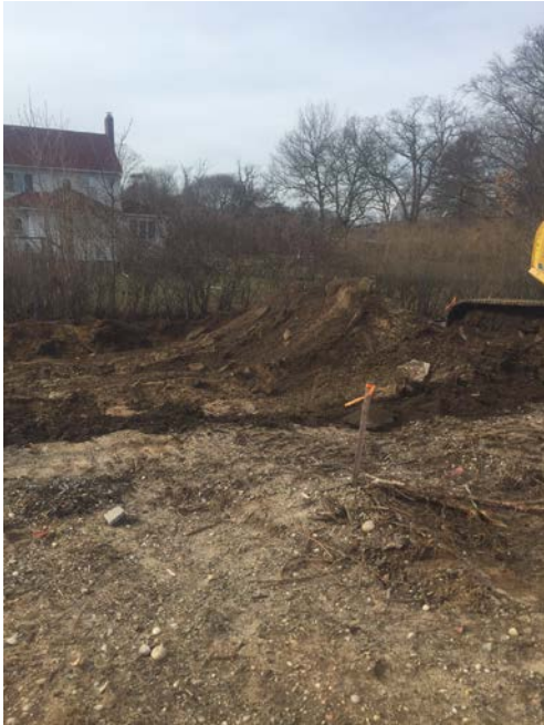
Excavation conducted in Area 5 cell I12 with Kobelco SK350 to 1' BGS (left picture) and excavation conducted in Area 5 cell H11 to 1' BGS
