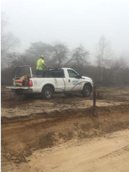
Grout being pumped into MW-02 for decommissioning (left picture) and casing being pulled using CAT 279C skid steer (right picture).
