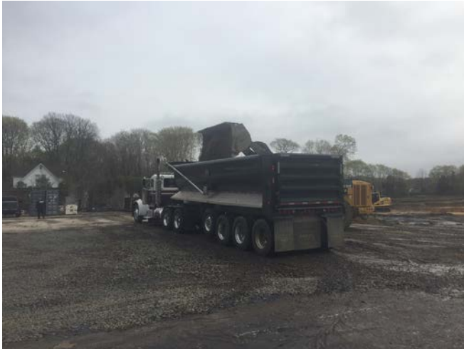
Truck being loaded from the stockpile using the JD-744K loader (left picture) and excavation observed in Area 11 cell AA12 to 3' BGS (right picture).
