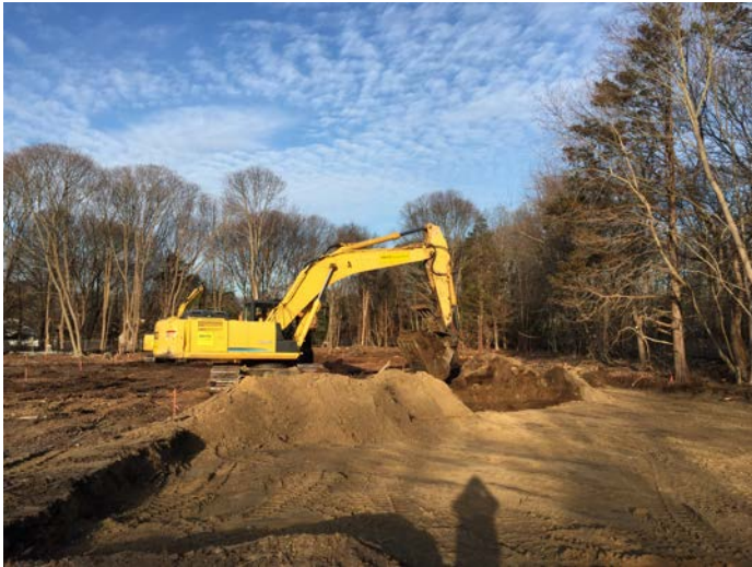
Excavation conducted with Kobelco SK350 in Area 18 cell IOI to 1' BGS (left picture) and excavation conducted in Area 19 cell GOI to 1' BGS (right picture).
