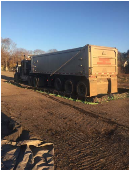
Trucks decontaminated prior to being scaled and exiting the site.
