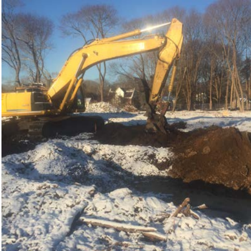
Excavation conducted in Area 18 cell IOF to 1' BGS (left picture) and excavation conducted in Area 17 cell MOC to 1' BGS (right picture).
