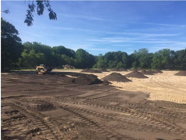
Onsite topsoil being placed spread in Areas 6 and 7 (left picture). 100 privet hedges delivered to the site (right picture).
