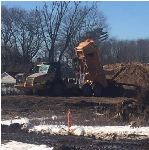
End dump placing material from cell J4 into the stockpile (left picture) and truck being weighed using the onsite scale (right picture).
