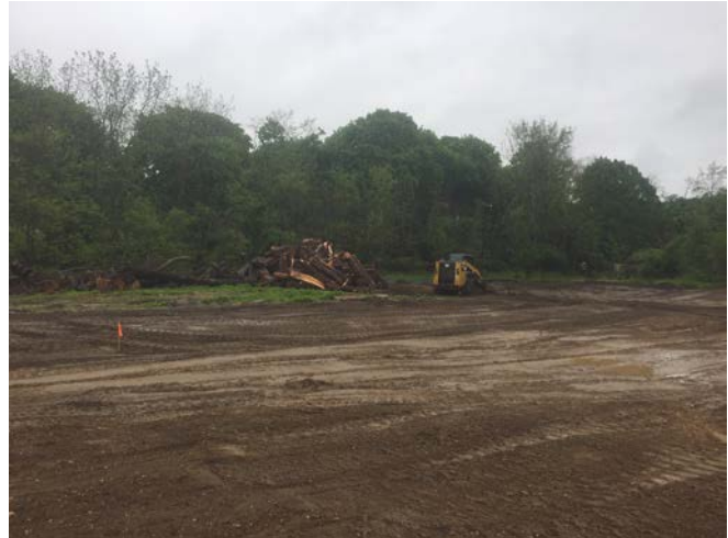
End dump loading with backfill material in Area 9 (left picture). CAT-279D grading in Area 1 as well as consolidating wood debris (right picture).
