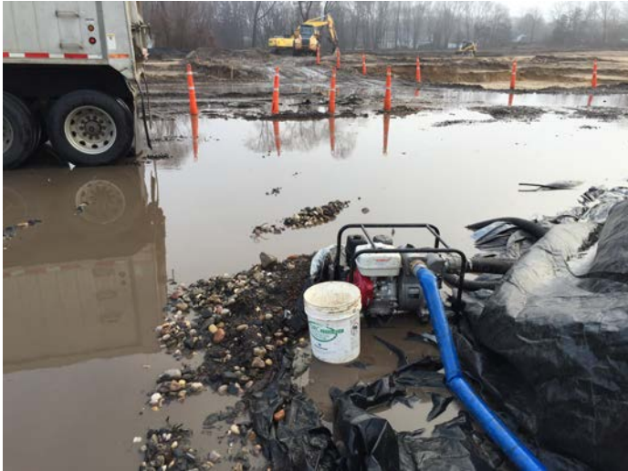
Dewatering conducted in the truck loading and Decontamination Pad areas (left picture). JD 744K loading trucks from the Excavated Soil Stockpile (right picture).
