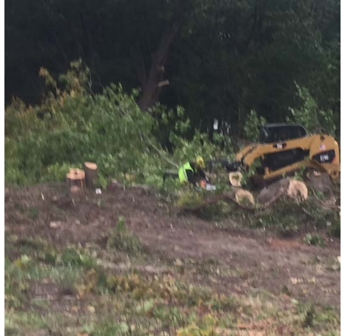
Tree cutting with chainsaw and the CAT 279C
