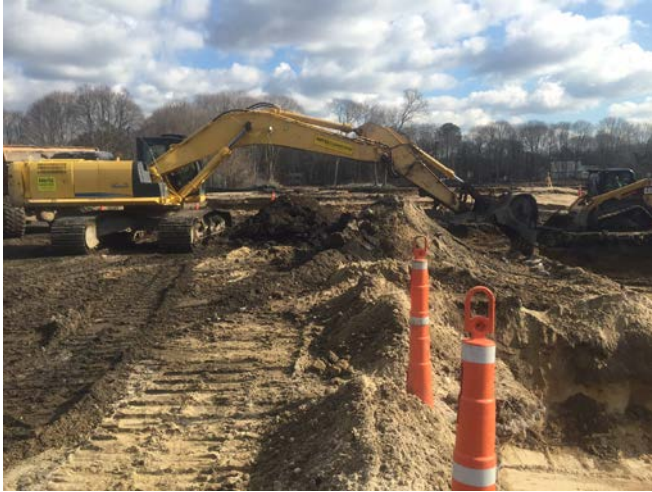
Excavation conducted in Area 10 in cell E9 with Kobelco SK350 to 1' BGS (left picture) and truck being loaded using the JD-744K loader (right picture).
