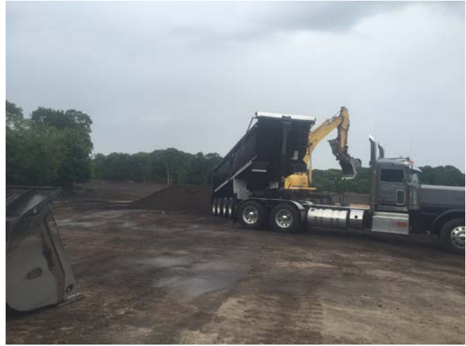
Topsoil placed and spread in Area 15 (left picture). Topsoil delivered to the site and placed in the stockpile (right picture).
