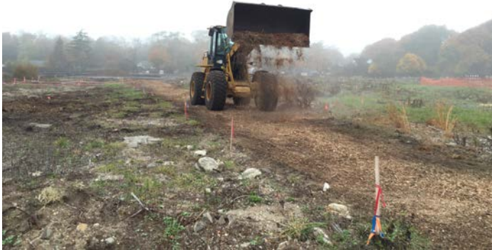
CAT 930H Front End Loader spreading woodchips along the temporary access road.
