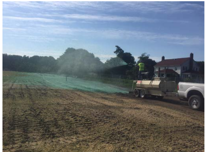
Hydroseeding observed (left picture). Hydroseeding observed (right picture).
