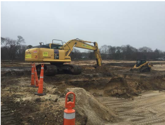
Excavation conducted in Area 10 cell F9 to 3' BGS (left picture). Truck being loaded using the JD-744K loader (right picture).
