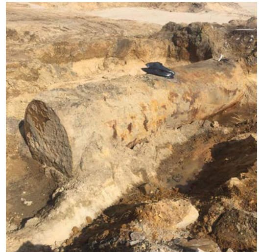
Excavation conducted in Area 4 cell J9 to 4-5' BGS (left picture). The exposed UST that is scheduled to be removed tomorrow (right picture).
