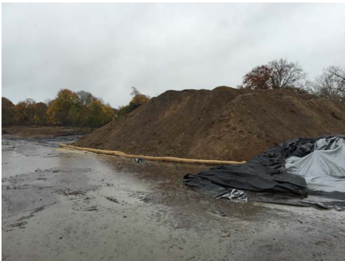
Installed straw wattles along the northern side of the Excavated Soil Stockpile.
