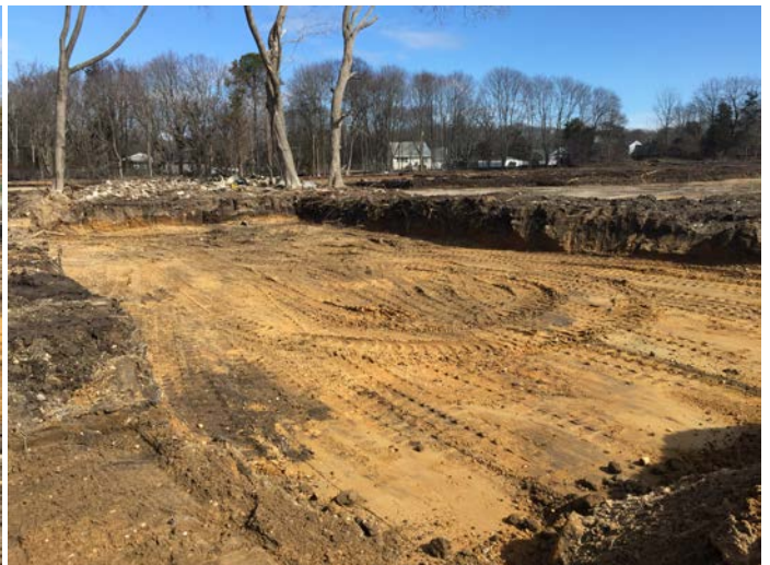
Excavation conducted with Kobelco SK350 in Area 19 cell EOB to 3' BGS (left picture) and completed excavation in Area 19 cells EOA and EOB to 3' BGS (right picture).
