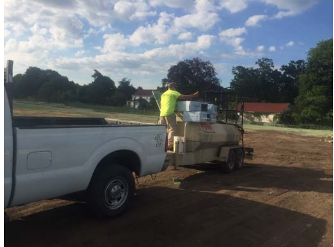
Water truck controlling dust and watering the already hydroseeded areas (left picture). Hydroseed mix being prepared (right picture).
