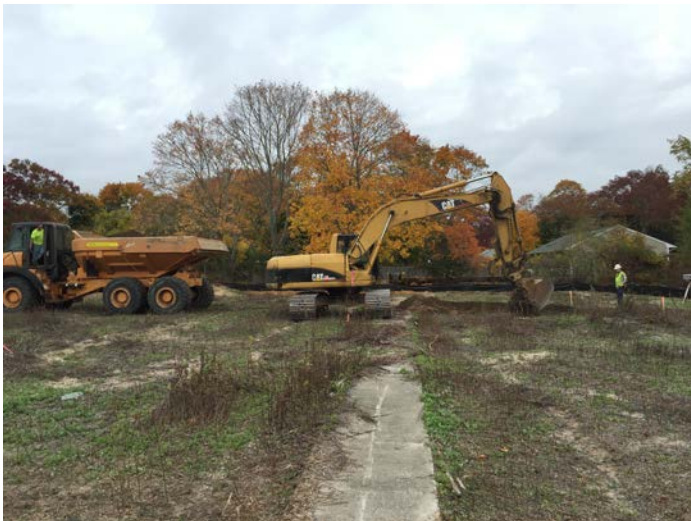
CAT 320 Excavator and End Dump excavating 1 foot of material from cell Y5.
