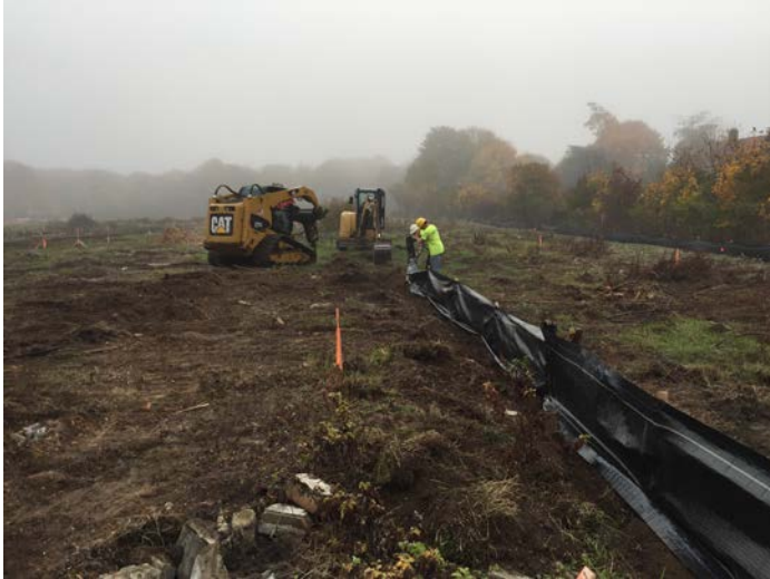
CAT 304E Excavator and CAT 279C Compact Track Loader installing silt fence on the southern side of the stockpile.
