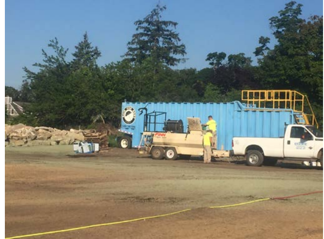
Water truck watering the already hydroseeded areas (left picture). Hydroseed mix being prepared (right picture).
