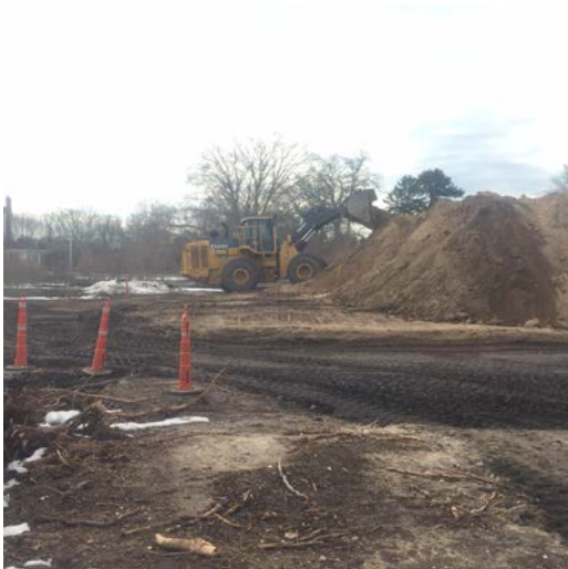
JD-744K loader used to maintain soil stockpile (left picture) and CAT 279C skid steer used to fine grade the excavation of cell H5 (right picture).
