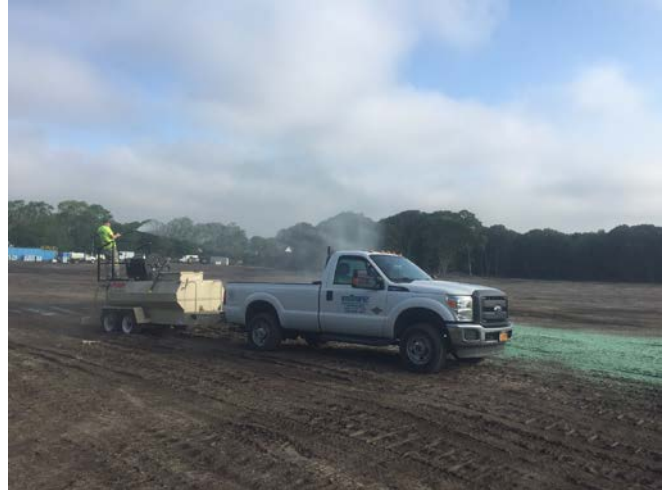
Hydroseed mix being prepared (left picture). Fertilizer mix applied to areas sprayed without fertilizer yesterday (right picture).
