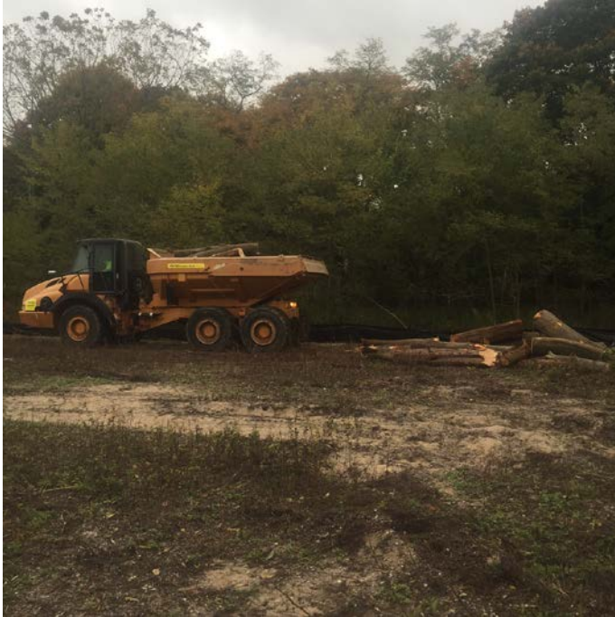
End dump used to relocate tree trunk pile to south-eastern most portion of site.
