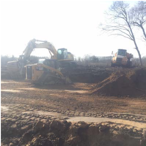
End dump placing excavated material into the stockpile (left picture) and excavation being conducted in Area 19 cell GOG to 1' BGS(right picture).
