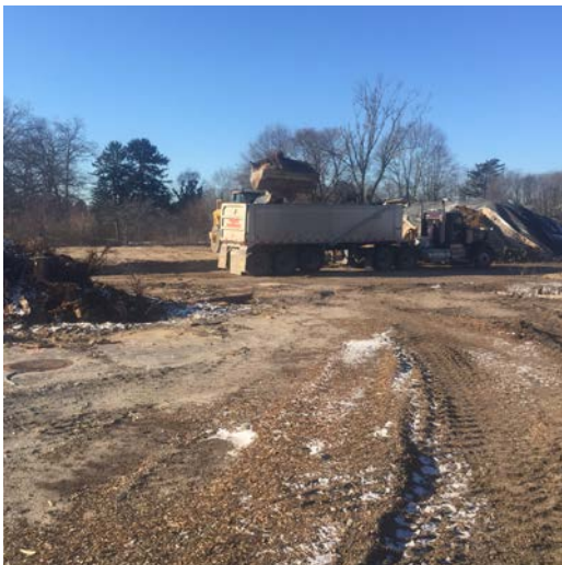
JD-744K loader loading truck with stockpiled soil (left picture) and stockpile covered with poly liner before leaving the site (right picture).
