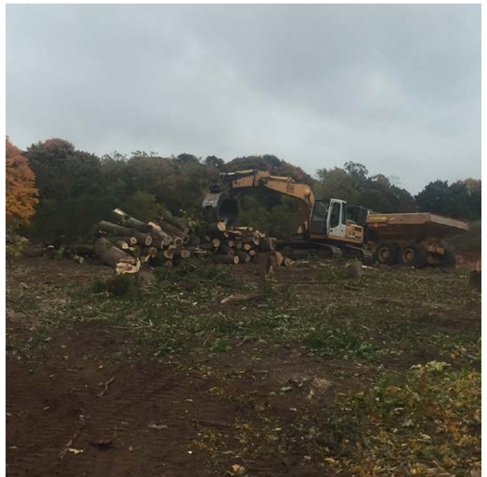
Tree trunks being loaded into end dump with the Liebherr 904.
