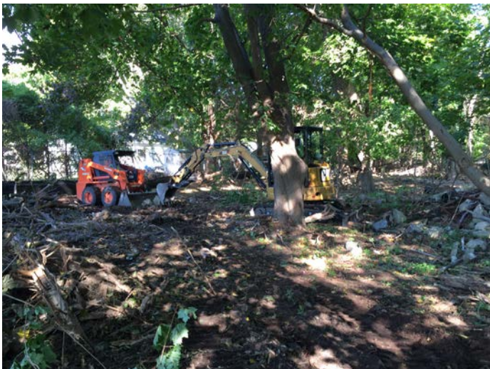
EnviroTrac clearing and grubbing northern portion of the site.
