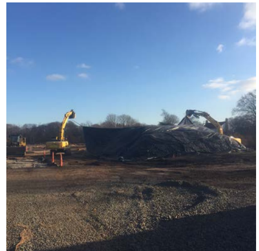
Stockpile covered with poly liner
