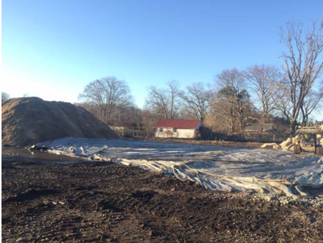
Stockpile poly extended to the west to allow more areas for excavation (left picture). Excavation conducted in Area 9 cell I8 to 3' BGS (right picture).
