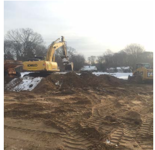
Excavation conducted in Area 8 cell O3 to 1' BGS (left picture) and excavation conducted in Area 8 cell N3 (right picture).
