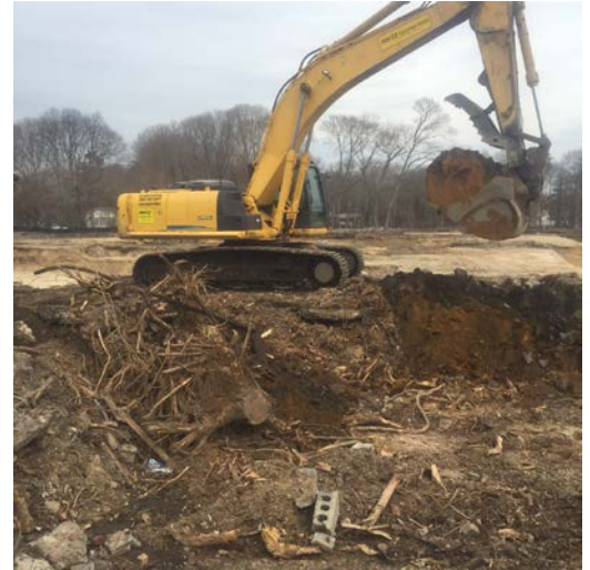
Excavation conducted in Area 15 cell D3 with Kobelco SK350 to 1' BGS (left picture) and excavation conducted in Area 16 cell C4 to 2' BGS.
