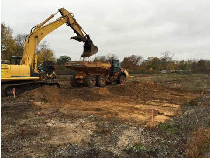
Kobelco SK250 Excavator, CAT 279C Compact Track Loader and End Dump excavating 1 foot of material from cells Q7, Q8, R7, R8, S7, S8, T7 and T8.
