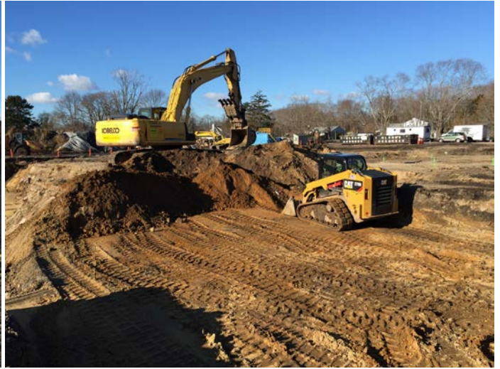
Excavation conducted with Kobelco SK350 and CAT 279D in Area 15 cell E1 to 3' BGS.
