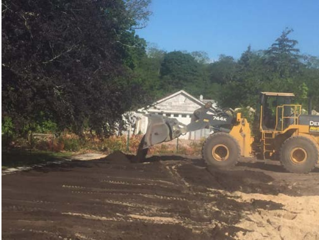
Offsite topsoil being placed to restore Cahill property (left picture). Onsite topsoil being delivered to the site (right picture).
