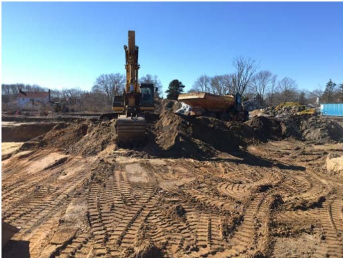
Excavation conducted with Kobelco SK350 in Area 15 cell D2 to 2' BGS (left picture). Completed excavation in Area 15 cells D1 and D2 to 2' BGS and cells E1 and half of E2 to 3' BGS (right picture).
