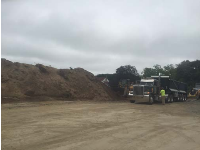
Truck being loaded from the stockpile using the JD-744K loader (left picture). Regrading material placed in Area 4 (right picture).
