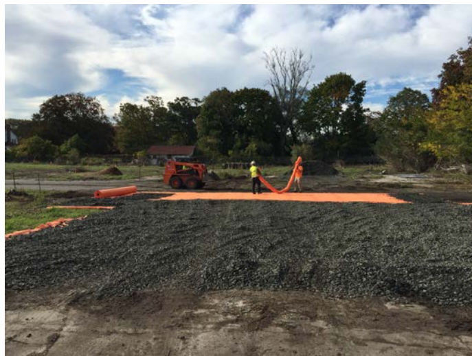
EnviroTrac installing construction entrance tracking pad.
