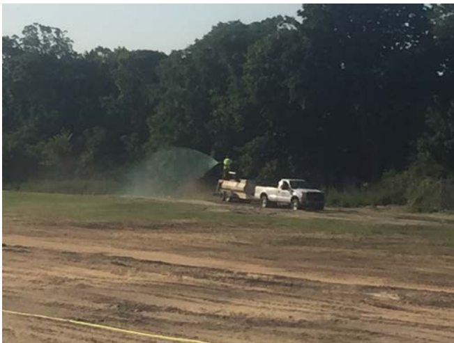
Hydroseeding observed (left picture). Chain link fence repair started at the corner of C0A and D0A (right picture).
