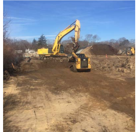
Excavation conducted in Area 5 cell G12 with Kobelco SK350 to 1-3' BGS (left picture) and excavation conducted in Area 5 cell G11 to 2' BGS
