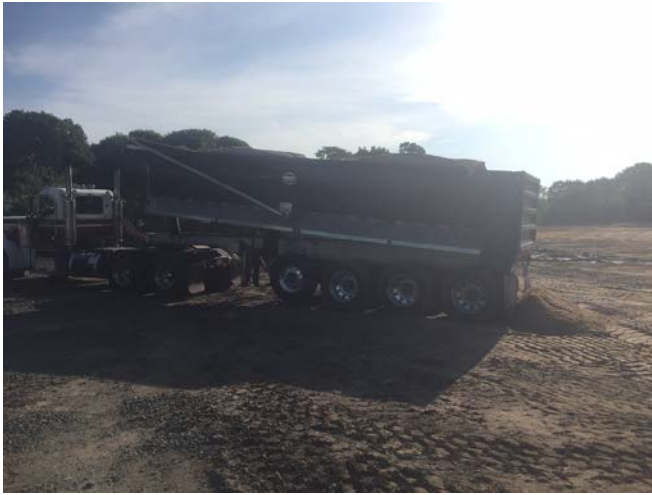
5 loads of common fill sand backfill delivered to the site (left picture). Offsite restoration with the backfill common fill sand observed (right picture).
