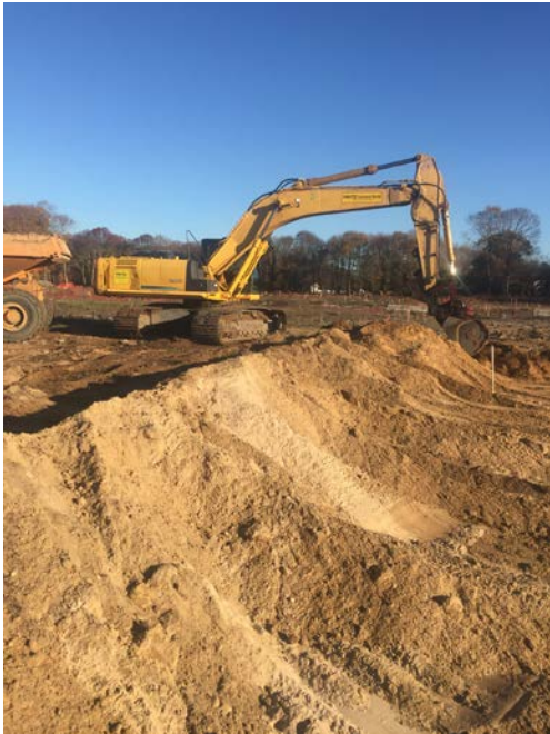
Kobelco SK350 Excavator and End Dump excavating 3 feet of material from cell P9 (left picture) and soil loadout being conducted by the JD744K (right picture).
