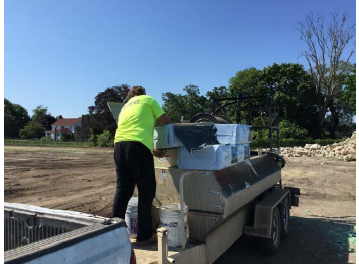
Hydroseeding observed (left picture). Hydroseed mix being prepared (right picture).
