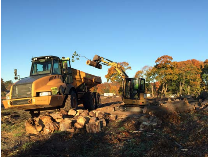
CAT 304E Excavator loading tree trunks into the end dump for relocation in the southeastern most portion of the site.
