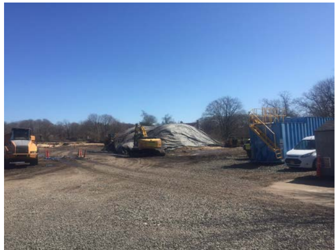
Excavation conducted in Area 4 in the remaining half of cell I9 (left picture). Stockpile covered with poly liner at the end of the day (right picture).
