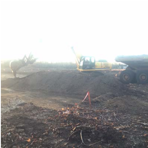
Excavation conducted with Kobelco SK350 in Area 19 cell FOJ to 1' BGS (left picture) and excavation conducted in Area 19 cell DOK to 1' BGS (right picture).
