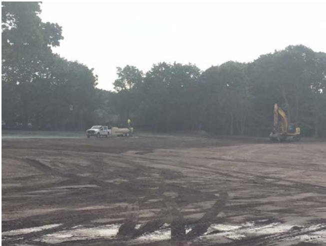
Hydroseeding observed and excavator tracking over topsoil (left picture). Hydroseeding observed (right picture).
