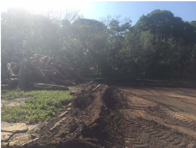
Wood debris moved in Area 1 to allow the overflow to follow the grading plan (left picture). LKMA onsite to survey the regraded areas for the as-built drawings (right picture).
