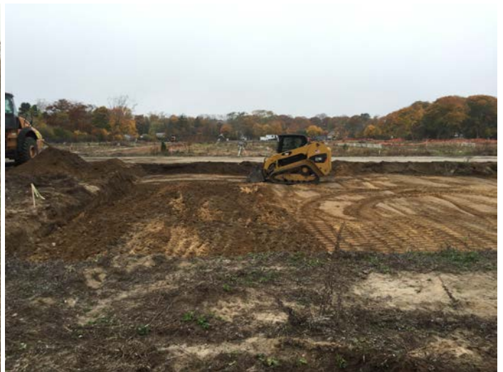
CAT 279C Compact Track Loader excavating 2 feet of material from cells W7 and W8.
