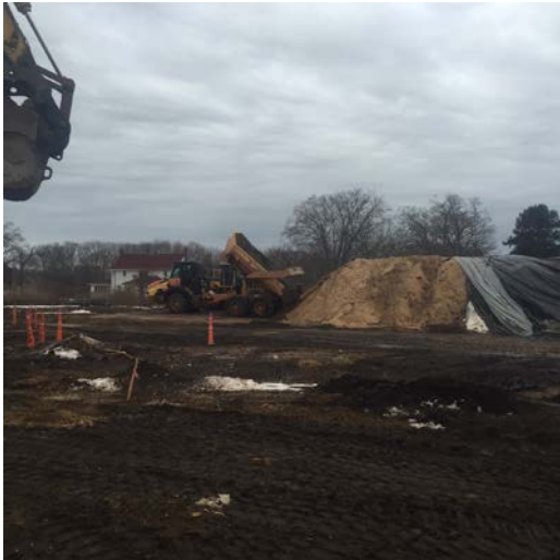
End dump placing excavated material into the stockpile (left picture) and base sample B-LOC being collected (right picture).
