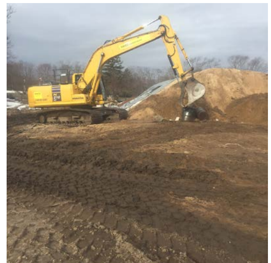
Excavation conducted in Area 16 cell E5 to 4' BGS (left picture) and some of the onsite drum from previous site activities crushed and disposed of with the outgoing stockpile soil (right picture).
