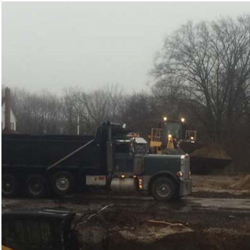
Truck loaded using the JD-744K loader from the stockpile (left picture) and excavation observed in Area 16 half of cell E6 to 4' BGS (right picture).
