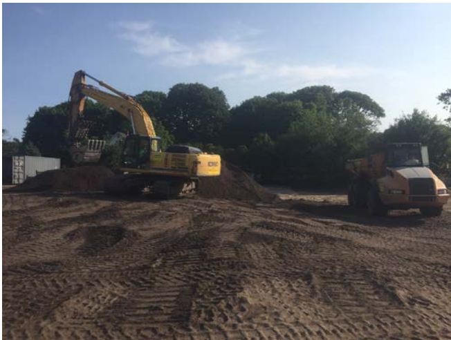
Topsoil being loaded into the end dump for placement (left picture). Topsoil spread in Areas 7 and 8 (right picture).
