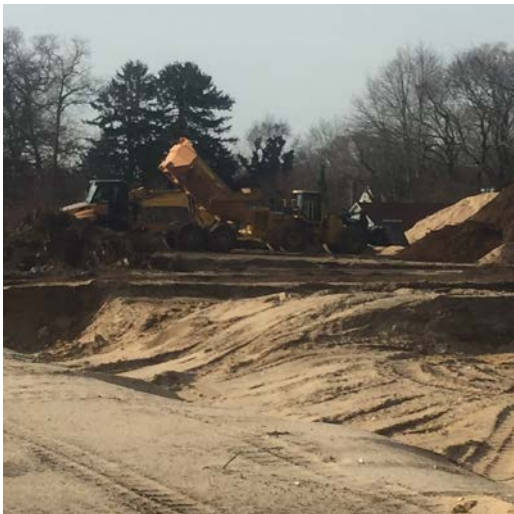
End dump placing material in stockpile and JD-744K loader maintaining stockpile (left picture) and excavation observed in Area 18 cell IOG to 1' BGS (right picture).
