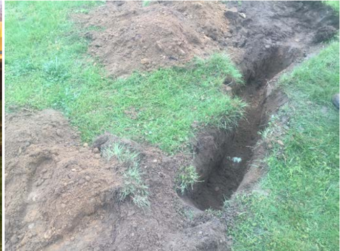
Hand excavation conducted to locate septic tank and line (left picture) and PVC septic pipe located (right picture).
