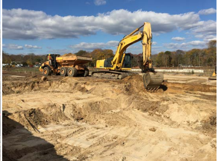
Kobelco SK250 Excavator and End Dump excavating 5 feet of material from cell T10 (left picture) and excavating 3 feet of material from cell T9 (right picture).
