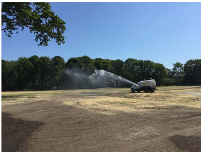
Hydroseed mix being prepared (left picture). Watering hydroseeded areas (right picture).
