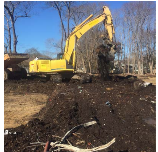
End dump placing excavated material into the stockpile (left picture) and excavation being conducted in Area 19 cell FOF to 1' BGS(right picture).
