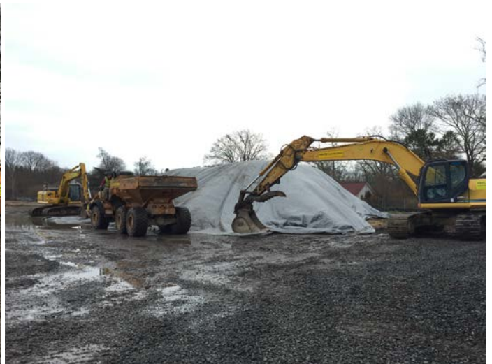
End dump placing excavated material into the stockpile (left picture). Stockpile covered with poly-liner and secured to the ground after completion of work (right picture).
