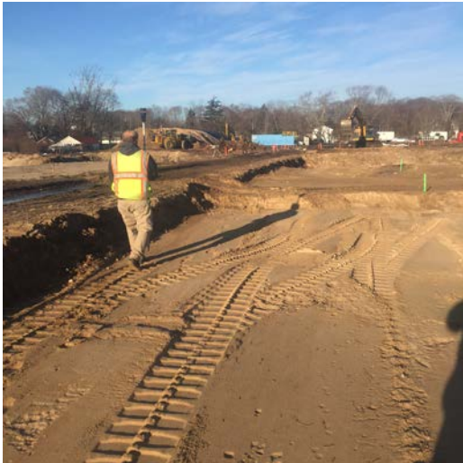
L.K. McLean Associates (LKMA) onsite to survey cut grades and lay out sample locations (left picture) and excavation conducted in Area 14 cell G5 to 1' BGS(right picture).
