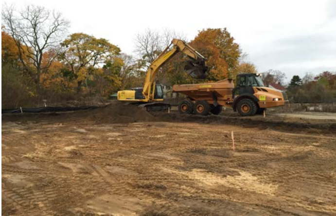
Kobelco SK250 Excavator and End Dump excavating 2 feet of material from cell W12.
