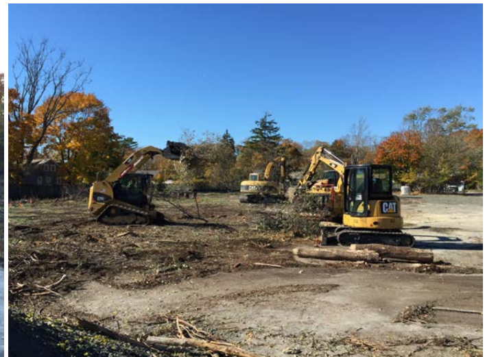
Bush debris and other vegetative brush gathering for wood chipping with the CAT 304E Excavator and CAT 279C Compact Track Loader.
