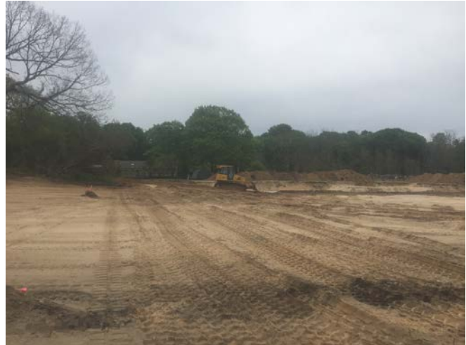
Regrading observed in Area 8 (left picture). Regrading observed in Areas 6 and 7 (right picture).
