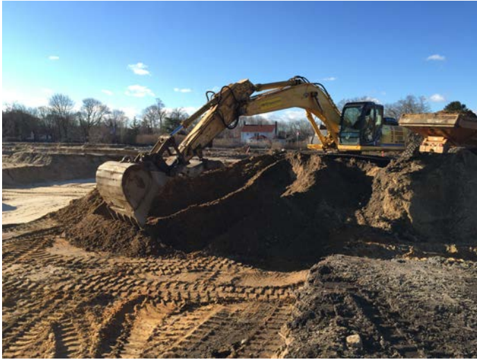
Excavation conducted with Kobelco SK350 and CAT 279D in Area 15 cell E1 to 3' BGS.
