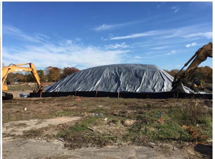
Excavated Soil Stockpile covered with the Supreme UV tarp and secured at end of day.
