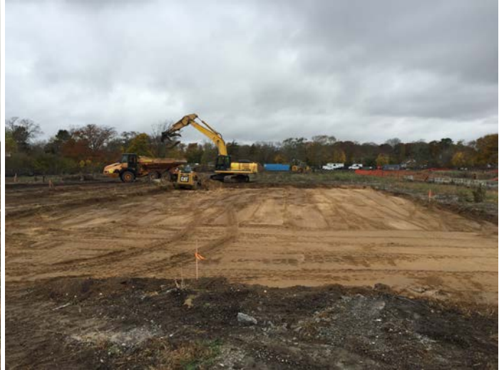
Kobelco SK250 Excavator, CAT 279C Compact Track Loader and End Dump excavating 1 foot of material from cells Q7, Q8, R7, R8, S7, S8, T7 and T8.
