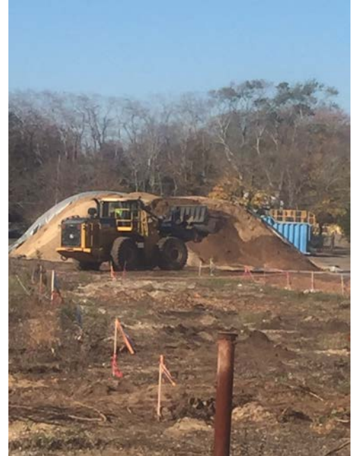
Kobelco SK350 Excavator and End Dump excavating 1 feet of material from cell Q9 (left picture) and soil stockpile being shaped by the JD744K (right picture).
