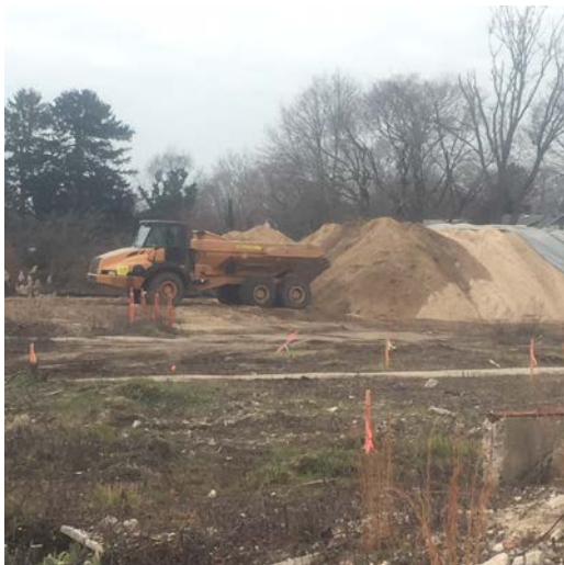
End dump placing material in stockpile
