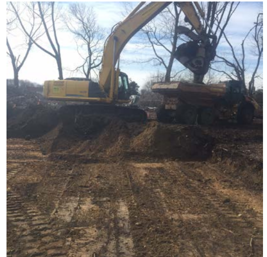
End dump placing excavated material into the stockpile (left picture) and excavation being conducted in Area 19 cell GOG to 1' BGS(right picture).
