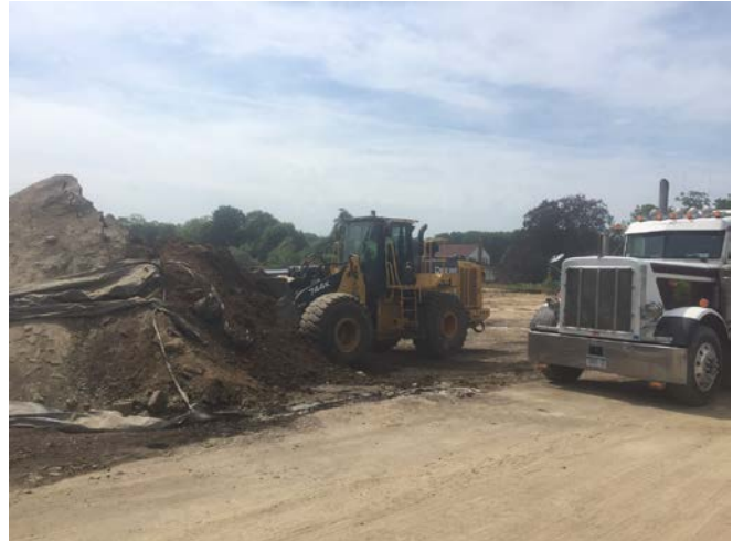
Offsite topsoil being spread in cells I13 and I14 (left picture). Truck being loaded from the stockpile using the JD-744K loader (right picture).
