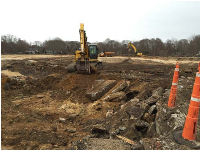
Concrete removed from cells E6 and F6 and placed in the Concrete Staging Area (left picture). Completed excavation in Area 2 for the additional excavation required per Field Order #7 in cells Q10 and R10 (right picture).
