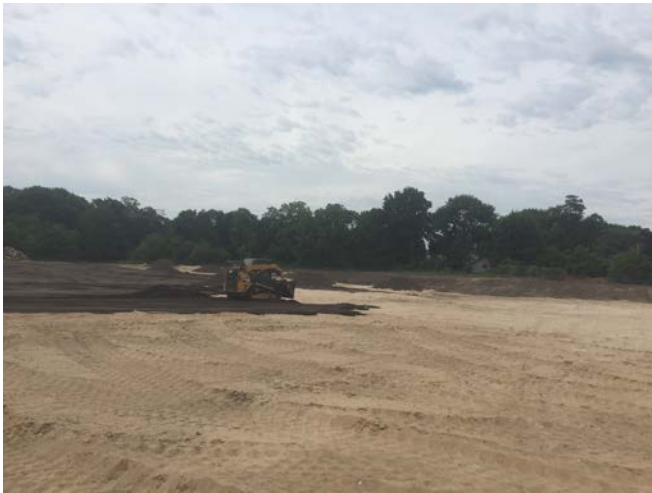
Topsoil spread in Area 9 (left picture). Topsoil being placed and spread in Area 8 (right picture).
