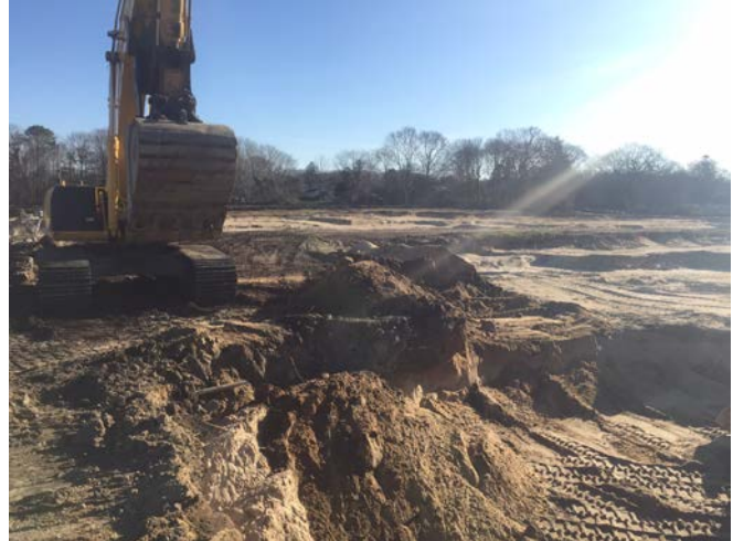
Stockpile poly extended to the west to allow more areas for excavation (left picture). Excavation conducted in Area 9 cell I8 to 3' BGS (right picture).
