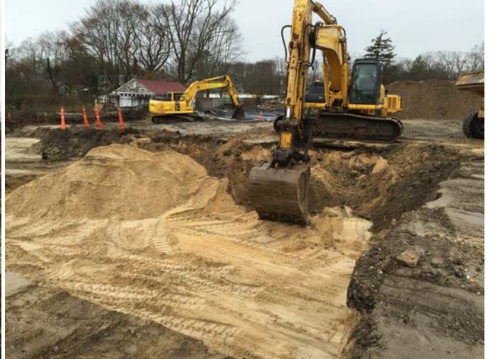
Excavation conducted in Area 9 cell G10 with Kobelco SK350 to 2' BGS (left picture) and excavation conducted in Area 10 cell F10 to 6' BGS (right picture).
