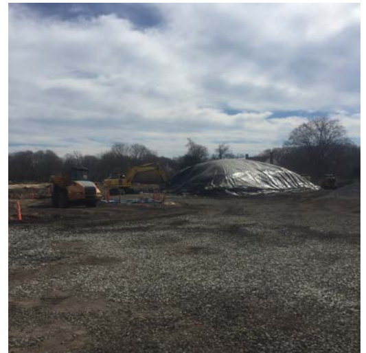
Excavation conducted in Area 2 for the redig per Field Order #7 in cell T7 (left picture). Stockpile covered with poly-liner following the completion of work today (right picture).
