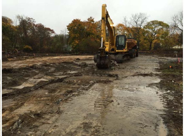
PC210 Excavator and End Dump excavating 4 inches of concrete from cell V8.
