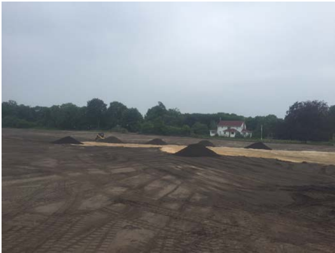
Topsoil being spread in Areas 14 and 16 (left picture). End dump loaded with topsoil from the stockpile (right picture).
