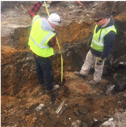
UST first exposed and depth measurement being taken (left picture). Sides of the UST exposed at the end of the day (right picture).
