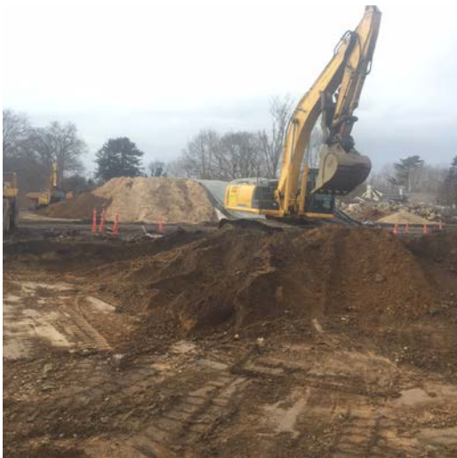
Excavation conducted in Area 16 cell E5 to 4' BGS (left picture) and some of the onsite drum from previous site activities crushed and disposed of with the outgoing stockpile soil (right picture).
