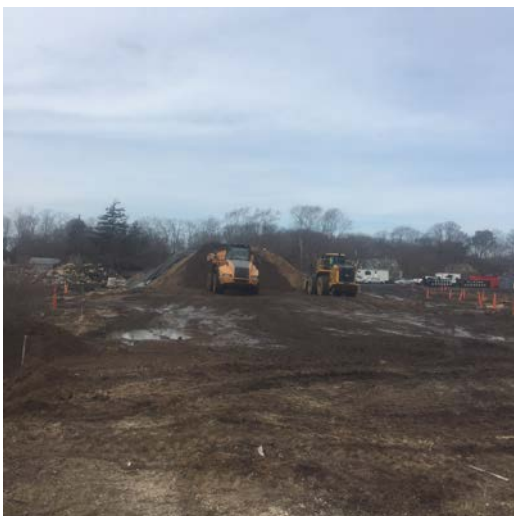
End dump placing excavated material into the stockpile (left picture). JD-744K loader loading a truck from the stockpile (right picture).
