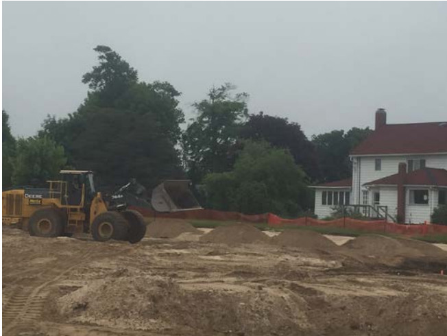
Common fill material used to restore some of the Cahill property excavation area (left picture). Regrading observed in Area 11 (right picture).
