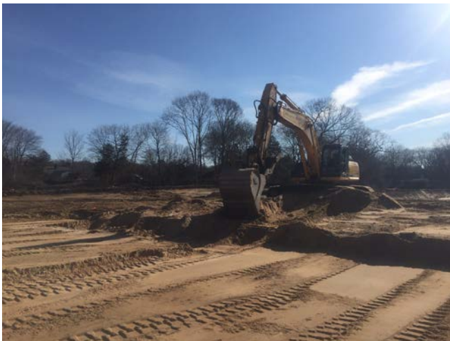
Excavation conducted in Area 13 in cell L1 per Field Order #11 to an additional 1' BGS (left picture). Excavation conducted in Area 8 cell N2 per Field Order #11 to an additional 1' BGS (right picture).
