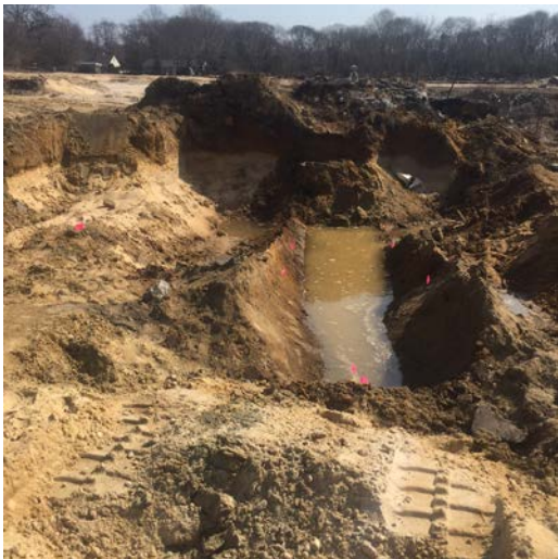
UST area after removal from the excavation area (left picture). The interior of the UST after cleaning (right picture).
