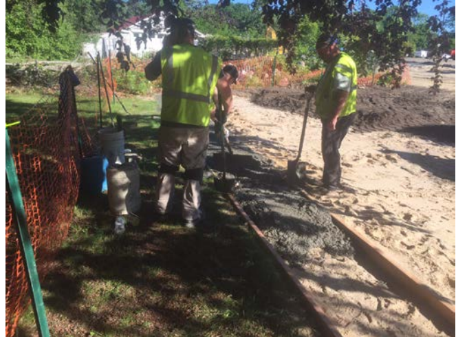
Onsite topsoil being delivered to the site(left picture). Concrete pouring observed in the offsite Cahill property forms (right picture).
