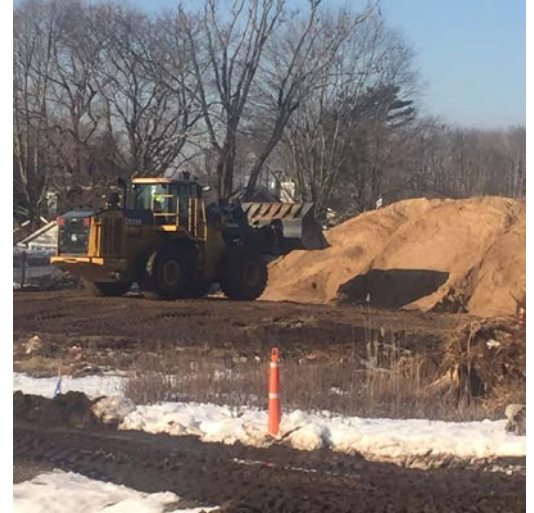
Excavation conducted in Area 8 cell J5 to 4' BGS (left picture) and JD-744K loader maintaining stockpile (right picture).
