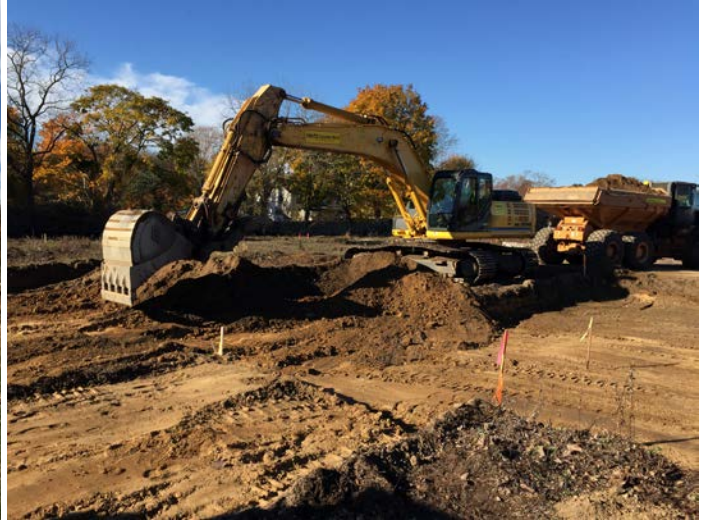
Kobelco SK250 Excavator and End Dump excavating 2 feet of material from cell X10.
