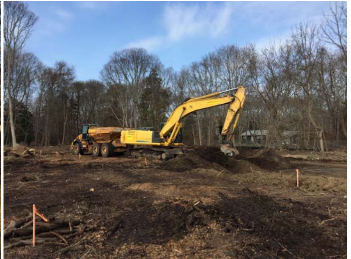
Excavation conducted with Kobelco SK350 in Area 18 cell IOI to 1' BGS (left picture) and excavation conducted in Area 19 cell GOI to 1' BGS (right picture).
