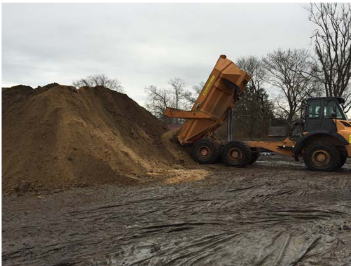
End dump placing excavated material into the stockpile (left picture). Stockpile covered with poly-liner and secured to the ground after completion of work (right picture).
