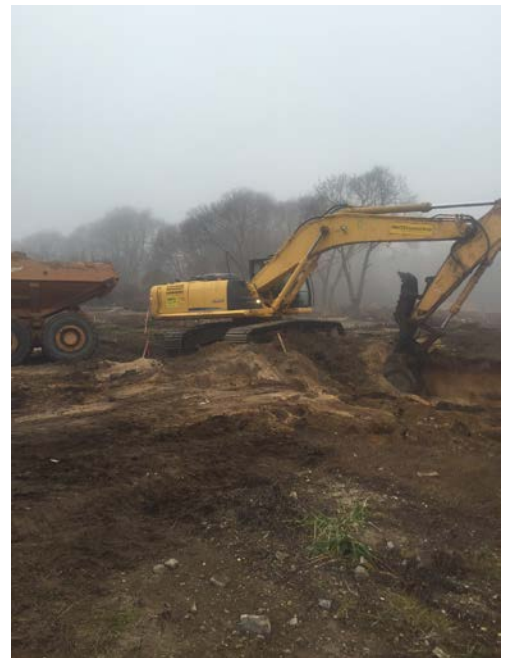
Excavation conducted in Area 14 cell 14 to a depth of 5'
