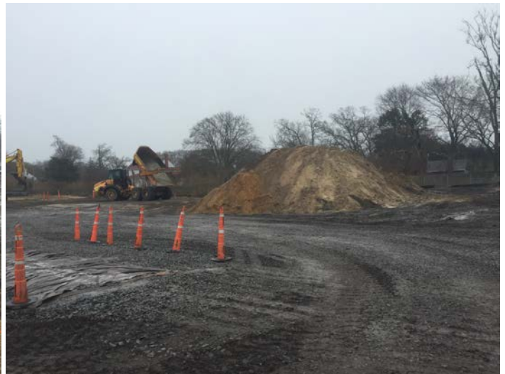
Excavation conducted in Area 10 in cell F9 with Komatsu PC210 to 3' BGS (left picture) end dump placing material in the stockpile (right picture).
