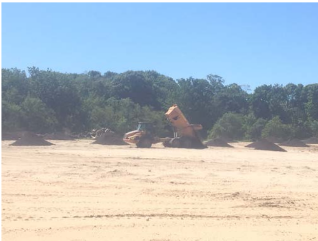
Onsite topsoil being placed in mini-piles in Areas 6 and 7 (left picture). Onsite topsoil being spread in Area 17 (right picture).
