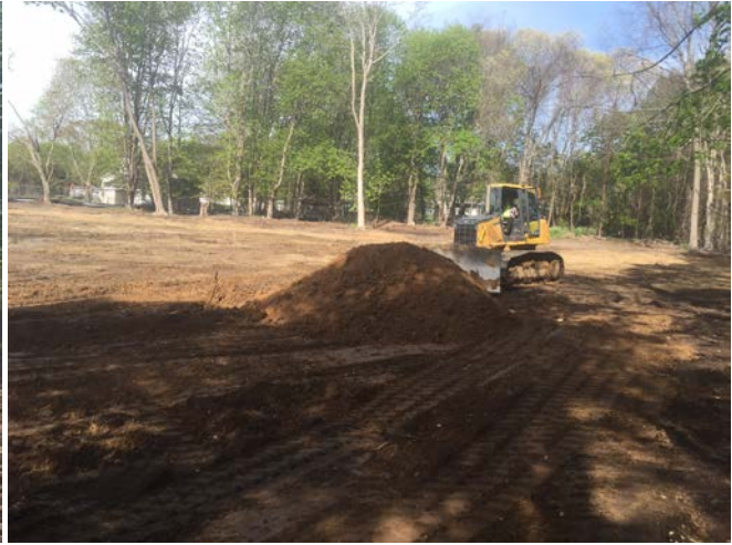
Backfilling/regrading observed in Area 19 (left picture) and the JD-750J bulldozer regrading in Area 19 (right picture).
