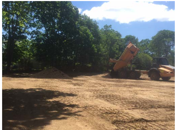
Onsite topsoil being loaded from the new stockpile into the end dump (left picture). End dump placing onsite topsoil in Area 18 (right picture).
