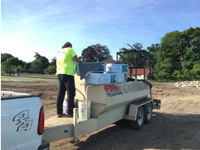
Hydroseed mix being prepared (left picture). Hydroseeding observed (right picture).
