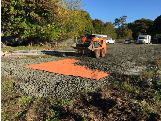
EnviroTrac installing construction entrance tracking pad.
