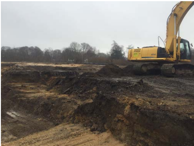
Excavation conducted in Area 11 one quarter of cell D7 to 1' BGS (left picture). Excavation conducted in Area 11 half of cell D10 to 1' BGS (right picture).
