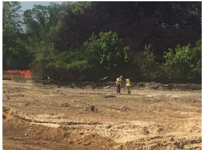
Wood debris moved in Area 1 to allow the overflow to follow the grading plan (left picture). LKMA onsite to survey the regraded areas for the as-built drawings (right picture).
