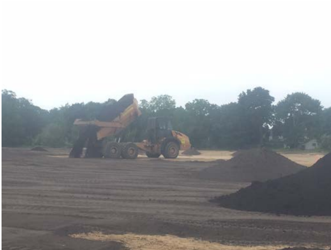
Topsoil placed in Area 17 (left picture). Privet hedges installed in topsoil berm on border between properties (right picture).
