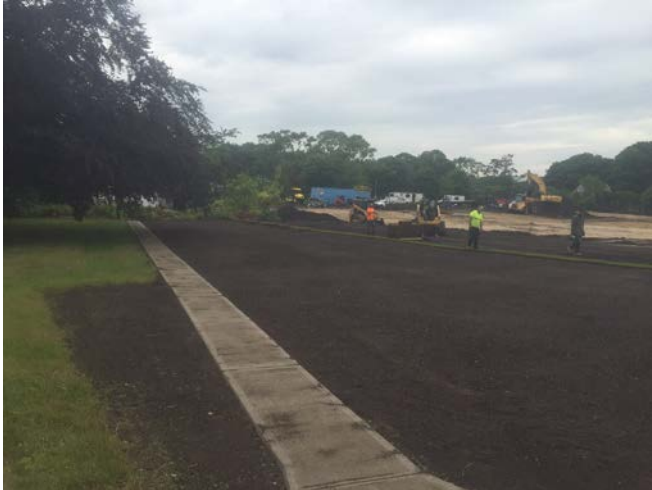
Sod installation started on the offsite property (left picture). Topsoil being delivered to the site and stockpiled (right picture).
