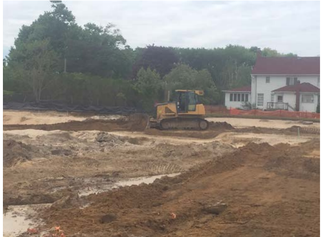
Bulldozer conducting regrading in Area 2 (left picture). Regrading observed in Area 5 (right picture).
