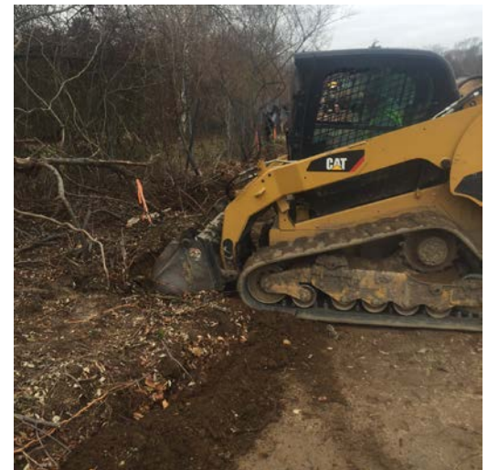
CAT 279C removing small strip of material along fence line.
