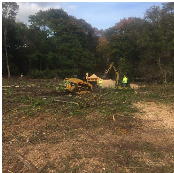
Wood chipper in use with the CAT 304E and 279C
