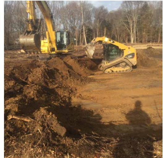
Excavation conducted in Area 18 cell JOG to 1' BGS (left picture) and excavation conducted in Area 18 cell IOH to 1' BGS (right picture).
