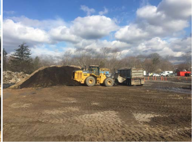
Excavation conducted in Area 10 in cell E9 with Kobelco SK350 to 1' BGS (left picture) and truck being loaded using the JD-744K loader (right picture).
