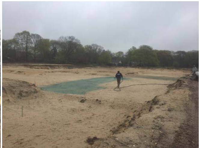
Orange construction fence installed around excavation areas (left picture). Hydroseeding conducted in cells K5 and L5 using the custom seed mix from the specifications (right picture).
