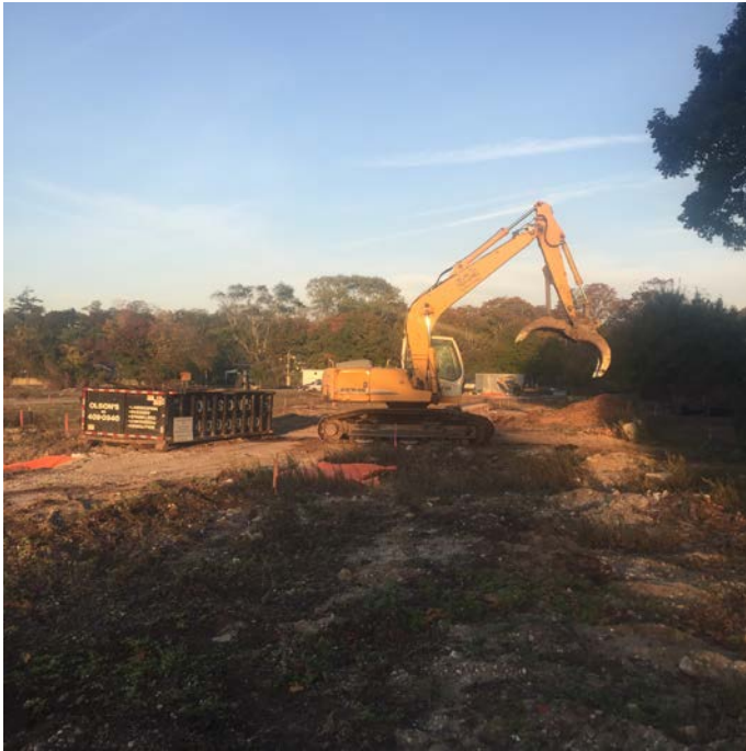
C&D debris loading into roll off container
