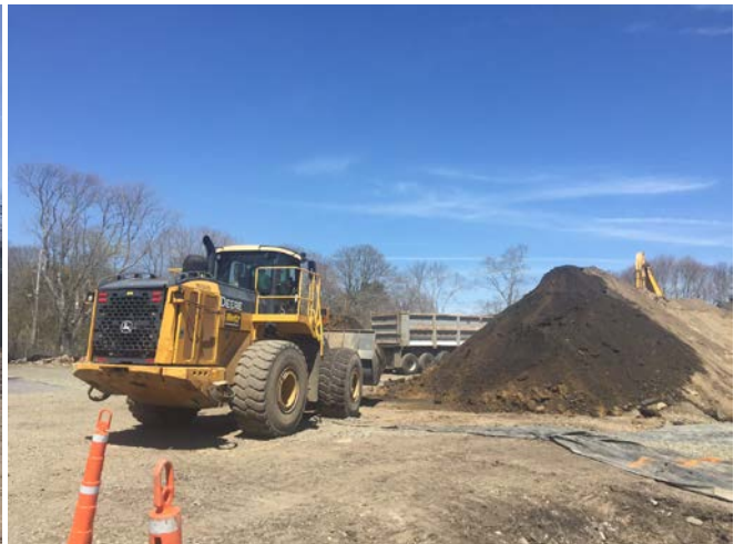
Excavation conducted in Area 11 in half of cell B7 to 1' BGS (left picture). Truck being loaded from the new stockpile using the JD-744K loader (right picture).
