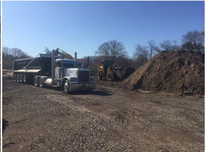
Excavation observed in Area 11 in cell C9 to 1' BGS (left picture) and truck being loaded from the stockpile using the JD-744K loader (right picture).
