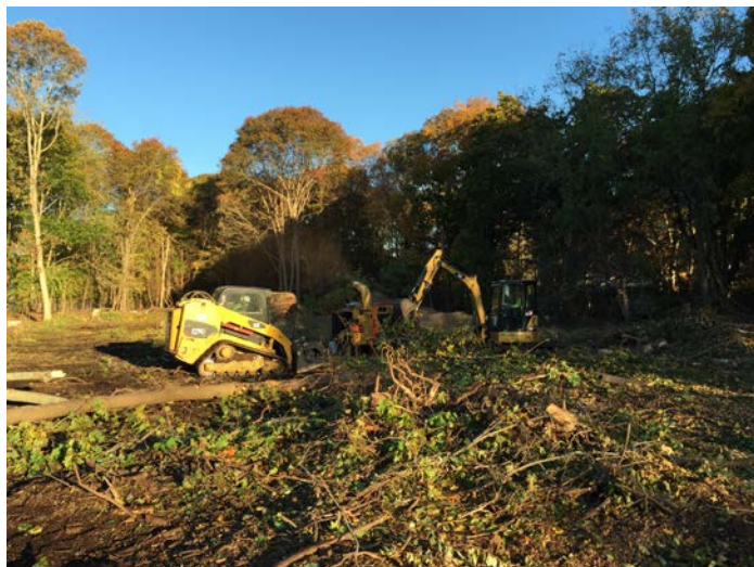
Wood chipping conducted with the CAT 279C and the CAT 304E.
