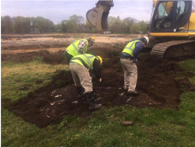
Hand excavation conducted to locate septic tank and line (left picture) and PVC septic pipe located (right picture).
