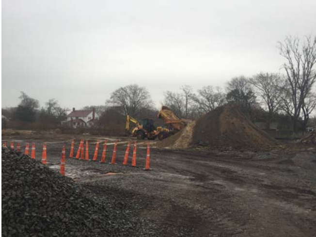
End dump placing excavated material into the stockpile (left picture) and excavation conducted in Area 16 in cell B6 to 1' BGS (right picture).
