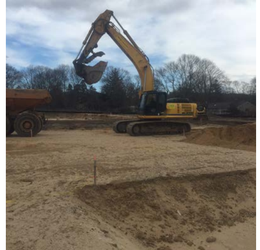
End dump placing excavated material into the stockpile (left picture) and redig excavation conducted in Area 2 cell T8 per Field Order #7(right picture).
