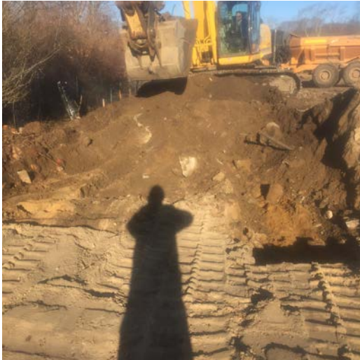
Excavation conducted in Area 5 cell G12 with Kobelco SK350 to 1-3' BGS (left picture) and excavation conducted in Area 5 cell G11 to 2' BGS
