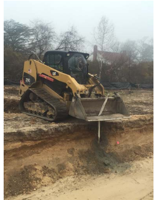
Grout being pumped into MW-02 for decommissioning (left picture) and casing being pulled using CAT 279C skid steer (right picture).
