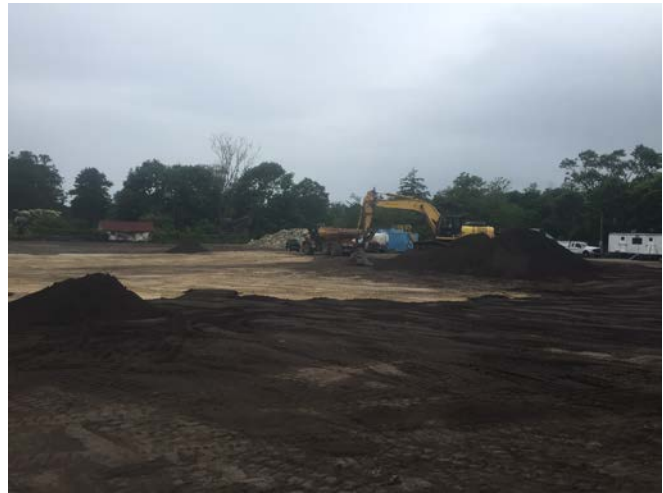
Topsoil being spread in Areas 14 and 16 (left picture). End dump loaded with topsoil from the stockpile (right picture).
