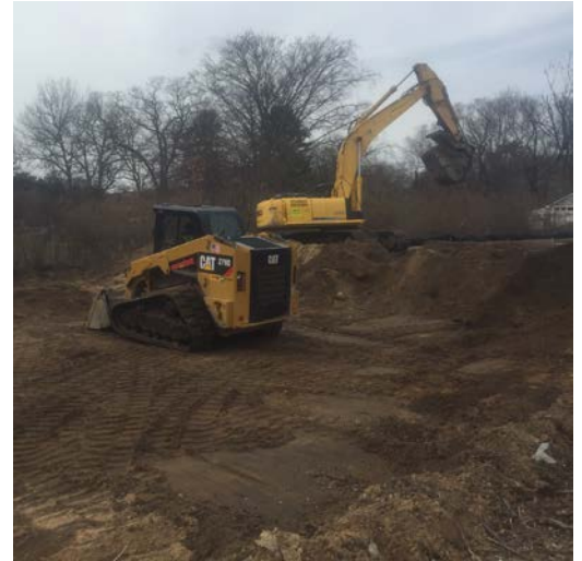
Excavation conducted in Area 5 cell I12 with Kobelco SK350 to 1' BGS (left picture) and excavation conducted in Area 5 cell H11 to 1' BGS
