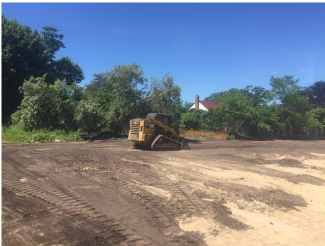
Onsite topsoil being spread in Area 3 (left picture). Onsite topsoil being loaded into end dump and truck delivering onsite topsoil (right picture).
