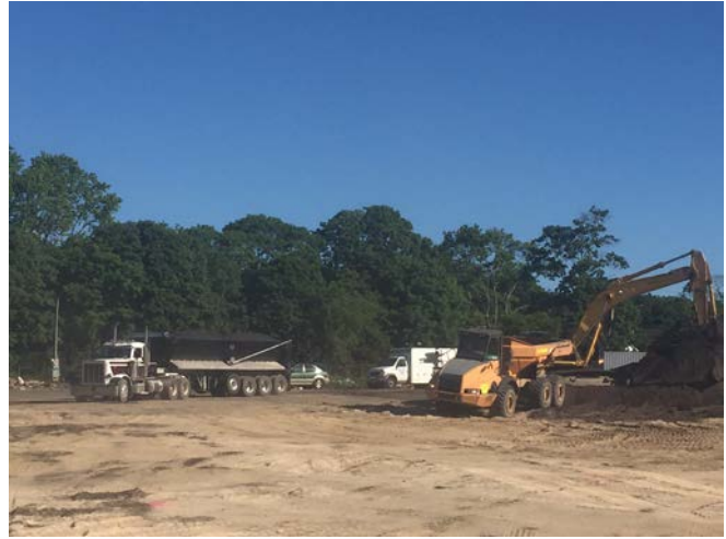
Onsite topsoil being placed spread in Area 5 (left picture). Onsite topsoil being delivered to the site while also being loaded into end dump (right picture).
