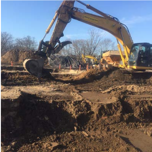
Excavation conducted in Area 15 cell D3 with Kobelco SK350 to 1' BGS (left picture) and excavation conducted in Area 16 cell C4 to 2' BGS.
