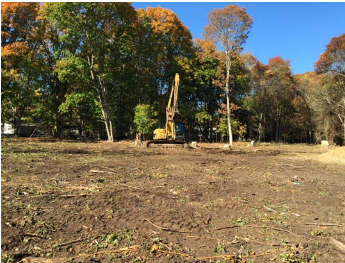
Leveling/rough grading with the CAT 320 Excavator.
