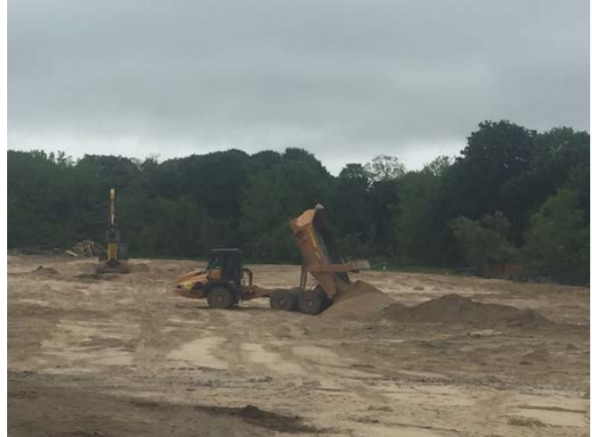
Truck being loaded from the stockpile using the JD-744K loader (left picture). Regrading material placed in Area 4 (right picture).
