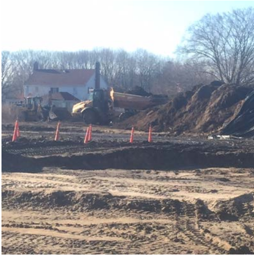
End dump placing excavated material into the stockpile (left picture) and excavation being conducted in Area 19 cell FOF to 1' BGS(right picture).
