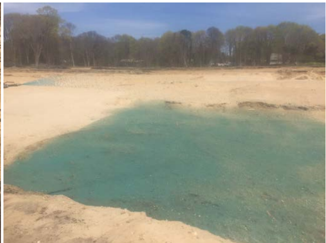
Confirmation sample B-AA11 being collected (left picture). Hydroseeding using Seed Mix A conducted in cell M5 (right picture).
