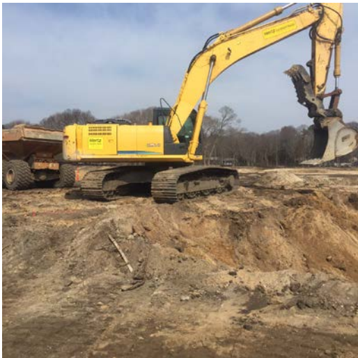
Excavation conducted in Area 4 cell J9 to 4-5' BGS (left picture). The exposed UST that is scheduled to be removed tomorrow (right picture).
