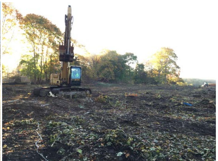
Leveling/rough grading with the CAT 320 Excavator.
