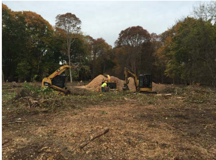
Tree/wood debris and smaller tree trunk gathering for wood chipping with the CAT 279C and the CAT 304E.
