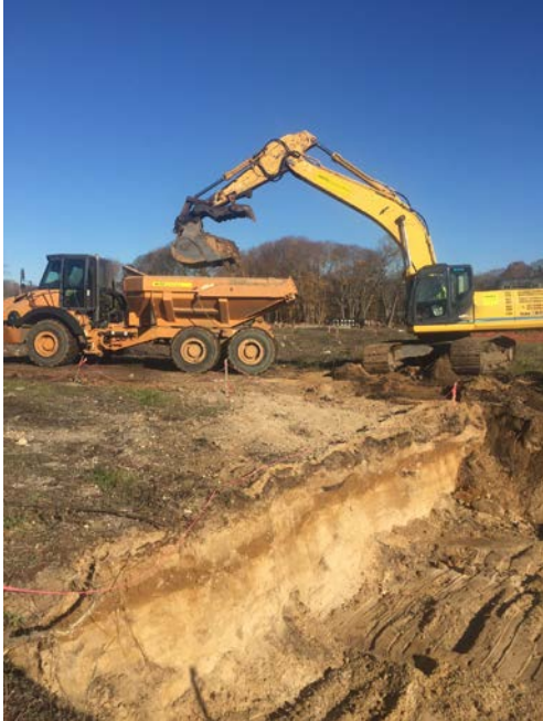
Kobelco SK350 Excavator and End Dump excavating 5 feet of material from cell K9 (left picture) and truck utilizing decontamination pad prior to being weighed. (right picture).
