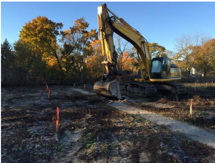
Kobelco SK250 Excavator removing concrete from cell Y10.
