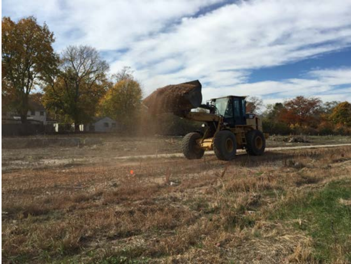
CAT 930H Front End Loader spreading woodchips along the temporary access road.
