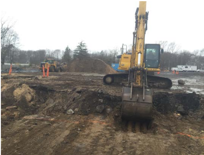
Excavation conducted in Area 10 in cell F9 with Komatsu PC210 to 3' BGS (left picture) end dump placing material in the stockpile (right picture).
