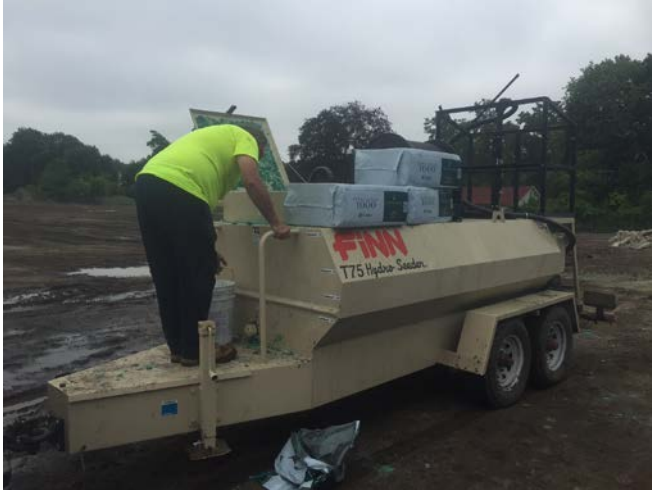
Hydroseed mix being prepared (left picture). Fertilizer mix applied to areas sprayed without fertilizer yesterday (right picture).
