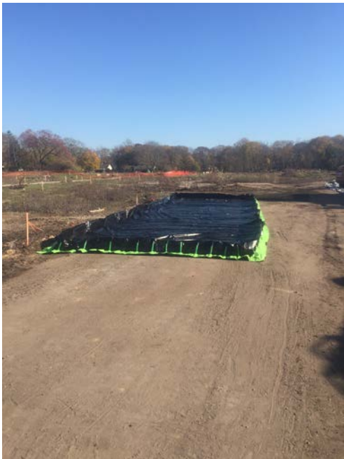
Decontamination pad setup near site entrance to prepare for soil hauling tomorrow.
