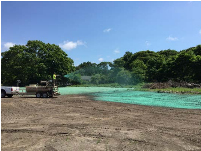
Hydroseeding observed (left picture). Watering hydroseeded areas (right picture).
