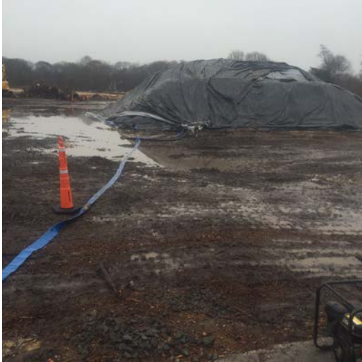
Pump set up to dewater the truck loading area into the frac tank(left picture) and excavation conducted in Area 16 cell D5 to 4' BGS (right picture).
