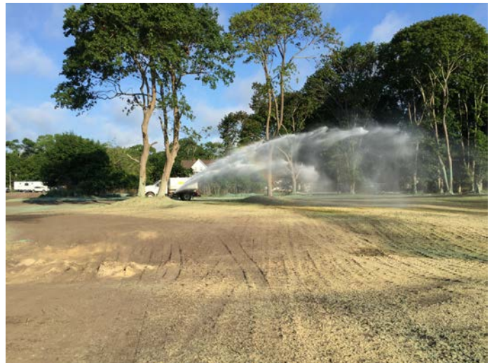
Hydroseeding observed (left picture). Watering hydroseeded areas (right picture).
