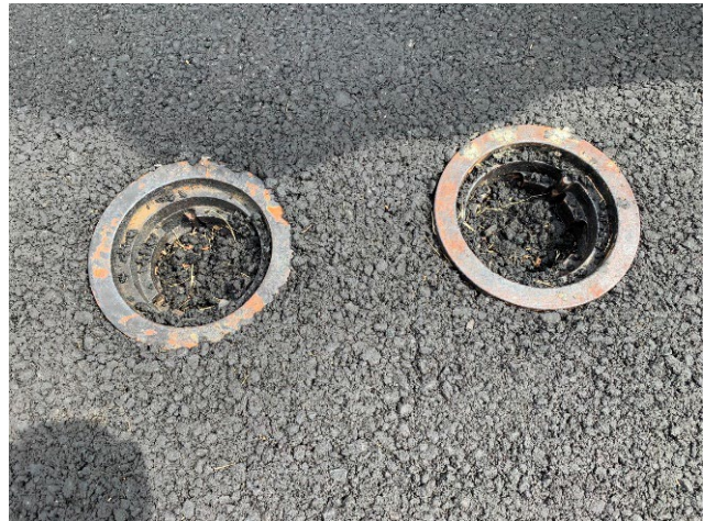
Photo 4: Destroyed off-site monitoring well WO-17 shown adjacent to unidentified utility manhole.
