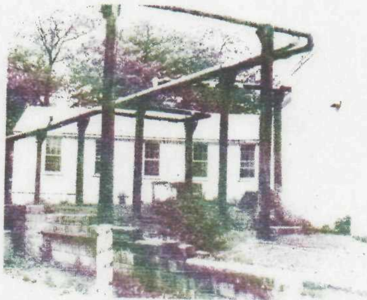
Steam heating piping located in back of Building # P-6 (Library).
