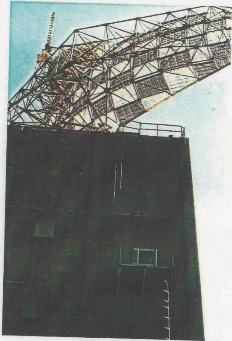
Radar tower, #P-201
