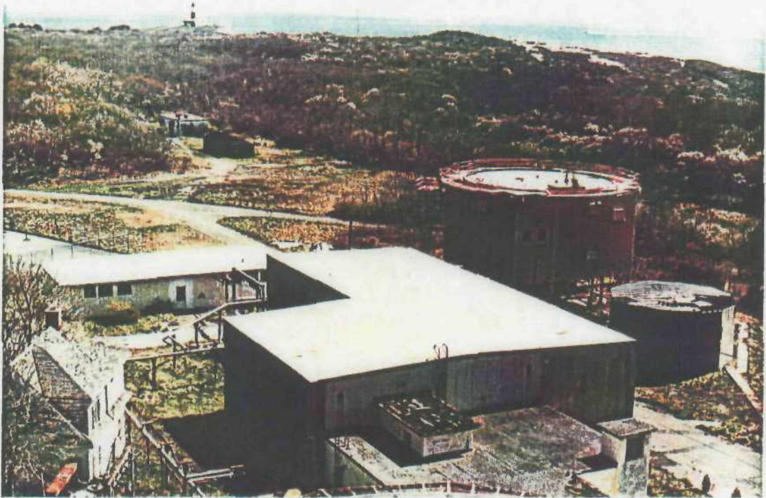
View of site from top of radar tower #P-201. From left to right: bldg. #P-107, #P-111, #P-101, #P-205-T.
