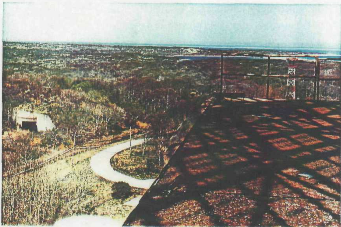
View of large bunker and dilapidated fence from roof of radar tower #P-201.
