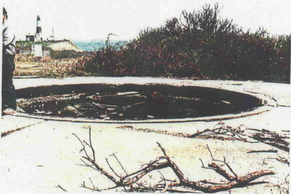
Sixteen-inch gun emplacement outside of large bunker #P-100.
