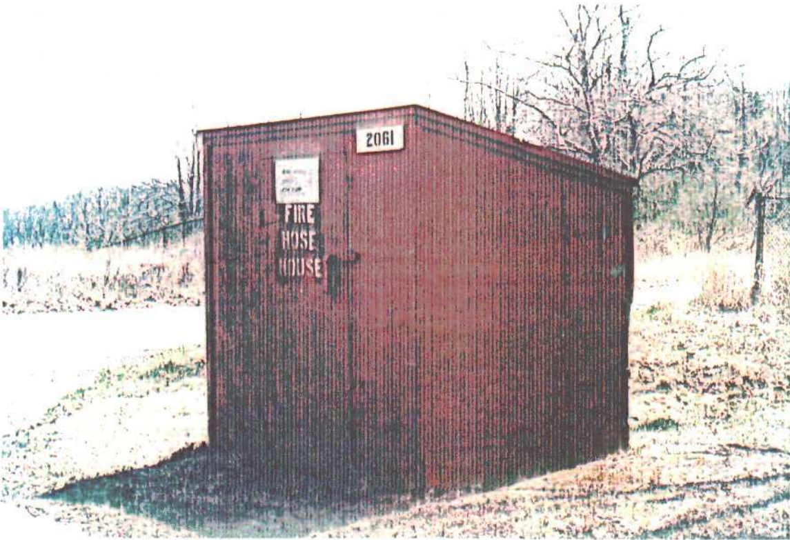
View of hose house (Bldg. #2061) located in eastern portion of site.
