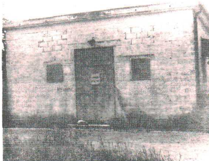
Building #P-99 (Warehouse).
