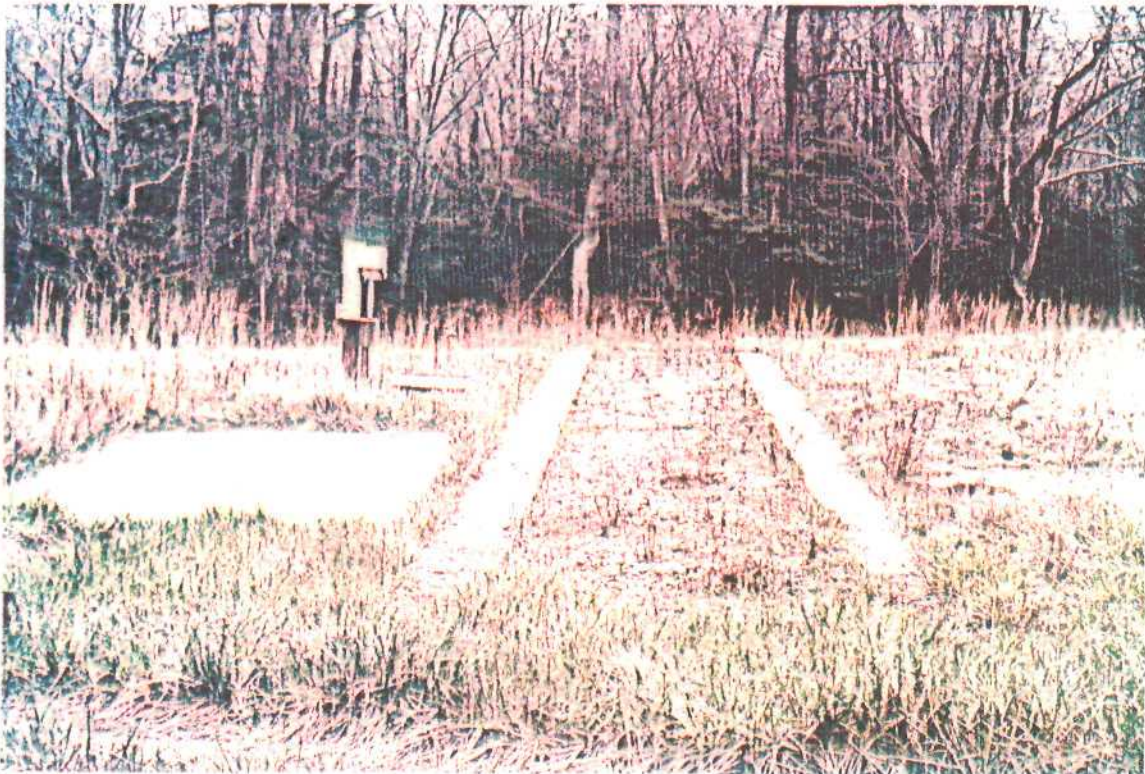
Concrete trailer pads with utility facilities.
