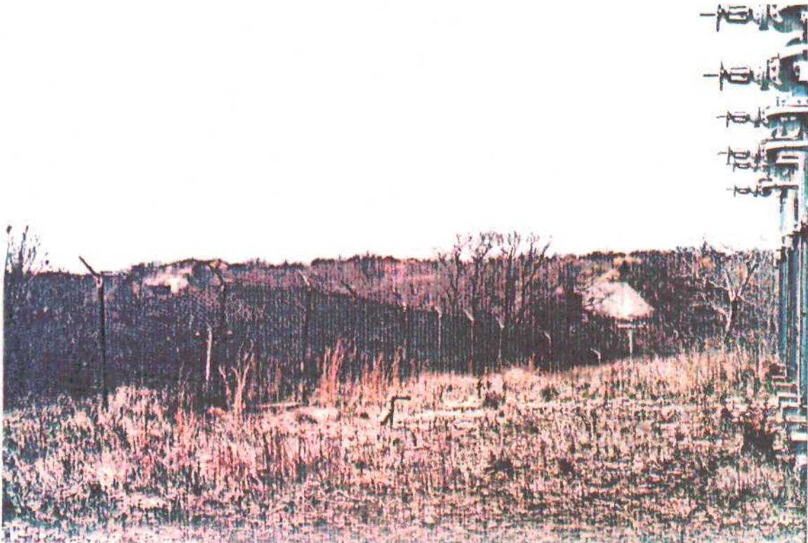
Underground fuel tank, field located adjacent to power plant (Bldg. #P-203), and one of two large bunkers in background.
