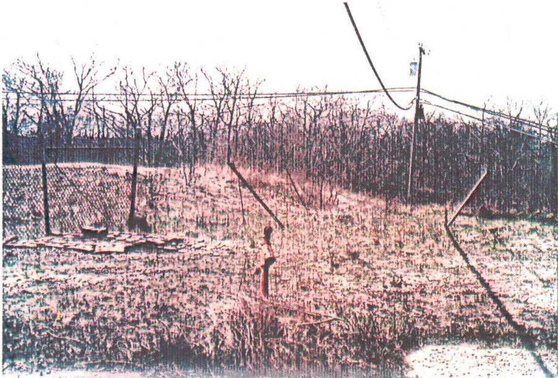
Underground fuel tank, field located adjacent to power plant (Bldg. #P-203).
