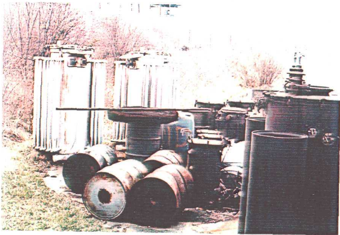
Transformers and switches removed.
