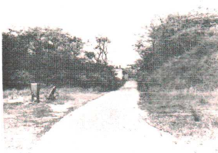
Gas Pump and Gas Tank in foreground, and Buildings #P-99 (Warehouse) and #P-98 respectively in background.
