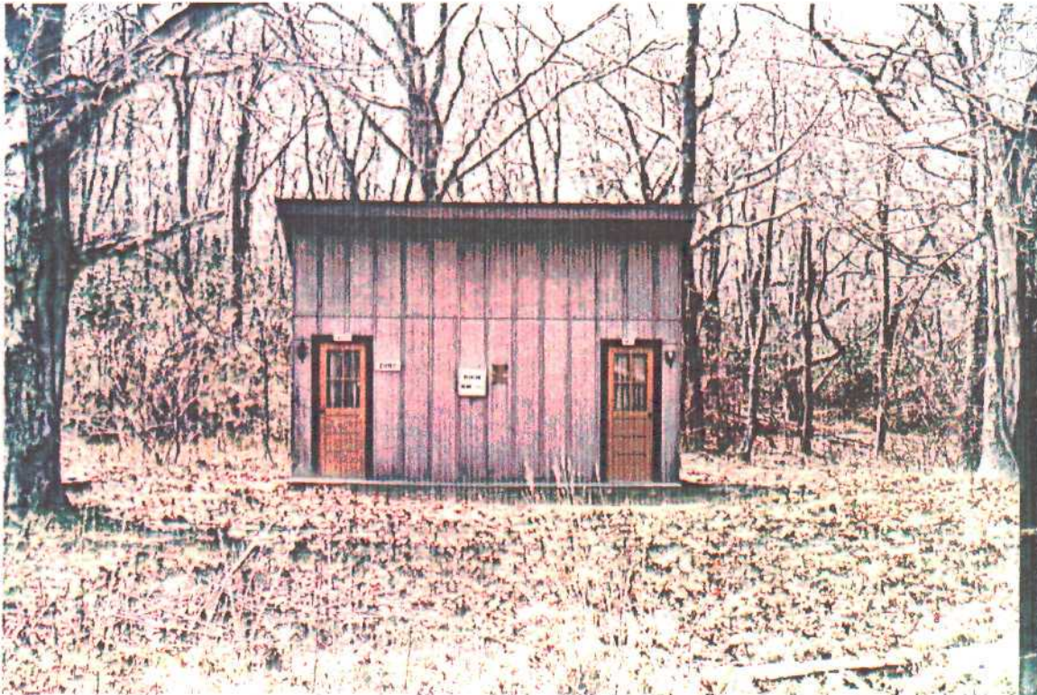
View of restroom facilities (Bldg. #P-116) located in eastern portion of site.
