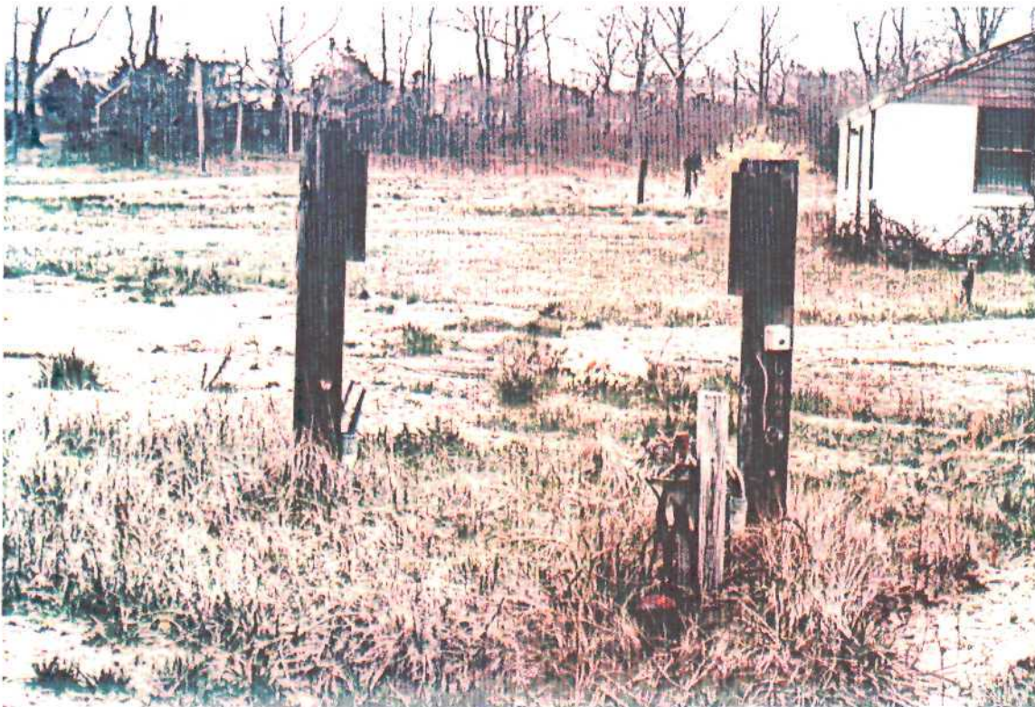
Utility facilities used for each trailer.
