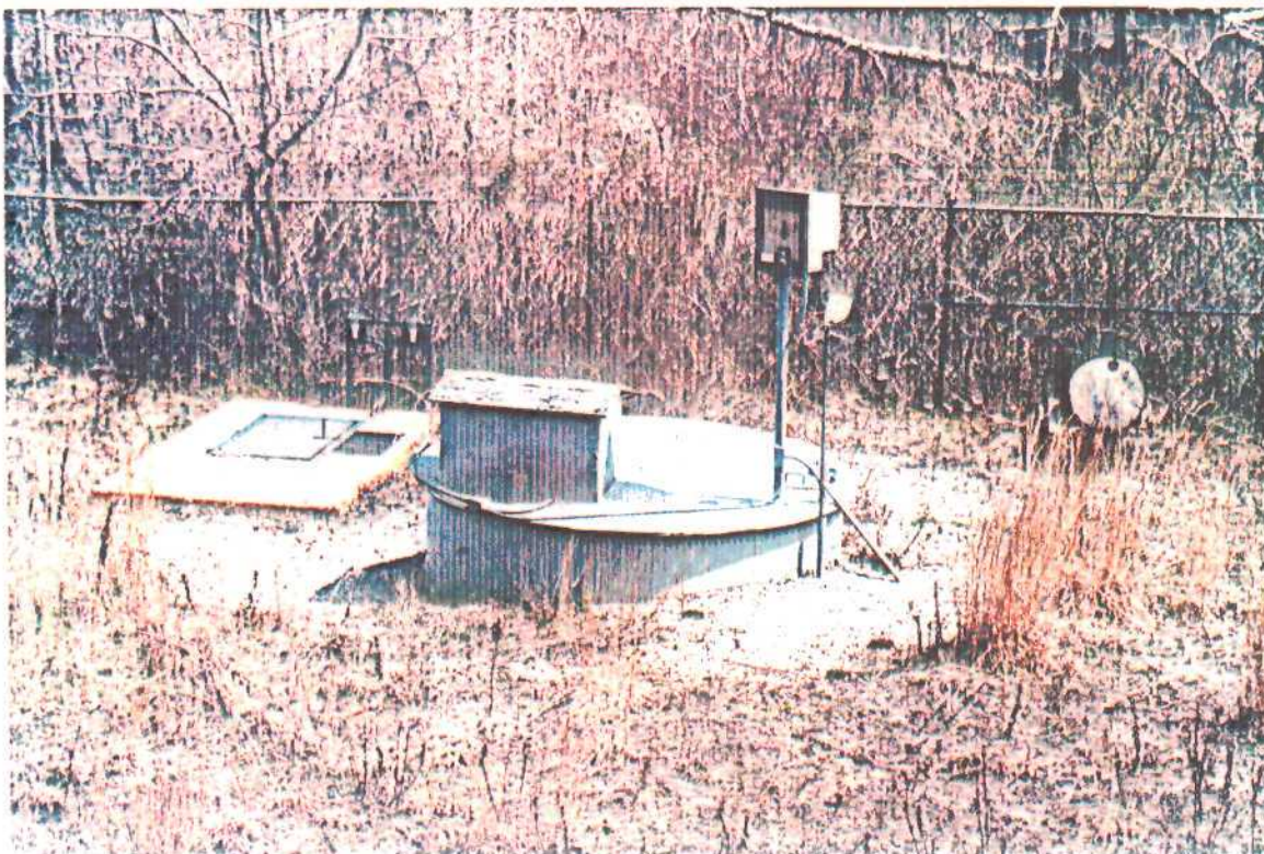
Portion of sewage treatment facilities.
