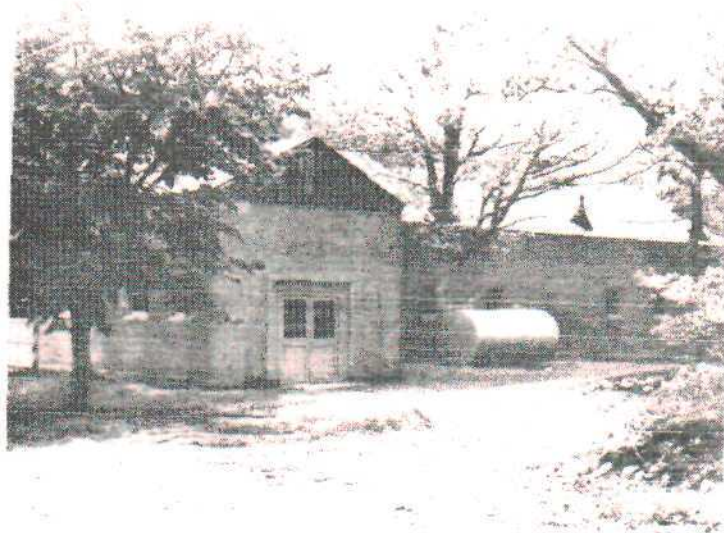
Building#P-31(Garage) - to be retained.
