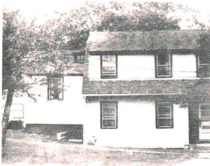
Front view of Building #T-1 (Dormitory).
