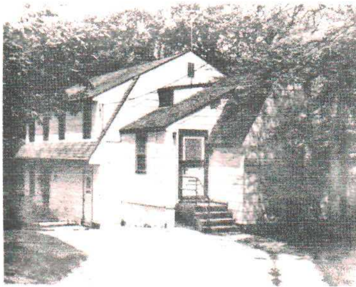
Front and side view of Building #P-17 (Dispensary).
