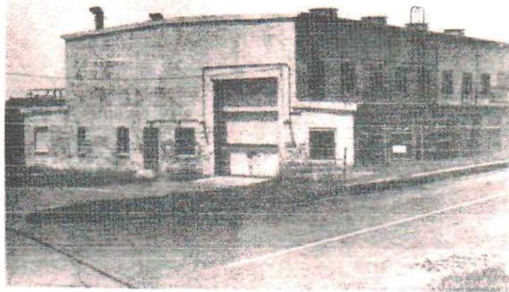
Building #P-203 (Power Plant).
