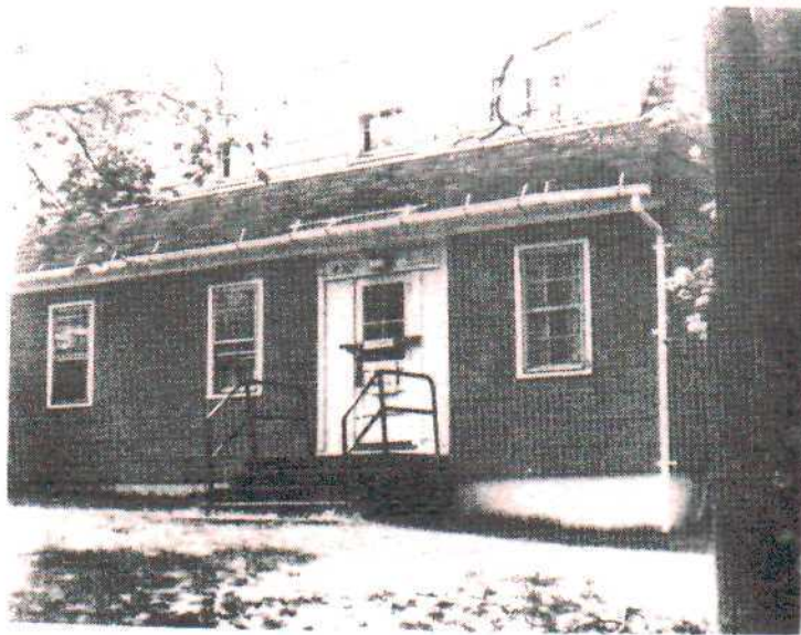
Front view of Building #P-14 (Dormitory).
