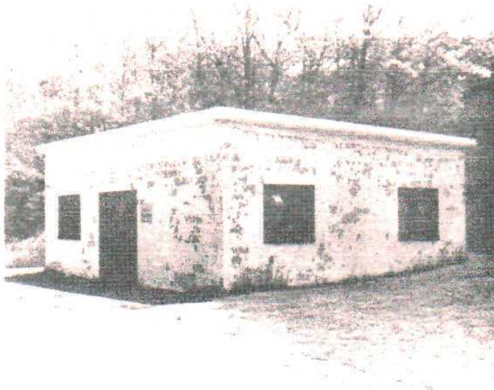
Building #P-21 (Water Treatment Plant)-to be retained.
