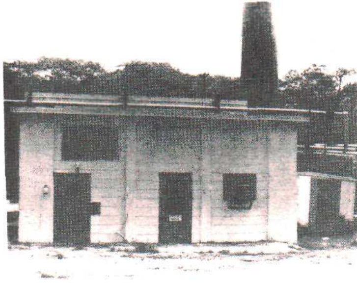
Building # P-105 (Heating Plant).
