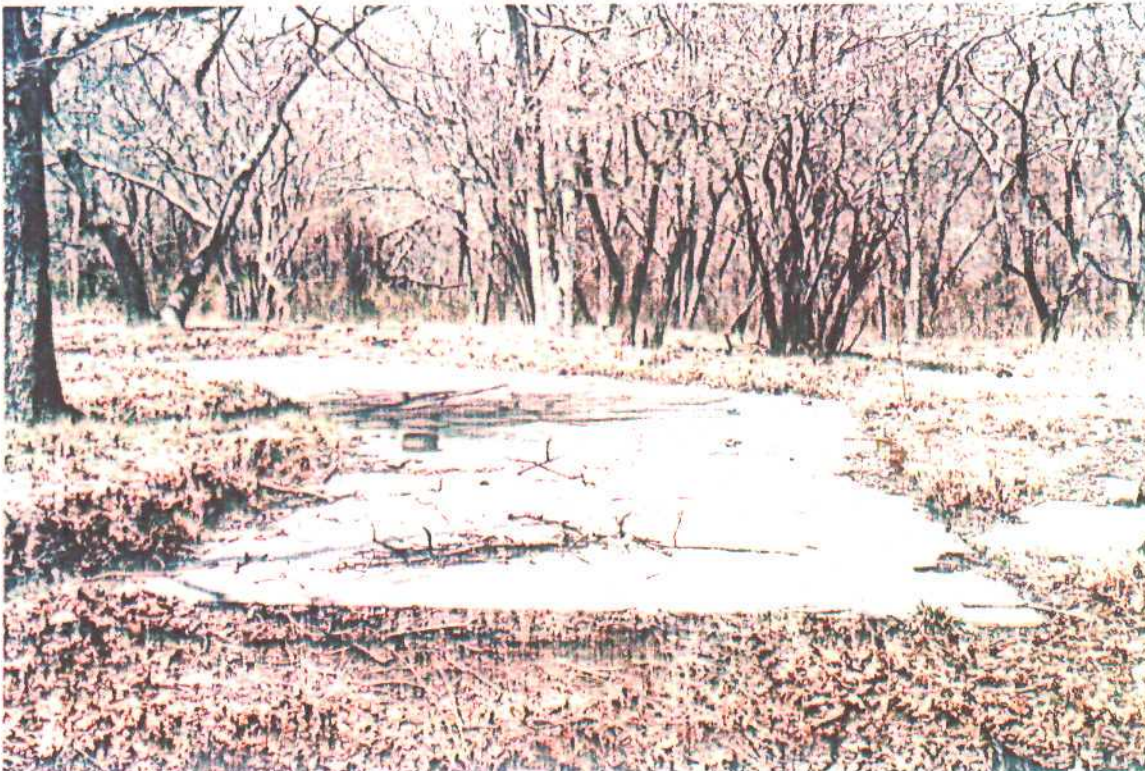
View of concrete slabs and utility post located in eastern portion of site.
