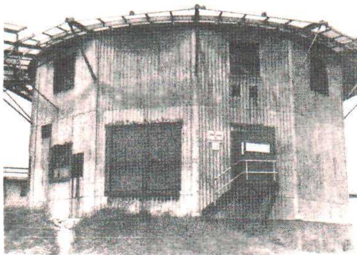
Building #P-208 (BCE Maintenance Shop).
