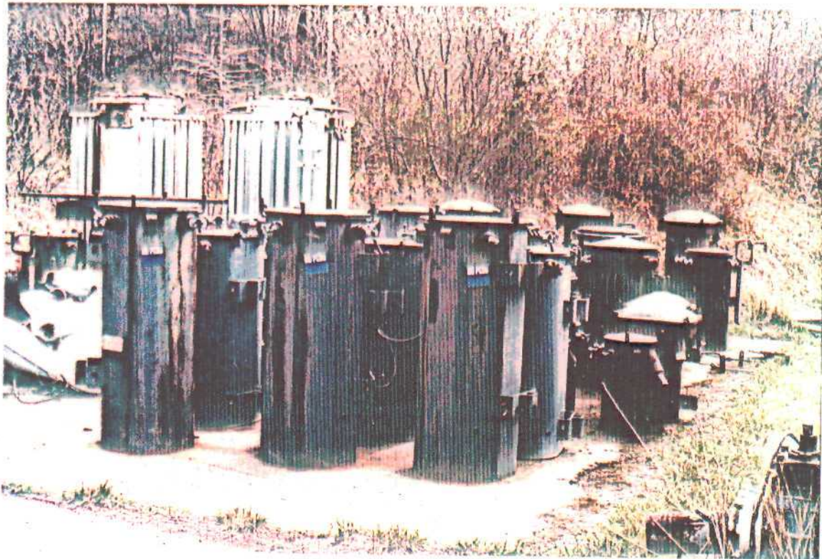
Transformers and switches removed.
