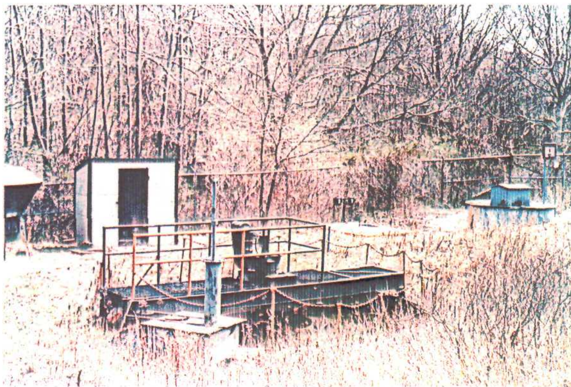
Portion of sewage treatment facilities.
