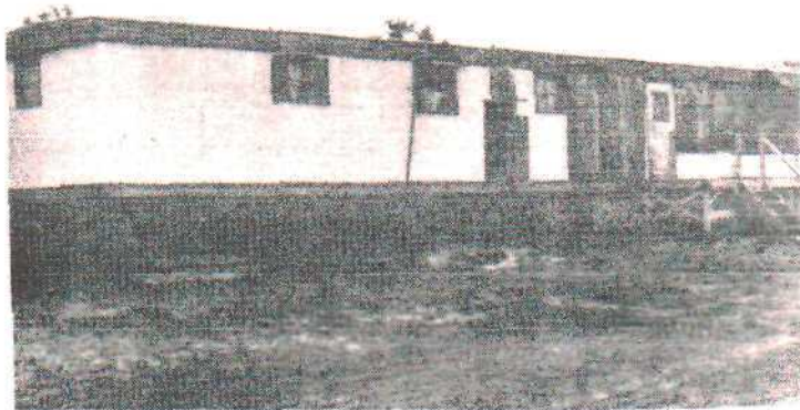
Trailer behind Building #P-104-R.
