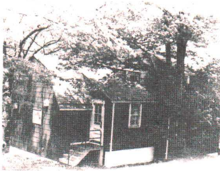
Back view of Building #P-11 (Dormitory).
