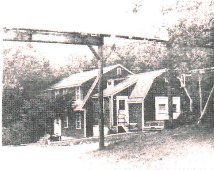
Building #P-4 (Dormitory)-to be retained.
