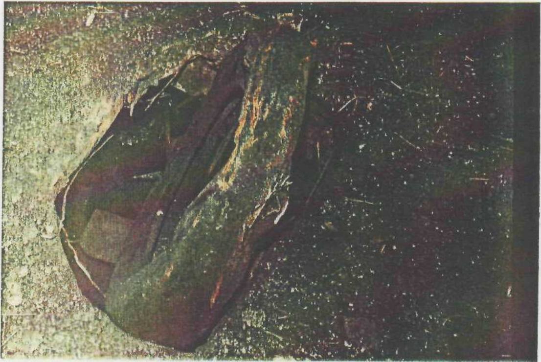
Open hole in floor of large bunker #P-100.
