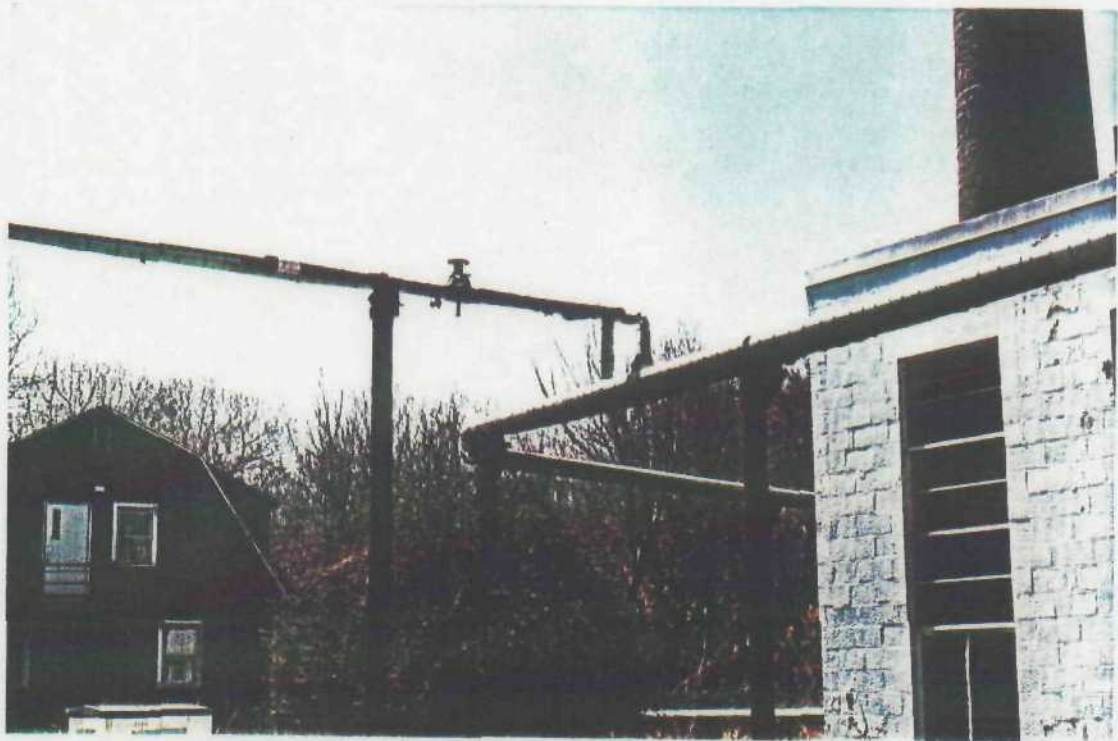
Central boiler room #P-105(on right) with exterior, asbestos-insulated pipes used for heating system. Bldg. #P-11 on left.
