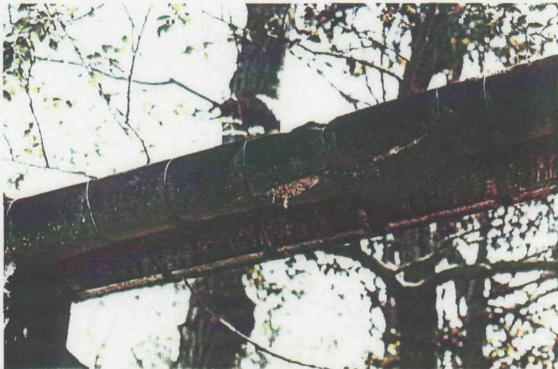
Asbestos-insulated pipes used for heating system with exposed asbestos leaking directly to the ground.
