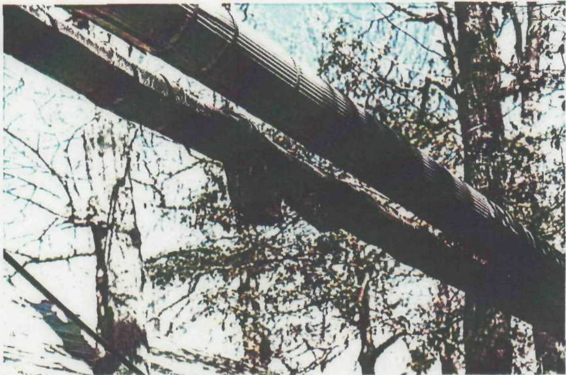
Asbestos-insulated pipes used for heating system with exposed asbestos is leaking directly to the ground.
