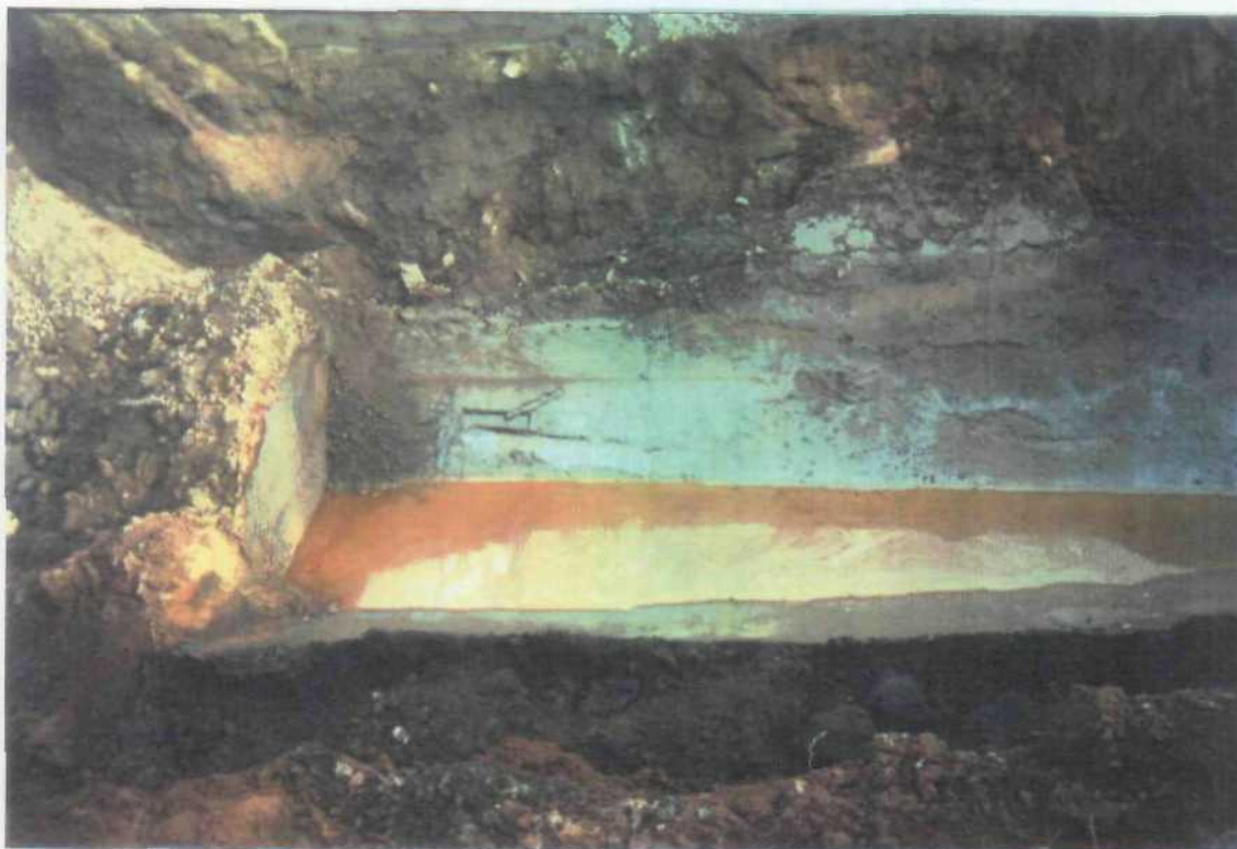
BOTTOM OF EXCAVATION, NOTE FREE PRODUCT ON SOIL AND WATER
