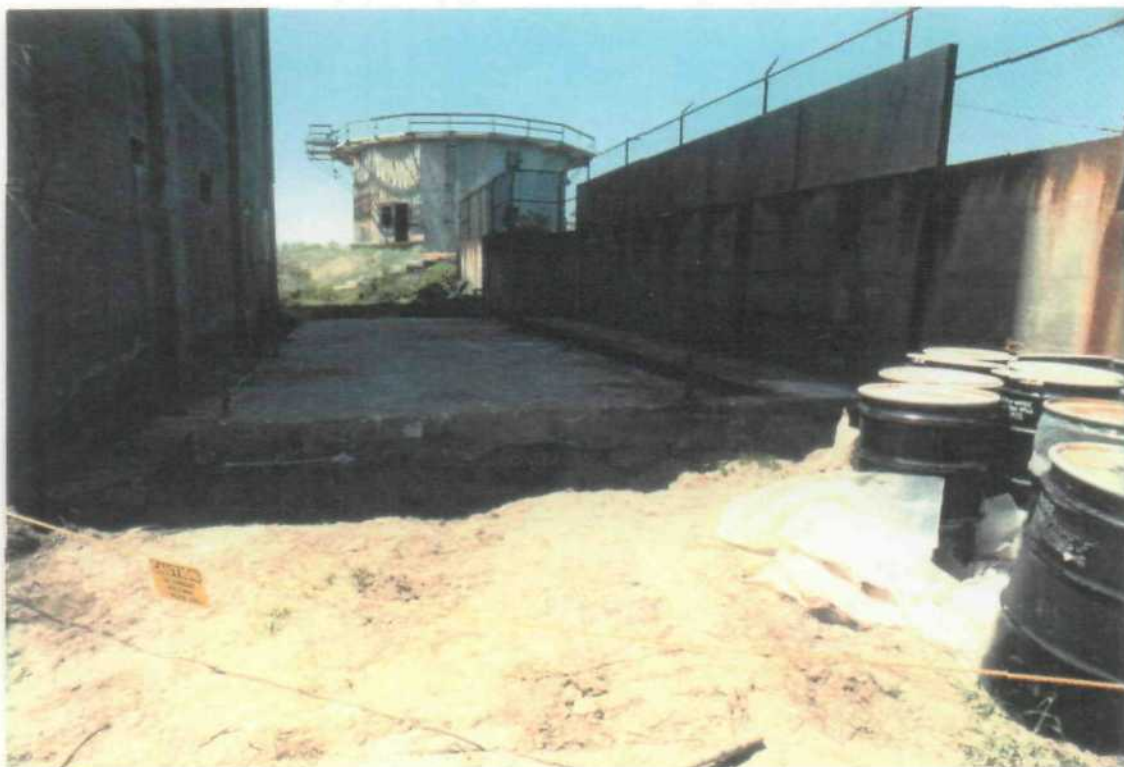
PCB TRANSFORMER SITE #3 POST EXCAVATION AND REMOVAL OF CONTAMINATED SOIL
