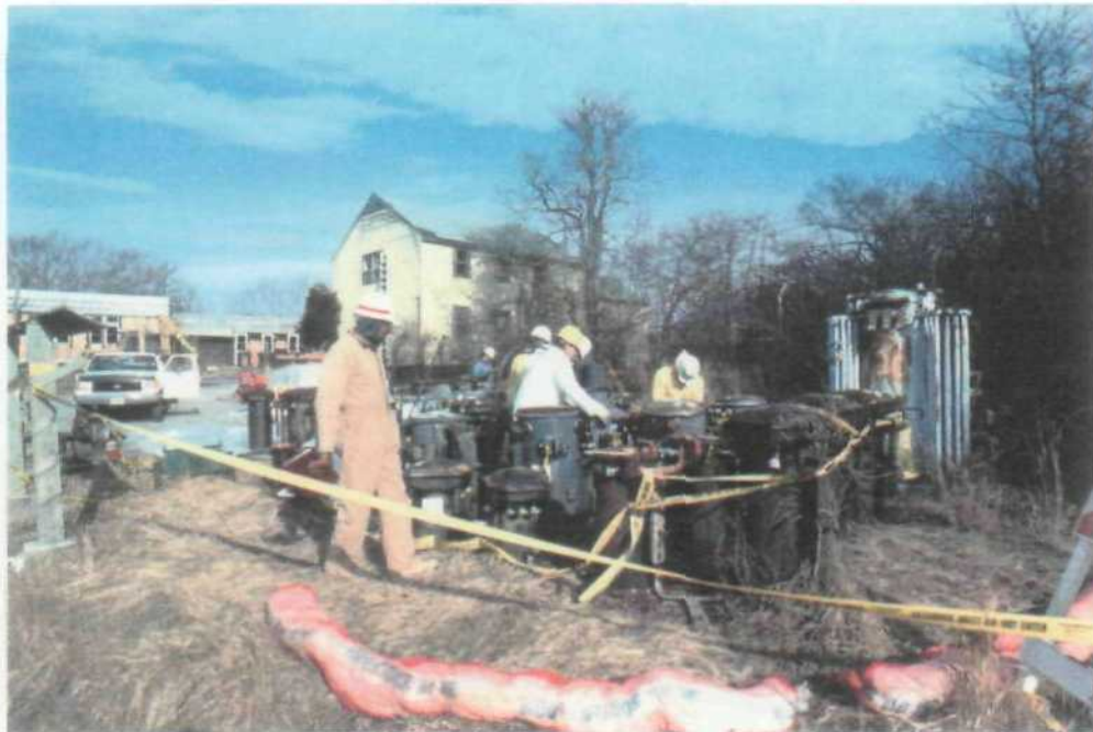
REMOVAL OF OIL FROM TRANSFORMERS FOR DISPOSAL
