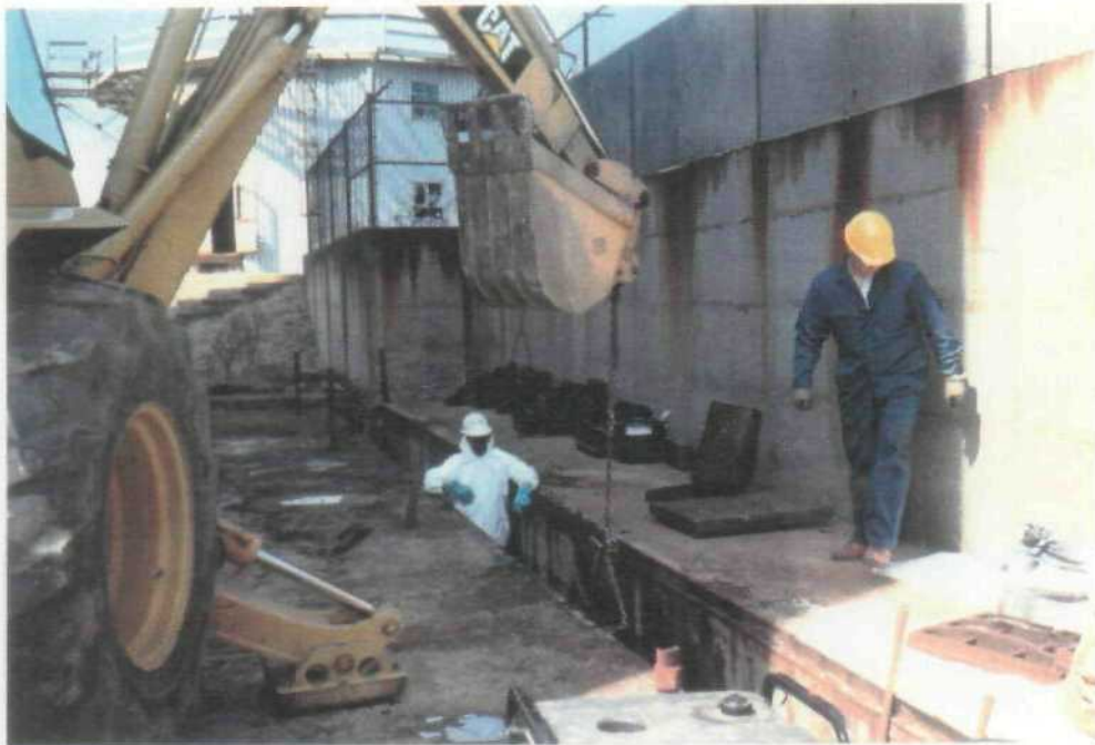
TRANSFORMER SITE #3 CLEANOUT OF CONDUIT TRENCH REMOVAL OF PCB OIL CONTAMINATED WATER, SLUDGE & DEBRIS
