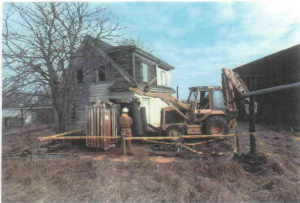
TRANSFORMER SITE #6 REMOVAL OF TRANSFORMER CARCASSES
