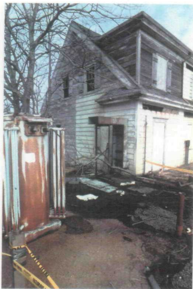
TRANSFORMER SITE #6 CONCRETE STAINED WITH PCB OIL
