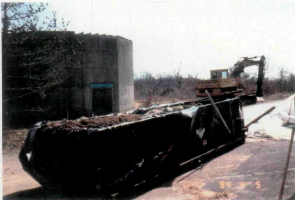
DOT CERTIFIED DISPOSAL CONTAINER FOR DIRT AND DEBRIS CONTAMINATED WITH PCBs; LINED WITH POLY "BACCIE"
