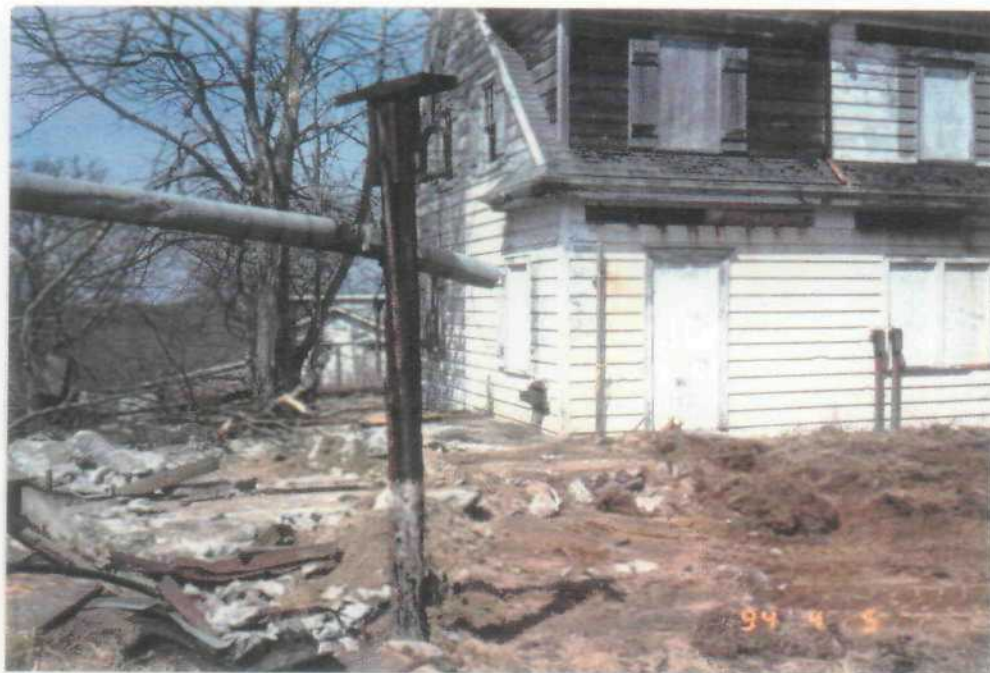
TRANSFORMER SITE #6 DEMOLITION OF CONCRETE STAINED WITH PCB OIL
