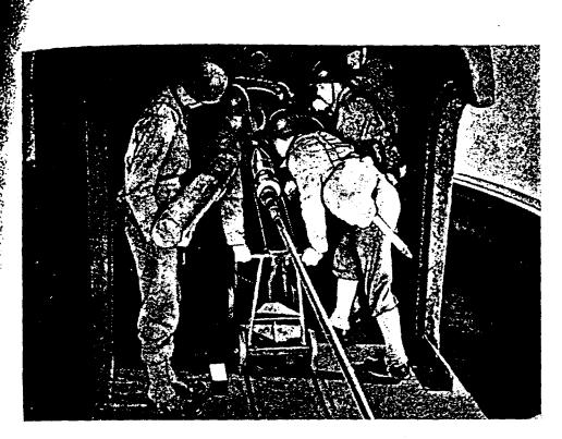
Figure 112. Loading carriage, 6-inch gun barbette carriage M1.
