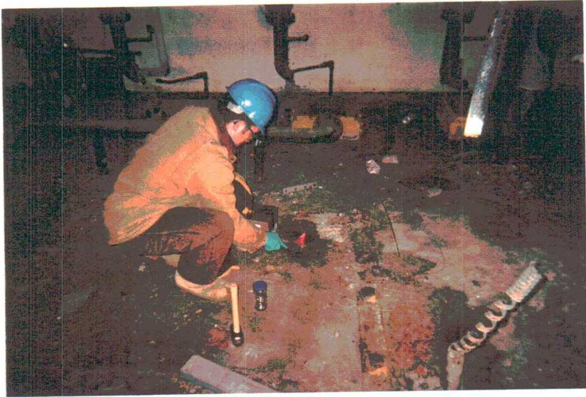
Photograph 1 - Chip sampling (C-1) in Building 10.
