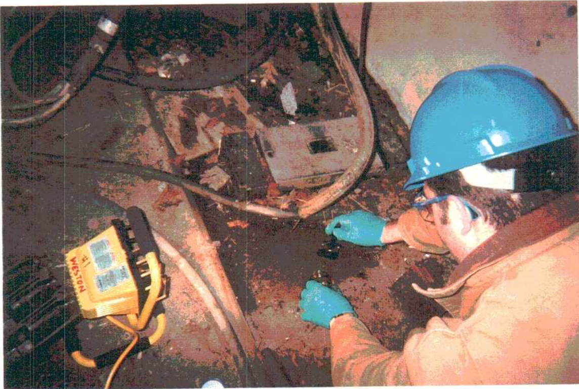
Photograph 2 - Chip sampling (C-2) in Radar Tower.
