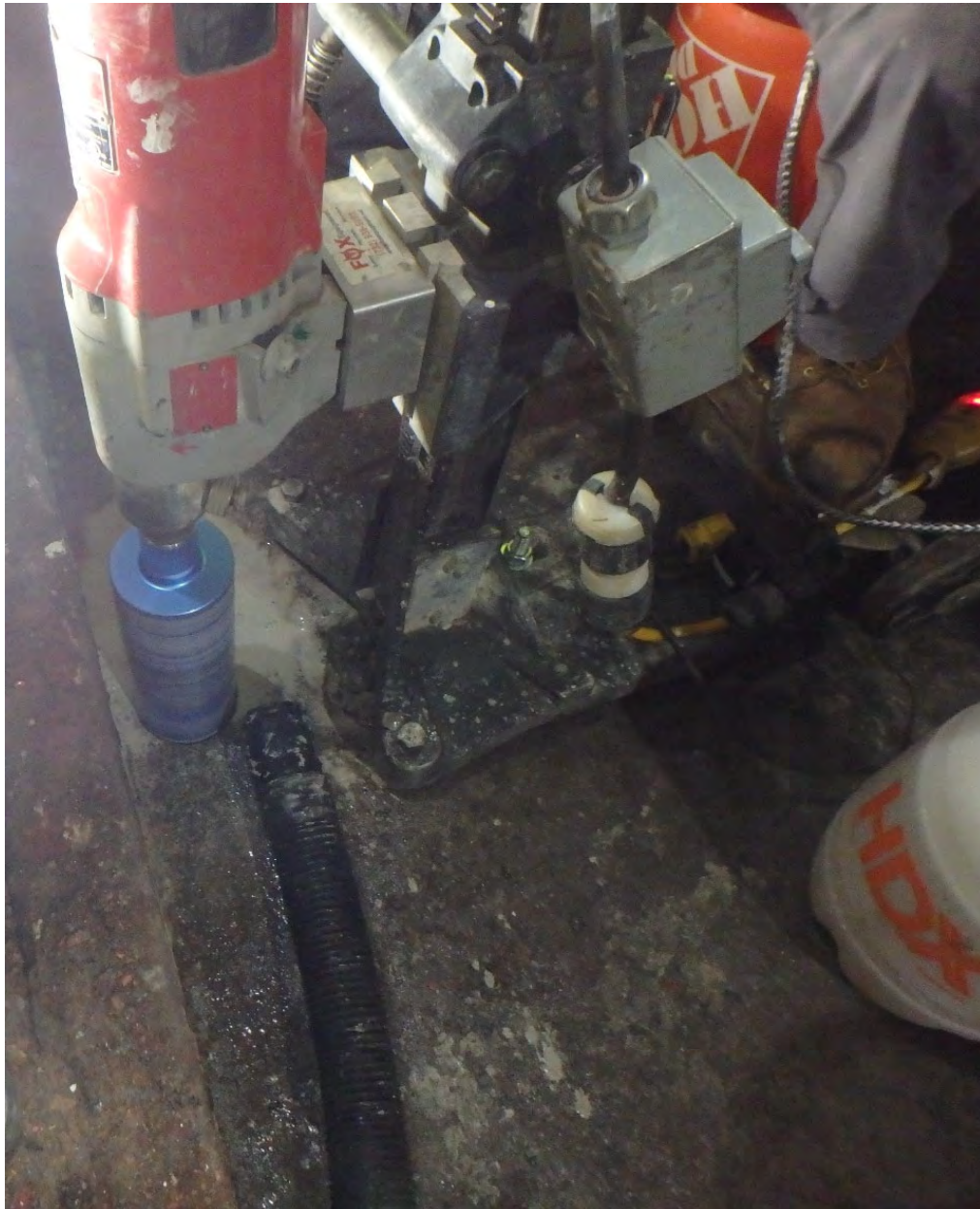
Concrete Sampling via Core Drill with Continuous Mist and HEPA Vacuum
