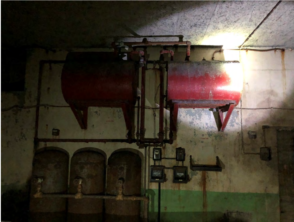
Wall-Mounted Above-Ground Storage Tanks (ASTs) Located within Battery #113
