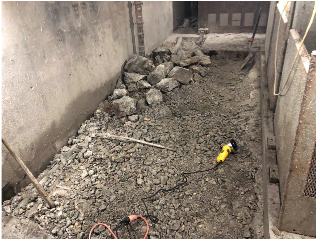
Full-Scale PCB-Impacted Concrete Removal via Jackhammers
