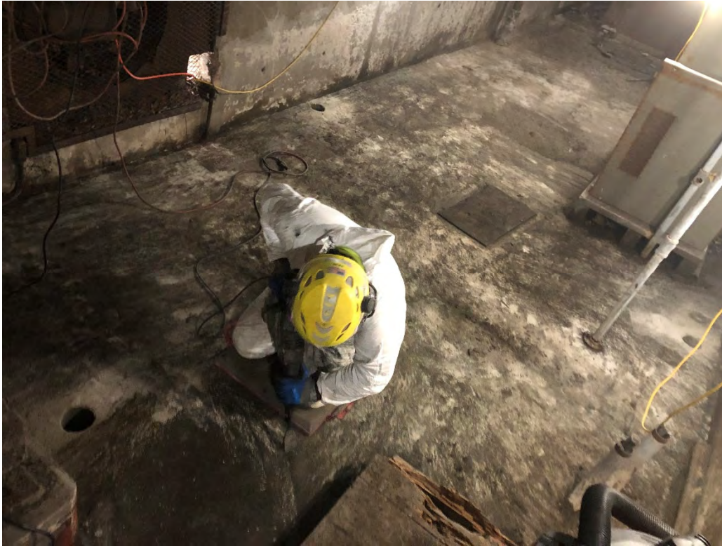
Limited PCB-Impacted Concrete Removal via Chipping Gun
