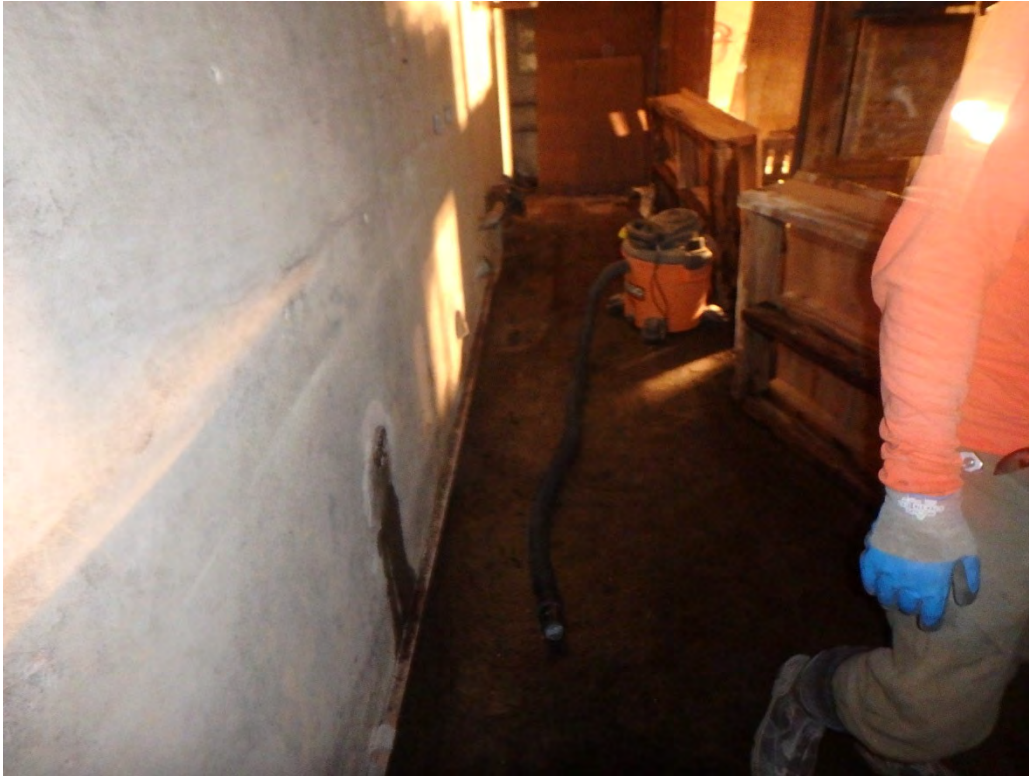
Cleaning and Pressure Washing Transformer Removal Area
