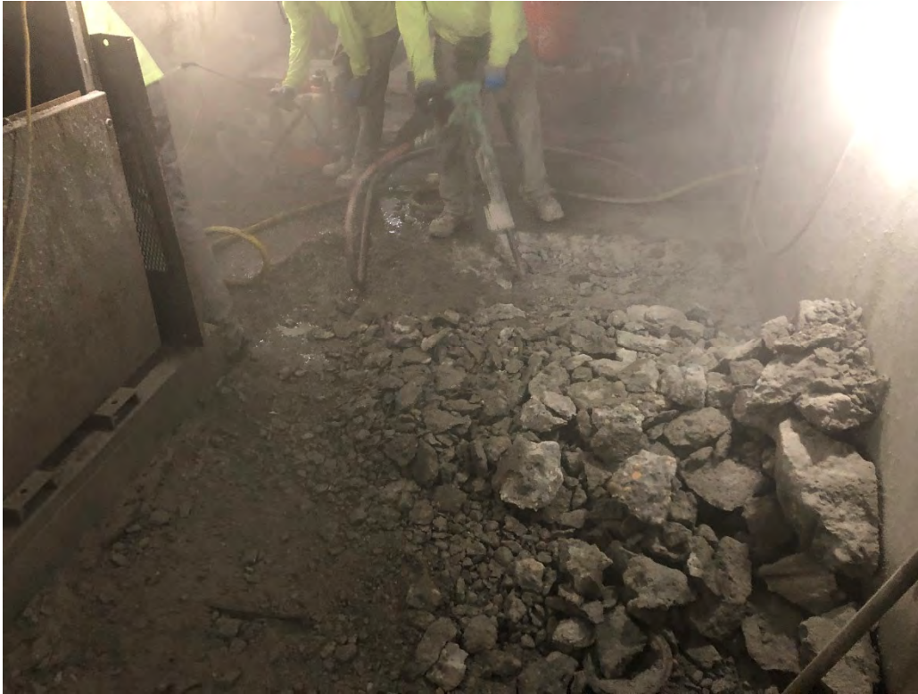
Full-Scale PCB-Impacted Concrete Removal via Jackhammers
