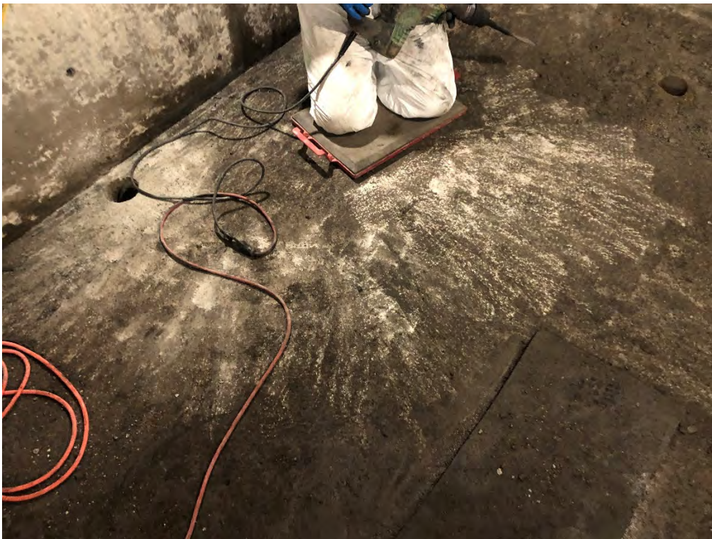
Limited PCB-Impacted Concrete Removal via Chipping Gun
