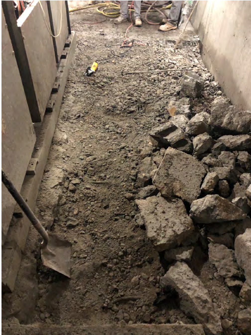
Full-Scale PCB-Impacted Concrete Removal via Jackhammers
