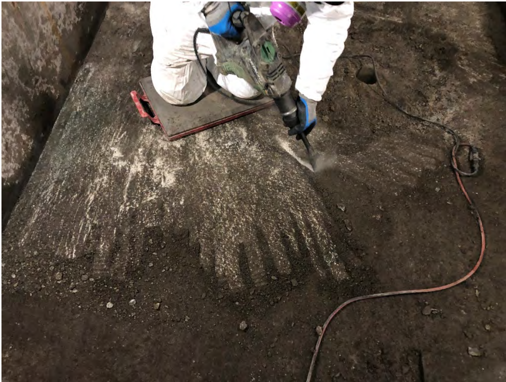
Limited PCB-Impacted Concrete Removal via Chipping Gun
