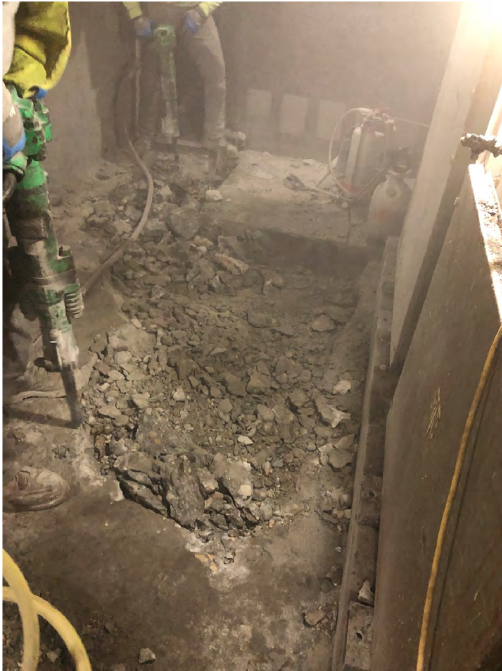
Full-Scale PCB-Impacted Concrete Removal via Jackhammers
