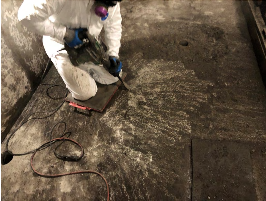
Limited PCB-Impacted Concrete Removal via Chipping Gun
