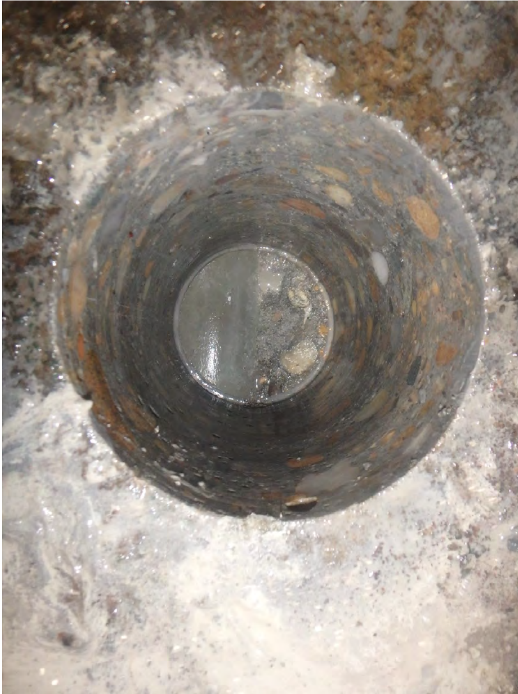
Aggregate Reinforcement Observed in Battery #113 Concrete
