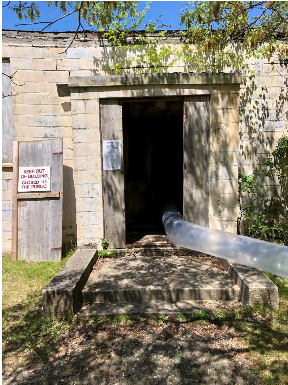
Negative Air Containment Asbestos Abatement
