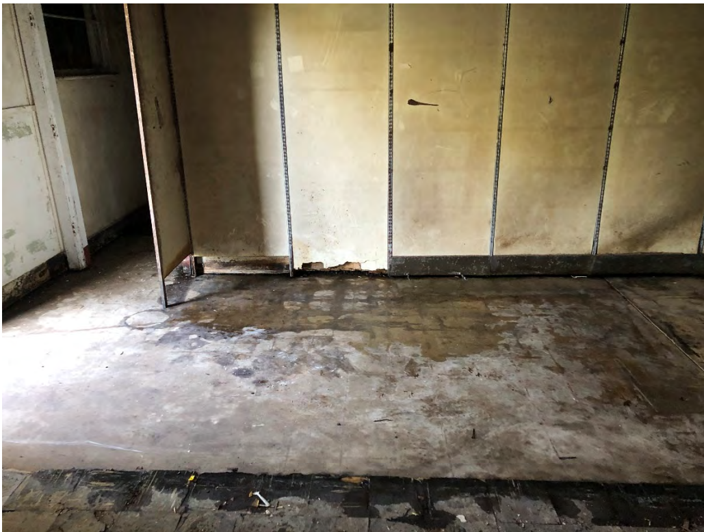
Stained Floor Abated of Asbestos-Containing-Material (ACM) Tiles
