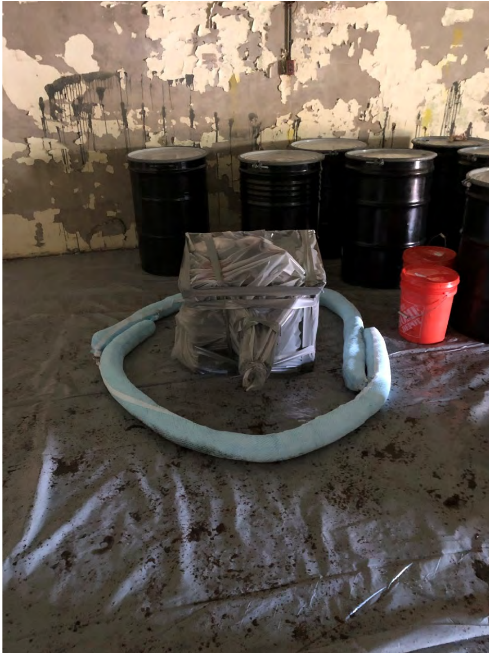
Transformer T2313 Removed from Battery #113 and Prepared for Proper Disposal
