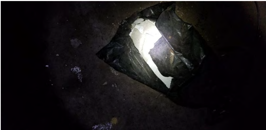
Bag Containing ACM Removed from Battery #113 and Properly Disposed of
