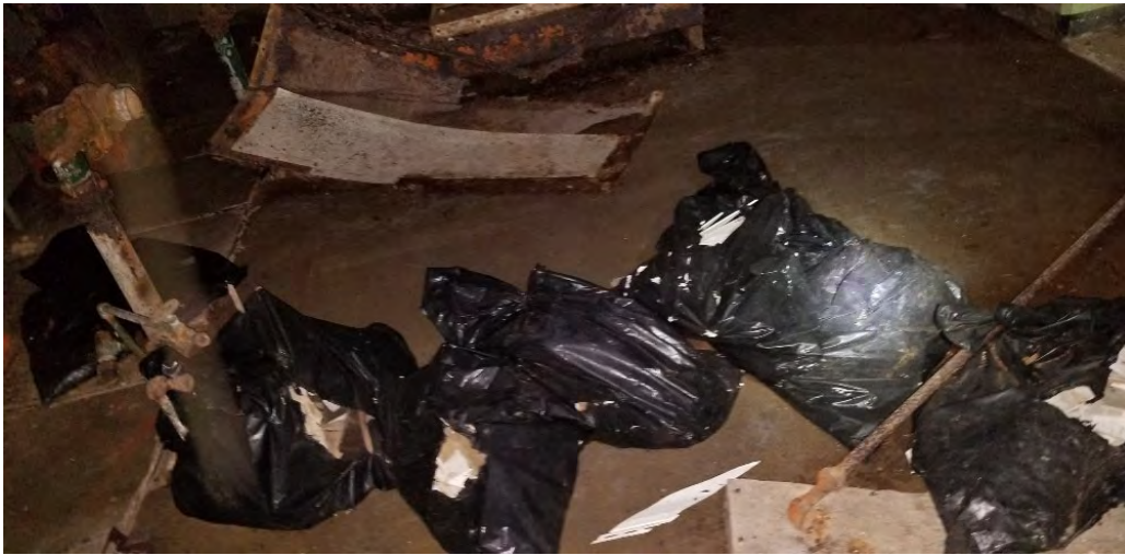
Bags Containing ACM Removed from Battery #113 and Properly Disposed of
