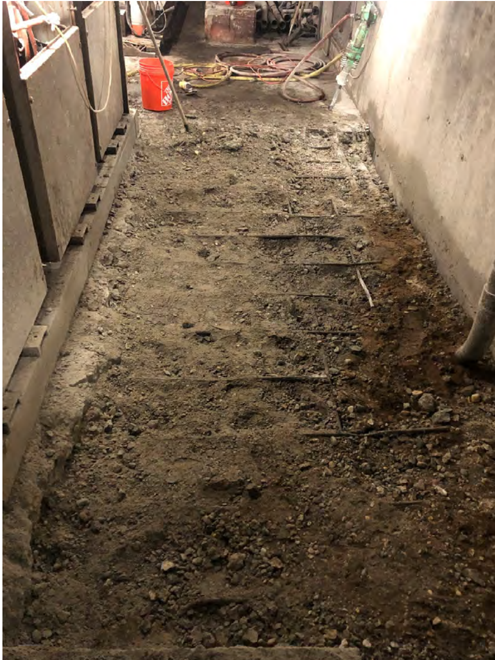
Full-Scale PCB-Impacted Concrete Removal via Jackhammers
