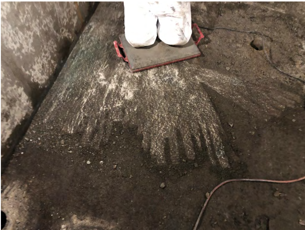
Limited PCB-Impacted Concrete Removal via Chipping Gun
