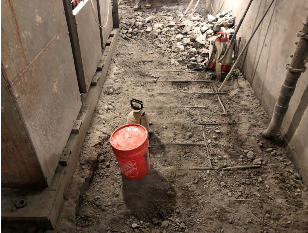
Full-Scale PCB-Impacted Concrete Removal via Jackhammers
