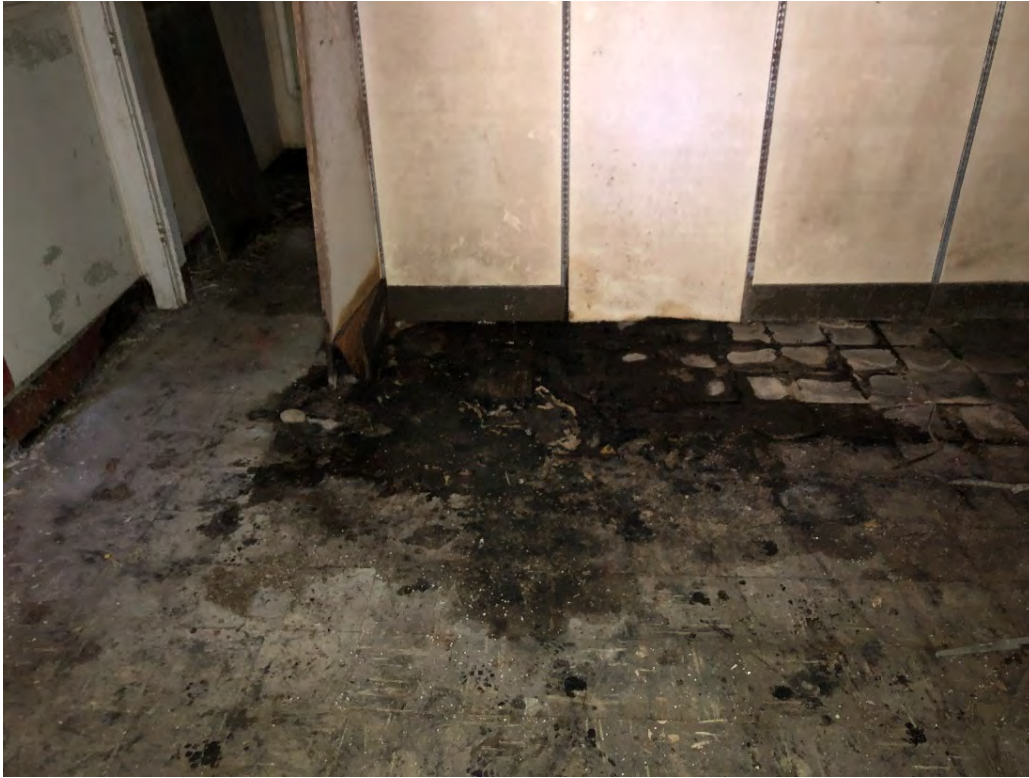
Tile Staining below HAZMAT Stockpile
