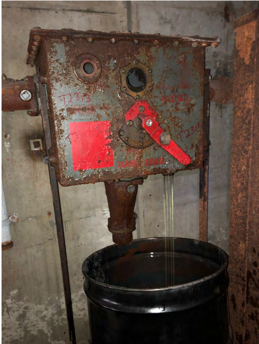
Removal of PCB-Fluids from Transformer T2313
