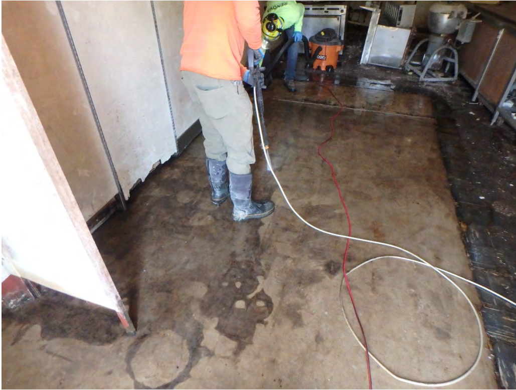
Pressure Washing Stained Concrete Floors
