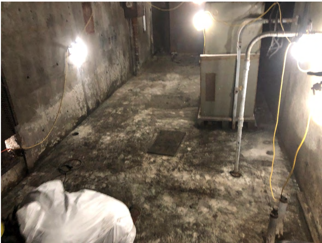
Limited PCB-Impacted Concrete Removal via Chipping Gun
