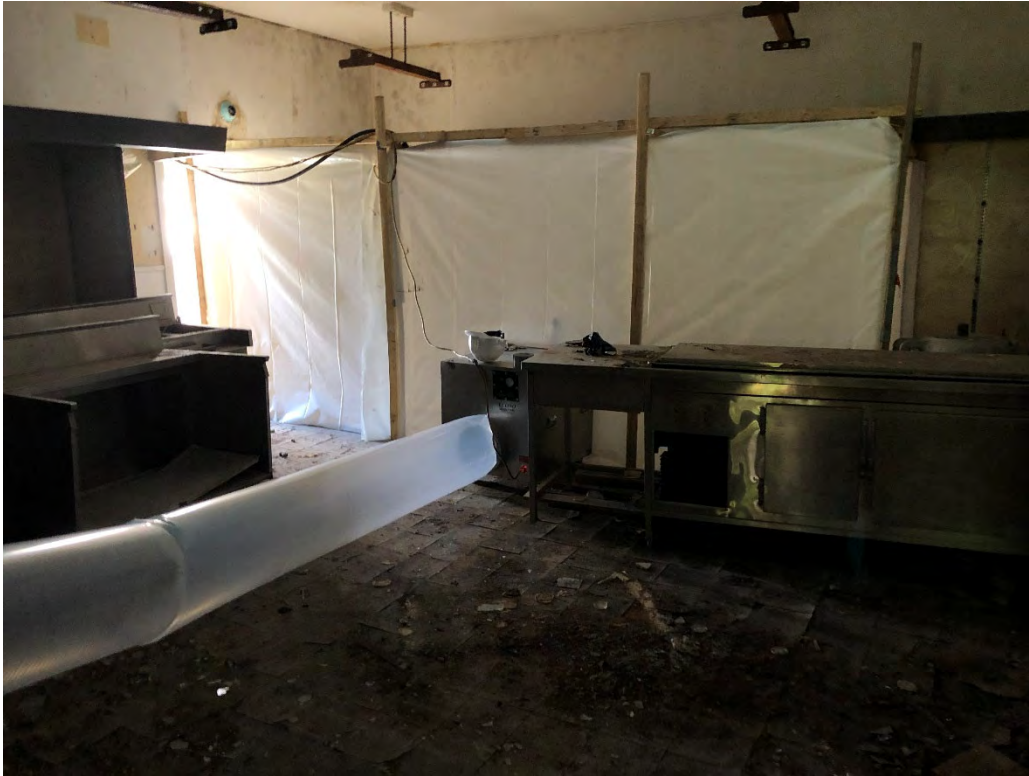
Negative Air Containment Asbestos Abatement
