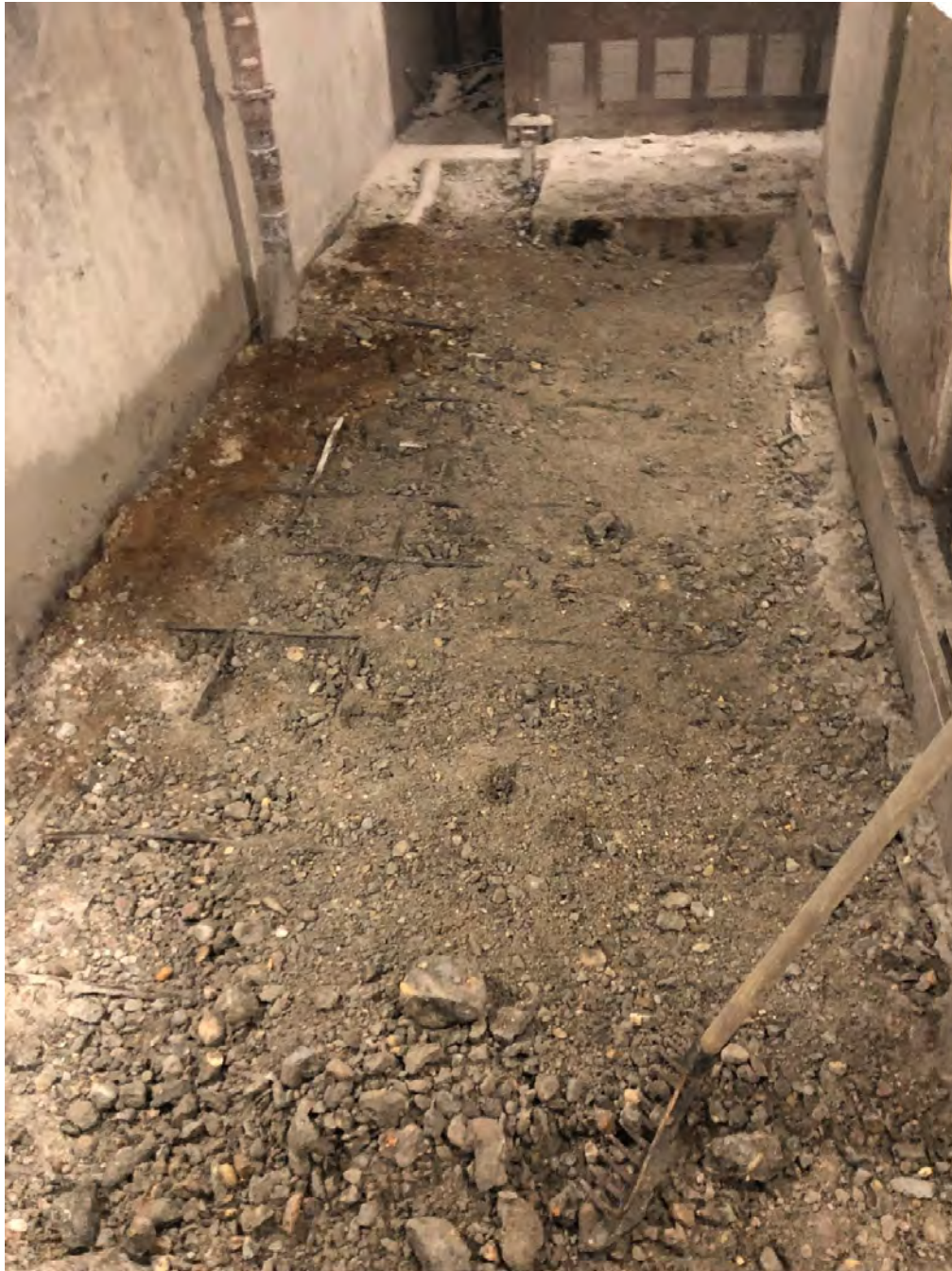
Full-Scale PCB-Impacted Concrete Removal via Jackhammers
