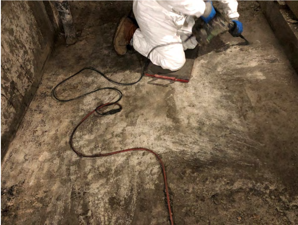
Limited PCB-Impacted Concrete Removal via Chipping Gun
