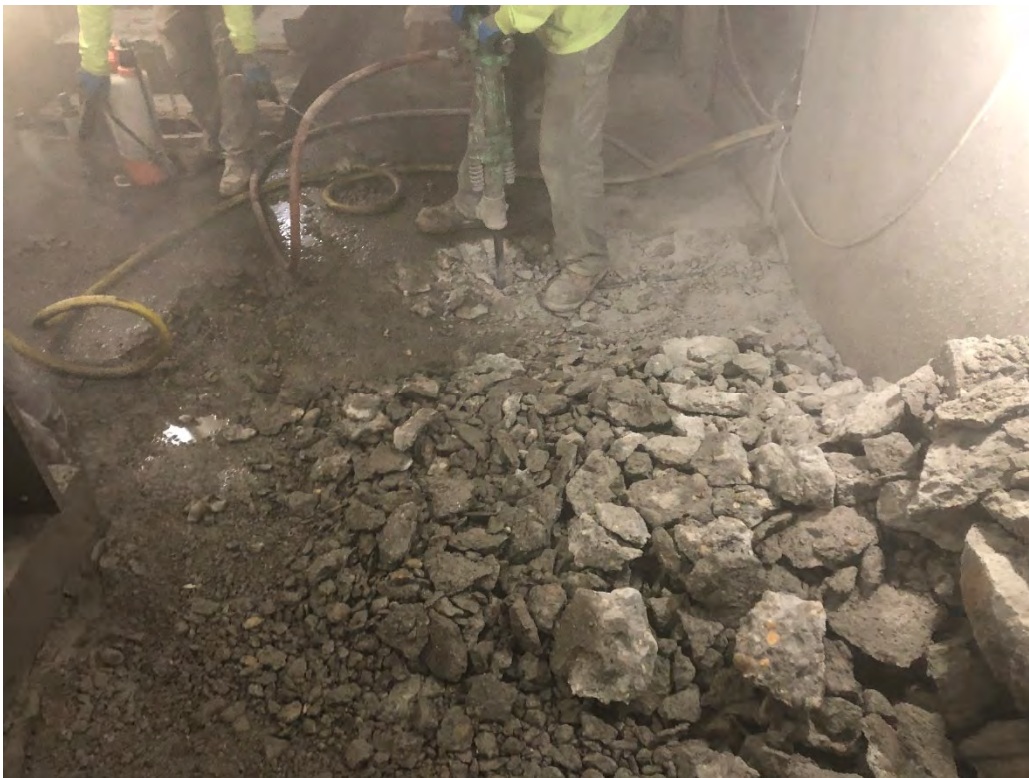
Full-Scale PCB-Impacted Concrete Removal via Jackhammers
