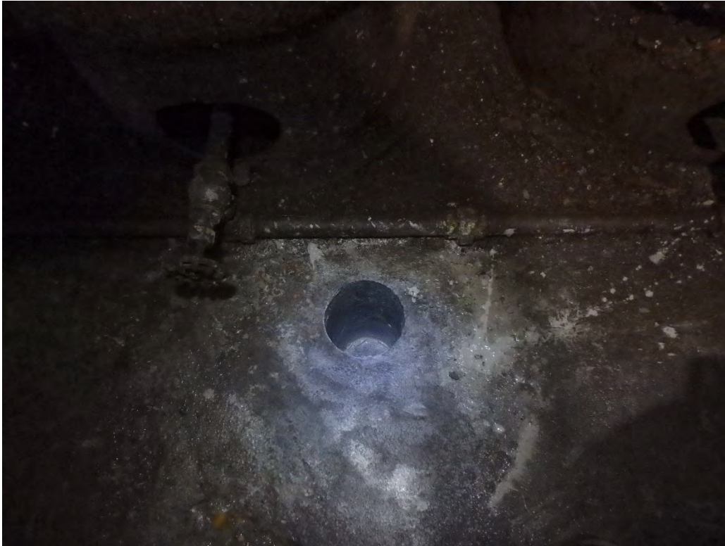
Concrete Core Sample Location
