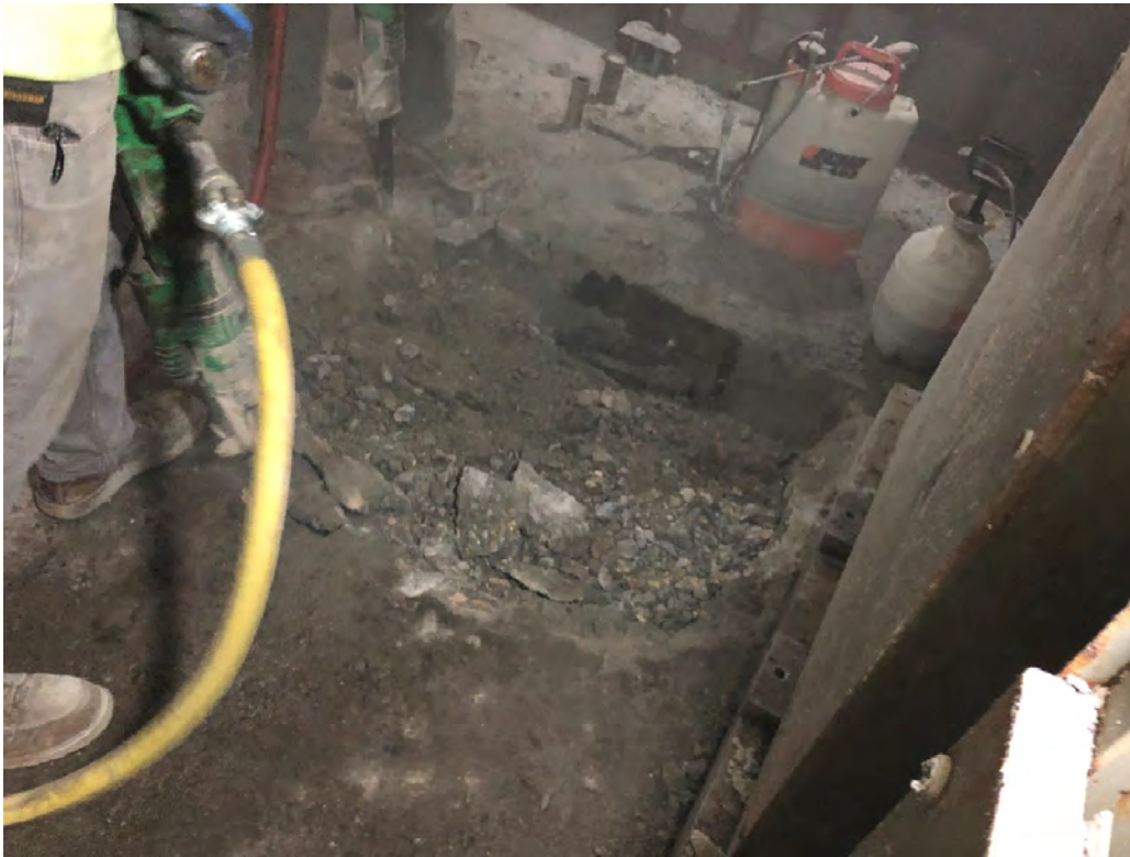
Full-Scale PCB-Impacted Concrete Removal via Jackhammers
