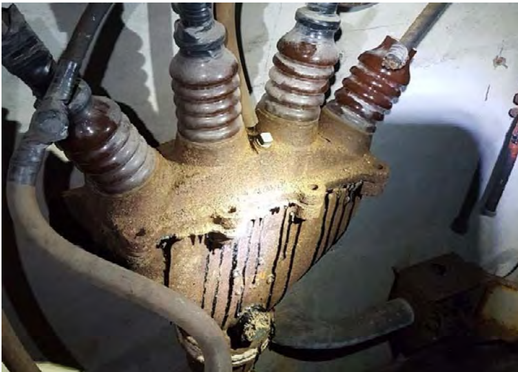
Polychlorinated Biphenyl (PCB) Fluid Dried on Exterior of Transformer
