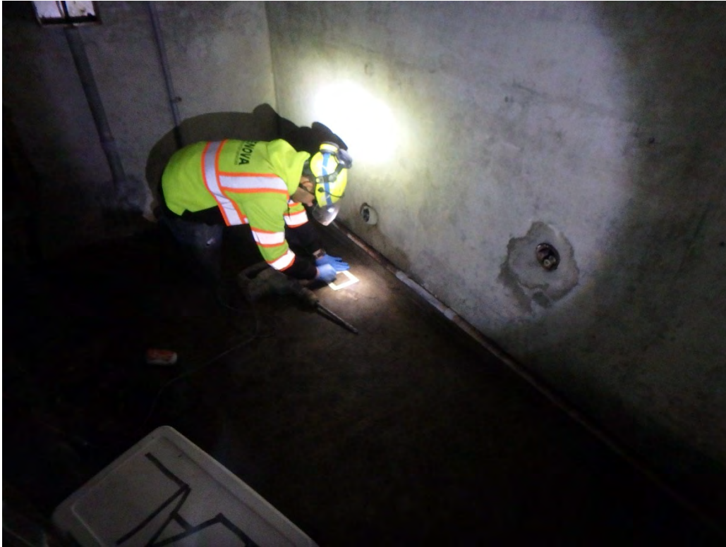
Concrete Chip and Wipe Sampling Transformer Removal Area
