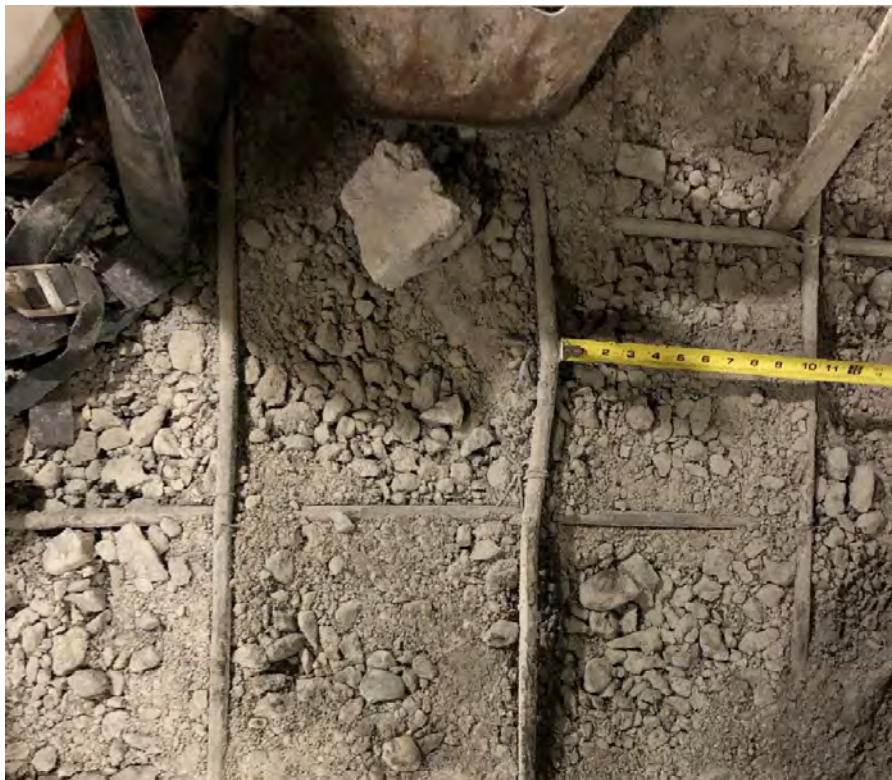
10" x 10" Rebar Observed in Battery #113 Concrete
