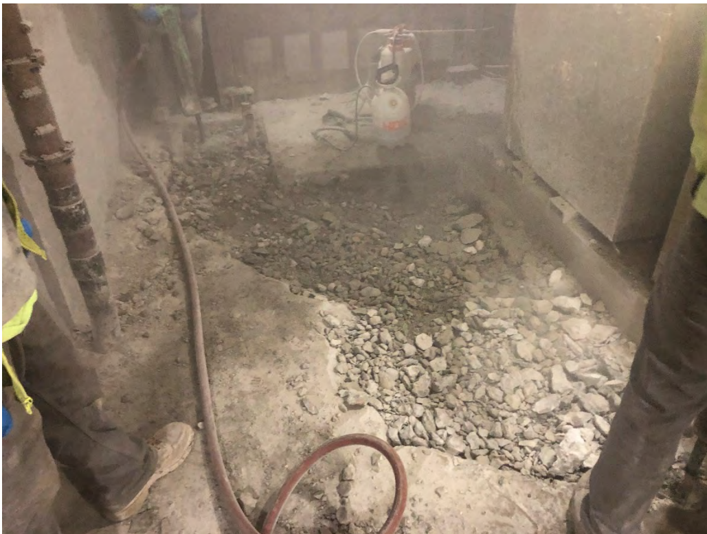
Full-Scale PCB-Impacted Concrete Removal via Jackhammers
