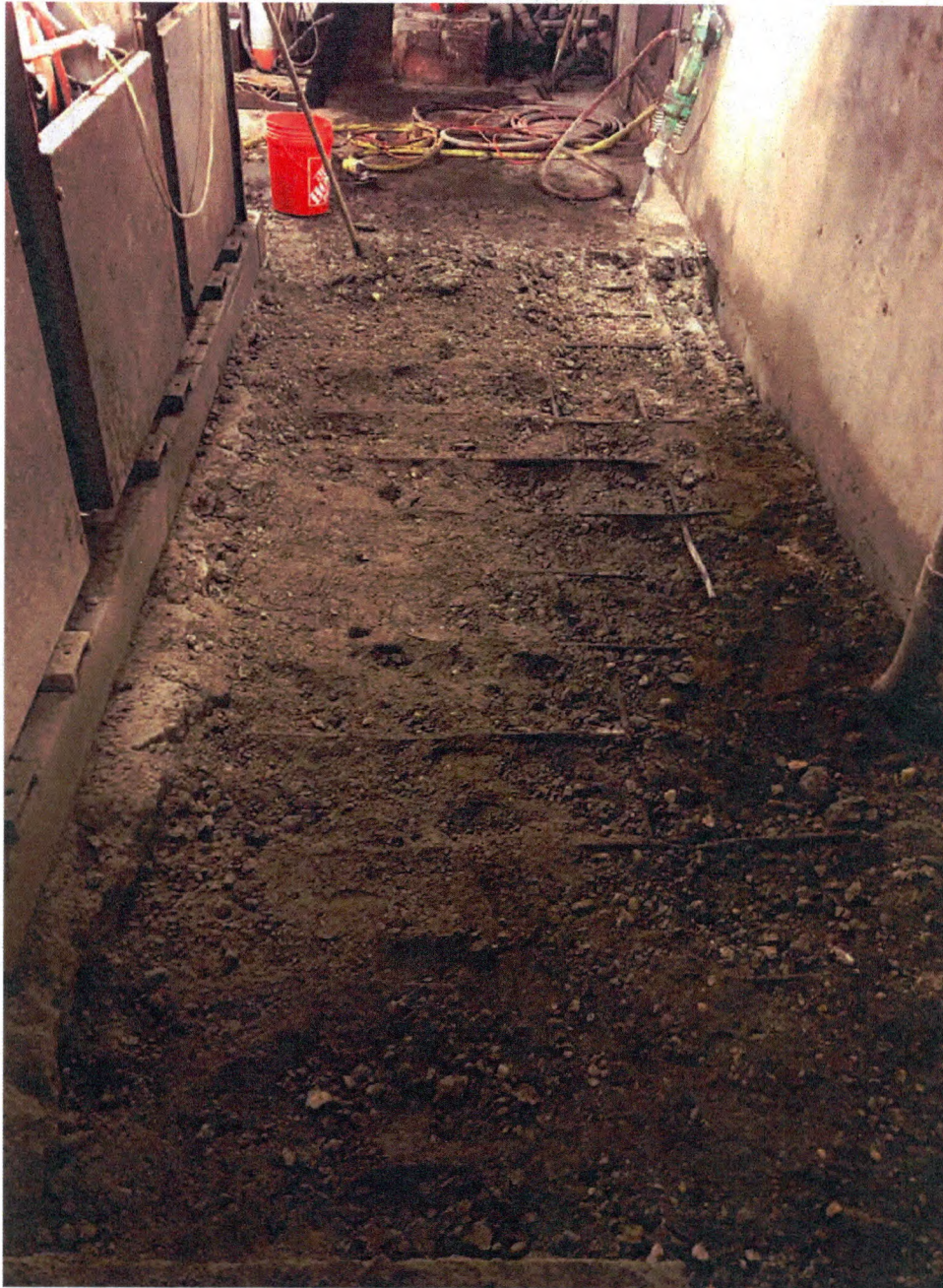
Full-Scale PCB-Impacted Concrete Removal via Jackhammers
