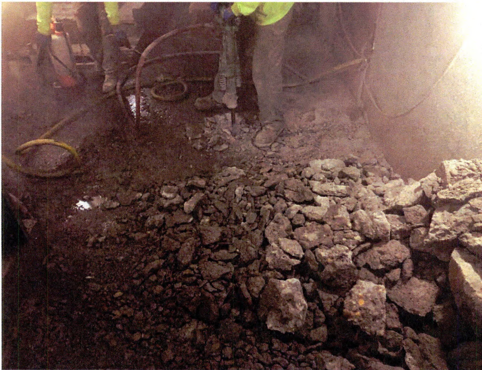
Full-Scale PCB-Impacted Concrete Removal via Jackhammers
