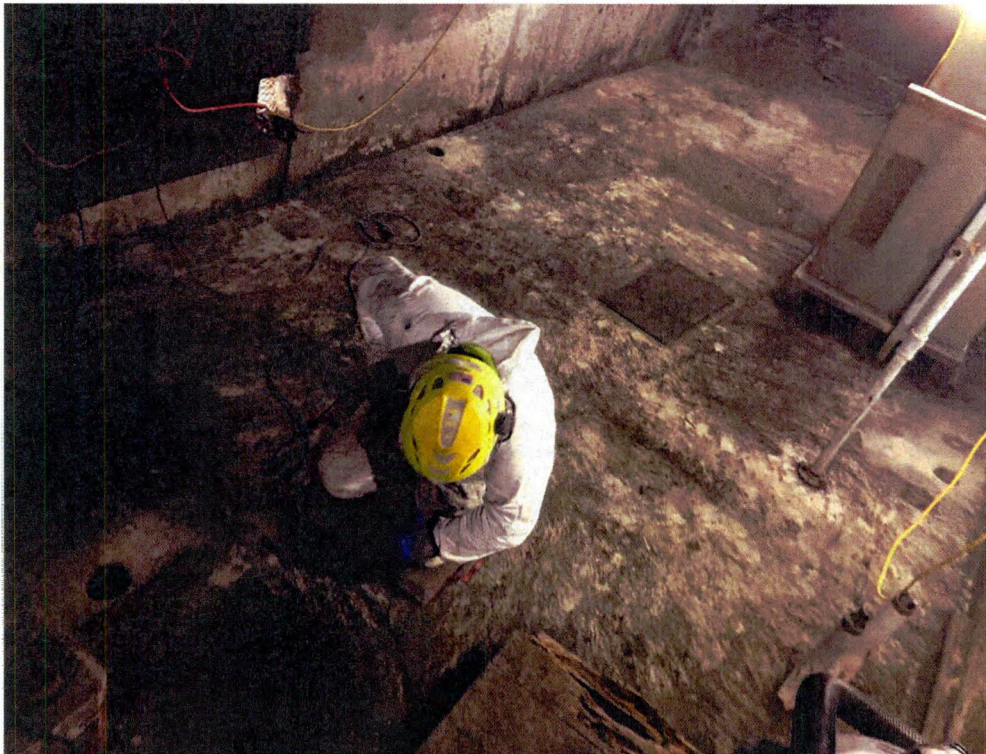
Limited PCB-Impacted Concrete Removal via Chipping Gun
