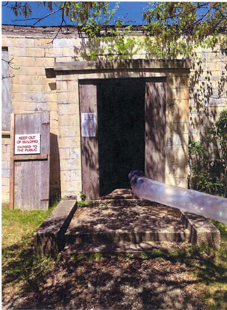
Negative Air Containment Asbestos Abatement
