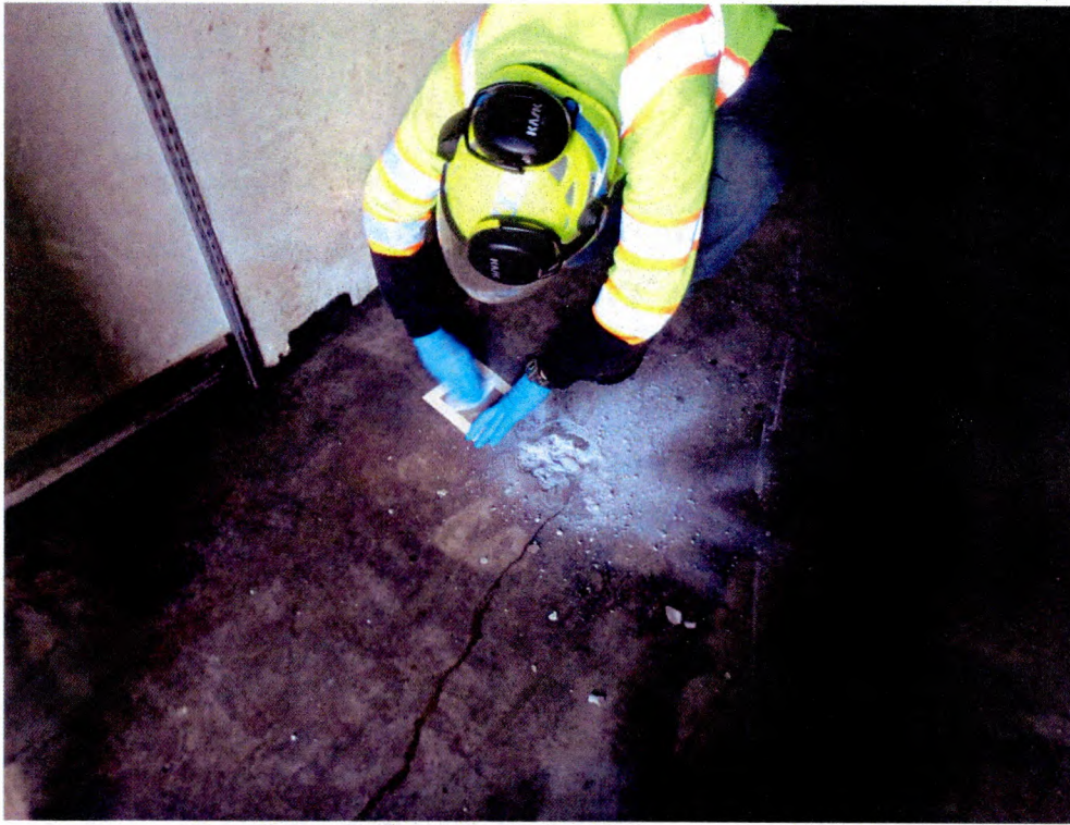
Concrete Chip and Wipe Sampling HAZMAT Removal Area
