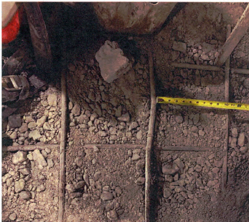
10" x 10" Rebar Observed in Battery #113 Concrete
