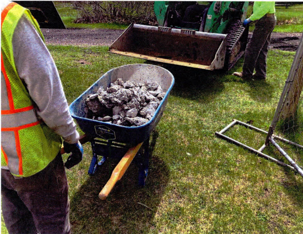
Loading PCB-Impacted Concrete for Disposal
