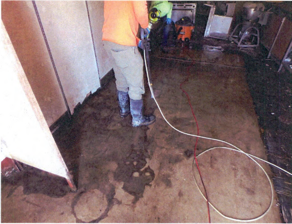
Pressure Washing Stained Concrete Floors
