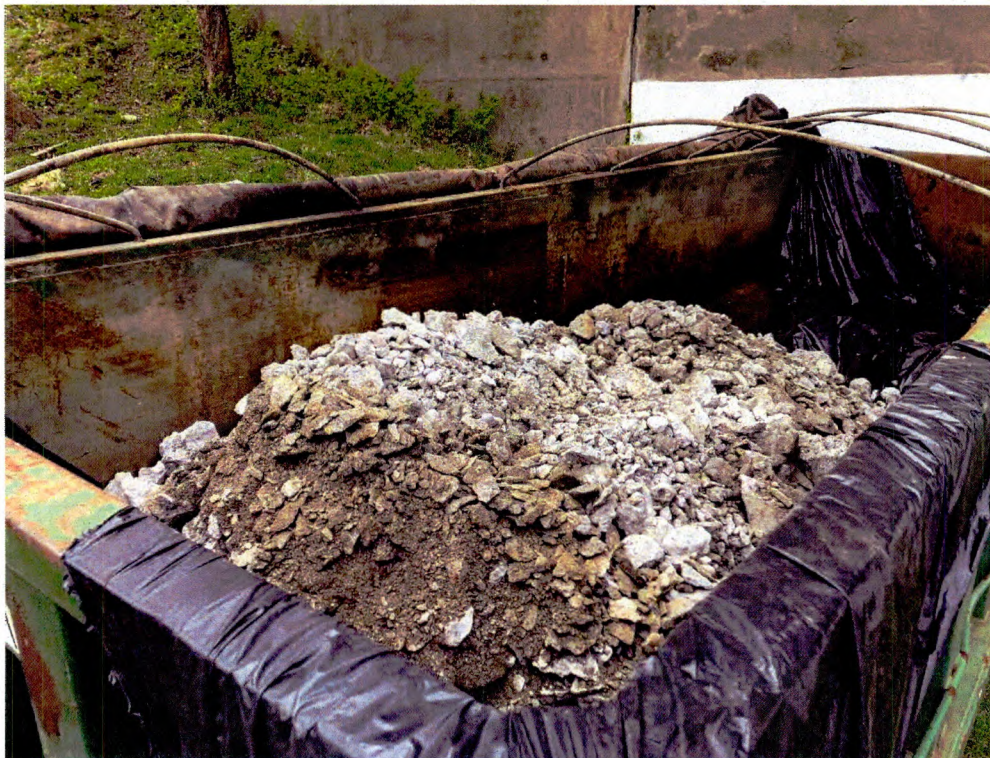
PCB-Impacted Concrete Spoils Prepared for Proper Disposal
