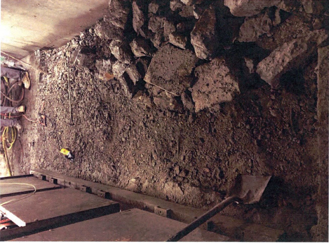
Full-Scale PCB-Impacted Concrete Removal via Jackhammers
