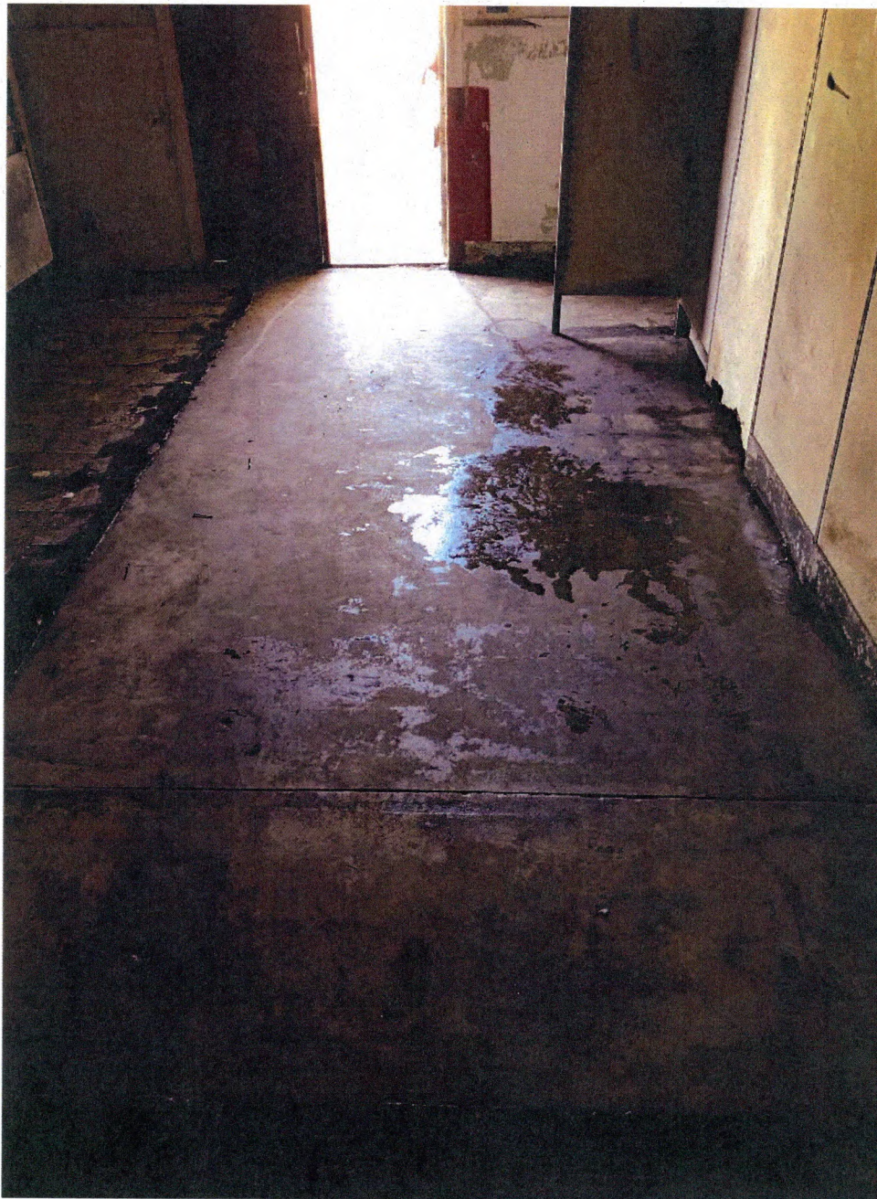
Stained Floor Abated of ACM Tiles
