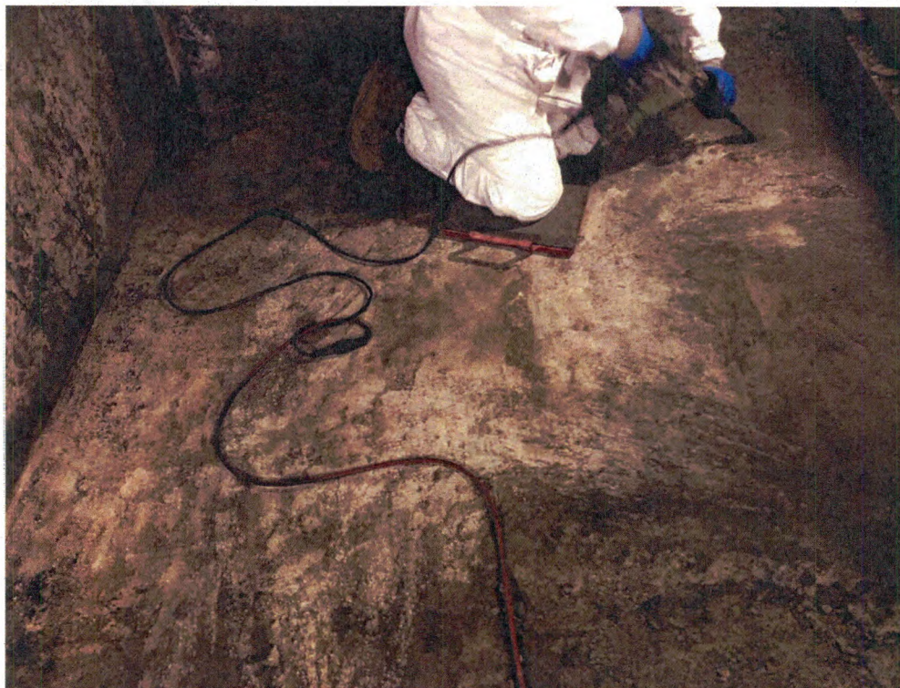
Limited PCB-Impacted Concrete Removal via Chipping Gun
