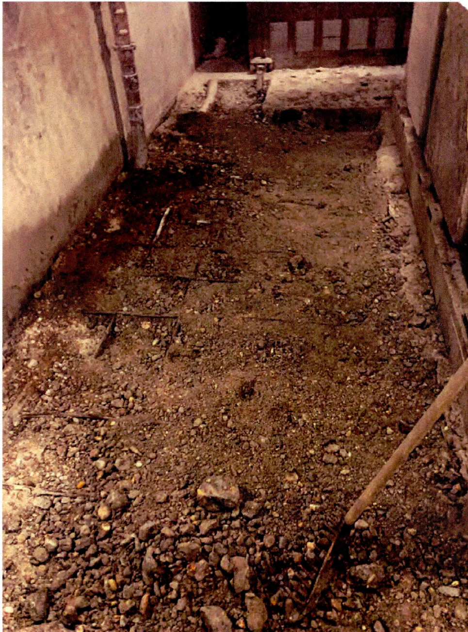
Full-Scale PCB-Impacted Concrete Removal via Jackhammers
