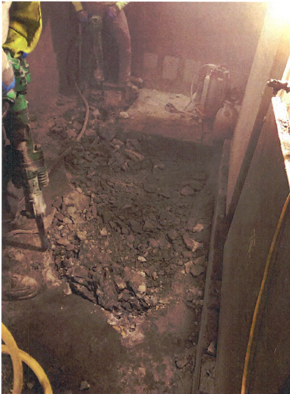
Full-Scale PCB-Impacted Concrete Removal via Jackhammers
