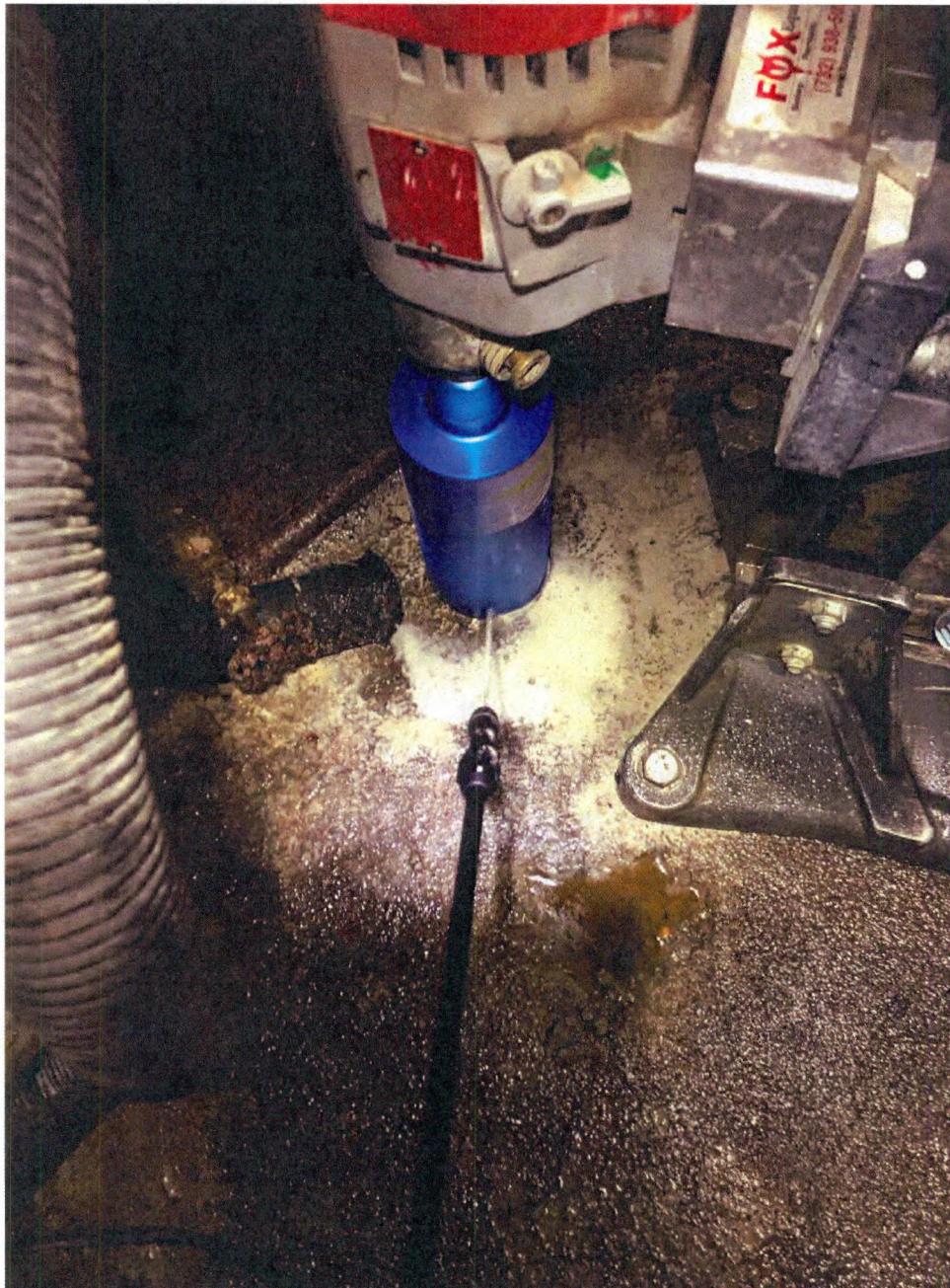
Concrete Sampling via Core Drill with Continuous Mist and HEPA Vacuum
