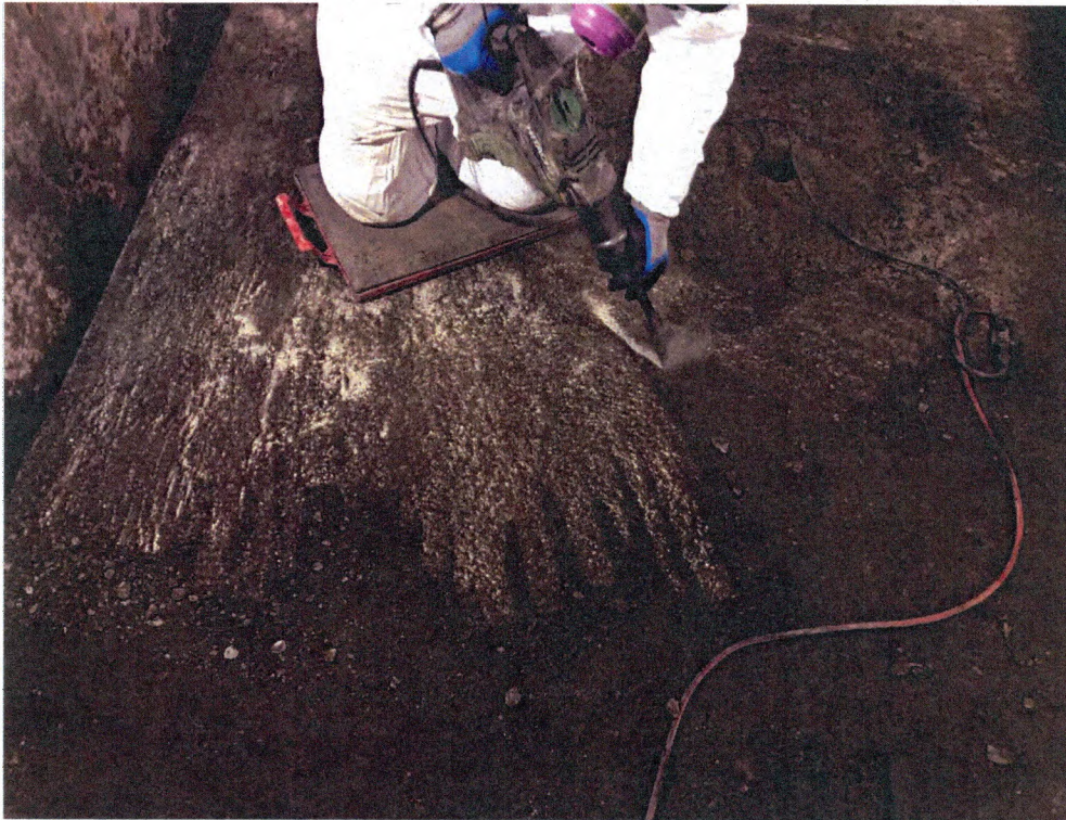
Limited PCB-Impacted Concrete Removal via Chipping Gun
