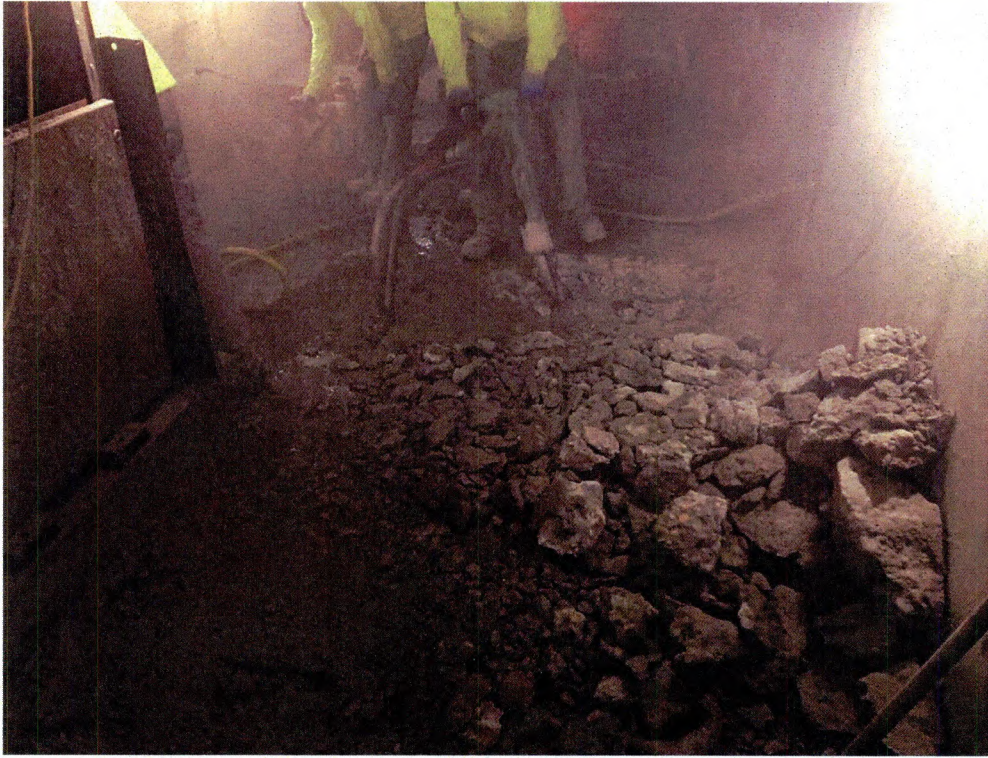
Full-Scale PCB-Impacted Concrete Removal via Jackhammers
