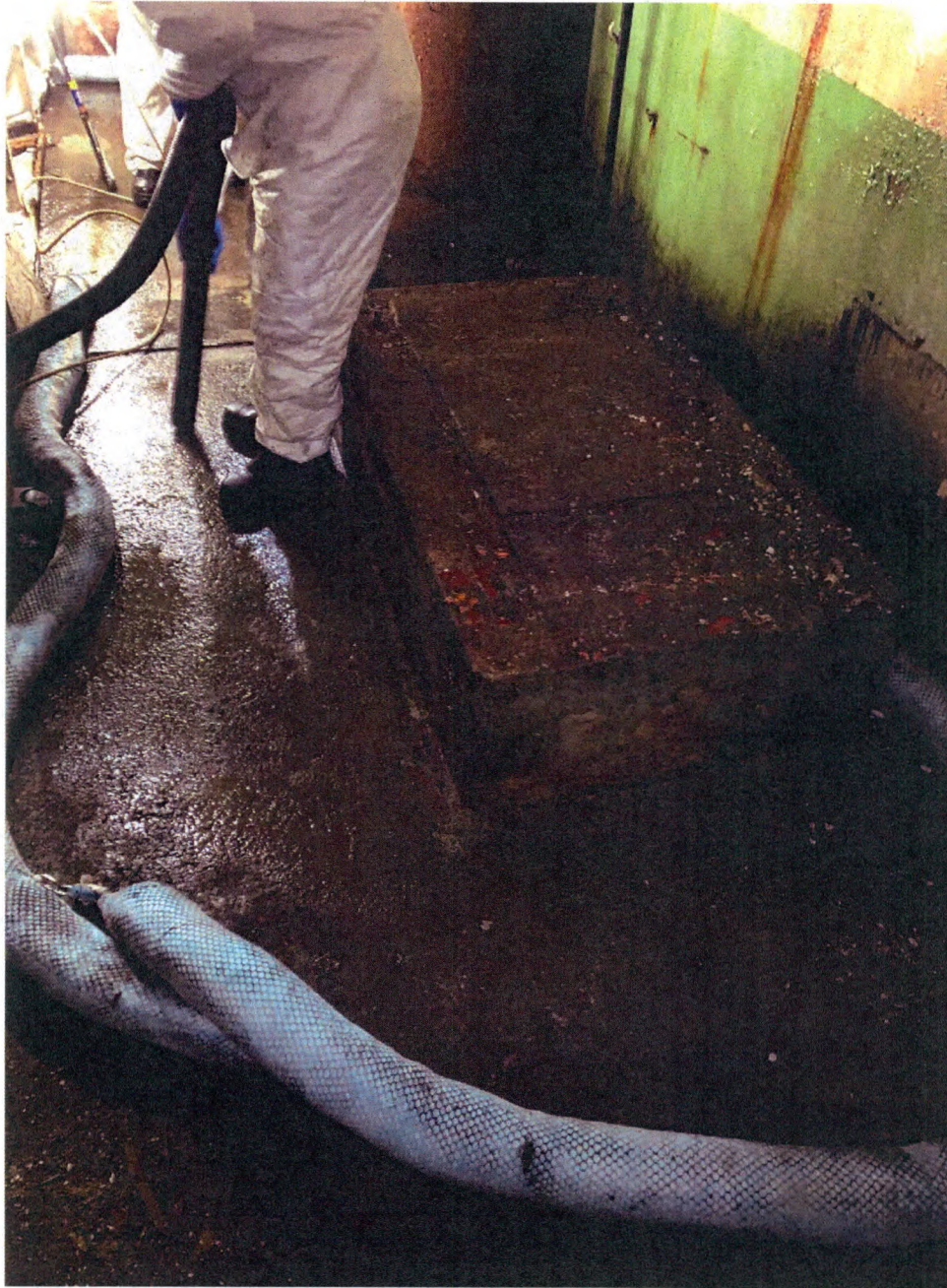
Cleaning and Pressure Washing AST Removal Area
