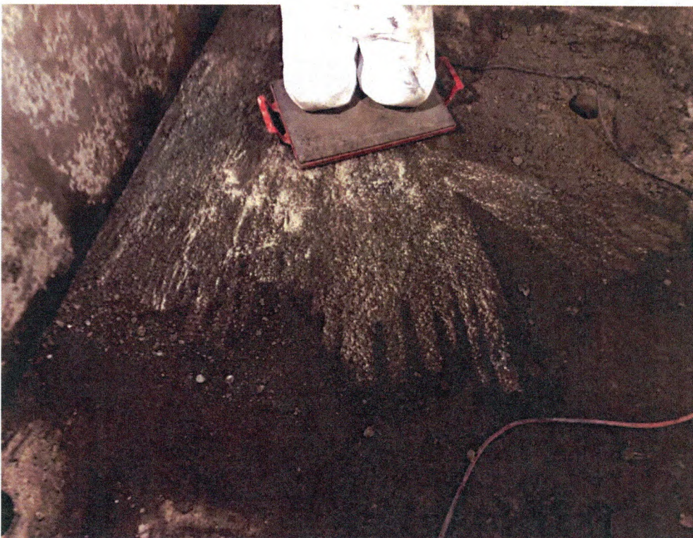
Limited PCB-Impacted Concrete Removal via Chipping Gun
