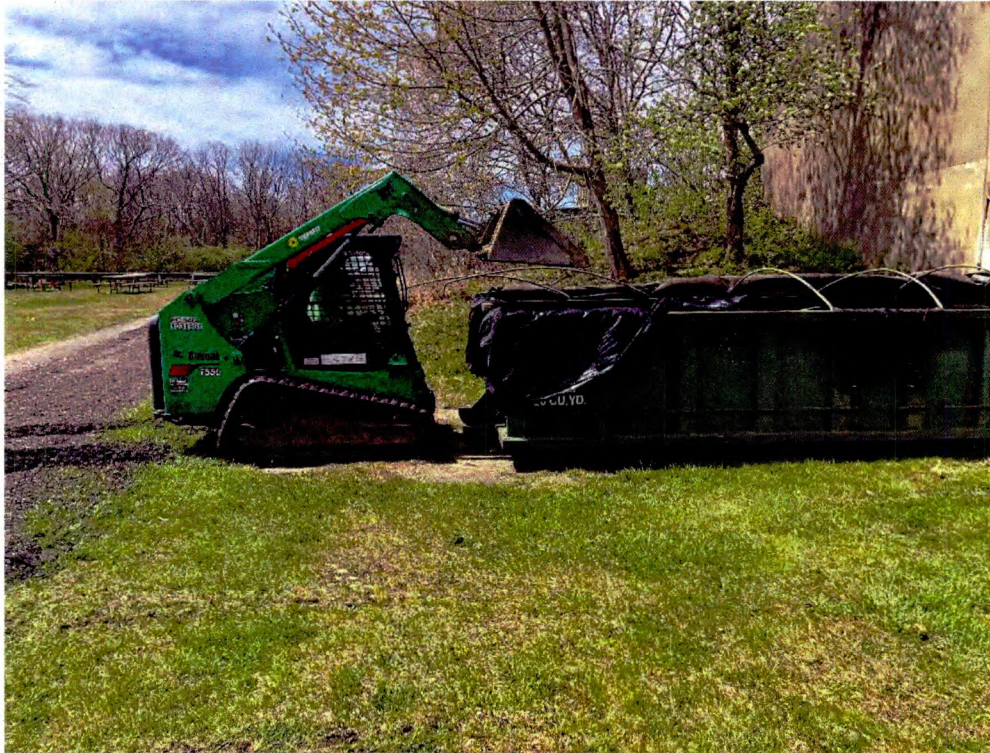
Loading PCB-Impacted Concrete for Disposal
