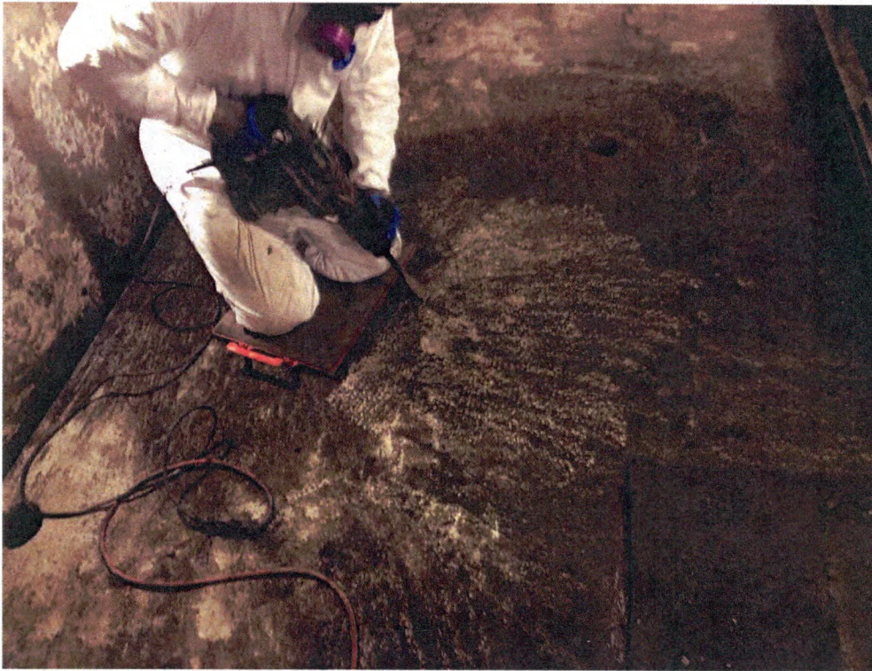
Limited PCB-Impacted Concrete Removal via Chipping Gun
