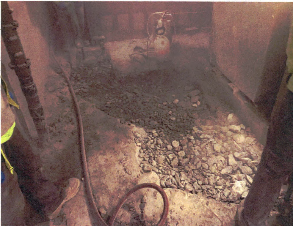
Full-Scale PCB-Impacted Concrete Removal via Jackhammers
