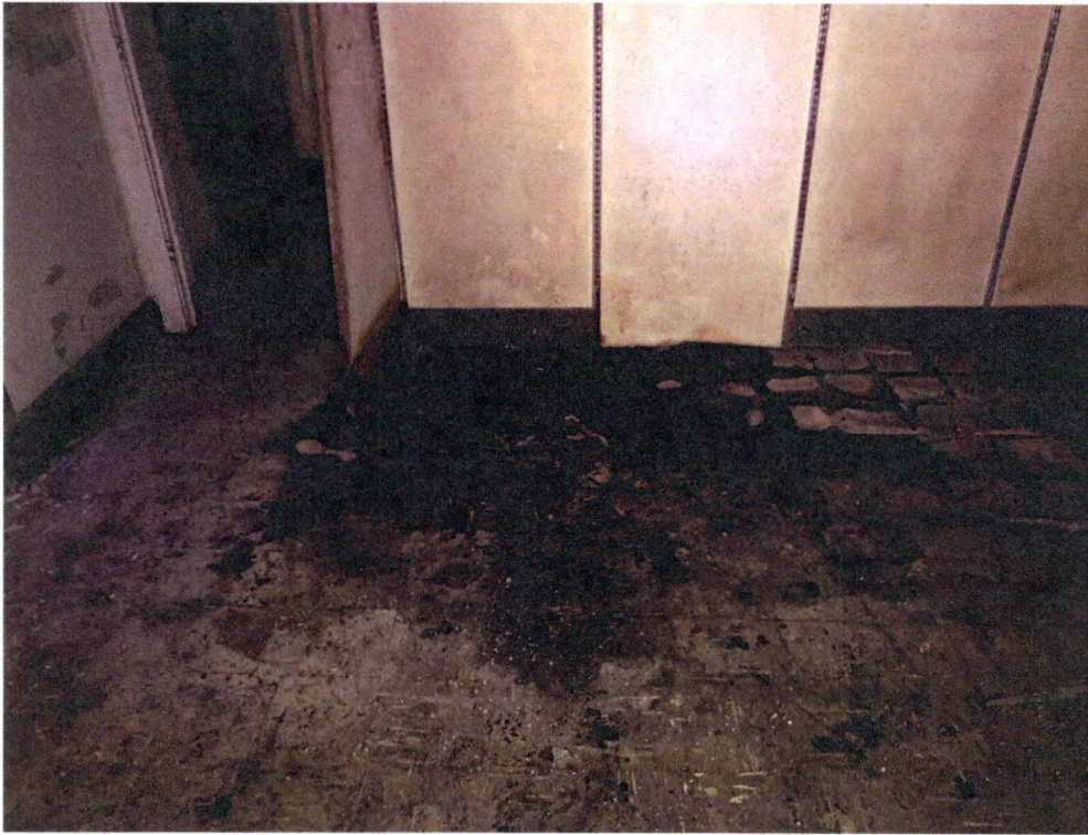
Tile Staining below HAZMAT Stockpile
