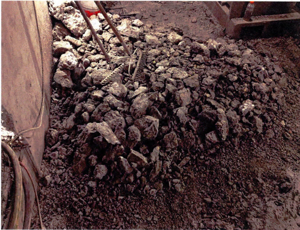
PCB-Impacted Concrete Stockpile
