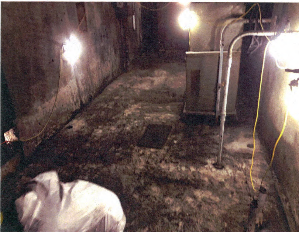
Limited PCB-Impacted Concrete Removal via Chipping Gun
