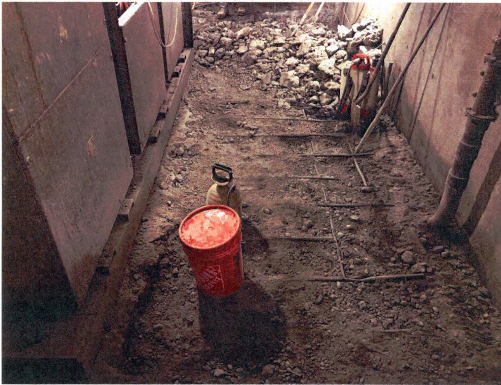
Full-Scale PCB-Impacted Concrete Removal via Jackhammers
