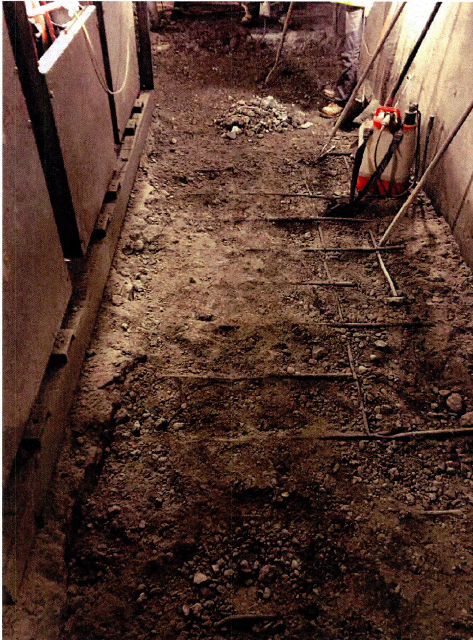
Full-Scale PCB-Impacted Concrete Removal Area
