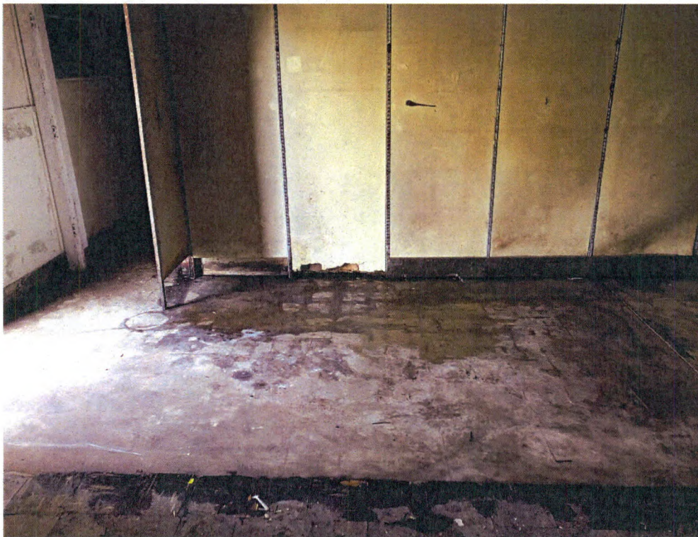
Stained Floor Abated of Asbestos-Containing-Material (ACM) Tiles
