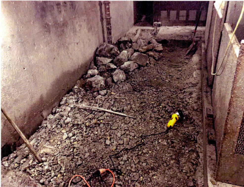
Full-Scale PCB-Impacted Concrete Removal via Jackhammers
