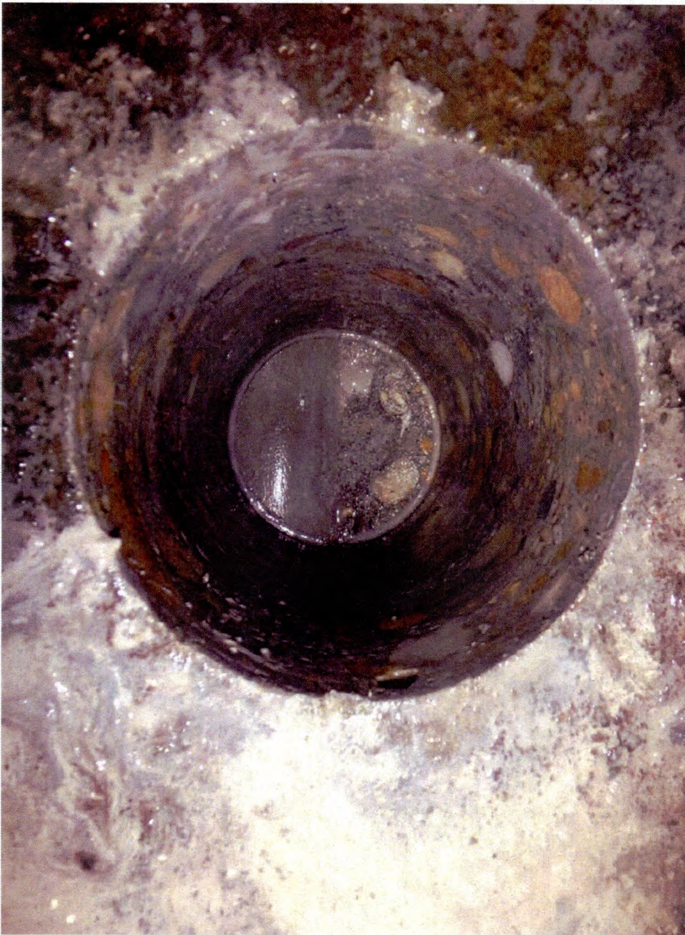
Aggregate Reinforcement Observed in Battery #113 Concrete
