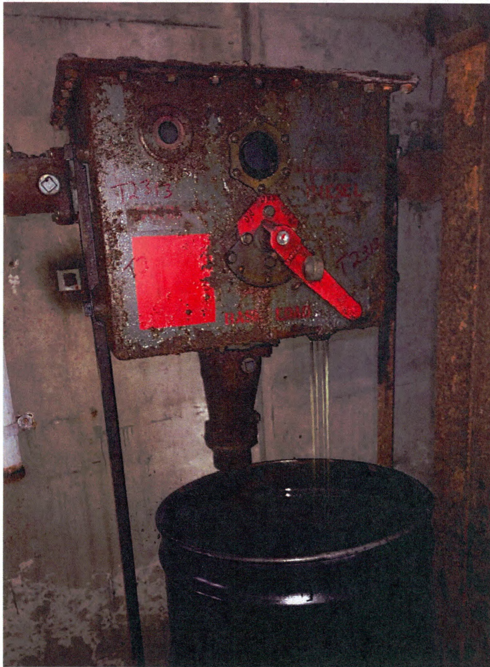
Removal of PCB-Fluids from Transformer T2313
