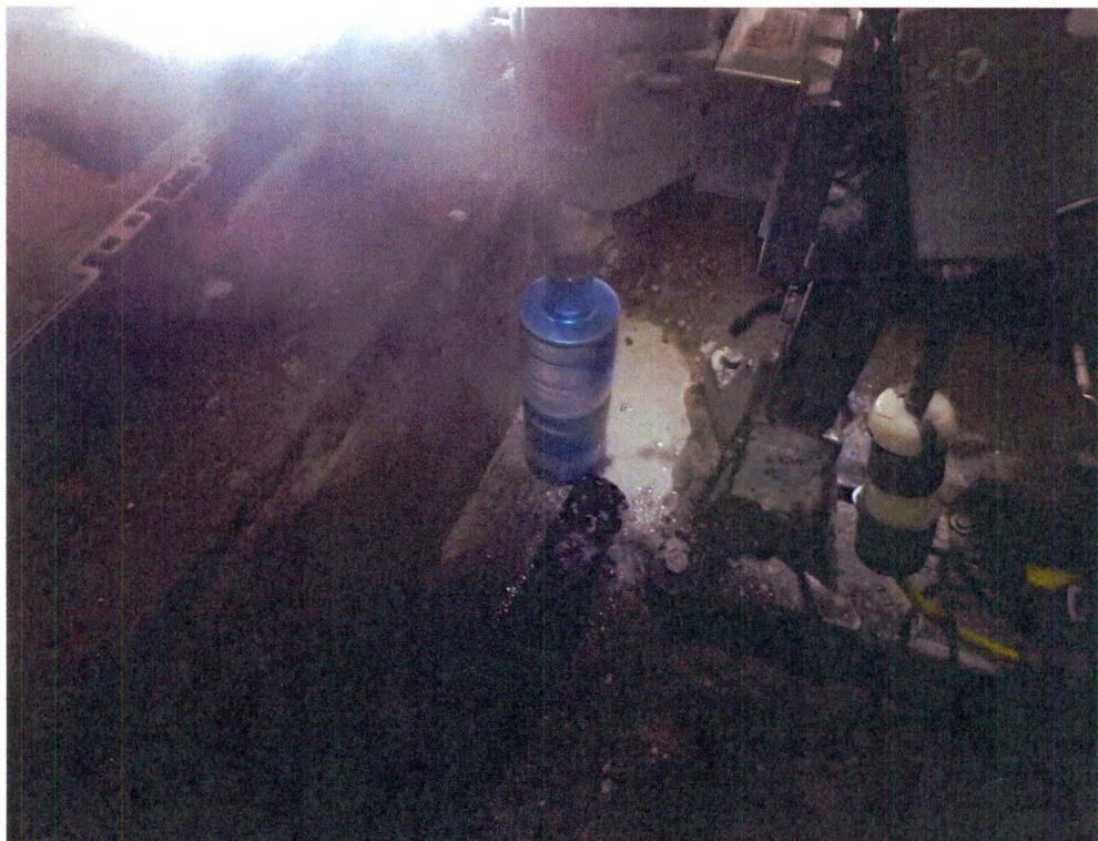
Concrete Sampling via Core Drill with Continuous Mist and HEPA Vacuum
