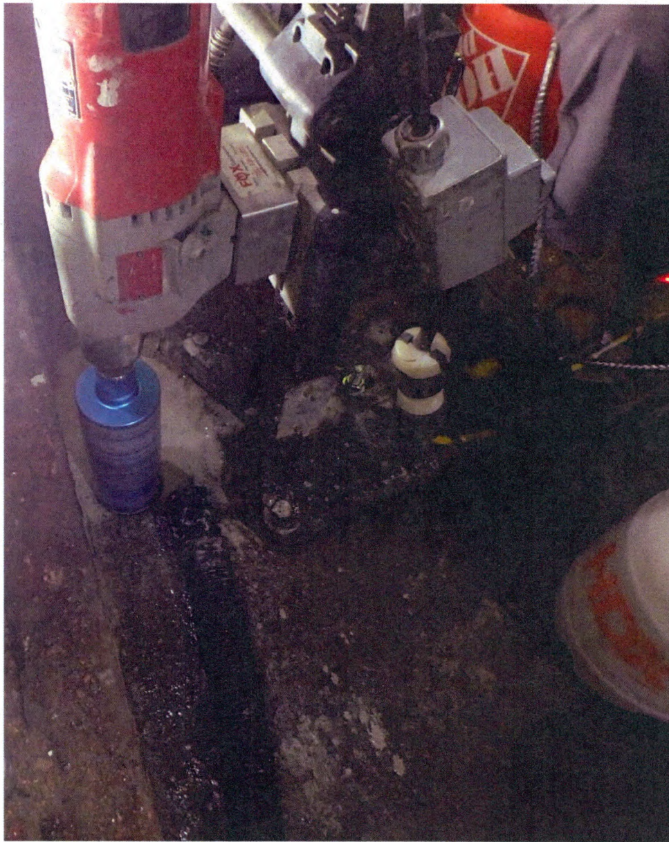
Concrete Sampling via Core Drill with Continuous Mist and HEPA Vacuum
