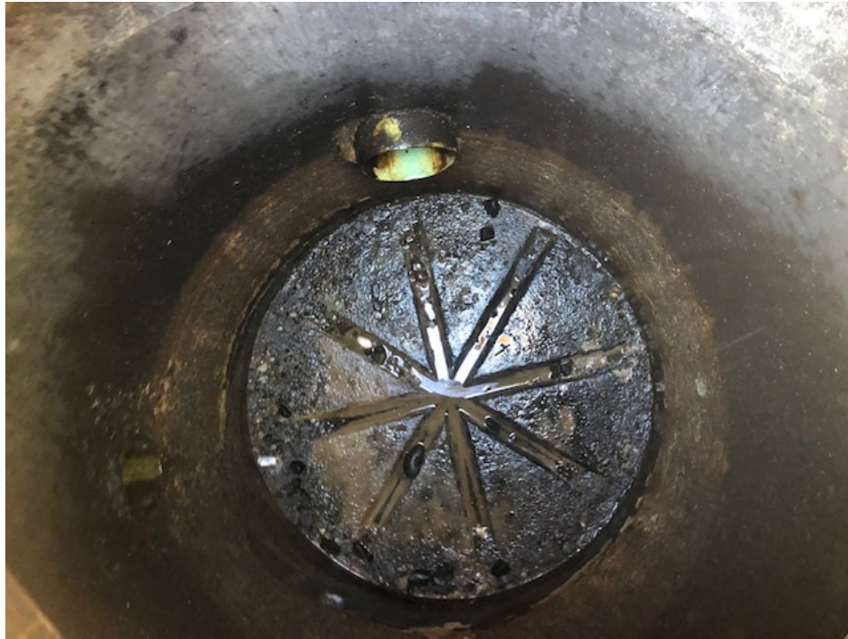
Photo 1: Typical Solid Bottom Structure Post Remediation
