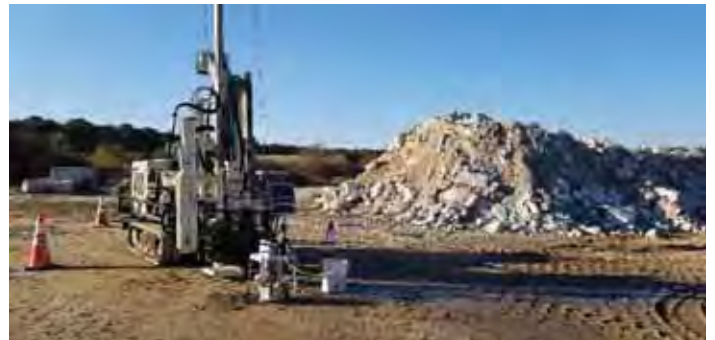
Geoprobe rig set-up, surrounded by construction cones.
