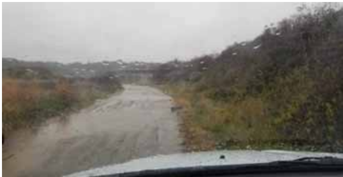
Flooding on the site path, caused by excessive rain.
