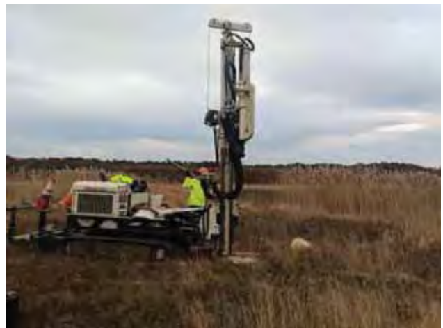
Geoprobe rig set up at GS/GW-2.
