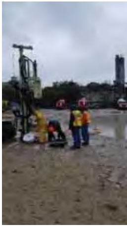
Geoprobe rig set-up at GS/GW-7.
