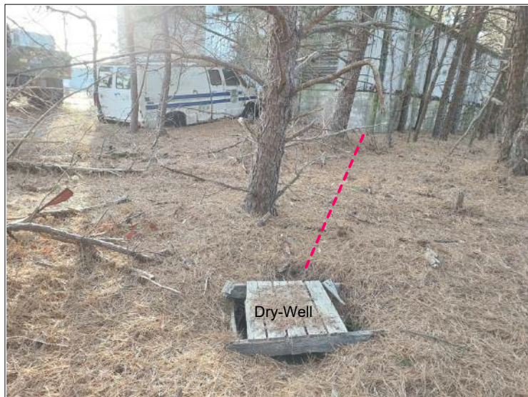
Photo showing the location of the observed piping running between the dry-well and the building. Building 206
