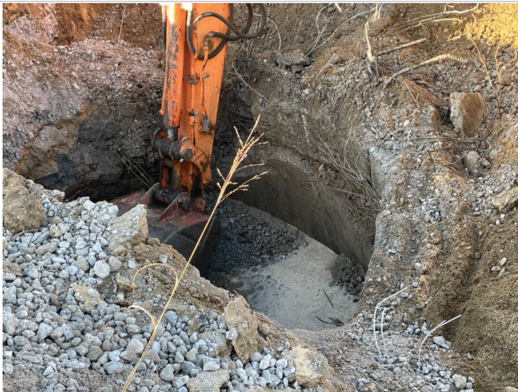
Burn Pit Excavation
