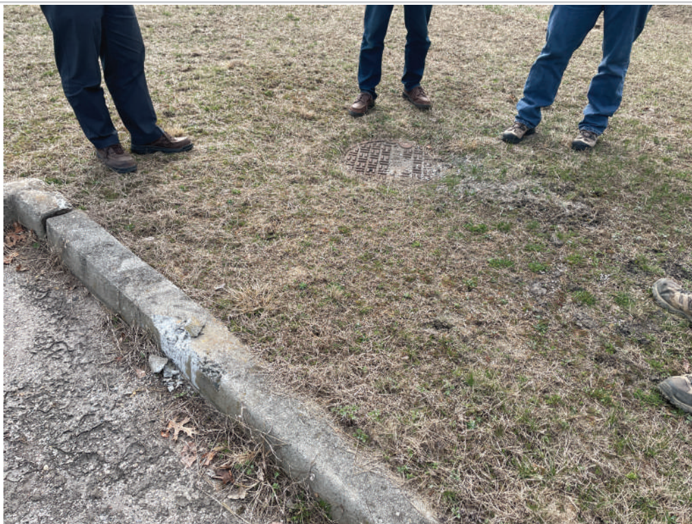
Storm Drain S-2
