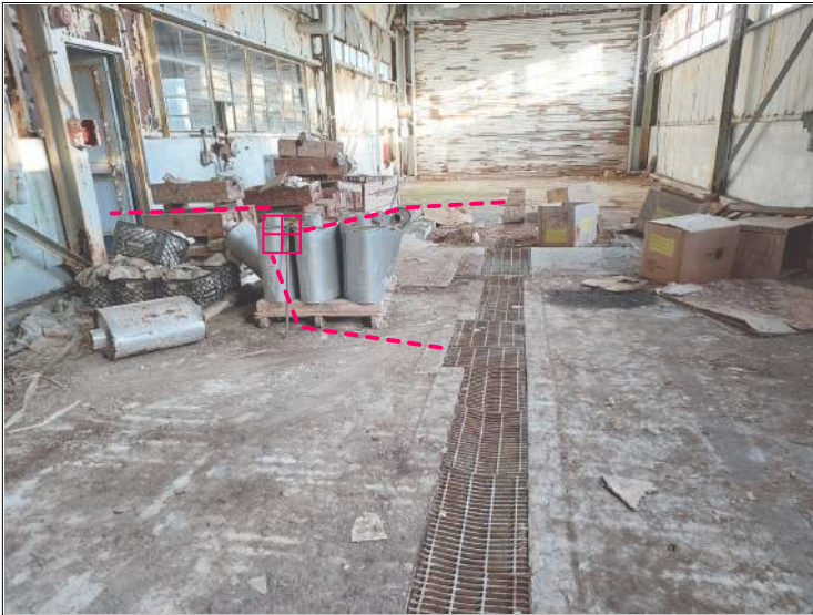
Photo showing the location of the observed piping running east through a catch basin, into the next room. Building 216
