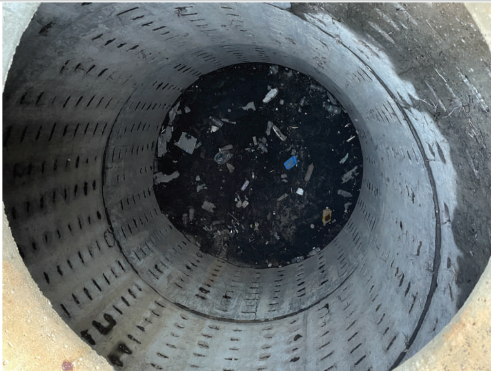
Storm Drain S-2 Interior
